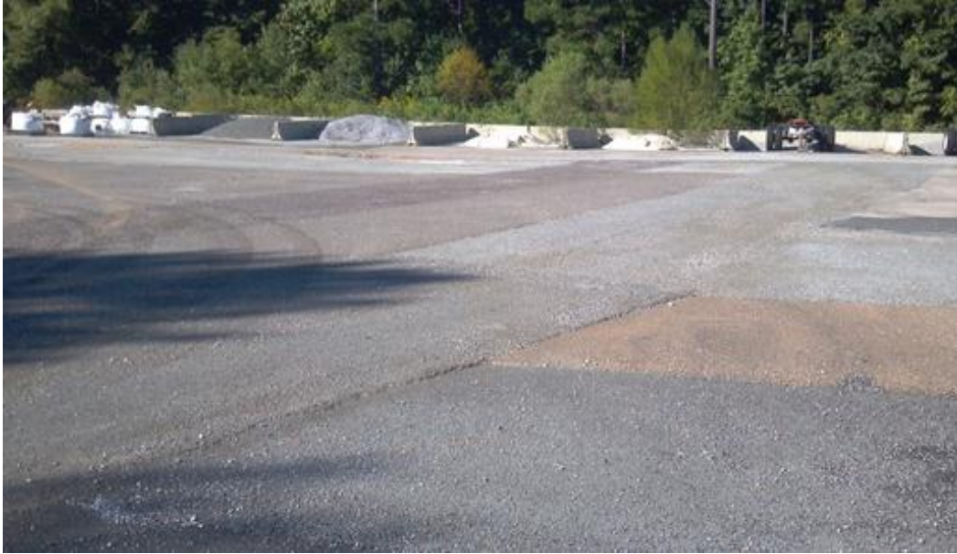
Figure B.3 – Rough Asphalt terrain
