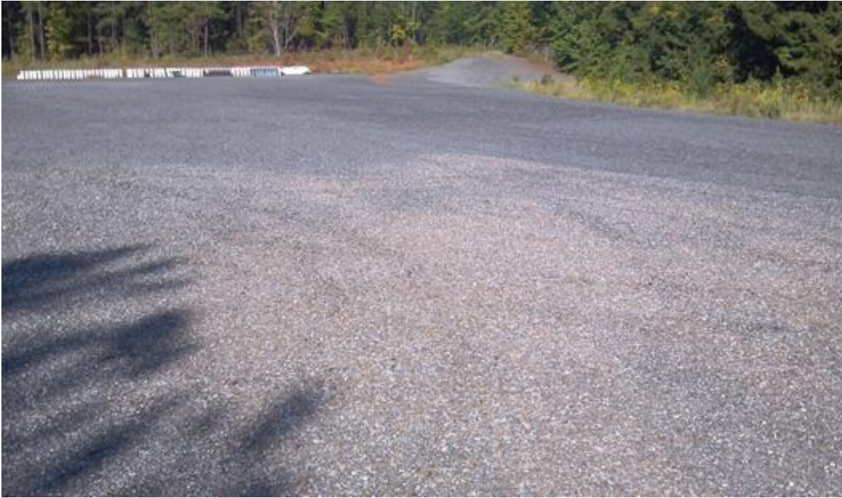
Figure B.4 – Packed Gravel terrain
