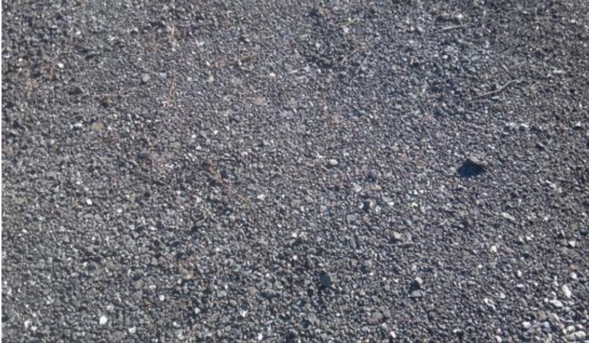
Figure B.6 – Packed Gravel terrain
