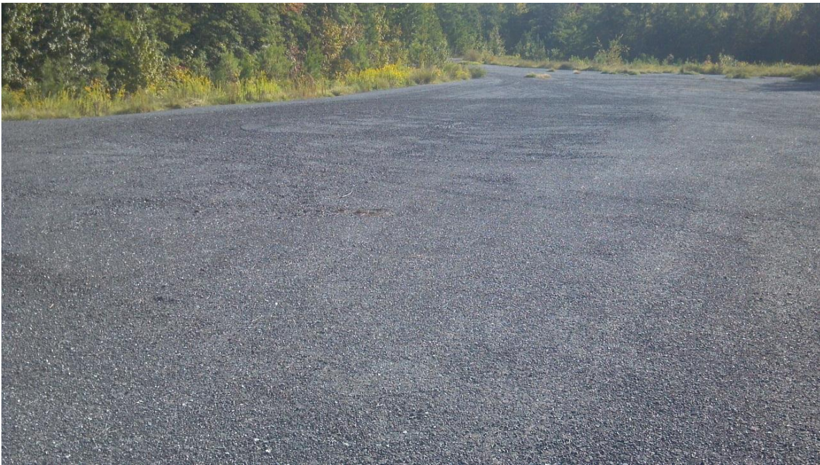
Figure B.5 – Packed Gravel terrain
