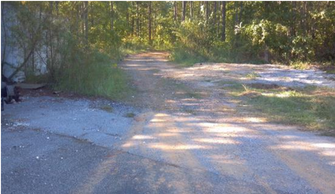
Figure B.12 – Transition from Dirt Path to Rough Asphalt
