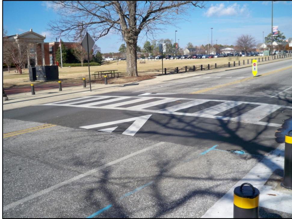
Figure 1.5 Speed Table w/Integrated Raised Pedestrian Crosswalk at Thach Pedestrian Concourse
