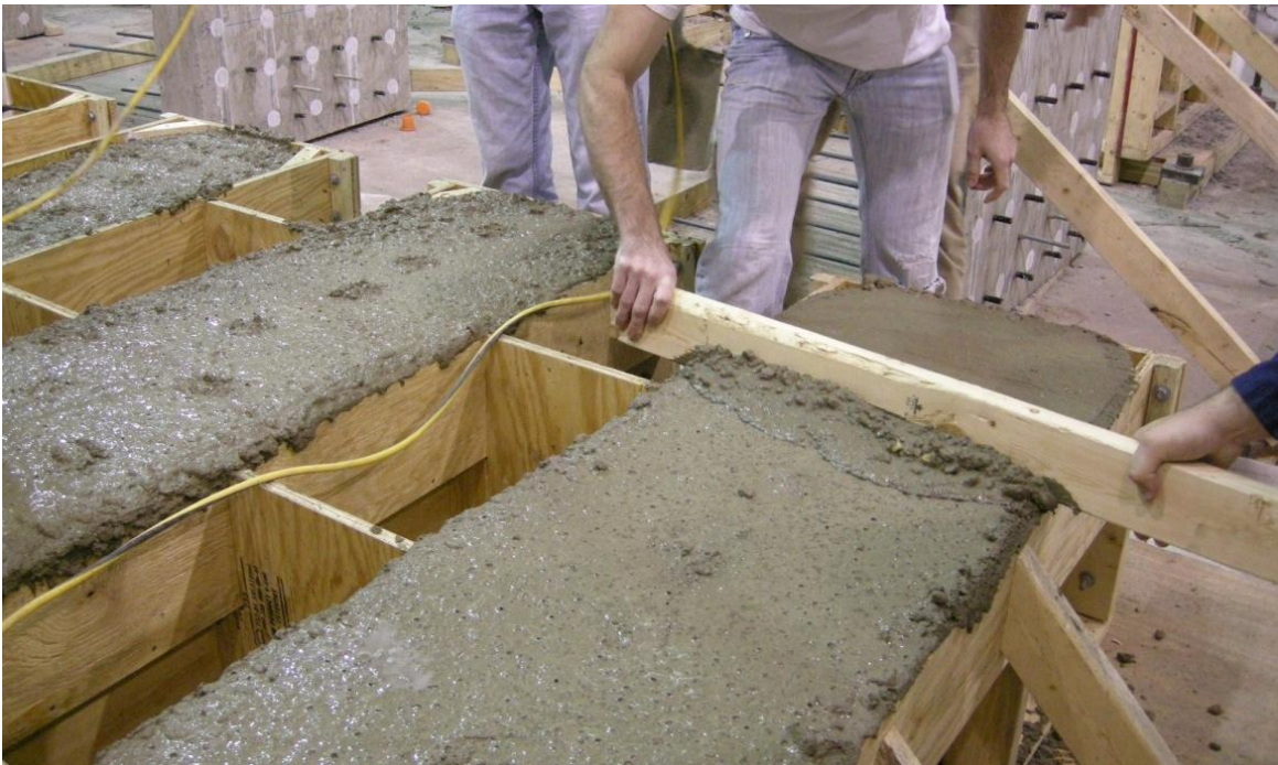
Figure 3.10 Striking of Excess Concrete
