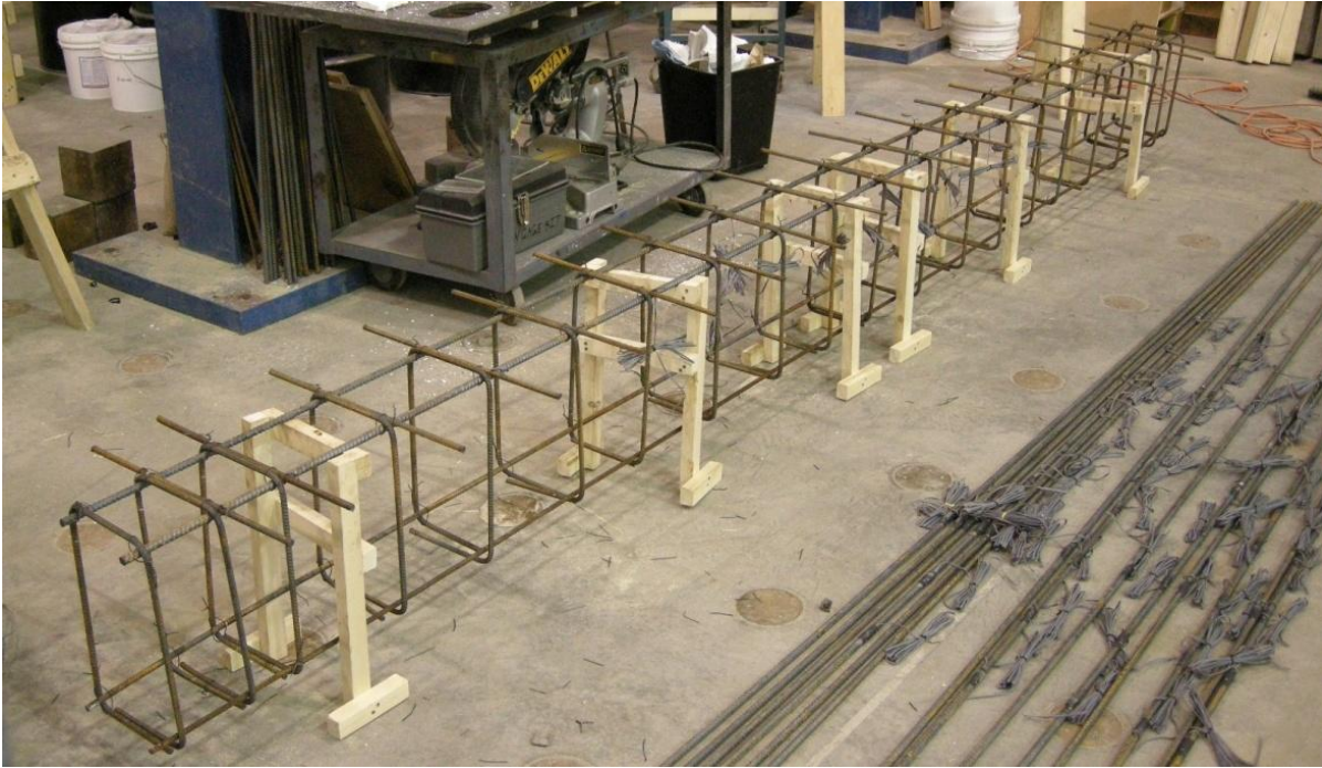
Figure 3.5 Assembled Reinforcement Cage
