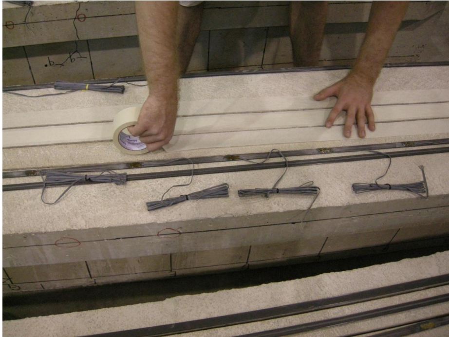
Figure 4.1 Taping of Grooves
