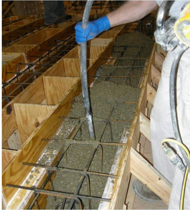
Figure 3.9 Mechanical Consolidation of Concrete
