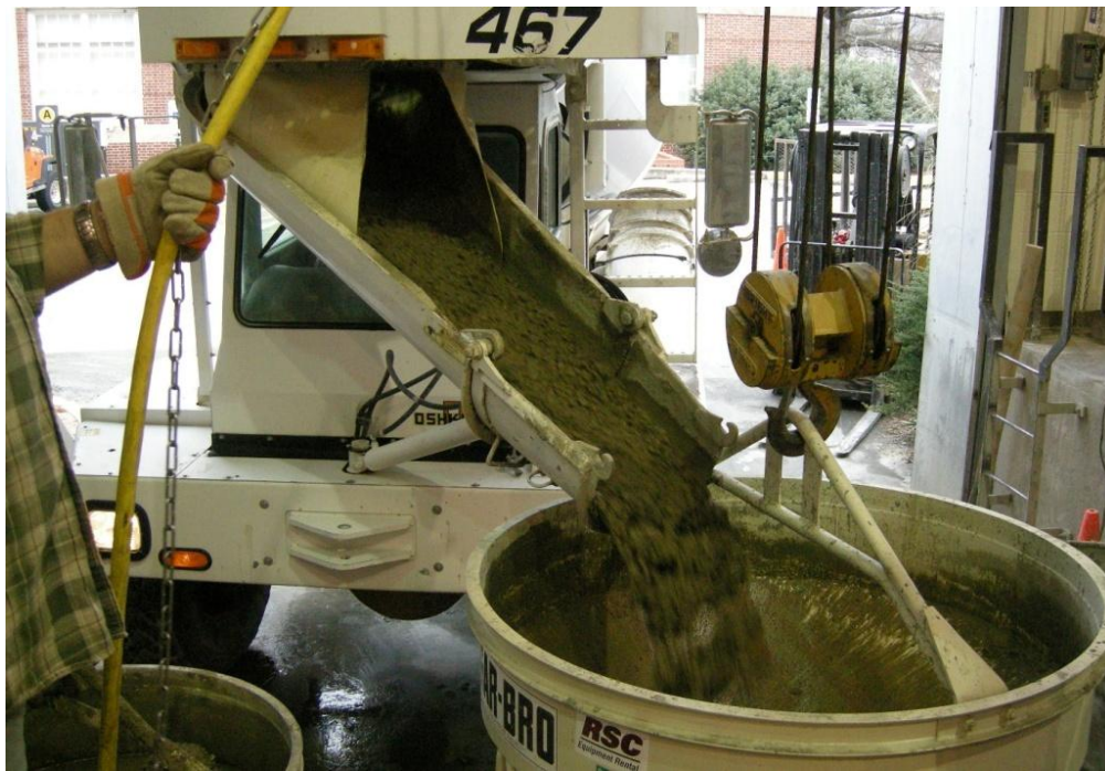
Figure 3.8 Introduction of Concrete to Crane Bucket
