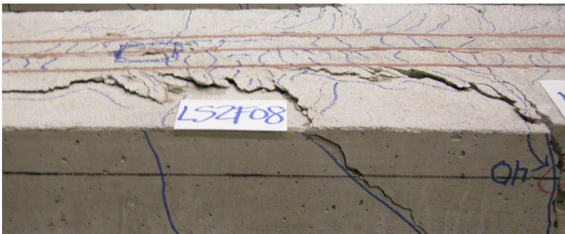
Figure 7.15 Failure Planes on Tension Face—LS2F08
