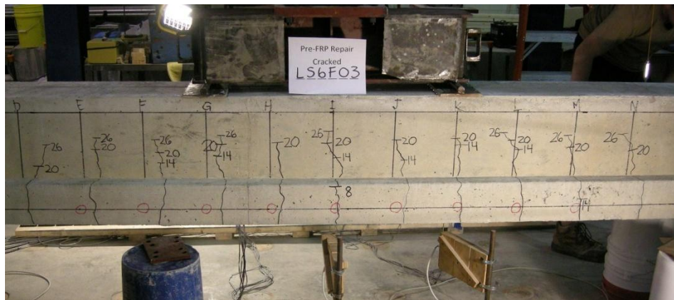
Figure 3.25 Typical Cracking Pattern for Specimens with \rho_s = 0.6\%
