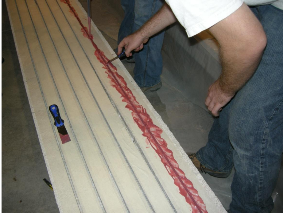
Figure 4.10 Striking Off Excess Epoxy
