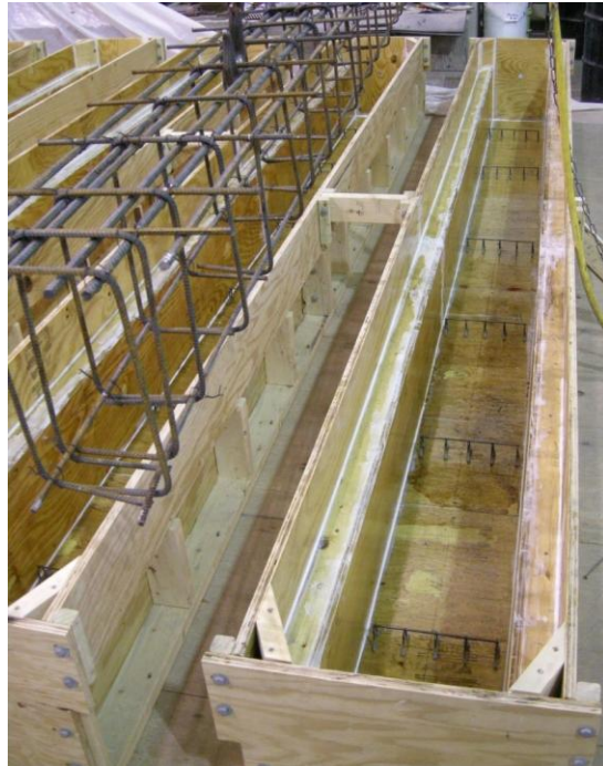
Figure 3.6 Installation of Reinforcement Cage
