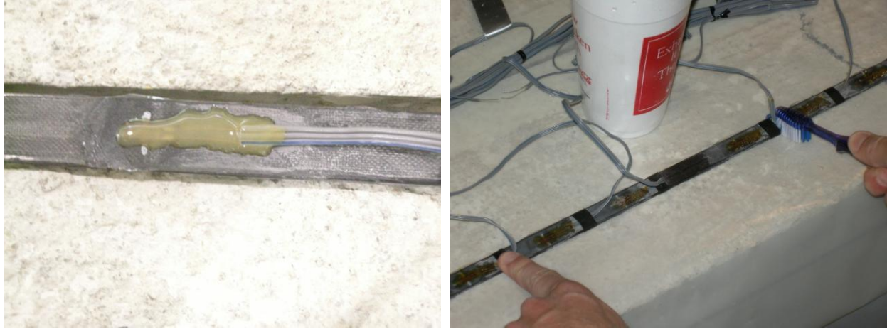
Figure 5.14 Final FRP Gage Preparation
