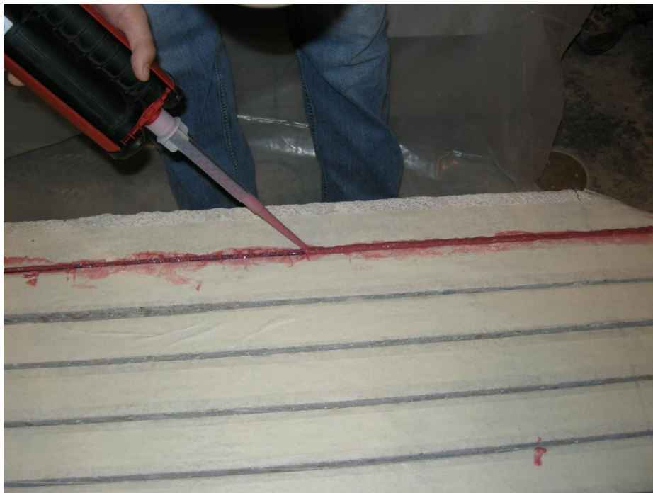
Figure 4.9 Final Application of Epoxy to Groove
