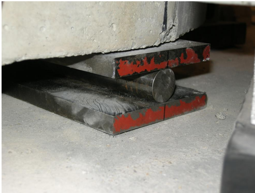
Figure 5.2 Initial Roller Assembly
