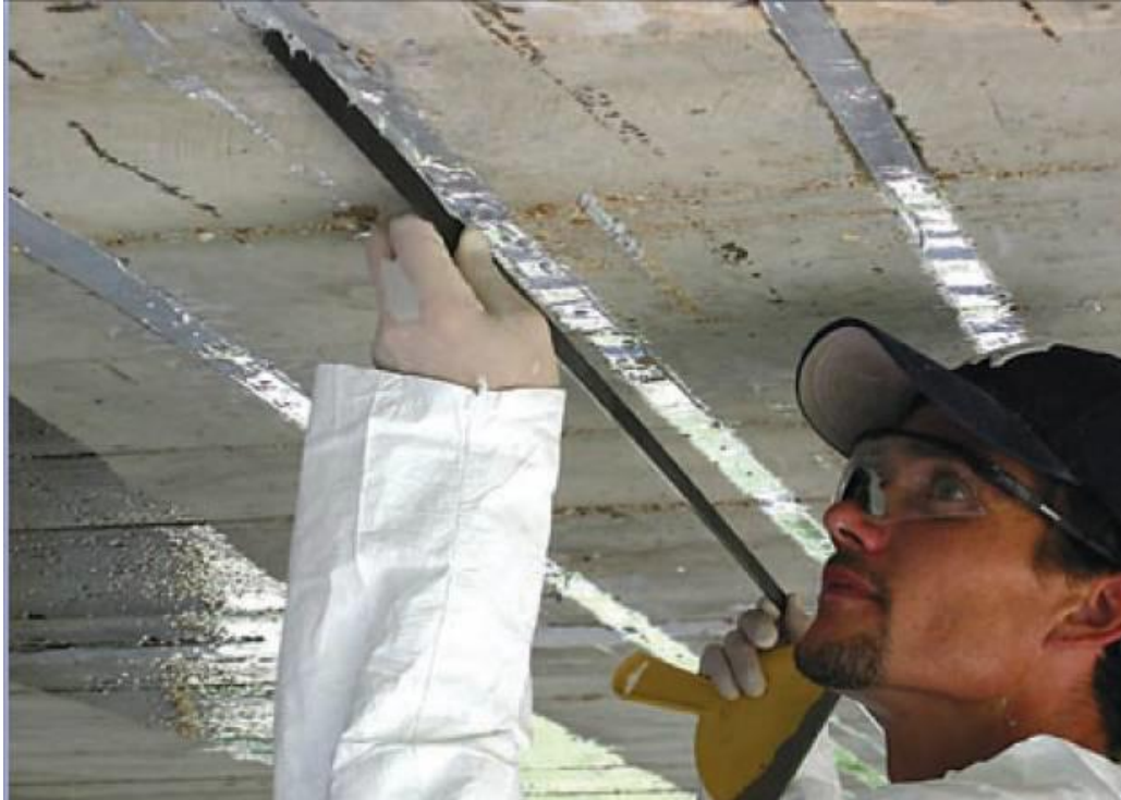
Figure 1.3 Field Installation of NSM FRP (Hughes Brothers 2011)
