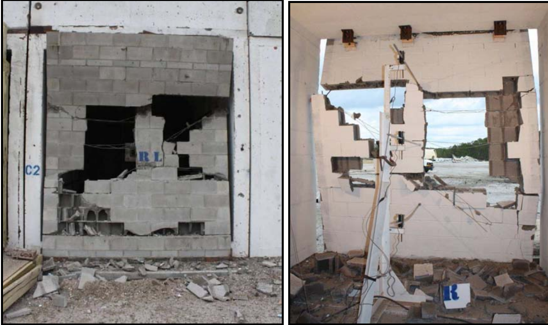
Figure 3.5. Breaching of 8-in. CMU wall after test 2
