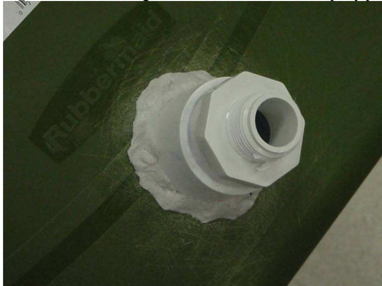
Fig. 2. Photo detailing attached drain to tub with Epoxy putty.
