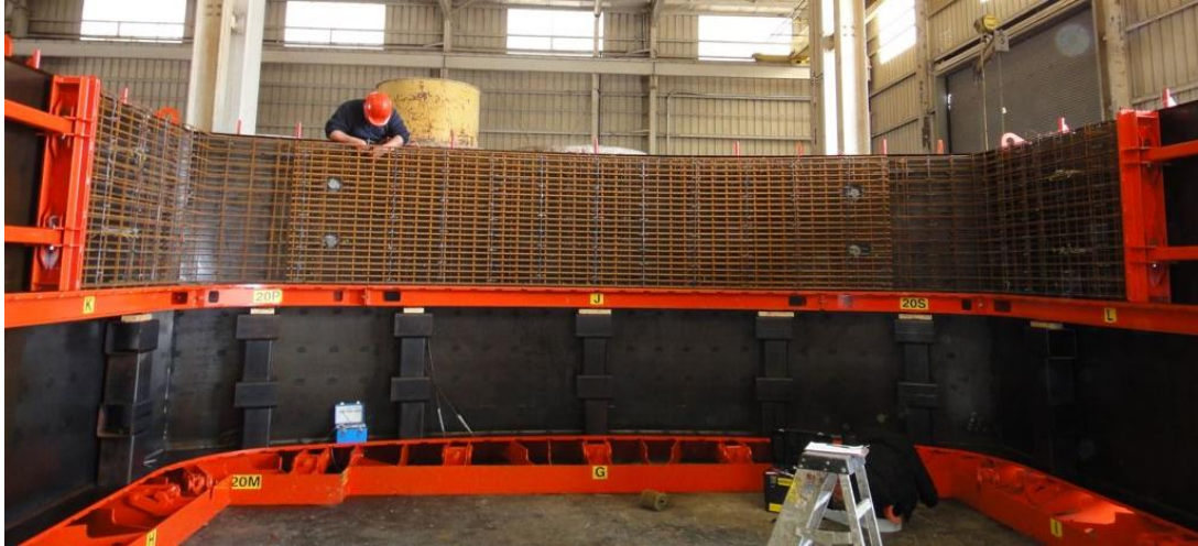
Figure 3-8: Reinforcing Cage of Precast Section Prior To Casting
