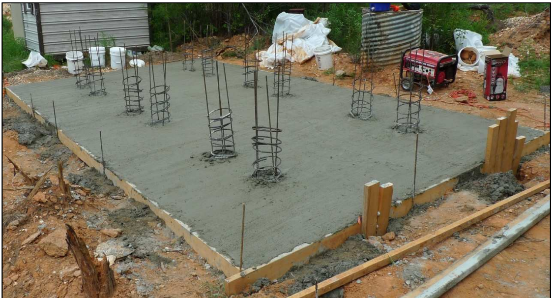
Figure 7.14: Finished strip footings and slab on grade
