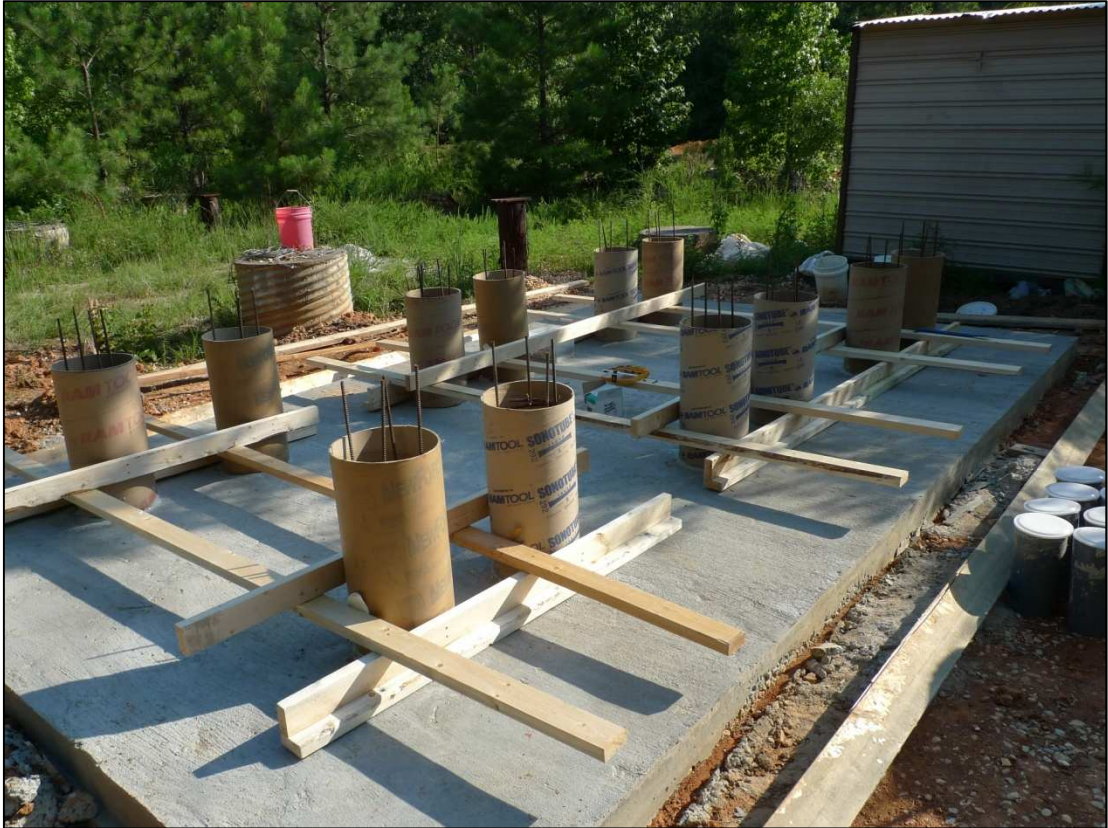
Figure 7.15: 12 inch SonoTubes column formwork
