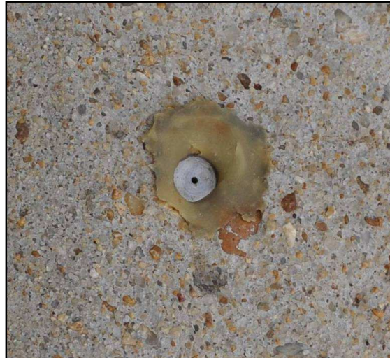
Figure 5.8: Example of installed DEMEC stud in the Bibb Graves Bridge.
