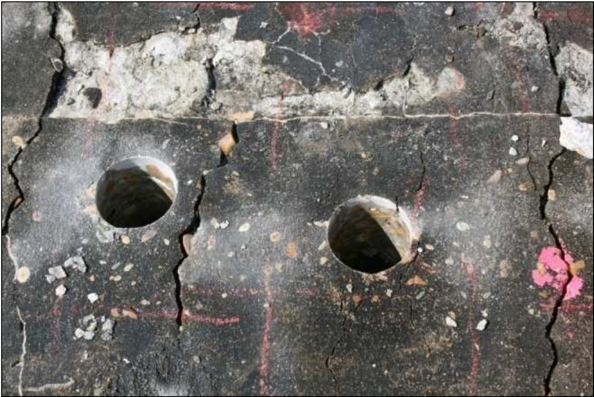
Figure A.5: Core holes left after drilling (ALDOT 2010)
