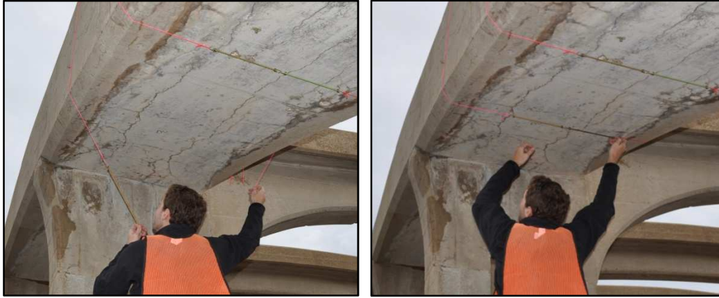
Figure 3.16: Installation of grid lines for crack survey
