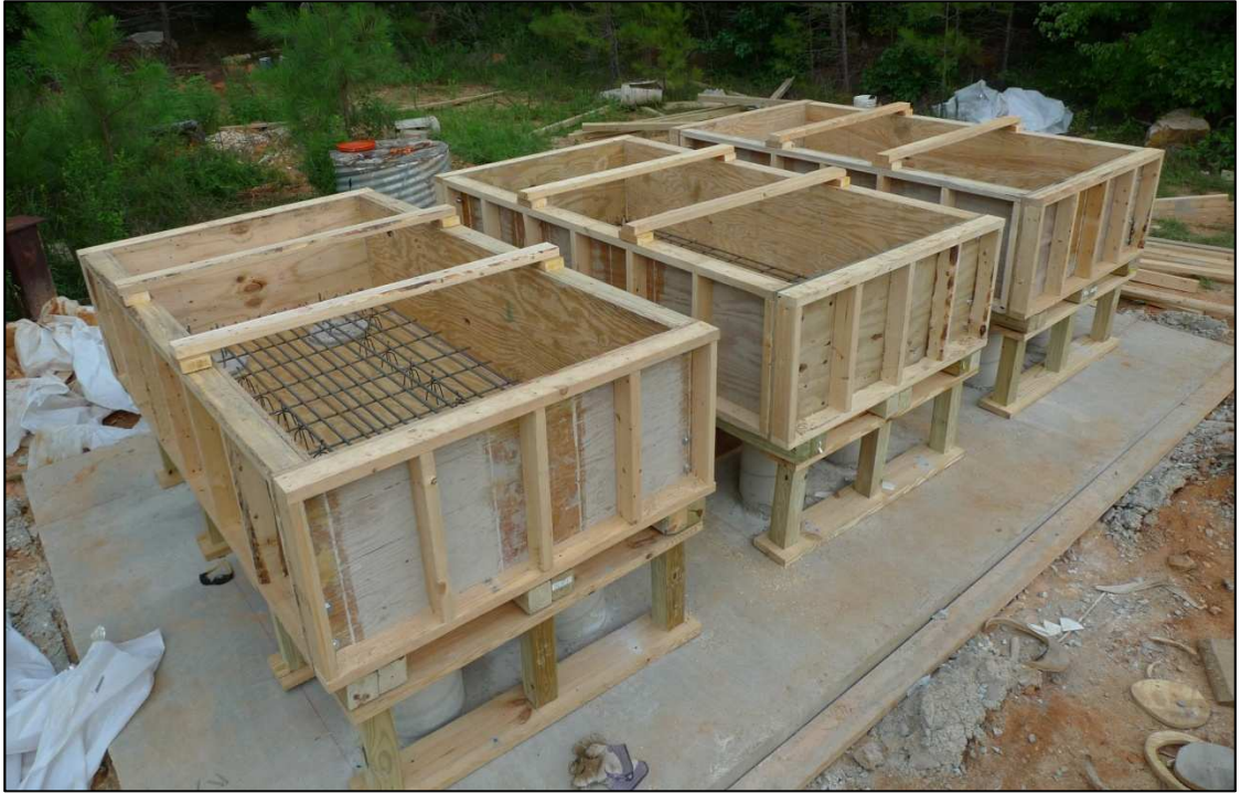
Figure 7.17: Arch test section formwork and reinforcement
