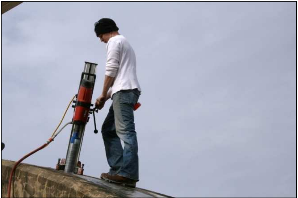
Figure A.3: Drilling for core specimen (ALDOT 2010)
