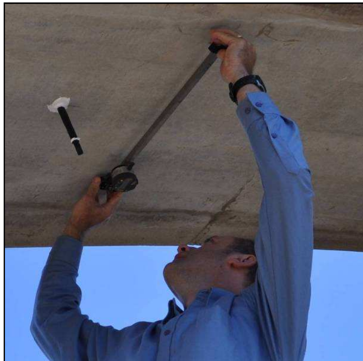
Figure 1.3: Concrete strain measurement being taken on the Bibb Graves Bridge
