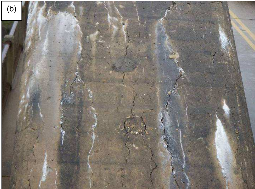
Figure 3.10: Arches on the Bibb Graves Bridge in 2010
