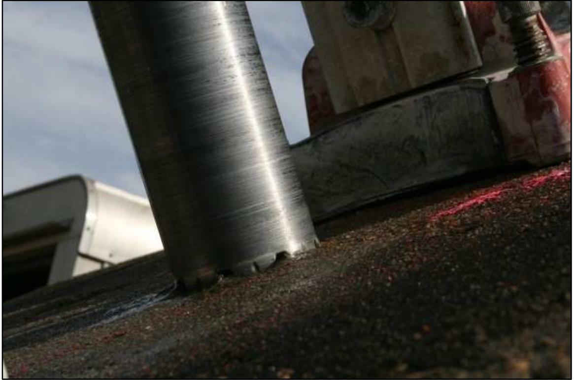
Figure A.2: Close up of drilling interface (ALDOT 2010)
