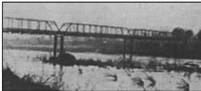
Figure 3.3: Iron bridge constructed in 1887 (Blackburn 1997)
