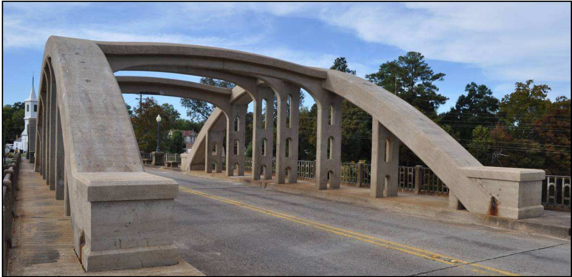
Figure 4.5: Water-blasted arches prepared for ASR mitigation procedure
