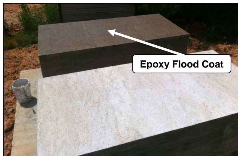
Figure 7.20: Epoxy flood coat application on arch test section
