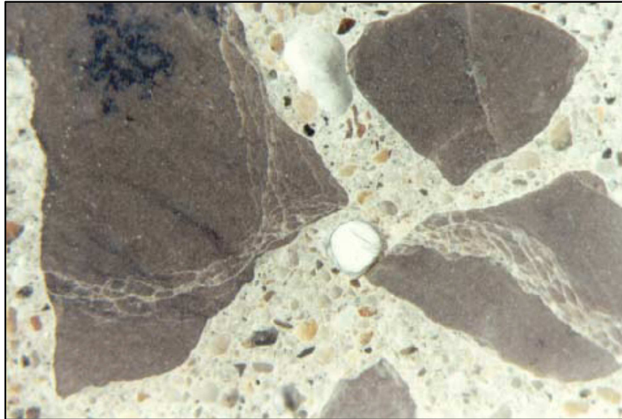
Figure 2.7: Extensive microcracking at 0.25 % expansion in aggregate particles and cement paste; also, a void filled with alkali-silica gel (Fournier et al. 2004)
