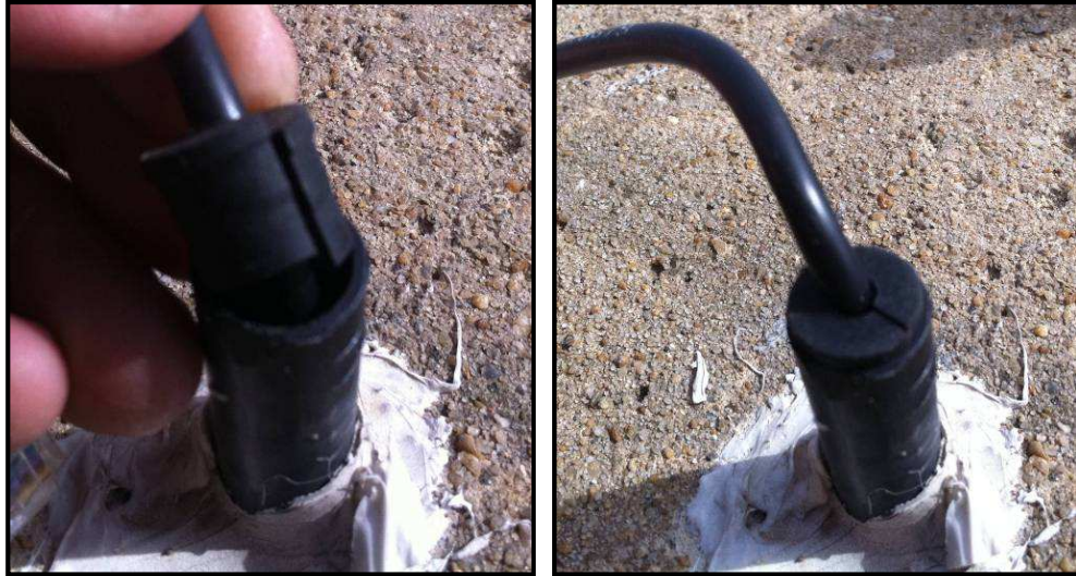
Figure 5.4: Plug being placed around probe wire
