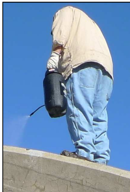
Figure 2.15: Silane being applied with a low-pressure garden sprayer
