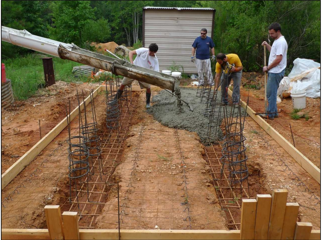
Figure 7.13: Construction of strip footings and slab on grade
