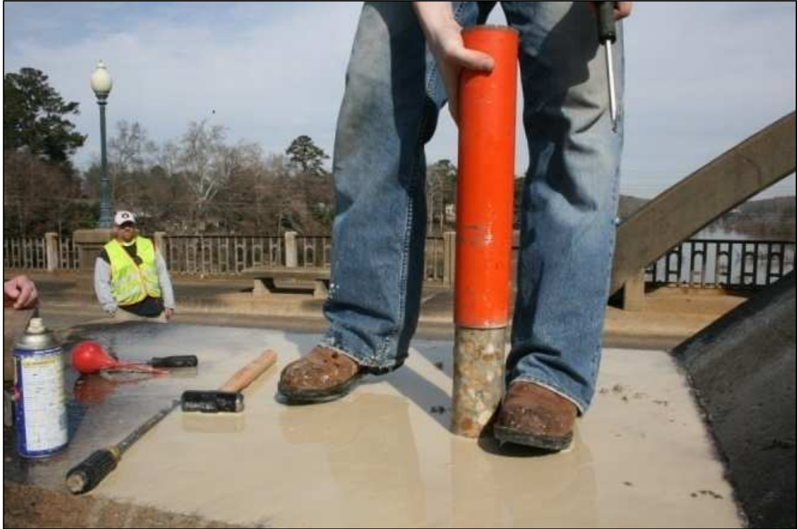
Figure A.6: Extraction of core samples (ALDOT 2010)
