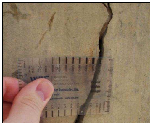
Figure 3.18: Crack width gauge in use
