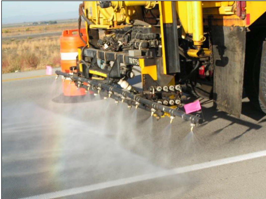
Figure 2.23: Topical application of lithium compounds (Fournier et al. 2010)
