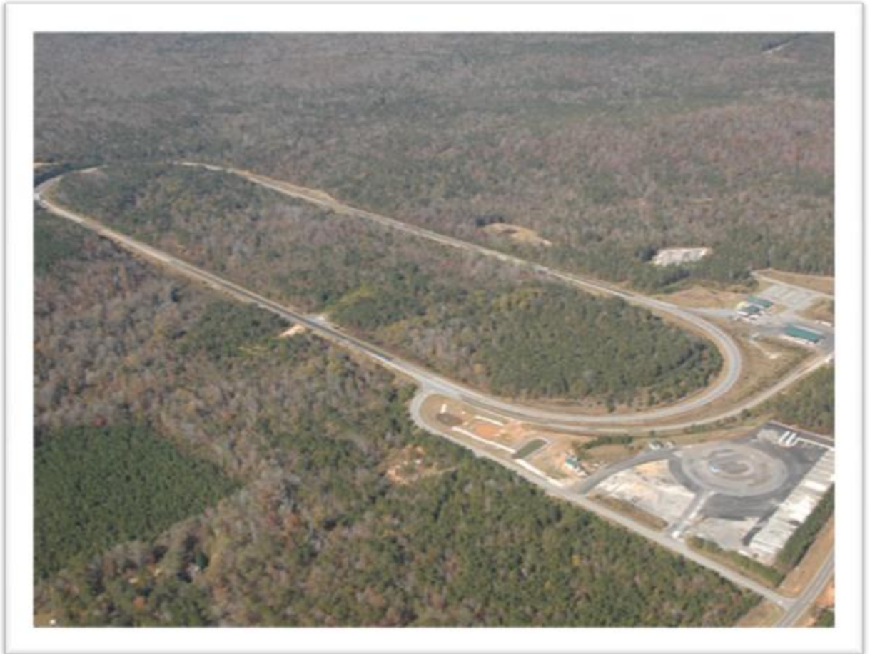
Figure 23. NCAT Test Track
