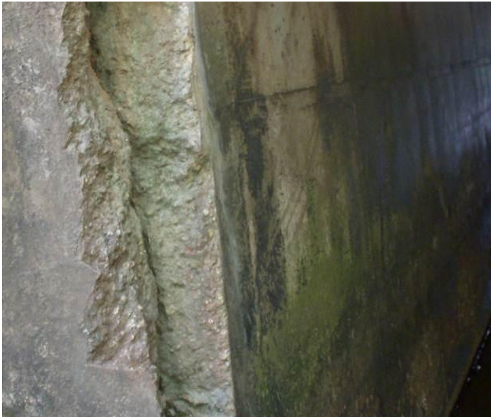
Figure 3-44: Wingwall Connection to the Culvert in Prattville Culvert on US-82
