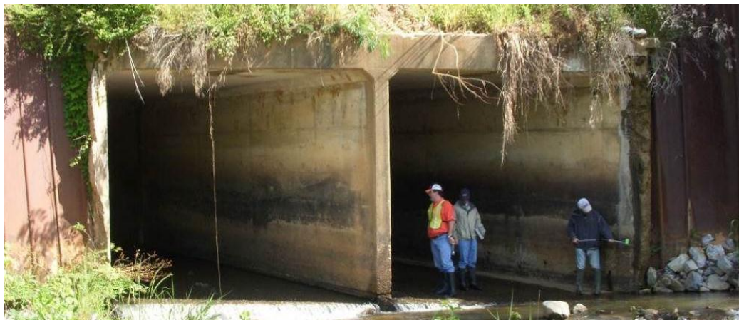
Figure 3-41: Entrance to Prattville Culvert on US-82
