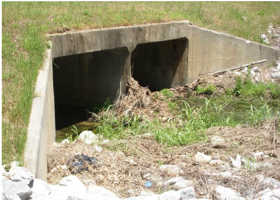
Figure 3-45: Entrance to I-85 North Culvert
