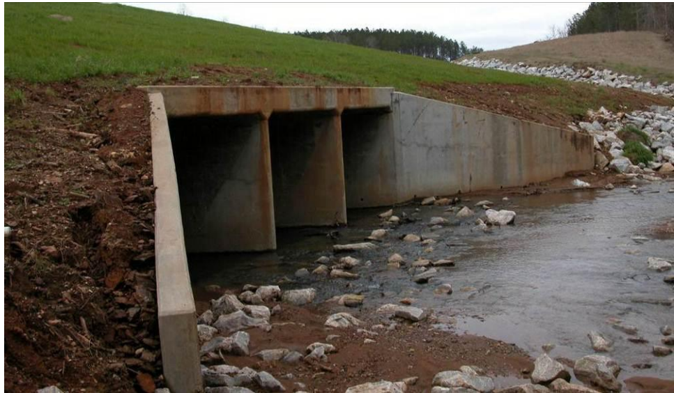
Figure 3-34: Dadeville Culvert at 45+31.55 Entrance
