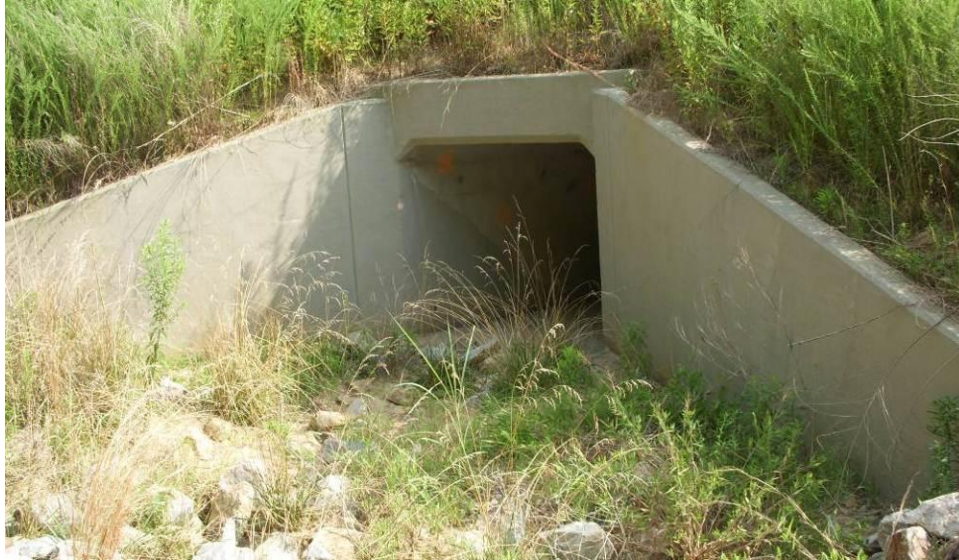
Figure 3-14: AEB Culvert at 257+69 Entrance
