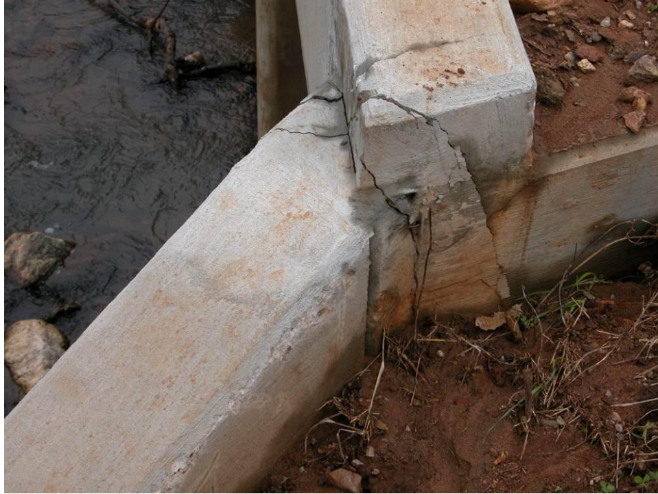
Figure 3-36: Dadeville Culvert at 45+31.55 Wingwall and Culvert Connection
