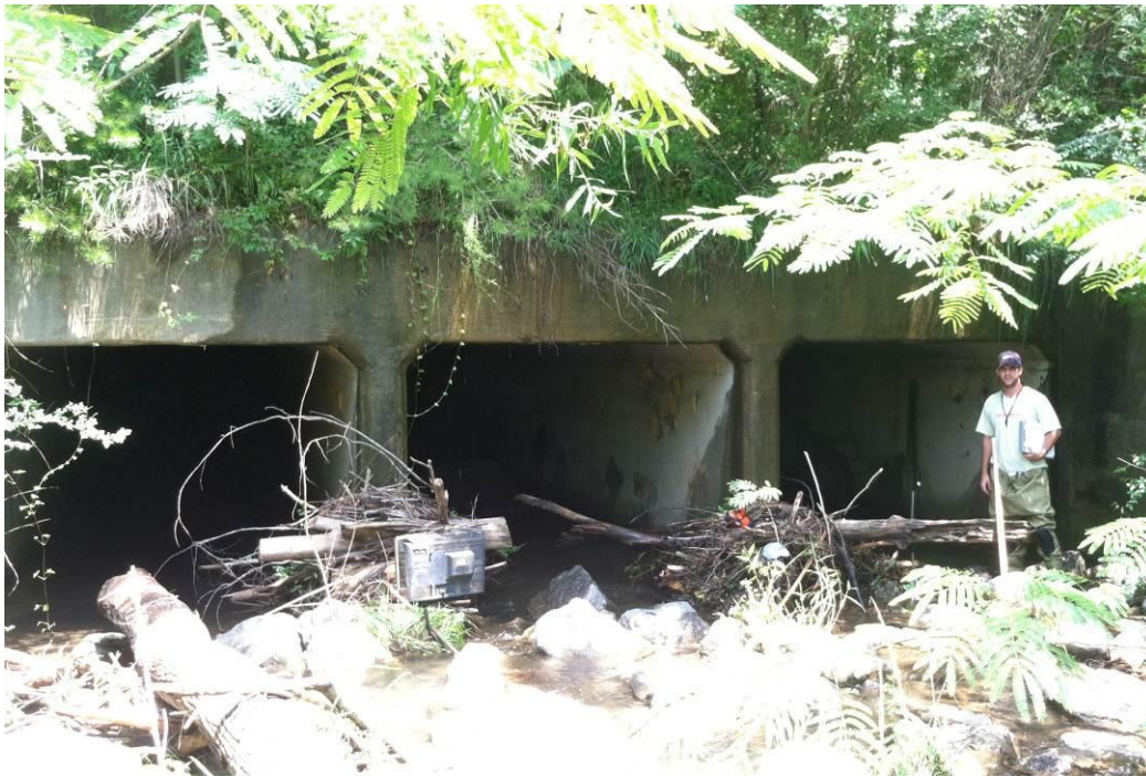
Figure 3-30: Corridor X Culvert at Exit 85 Southern Entrance
