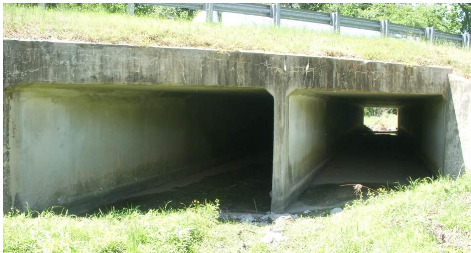
Figure 3-46: Entrance to I-85 South culvert
