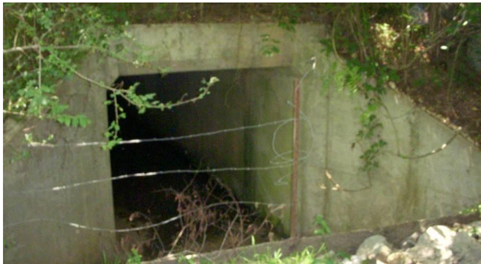
Figure 3-38: Dutton Culvert at 548+23 Entrance
