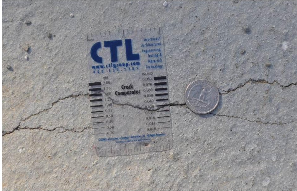
Figure 3-21: Ceiling Crack on the Outside of Centreville Culvert at 1808+98
