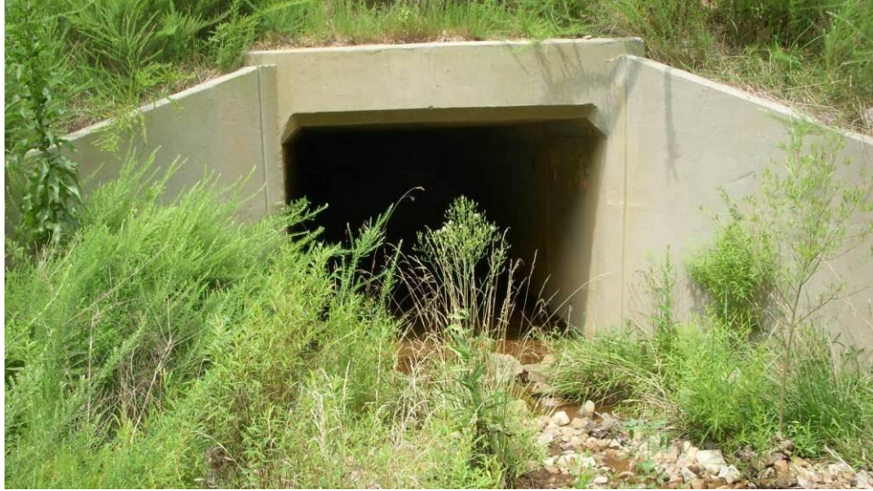
Figure 3-8: AEB Culvert at 175+70 Entrance
