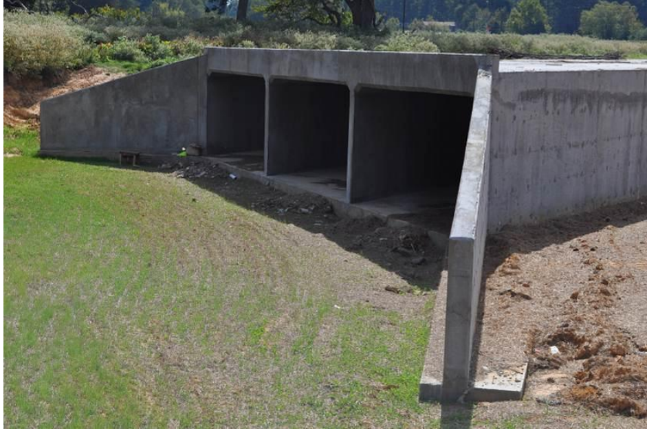
Figure 3-18: Centreville Culvert at 1808+98 Entrance
