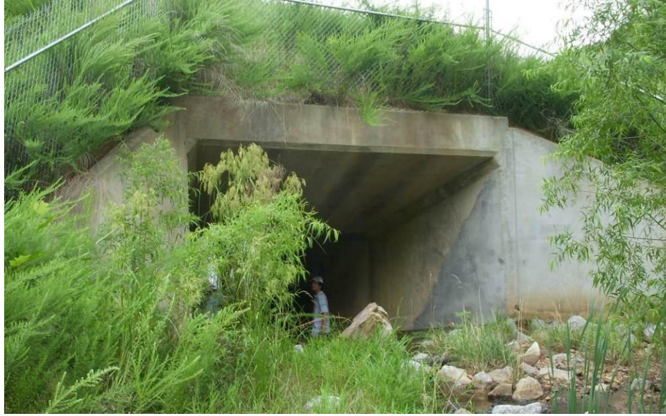
Figure 3-3: AEB Culvert at 149+60 Entrance
