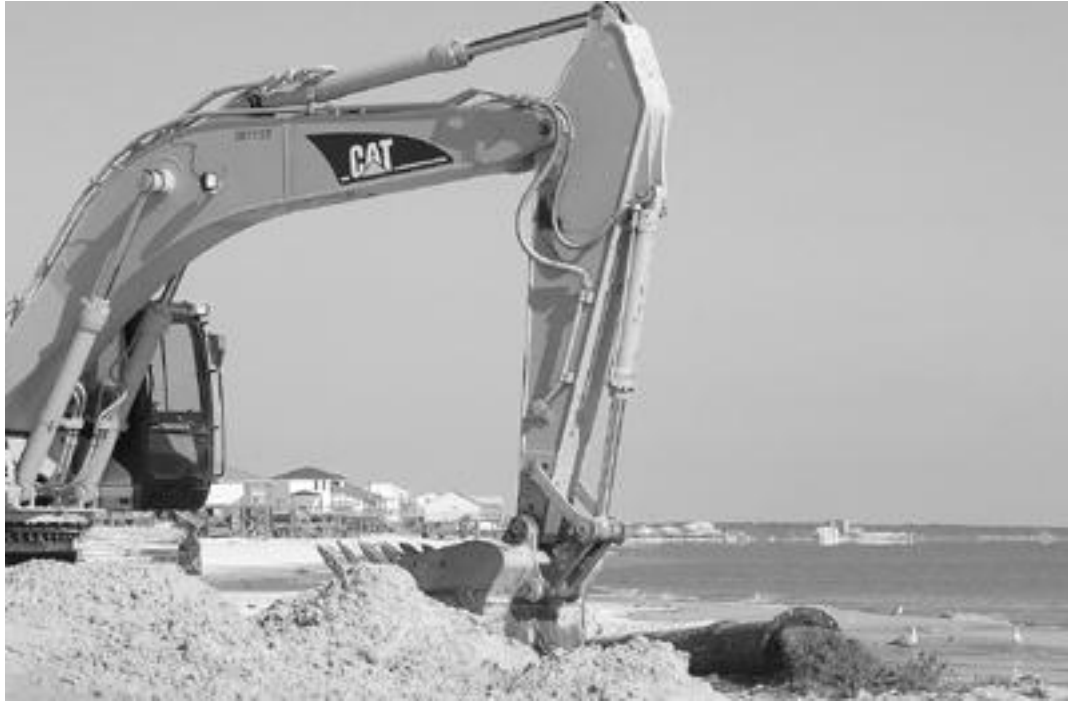
Figure 24. Berm/Beach re-nourishment strategy on Dauphin Island West End (Associated Press 2007)
