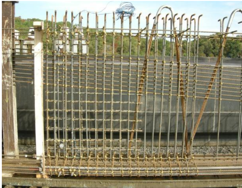
Figure 3-3: Thermocouple Wiring Installed in Unfinished Girder
