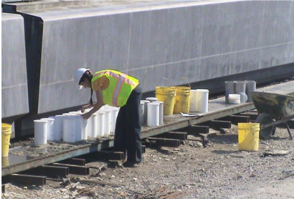
Figure 3-7: Concrete Cylinder Molds Used in Casting Test Specimens
