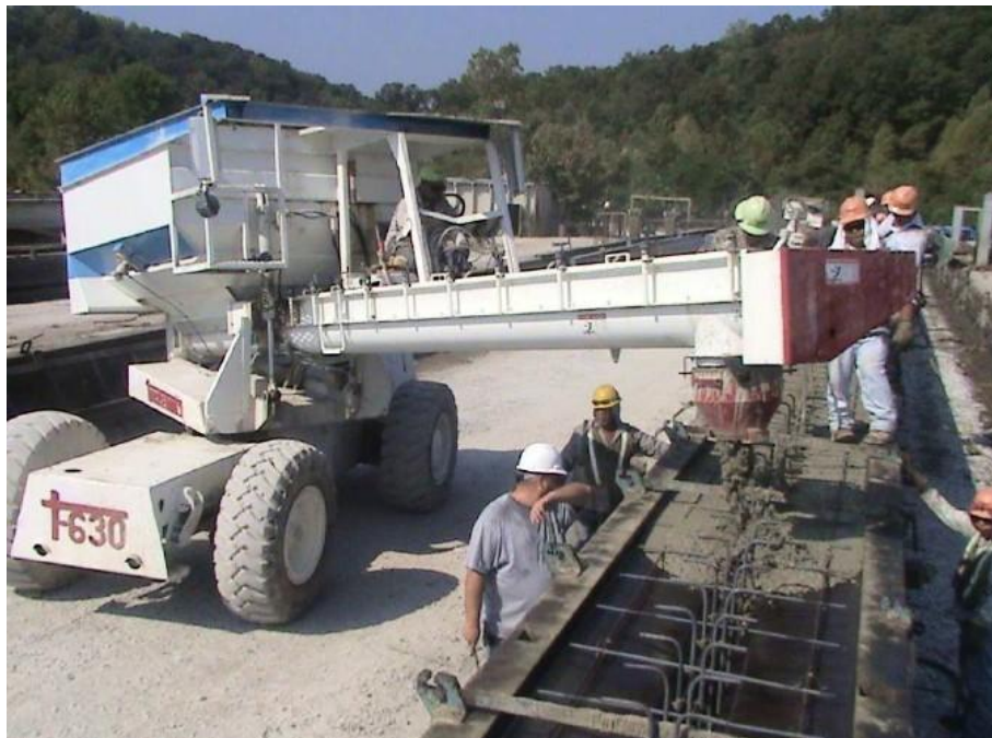
Figure 3-6: Concrete Delivery Vehicle Filling Girder Forms
