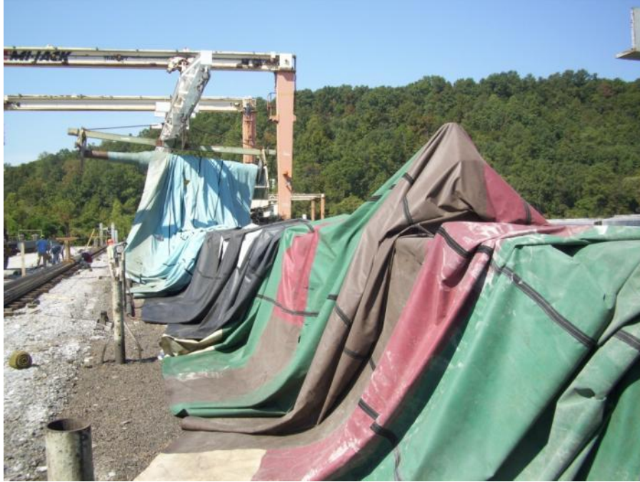
Figure 3-19: Covering the Girders and Test Cylinders for Tarp Curing
