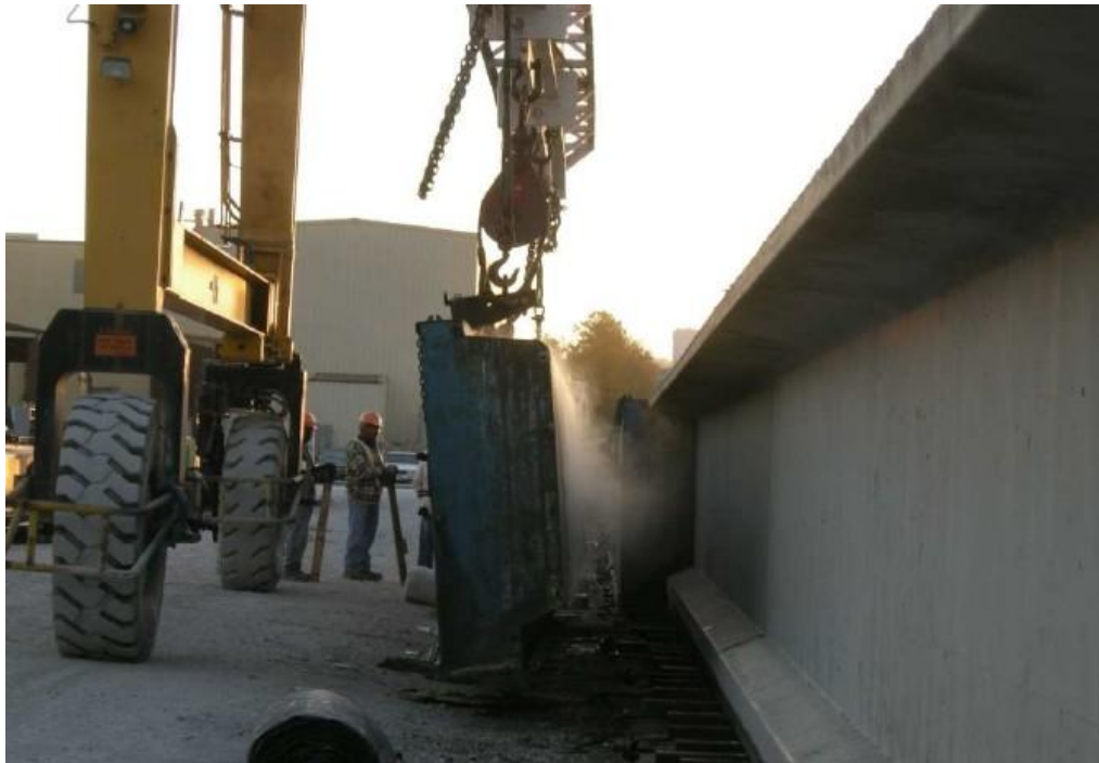
Figure 3-21: Removal of Side Forms from Girders
