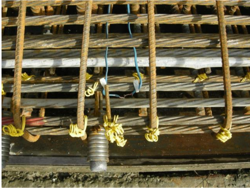
Figure 3-4: Close-up of Thermocouple Ends in Bottom Flange of Girder
