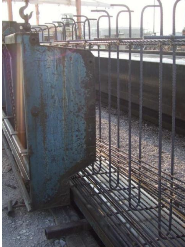
Figure 3-5: Girder Formwork Being Put in Place
