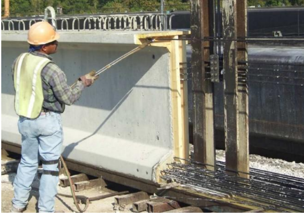
Figure 3-25: Flame-Cutting the Prestressing Strands
