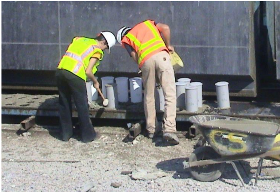
Figure 3-9: Casting and Tamping Test Specimens for SCC Mixtures
