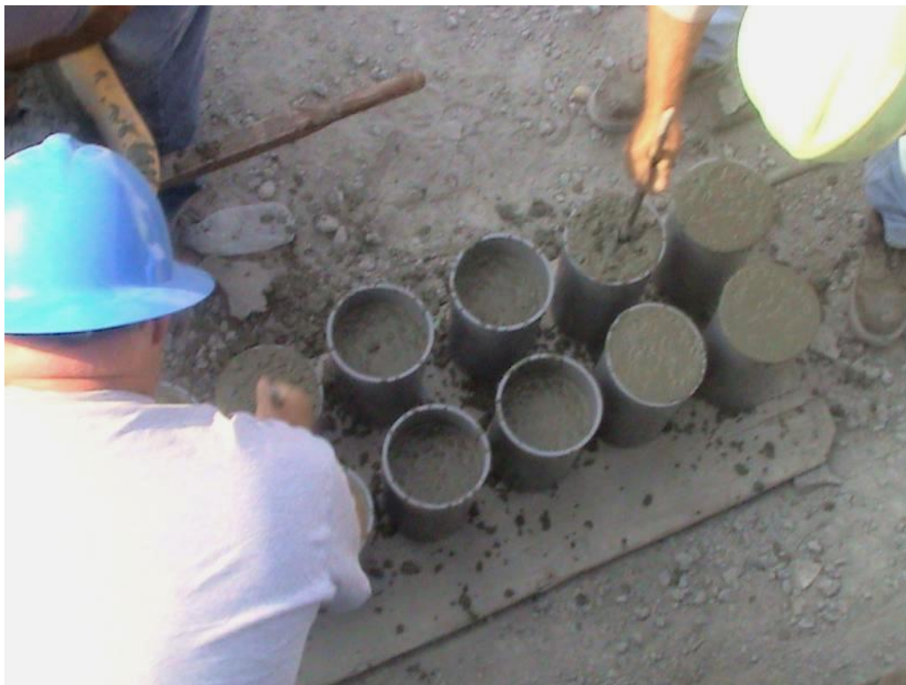
Figure 3-8: Casting and Rodding Test Specimens for CVC Mixtures
