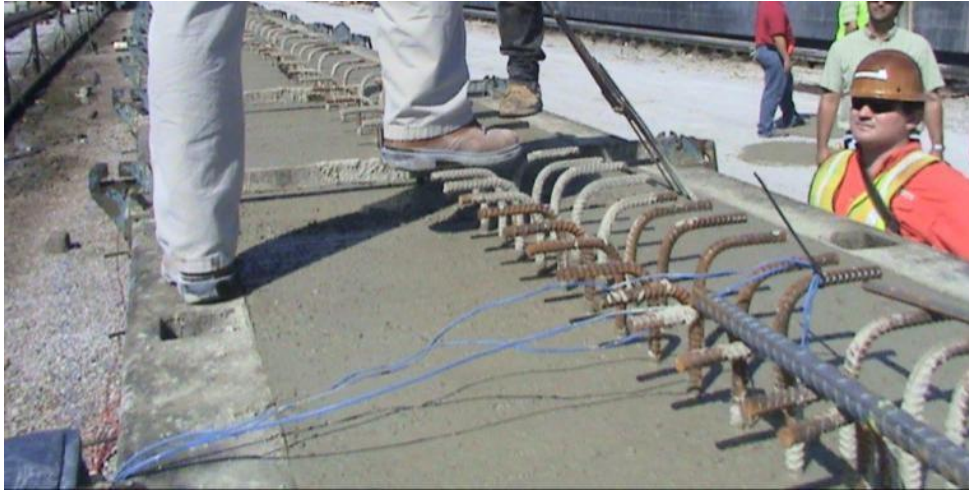
Figure 3-16: Thermocouple Wires in Concrete Girder
