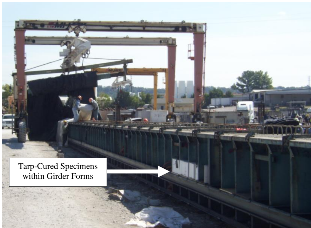
Figure 3-12: Placement of Curing Blankets and Weatherproof Tarp
