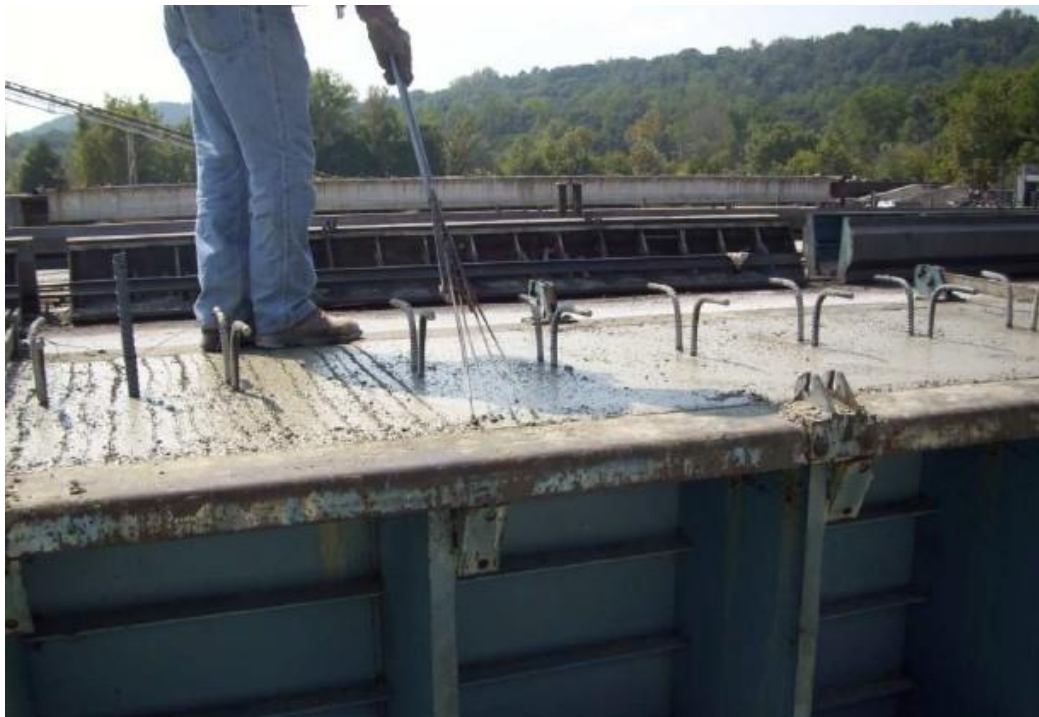
Figure 3-10: Roughing Girder’s Concrete Surface
