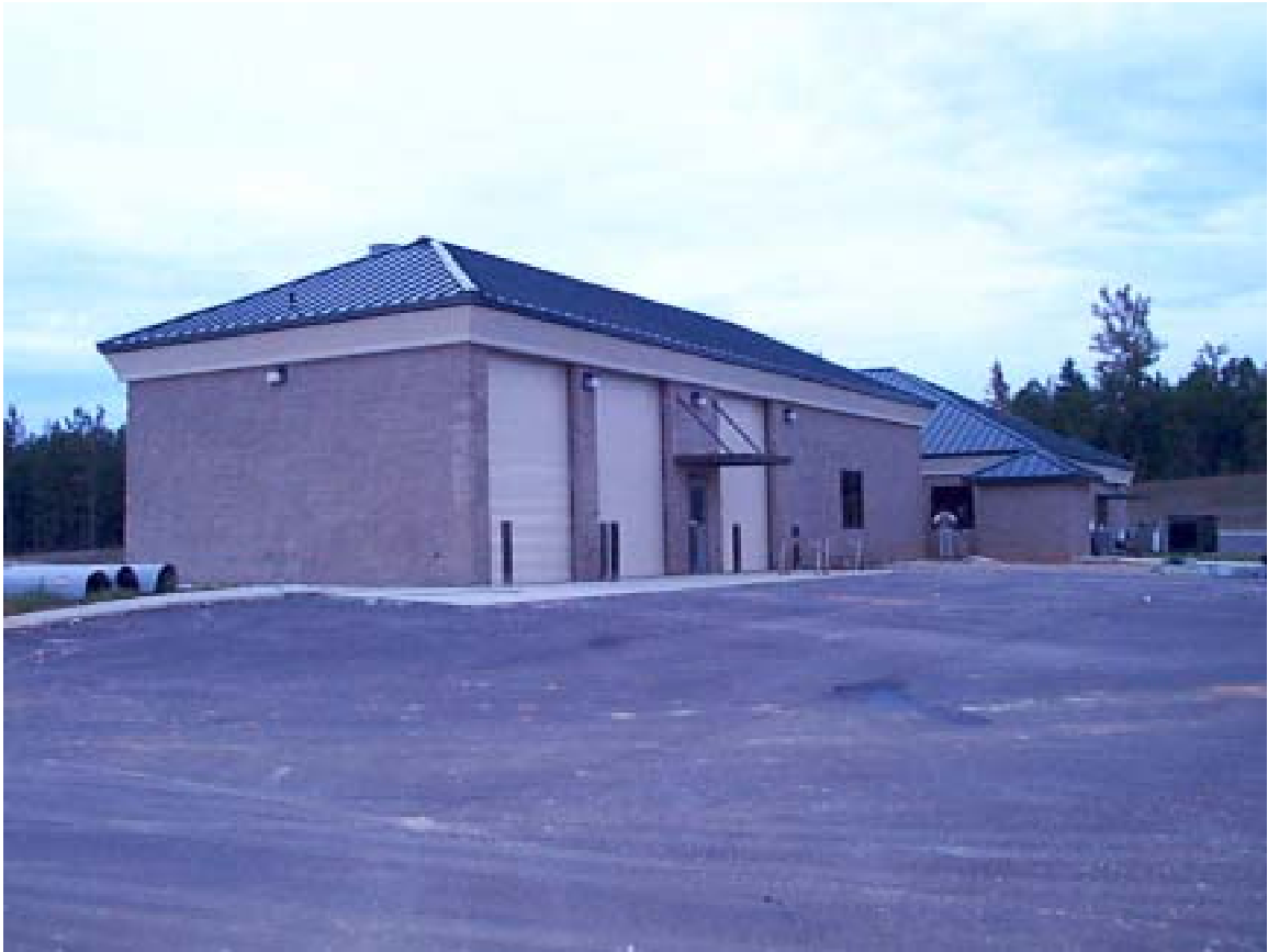
FIGURE 3.8 Track's On-site Truck Maintenance Building (Testing Laboratory in Background).
