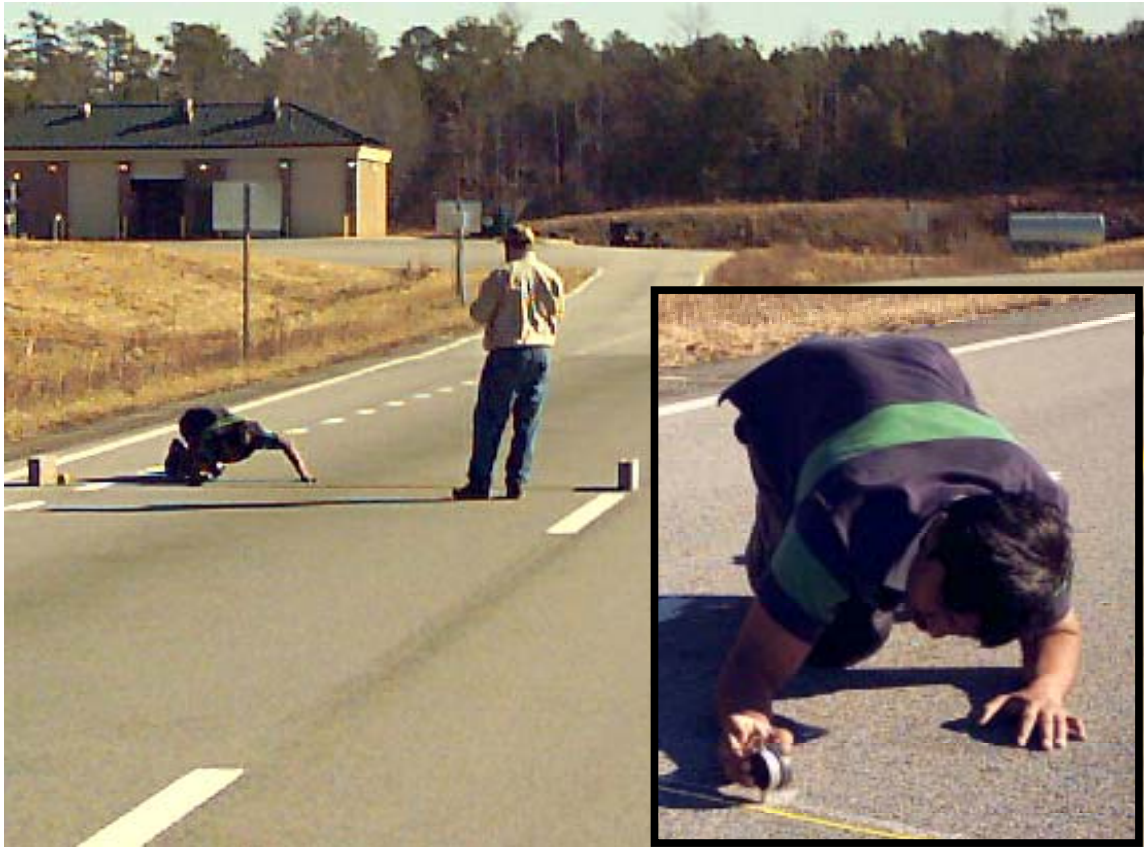
FIGURE 4.4 Stringline Measurements After Completion of Traffic.
