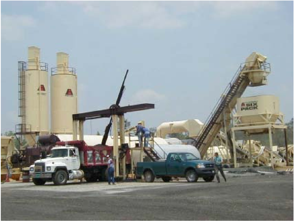
FIGURE 3.5 Production and Sampling of Hot-Mix at Track's On-site Plant.
