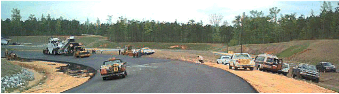
FIGURE 3.7 Placement and Compaction of Experimental Mix in East Curve.
