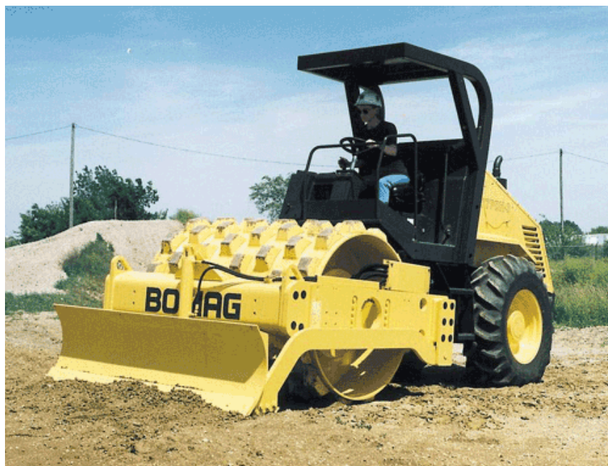
Figure 2.25: Sheepsfoot roller used to compact soil-cement base (FHWA 2011)
