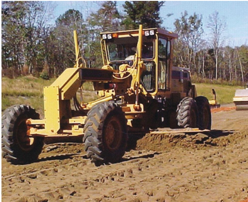
Figure 2.24: Spreading operations (Halsted et al. 2006)
