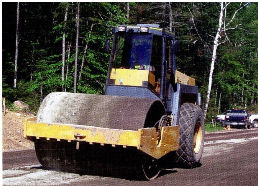
Figure 2.27: Steel-wheel vibratory roller used to compact soil-cement base (Halsted et al. 2006)
