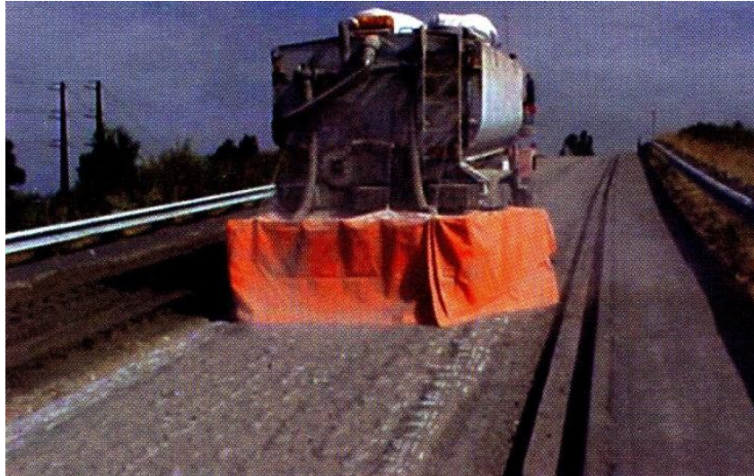
Figure 2.21: Application of cement to roadbed by mechanical spreader (Halsted et al. 2006)
