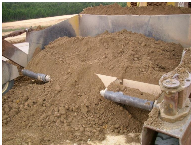
Figure 3.3: Paving hopper from soil-cement construction
