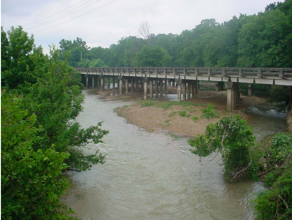
Figure 38. Highway 79 Bridge, looking upstream.
