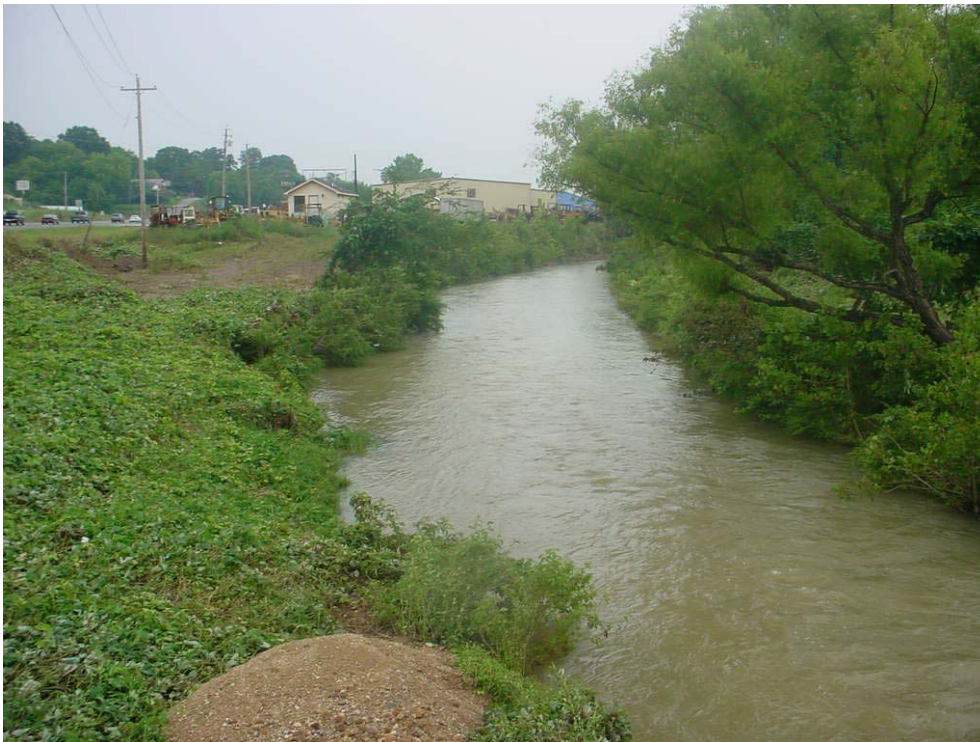
Figure 37. Section H, looking downstream.
