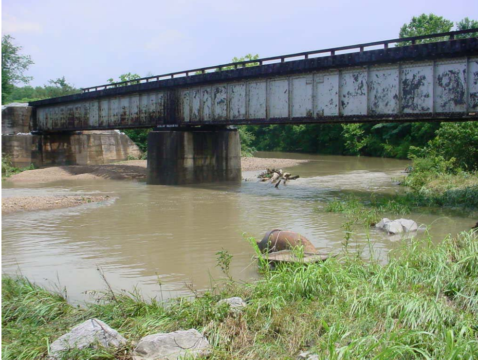
Figure 34. Railroad Bridge, looking upstream.
