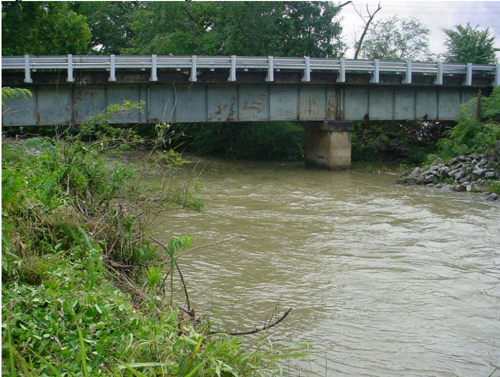
Figure 31. Alabama Power Company Bridge, looking upstream.
