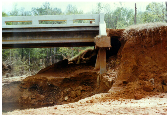
Figure 1-1. Example of Bridge Scour
