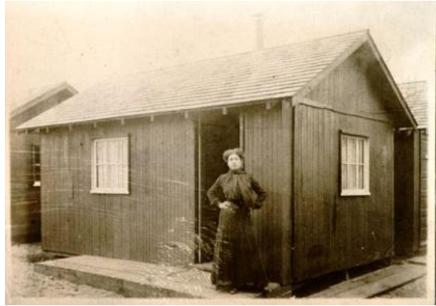
Figure 22: Earthquake Shack after Earthquake of 1906 in San Francisco, California Photo by: San Francisco History Center, SF Public Library
