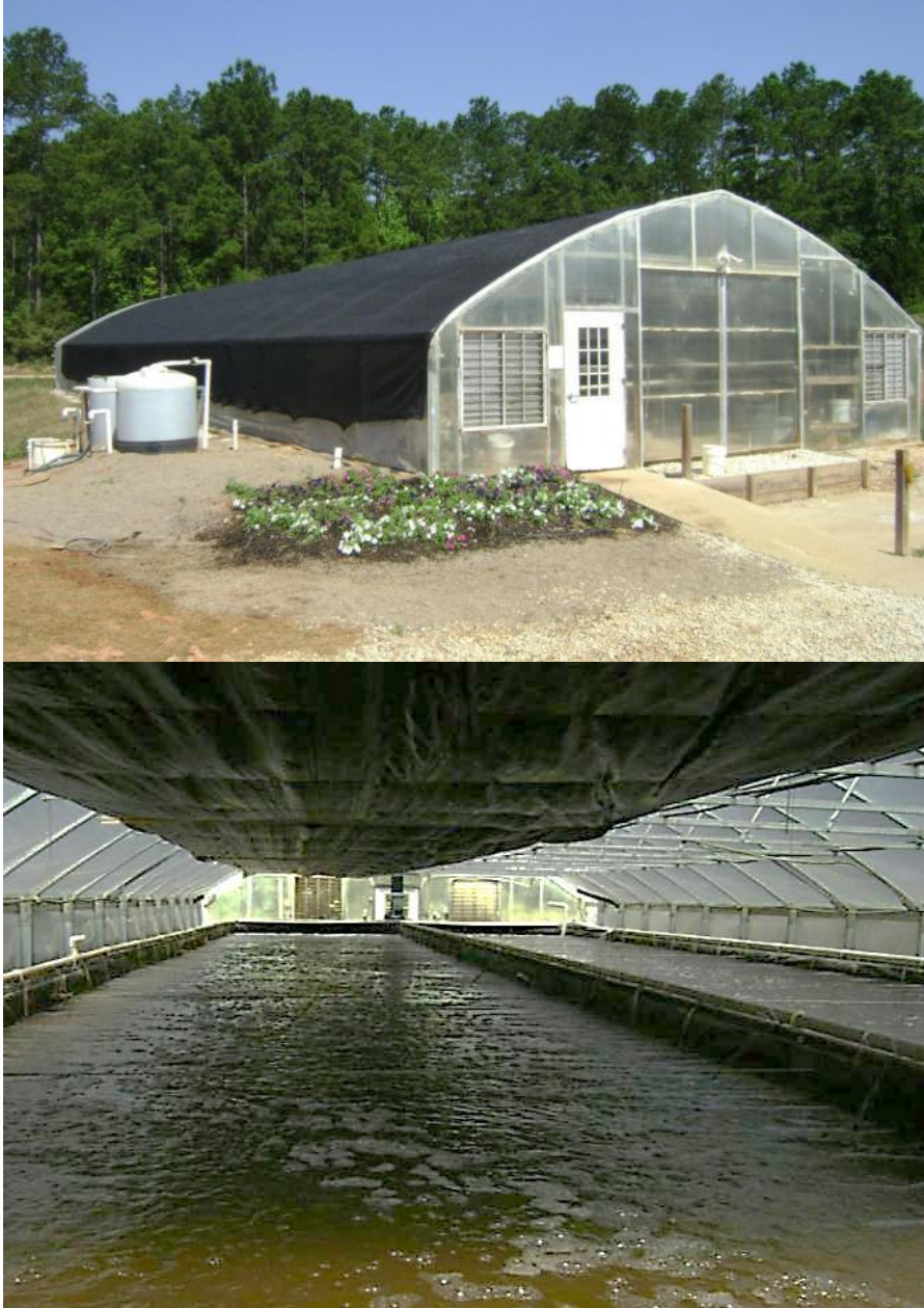
Figure 1A. The greenhouse (top) at the E.W. Shell Fisheries Center, North Auburn Unit, in Auburn, Alabama containing the 100-m 3 biofloc, recirculating aquaculture system (bottom) producing Nile tilapia ( Oreochromis niloticus ) and where discharged effluent was collected.
