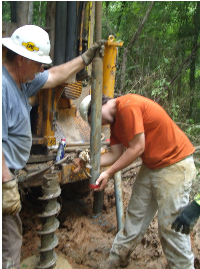
Figure 3.30: Shelby tubes being prepared to take out of the site
