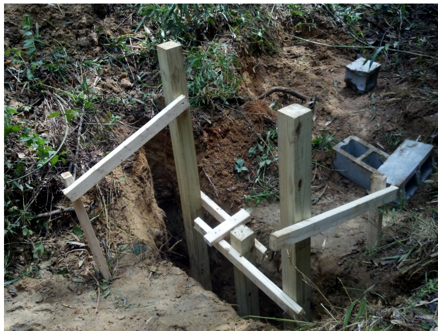
Figure 3.13: Support post for the rectangular weir
