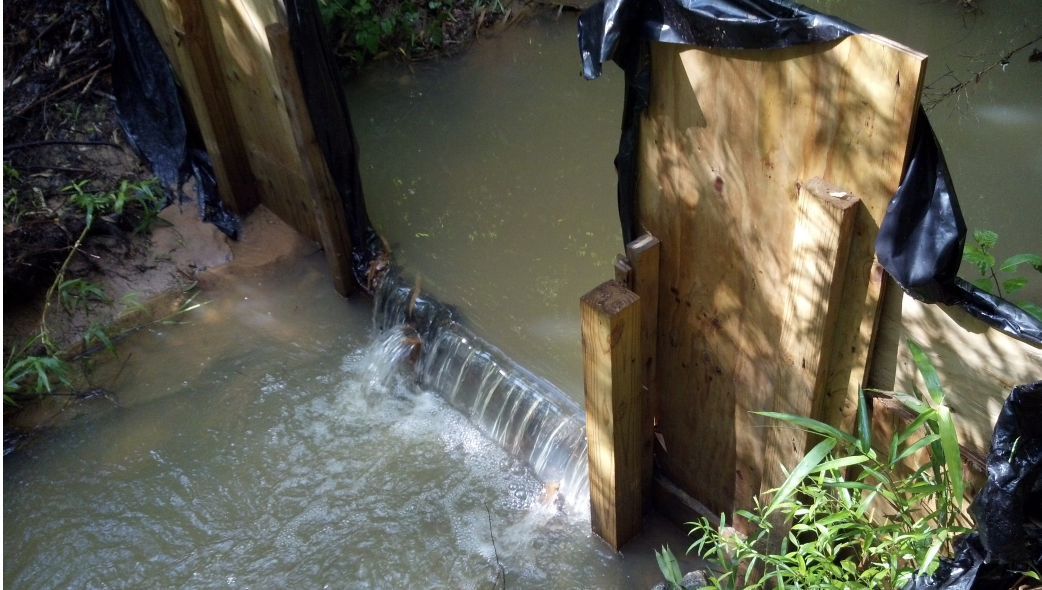
Figure 3.14: Upstream view of rectangular weir
