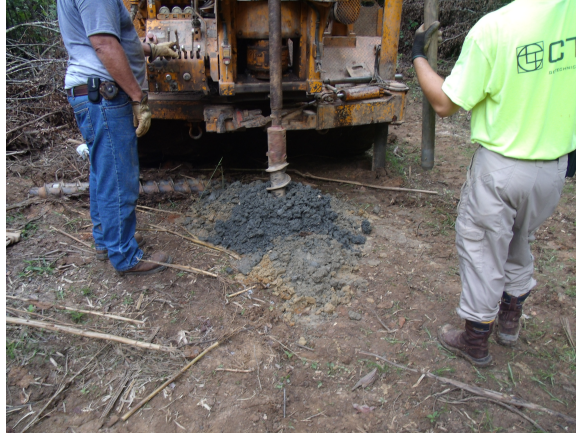
Figure 3.28: Soil exiting the bore hole from approximately 4.6 m below the surface
