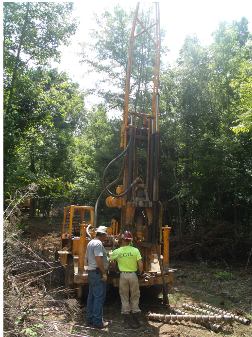
Figure 3.27: Setting up to drill boring
