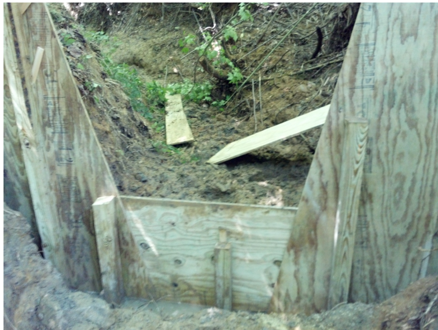
Figure 3.9: Downstream view of the Cipolletti weir
