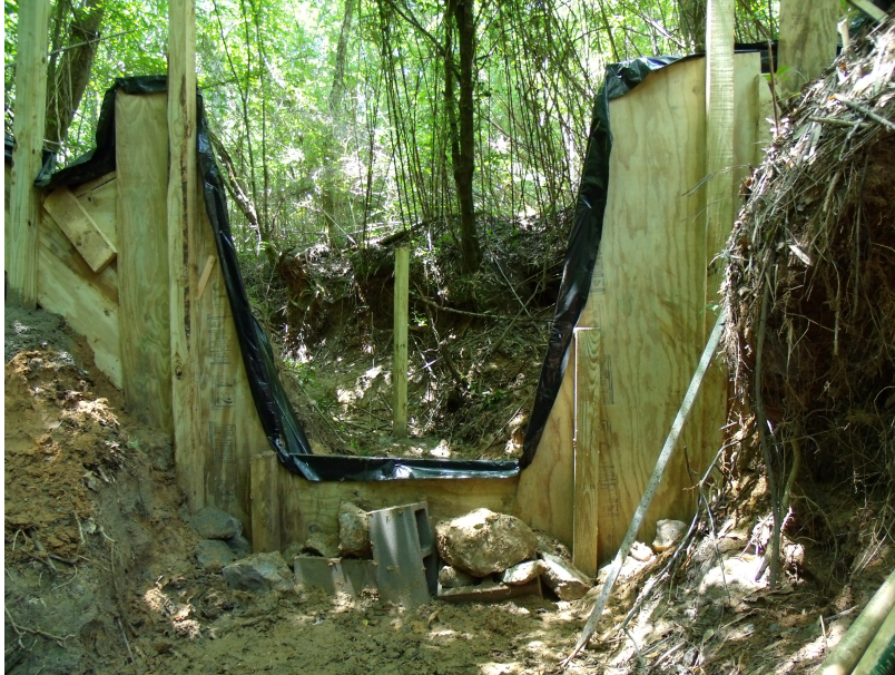
Figure 3.11: Finished Cipolletti weir looking upstream: completed (June 1st 2012)
