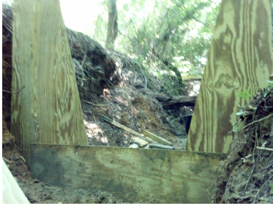
Figure 3.8: Upstream view of the Cipolletti weir
