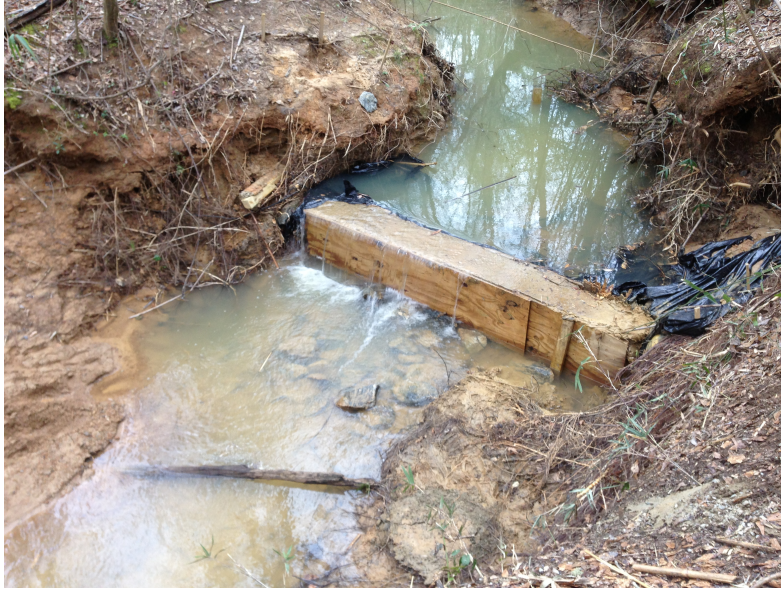
Figure 3.18: Upstream view of broad crested weir
