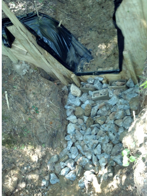
Figure 3.10: Riprap placed at the downstream side of the Cipolletti weir
