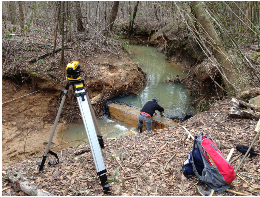
Figure 3.35: Surveying a downstream cross section
