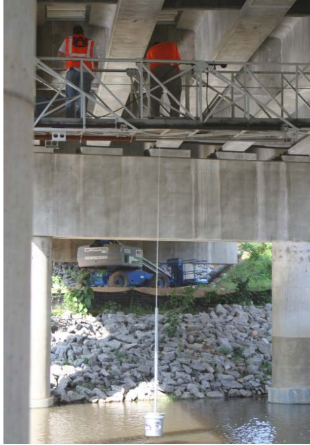
Figure 3.32. Deflectometer-wire anchoring device being lowered into Hillabee Creek.
