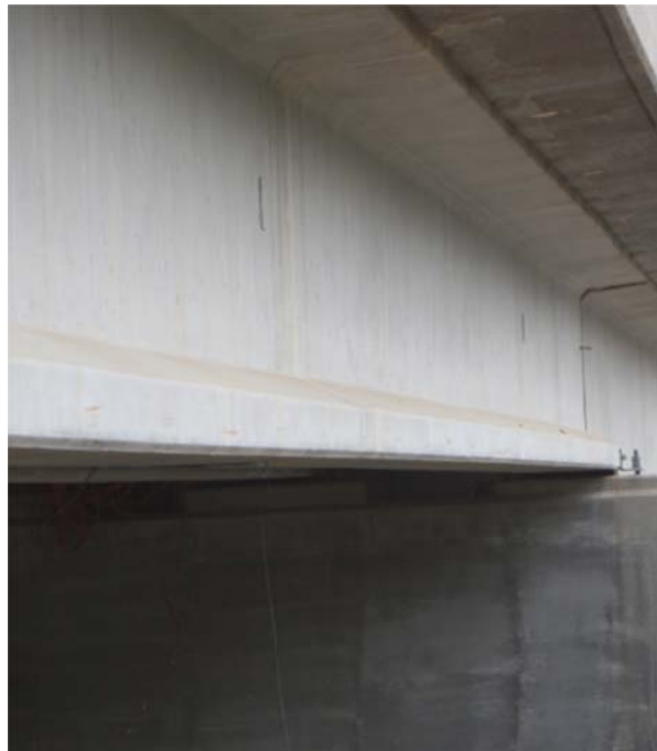
Figure 3.1. Exterior, VC BT-54 girder in span 4.
