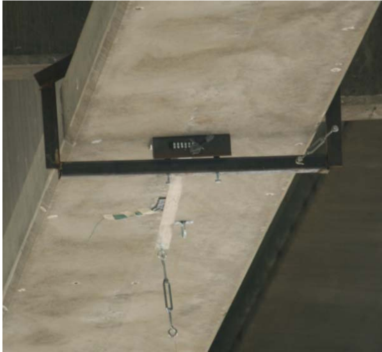
Figure 3.30. A deflector attached to a girder over span 3.
