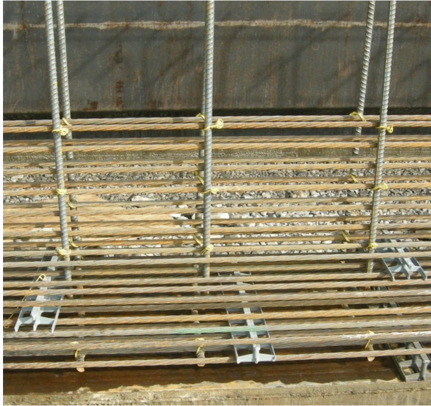
Figure 3.22. Prestressing wire surface condition (Johnson 2012).
