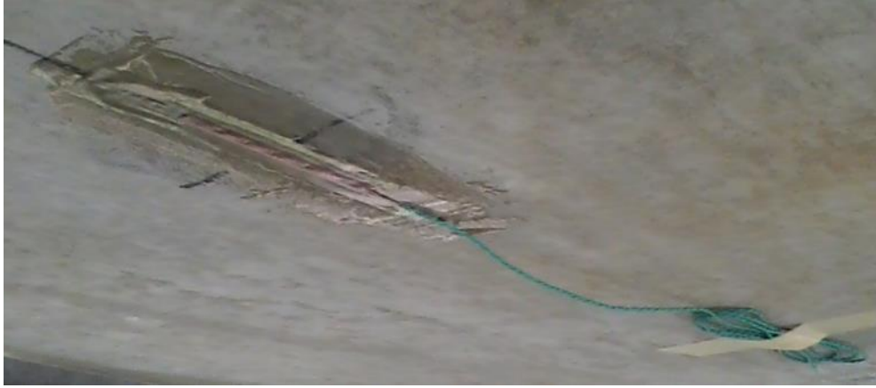
Figure 3.25. Thin layer of epoxy placed over the strain gauge for waterproofing.
