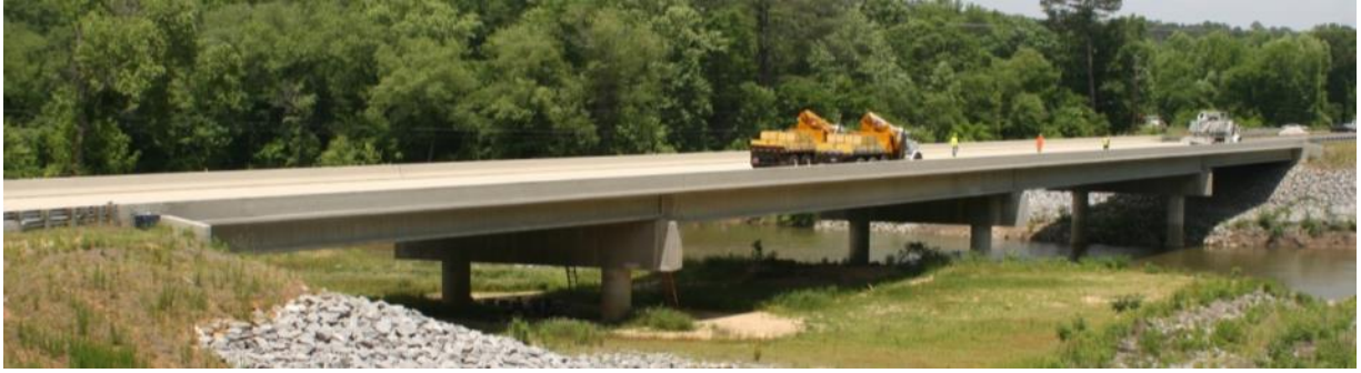
Figure 1.1. Load trucks on Span 2 (SCC Girders) of the Hillabee Creek Bridge during testing.
