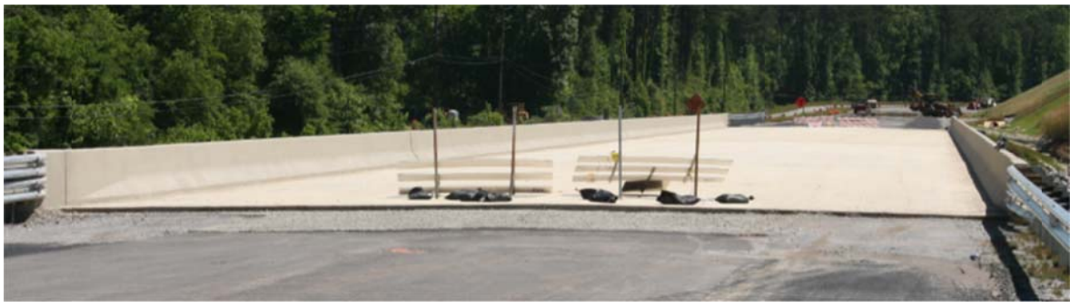
Figure 3.6. Bridge deck and barriers in place.
