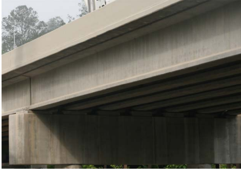
Figure 3.2. SCC BT-72 girders.
