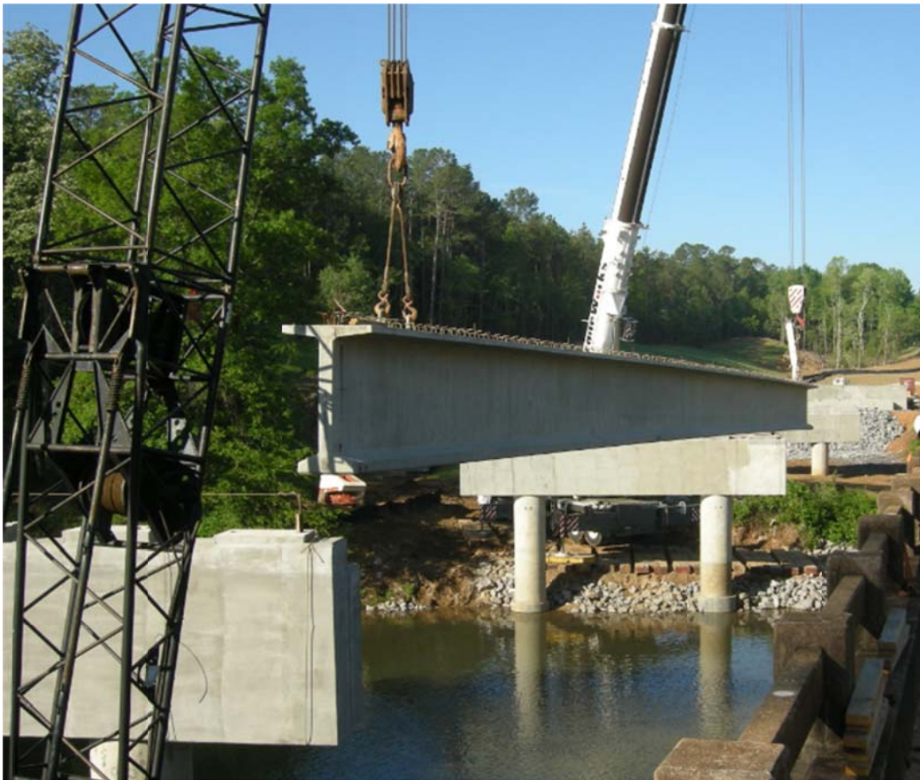
Figure 3.7. A span 3 (VC) girder lowered into position.
