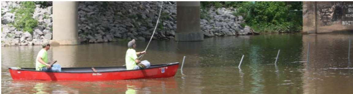
Figure 3.33. Placing deflectometer-wire anchors.
