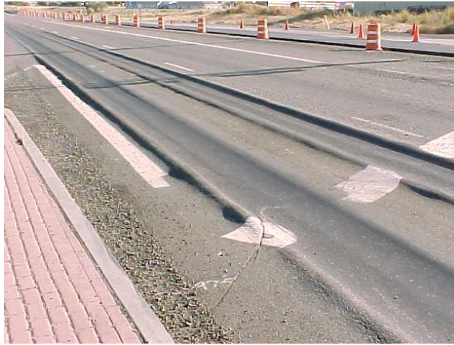
Figure 2.2 Rutting ( Rutting, 2008 )
