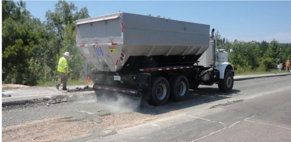
FIGURE 3.5 Portland Cement Being Spread on Section S12
