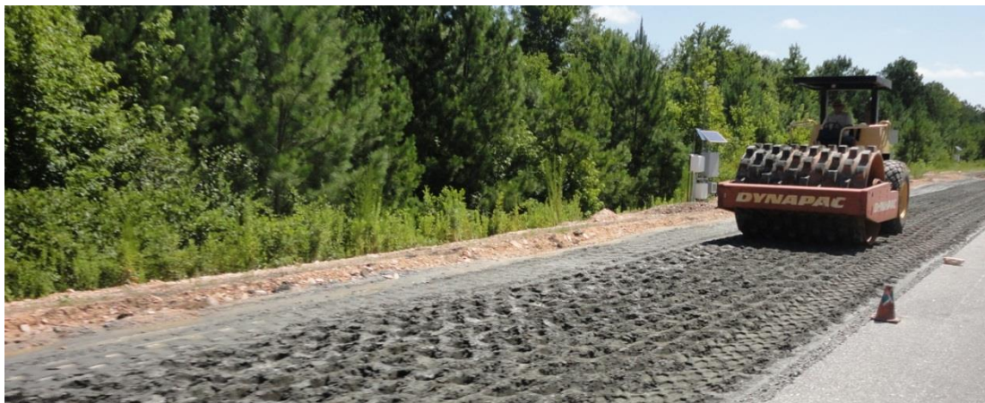
FIGURE 3.4 Granular Base Material Being Compacted
