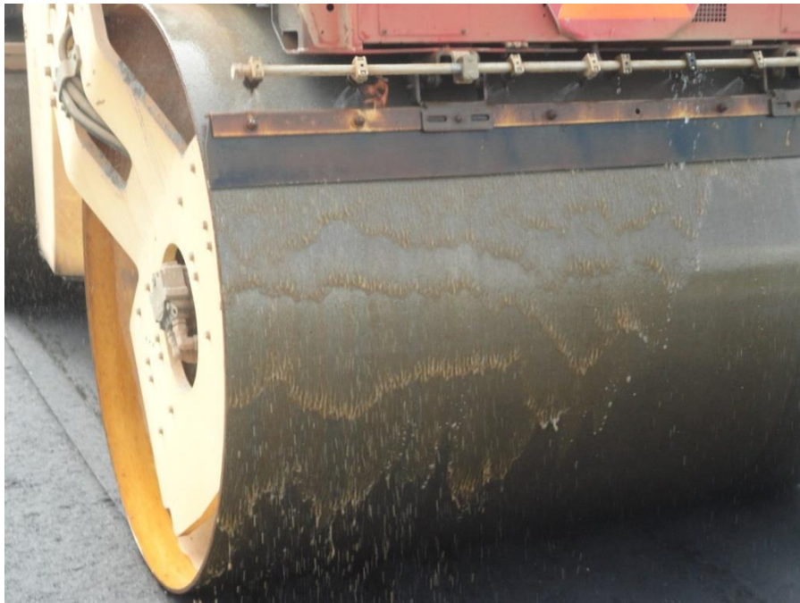
FIGURE 4.3 Water Sprayed on the Drum of the Vibratory Roller
