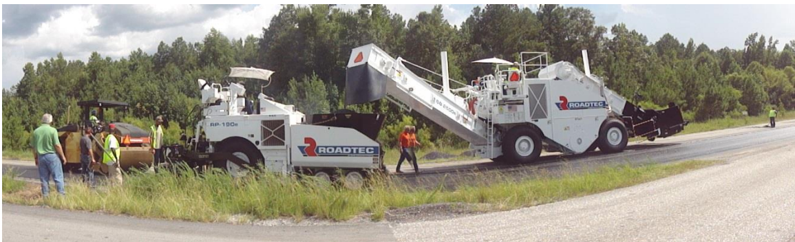
FIGURE 3.9 Paving Process at the NCAT Test Track
