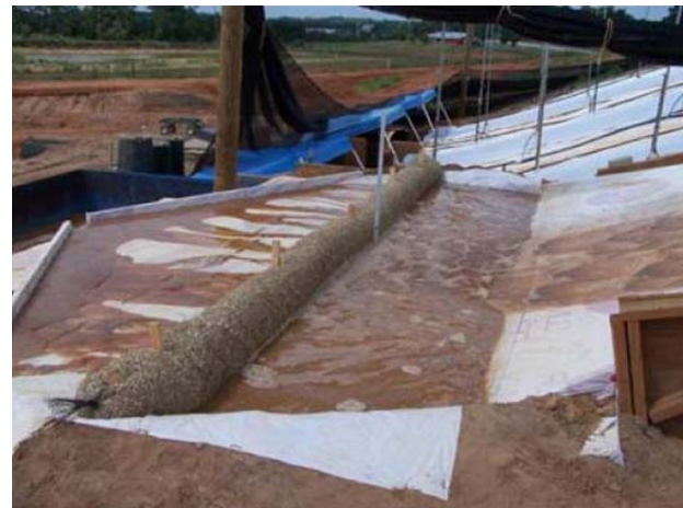
(b) wattle ponding sediment-laden sheet flow
