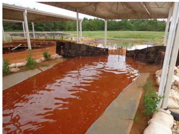
(b) ditch check impoundment
