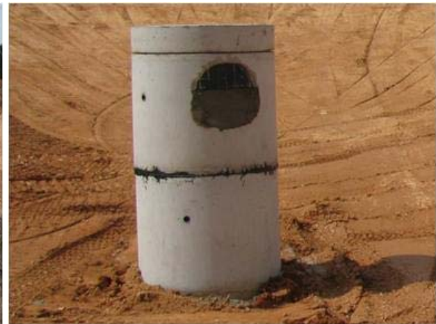
(b) upper three sections of the riser
