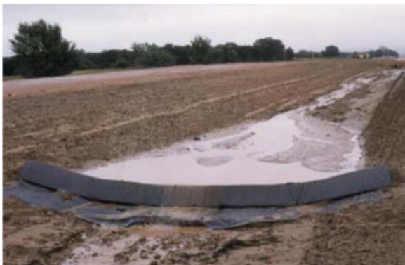
(a) silt dike in a bare earthen swale
