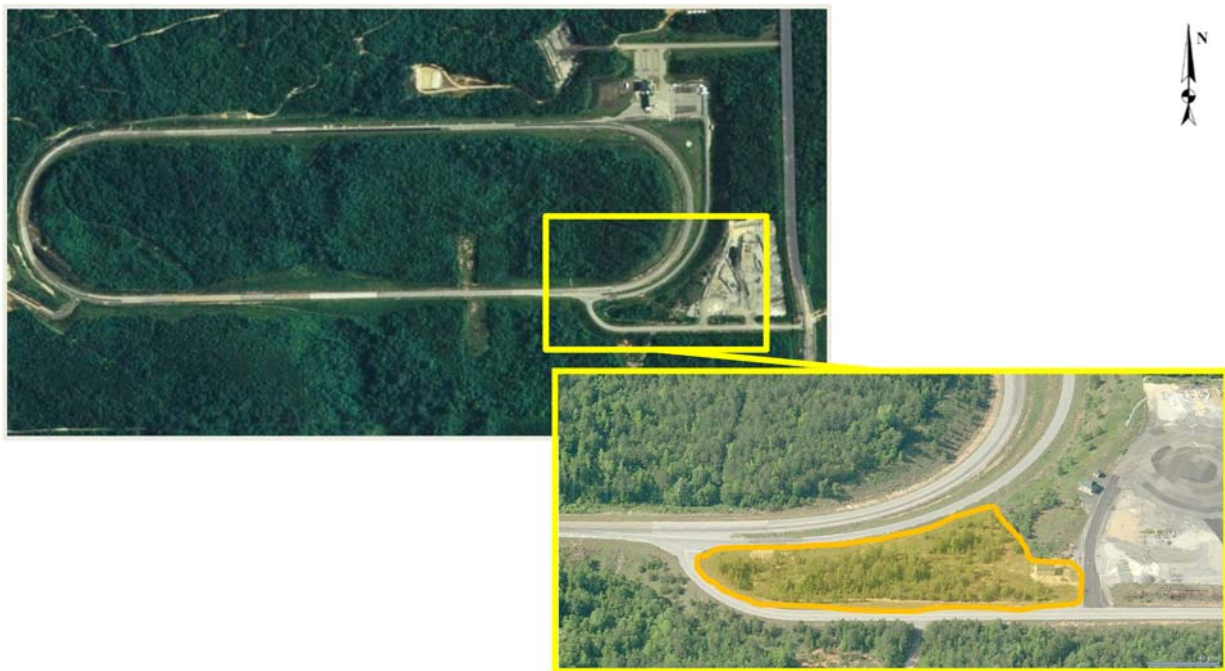
Figure 3.1: Preconstruction Aerial View of the Facility Location (Google Earth).
