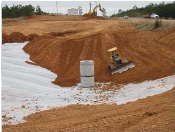
(a) spreading of cover soil
