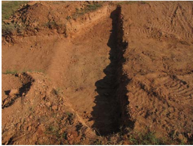
(a) excavation of head of conveyance channel
