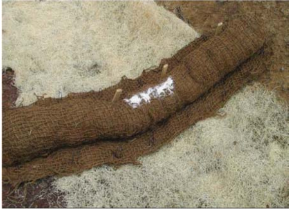
(a) coir wattle w/PAM dosing check dam
