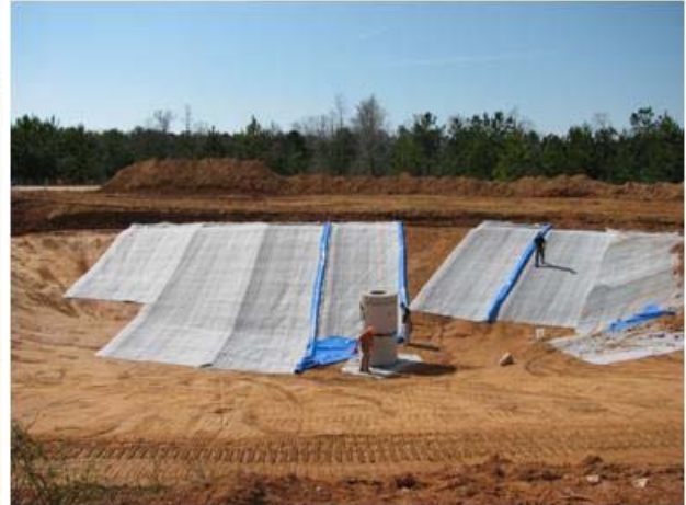
(b) first set of installed liner
