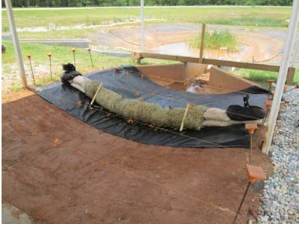
(a) Erosion Tech: Wheat Straw Sediment Logs
