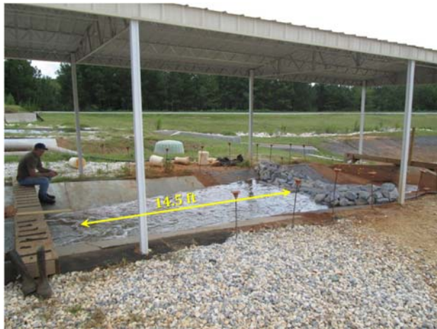
(a) riprap ditch check w/no choker
