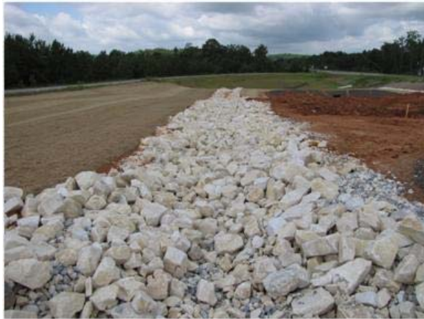
(c) outlet channel responsible for conveying discharge to the retention pond
