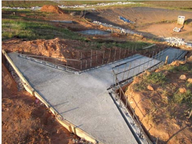
(c) reinforcement of retaining walls
