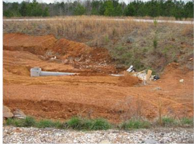
(b) relocation of the riser pipe
