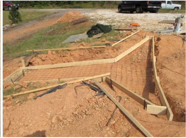
(b) form or conveyance channel slab
