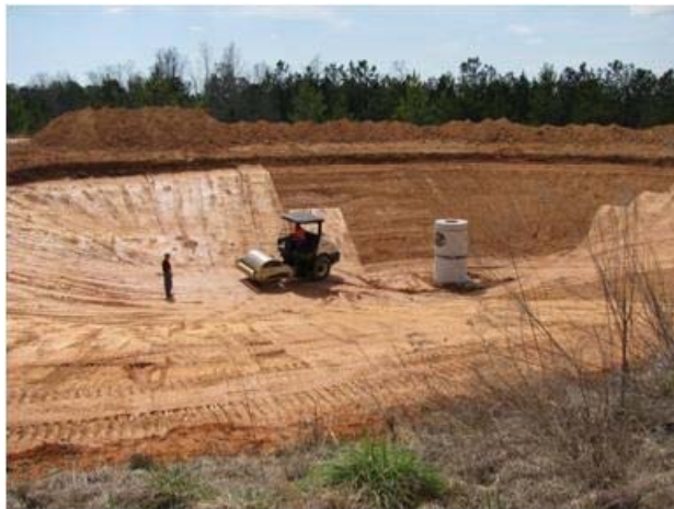
(a) final location of the permanent riser
