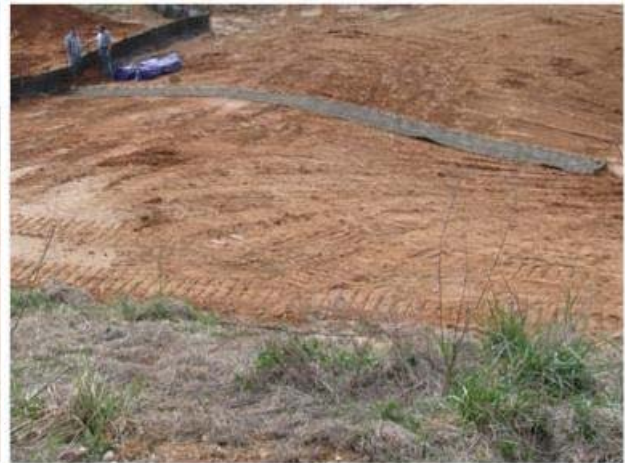
(b) installation of TRM
