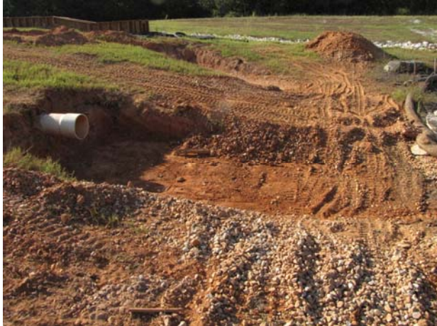
(a) excavation of drop inlet discharge area
