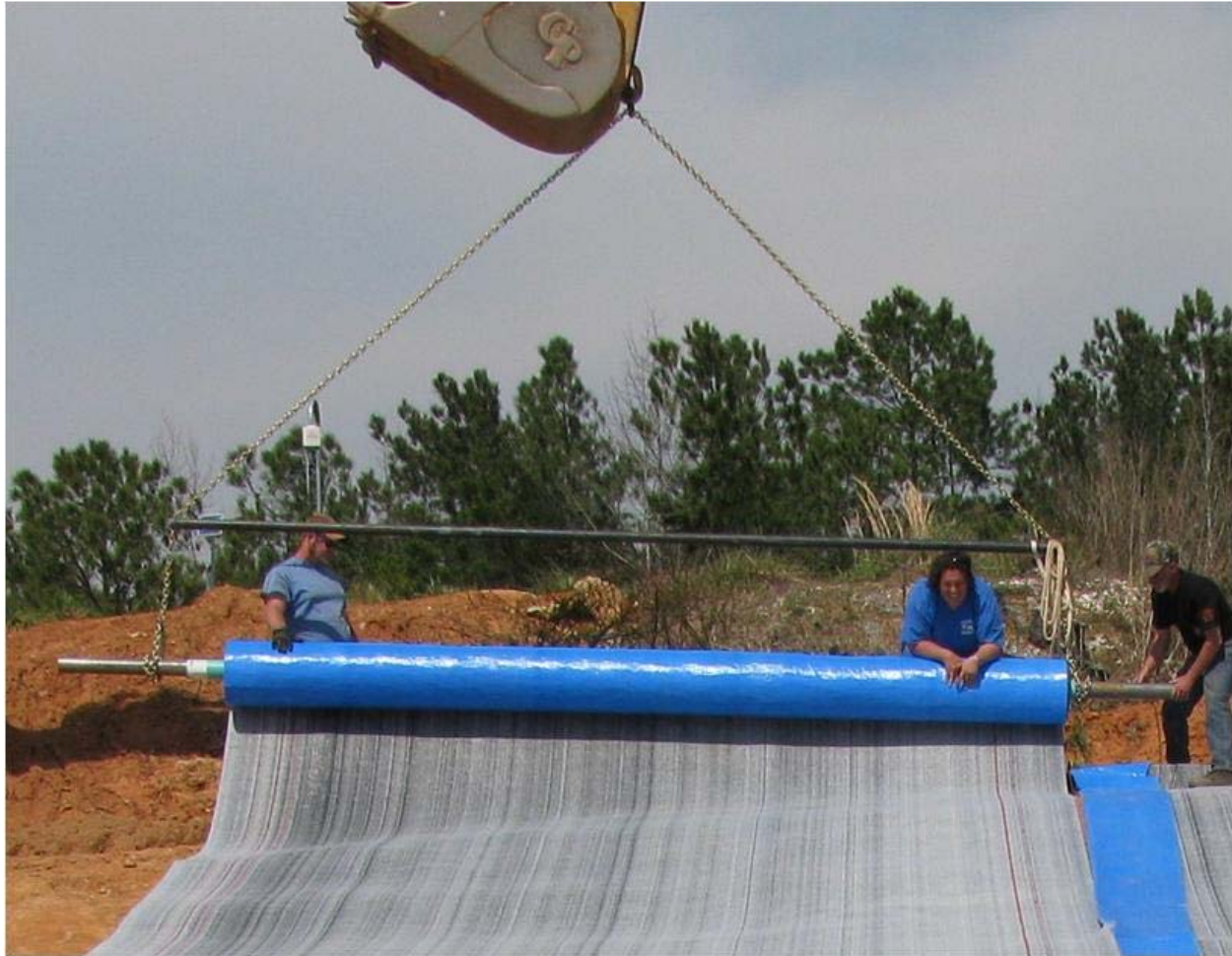
Figure 4.7: Pond Liner Installation Set Up.
