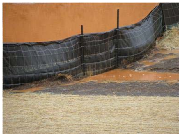
(a) silt fence impounding facility runoff
