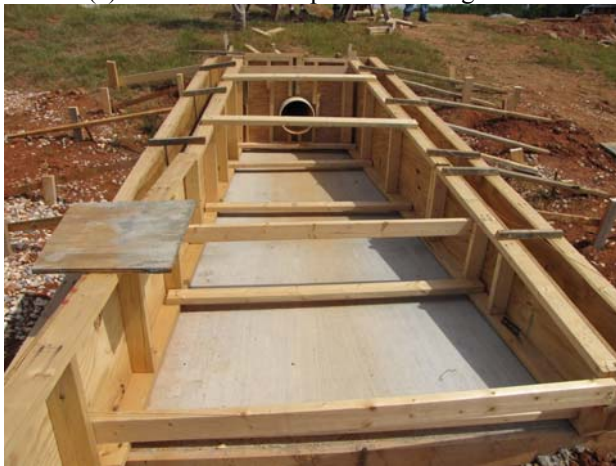
(c) retaining walls forms
