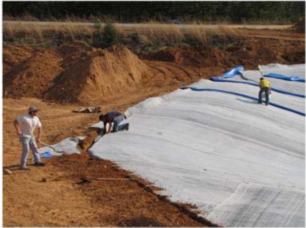
(f) keying in of and final installation of the pond liner
