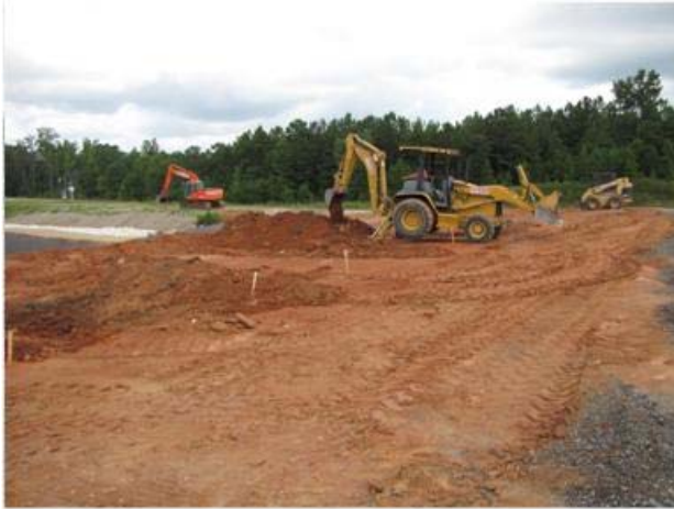
(a) backhoe used to excavate test channels
