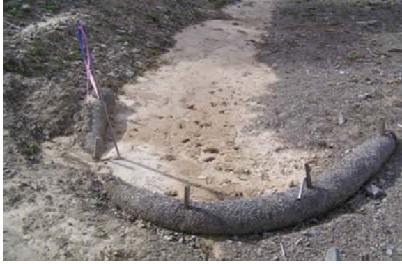
(a) wattle ditch check in a wide bottom ditch
