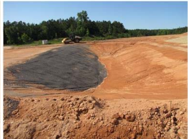
(b) first half of the pond lined with RAP
