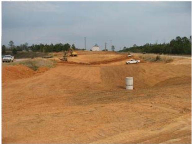
(b) final grade of the retention pond
