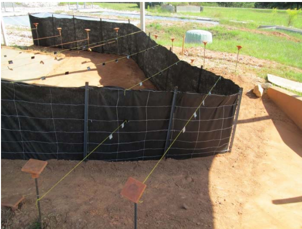
(a) standard ALDOT installation w/ extended sides
