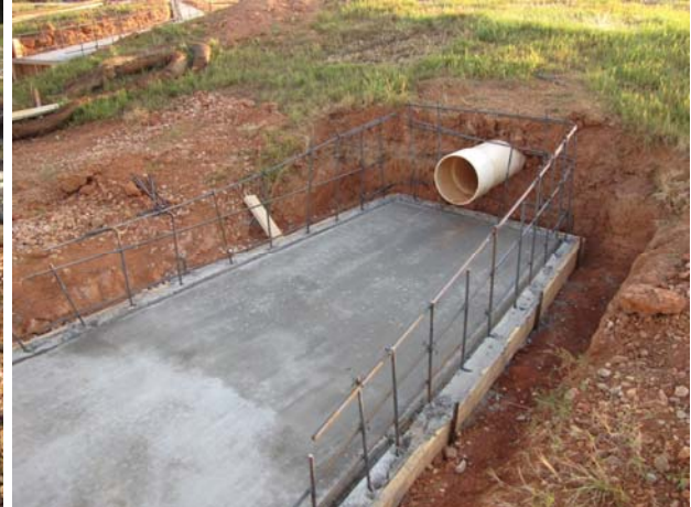
(b) slab and reinforcement
