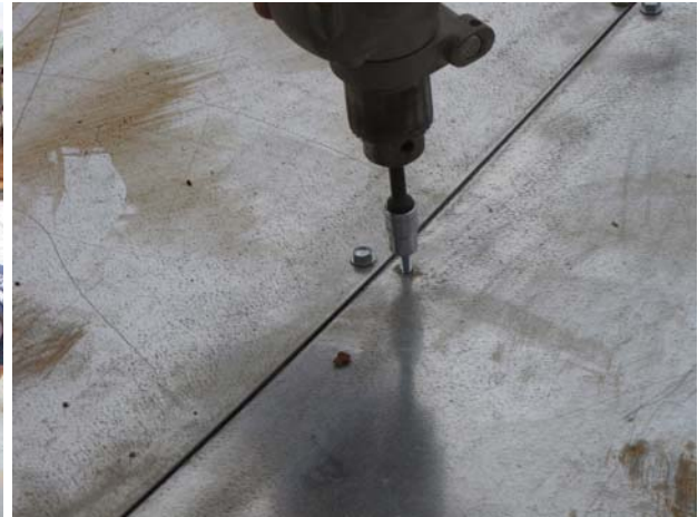
(b) seaming together liner sections
