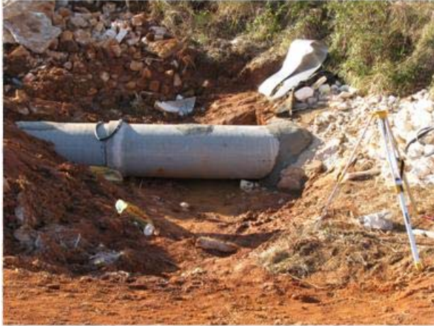
(a) 24 inch RCP tied into existing culvert
