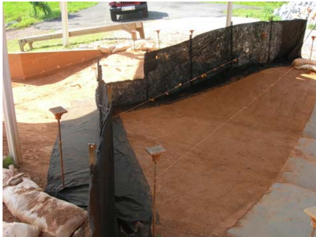
(a) underlay and pinning of fence
