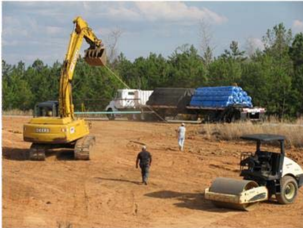
(a) truck bed of Akwaseal rolls
