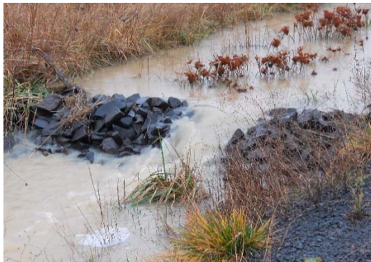
(a) rock ditch check ponding flowing runoff
