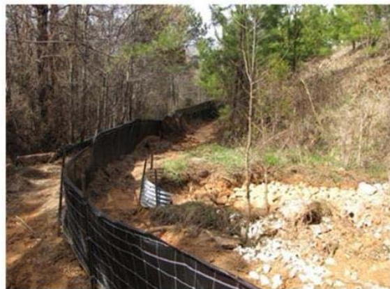
(b) outlet side of concrete culvert
