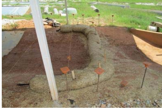
(f) downstream staking w/trenching
