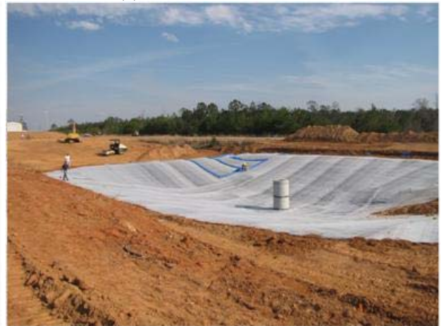
(d) retention pond liner completely unrolled
