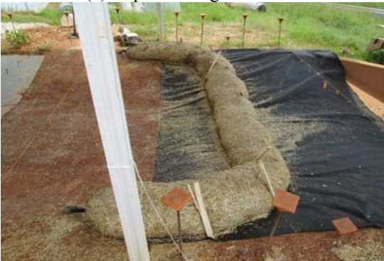
(g) teepee staking w/8 oz. FF + trenching
