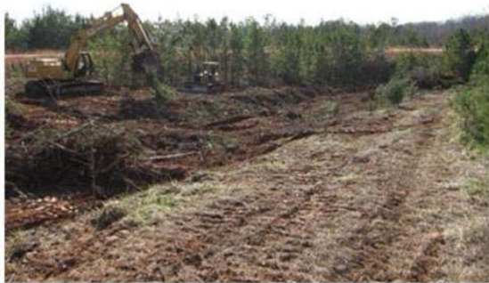
(c) clearing and grubbing stage
