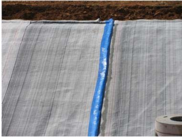
(e) seaming together of liner using granular bentonite
