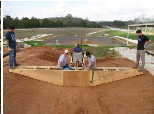
(b) fine grading using mold
