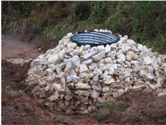
(c) final installation of ESCP temporary riser
