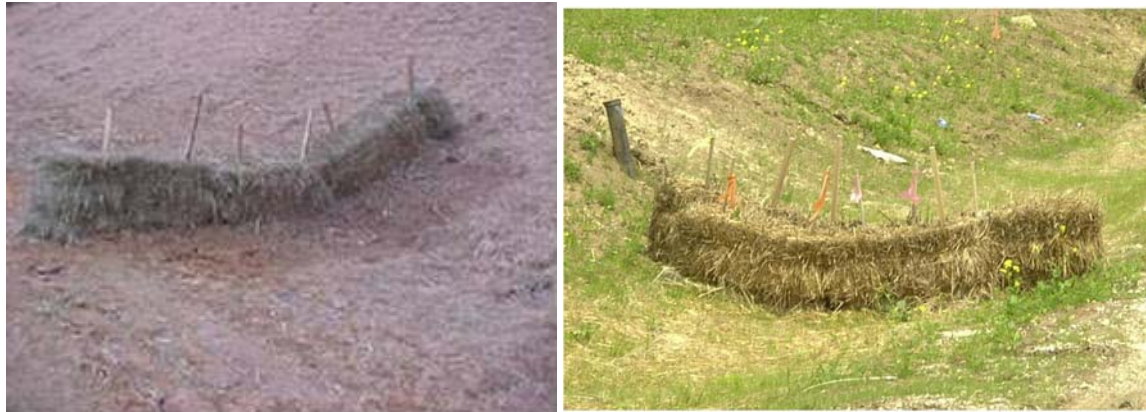
(a) typical hay bale installation on bare soil
