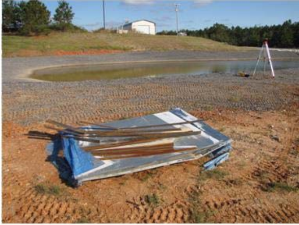
(a) sheet metal channel liner and angle iron
