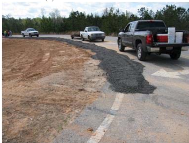
(c) RAP berm constructed to convey runoff
