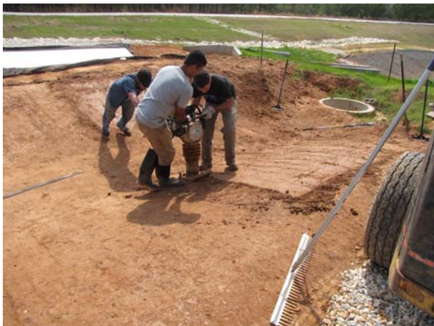
(a) grading and compaction
