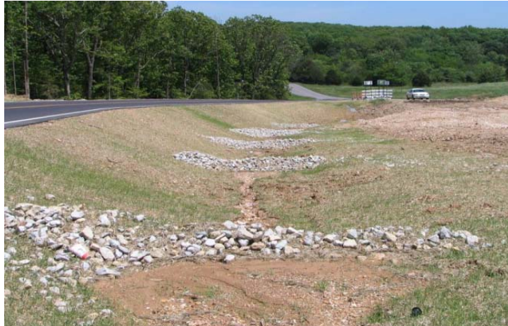
(c) rock ditch checks retaining sediment
