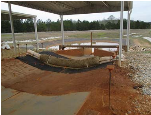
(e) East Coast Erosion: EC Wattles 100% Agricultural Straw
