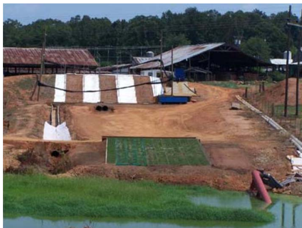
Figure 2.7: TRI's Denver Downs Research Facility (TRI 2010).
