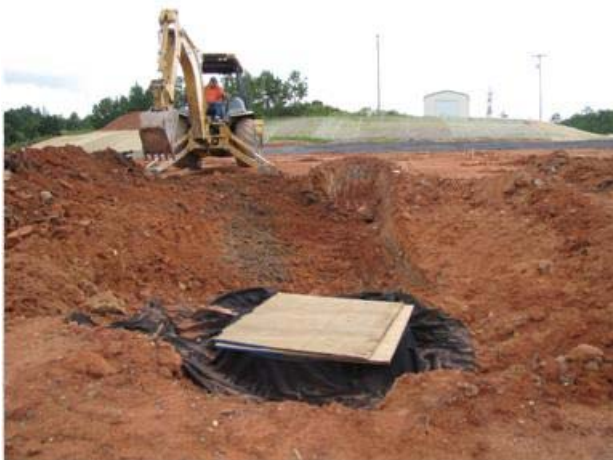
(c) rough excavation of the middle drop inlet testing channel
