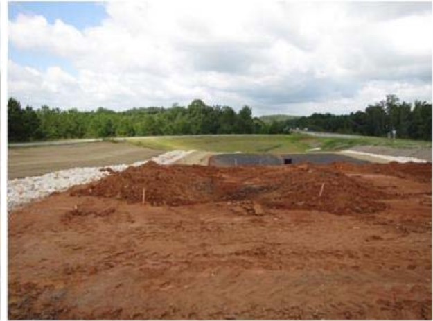
(b) rough excavation of the left test channel
