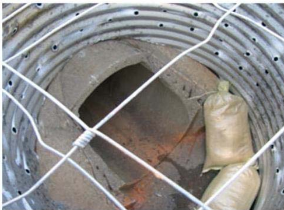
(a) perforated riser pipe installed over existing 24 inch reinforced concrete pipe
