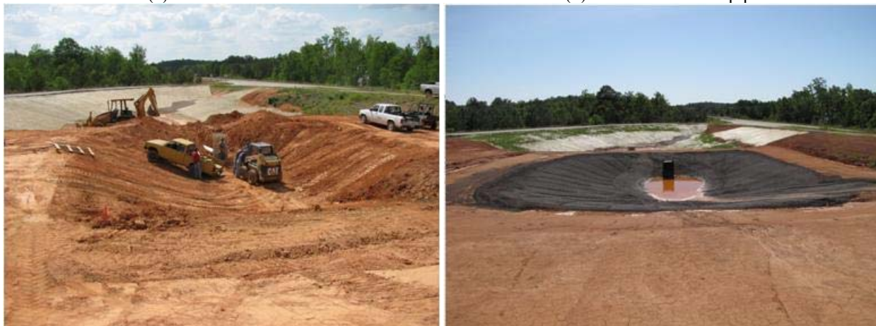
(c) rough grade of the sediment basin
