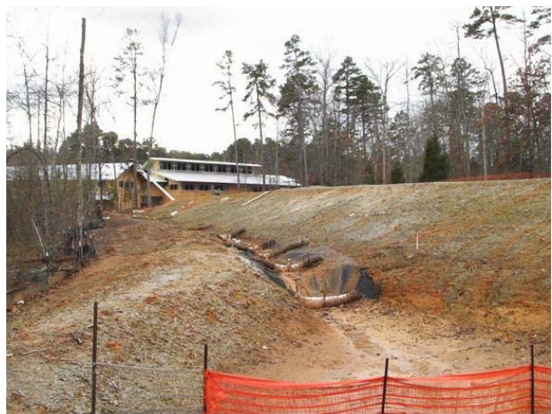
(b) fiber check dam and PAM dosing test channel
