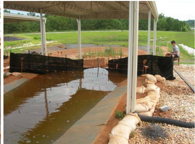
(b) resulting impoundment pool
