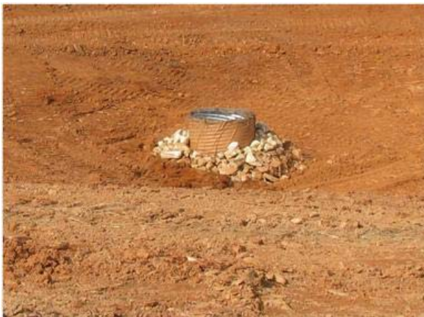
(a) temporary riser pipe relocation
