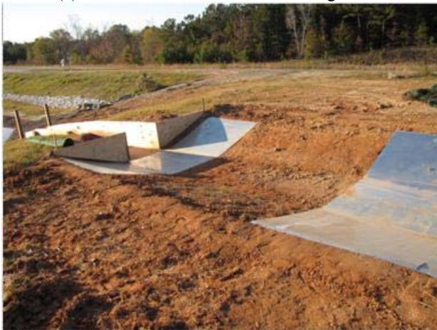
(c) earthen section of the channel after liner installation
