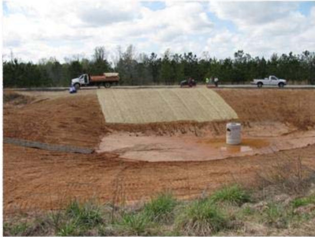
(a) installation of new ECBs
