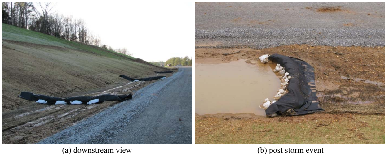
Figure 2.15: Sand Bag Ditch Check on ALDOT Project in Franklin County, AL.
