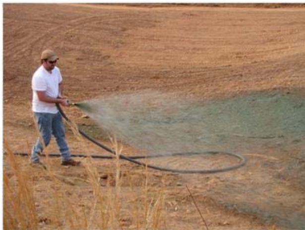
(c) hydromulching pond banks
