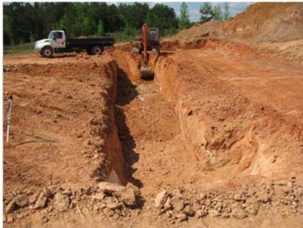
(a) initial excavation of the storage pond
