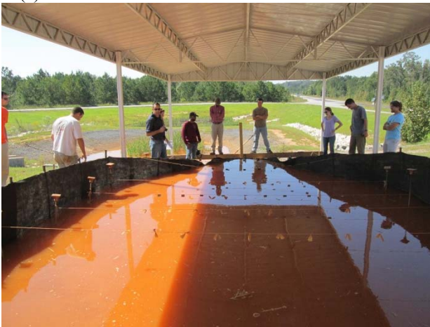
(c) silt fence full pool length
