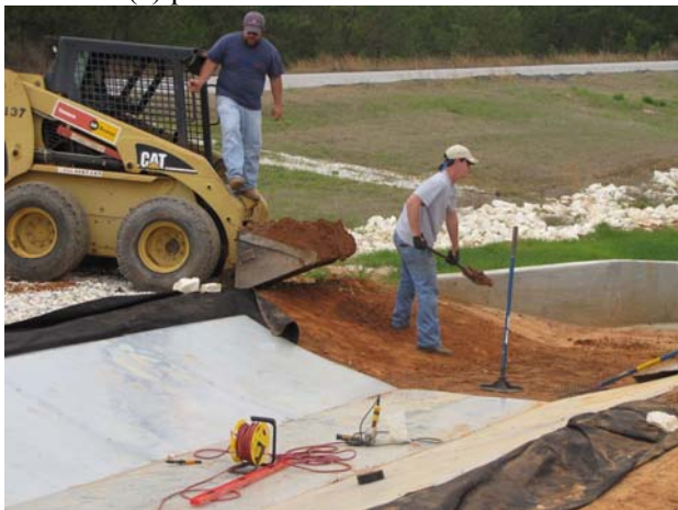
(c) grading of installation area
