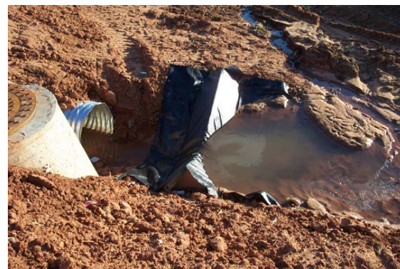
(b) silt dike ditch check protecting culvert
