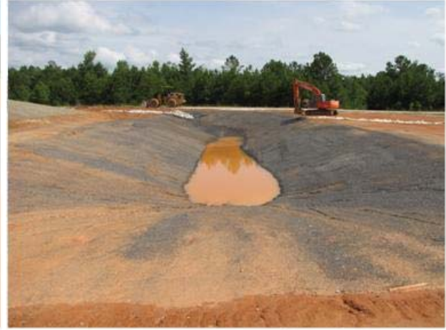
(d) completed lining of the storage pond
