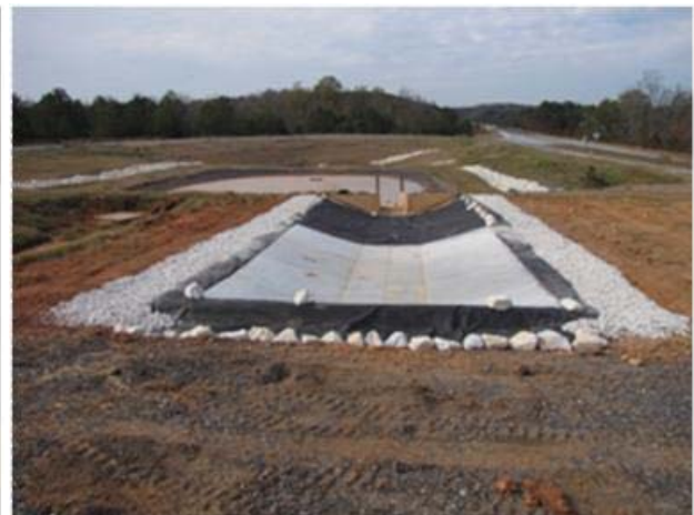
(f) final installation of the channel prototype
