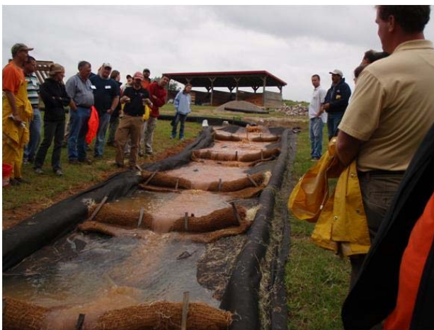
(a) ditch check spacing performance channel
