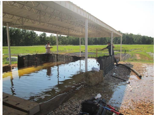
(b) full pool w/ flow overtopping channel banks
