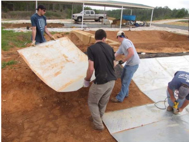
(a) placement of sheet metal liner
