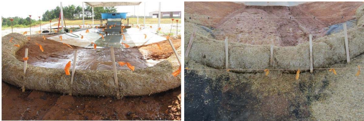
(a) downstream staking + trenching
