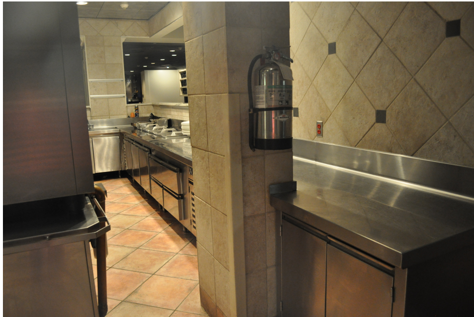
Figure 42: Photo of restaurant kitchen structural column
