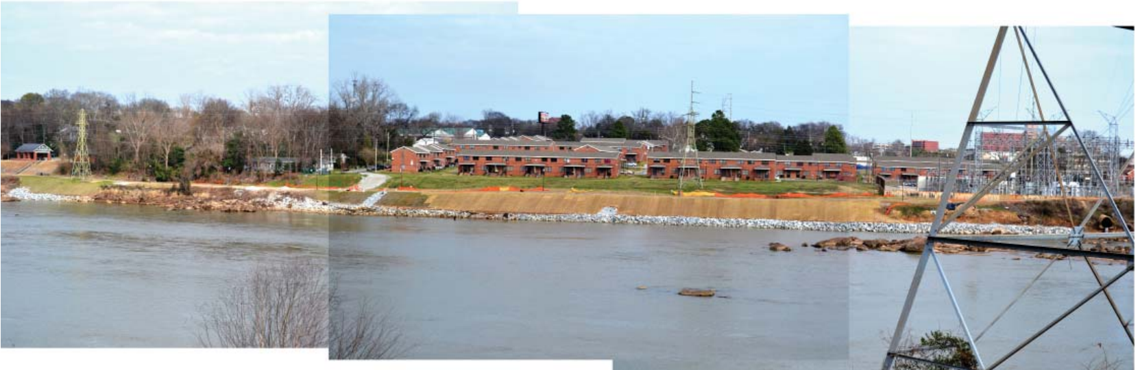
TOP: View of the design site from across the Chattahoochee River BOTTOM: Looking north towards the design site
