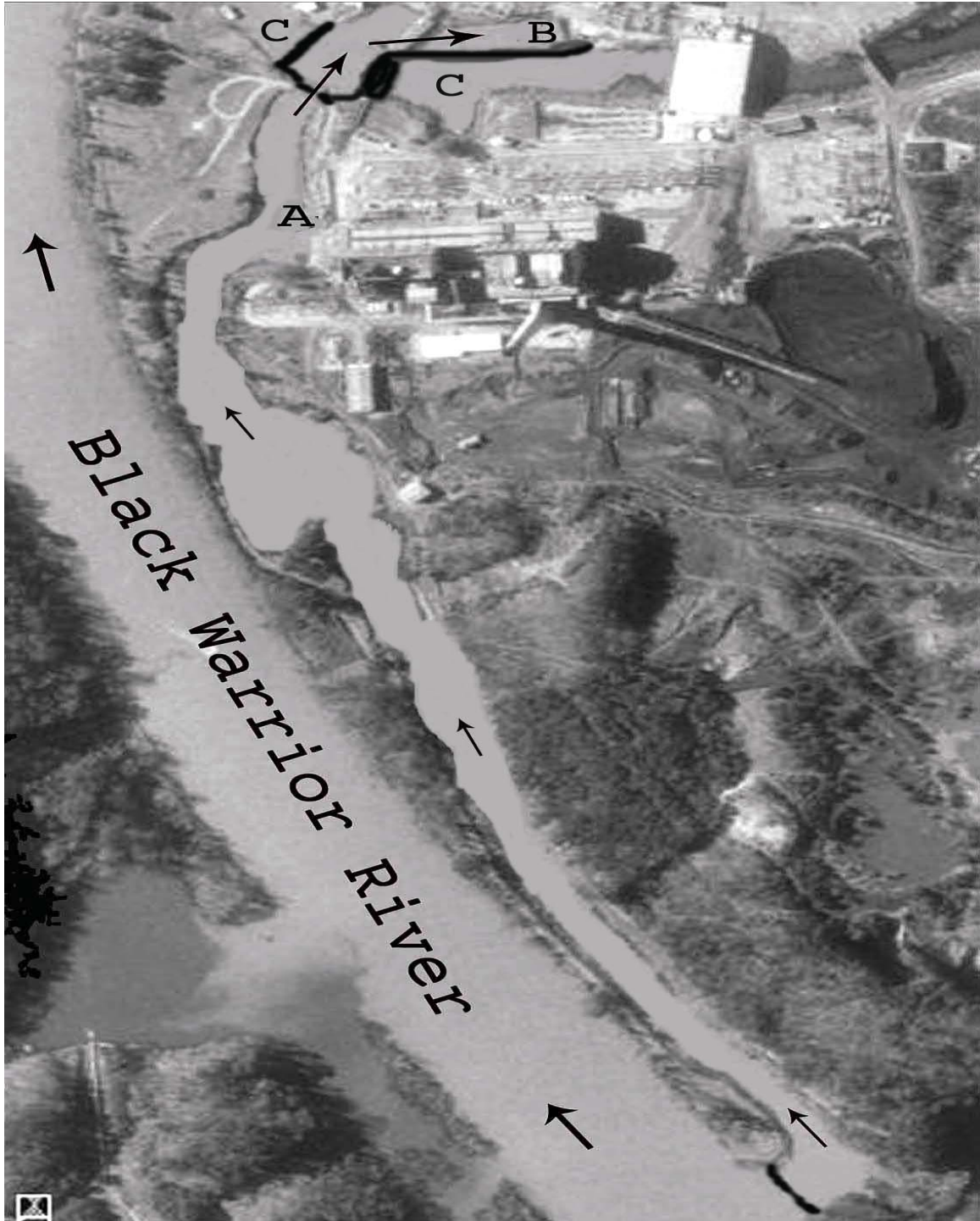
FIGURE 4. – Intake canal diagram and location of cooling water intake structures for Gorgas Steam Plant located on the Mulberry Fork of the Black Warrior River, Alabama (U6-U7 intake located at point A, U8-U10 intake located at point B and the discharge canal is located at points C. Arrows indicate river and intake flow).
