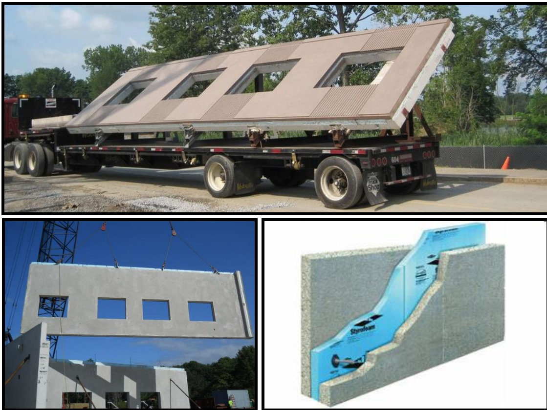
Figure 2-3: Precast/Prestressed Sandwich Wall Panels
