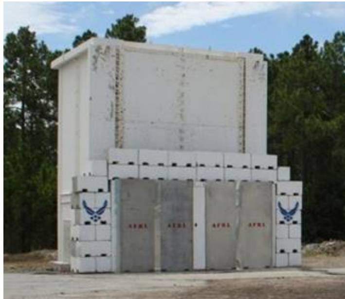
Figure 3-26: Single Span Reaction Structure for Full-Scale Dynamic Tests (Naito et al. 2011b)
