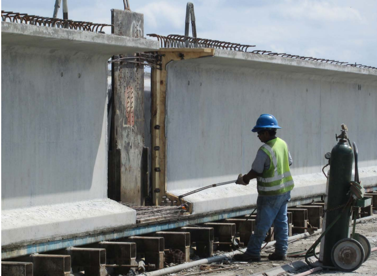
Figure 3.22: A Worker Cutting the Bottom Strands
