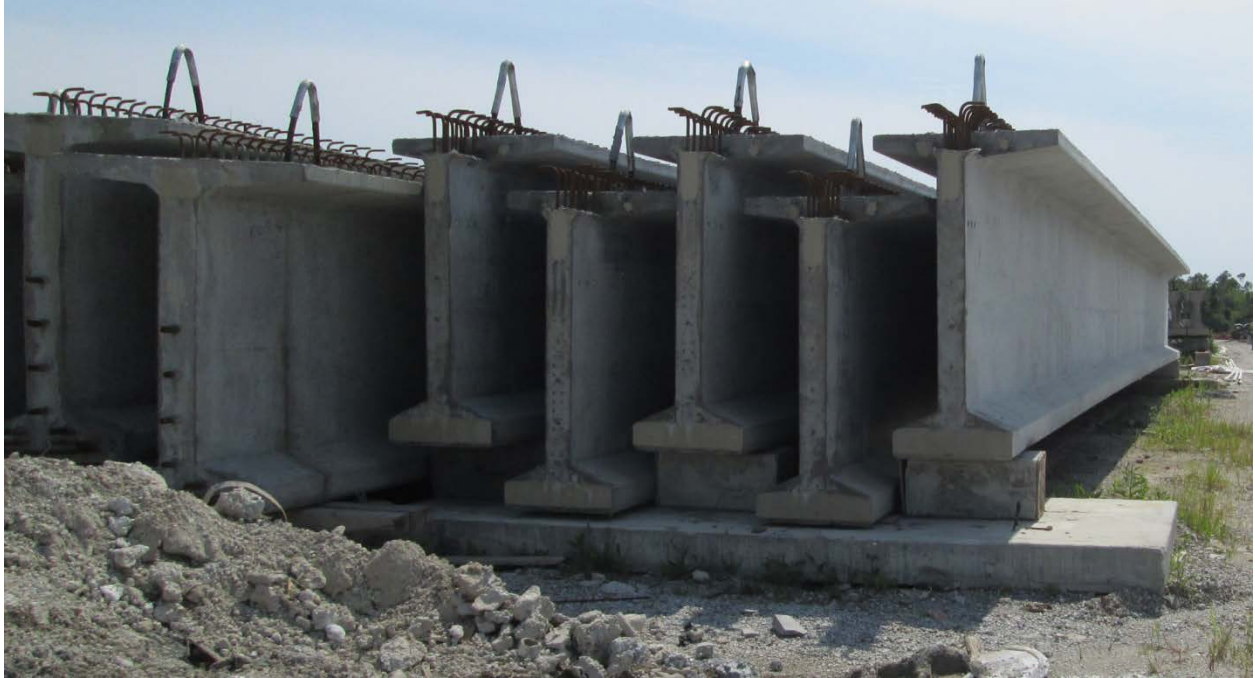
Figure 3.26: Example Girder Storage Conditions for Plant C
