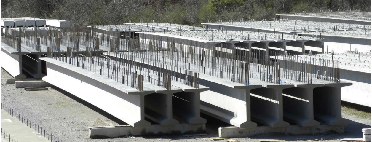
Figure 3.24: Example Girder Storage Conditions for Plant A
