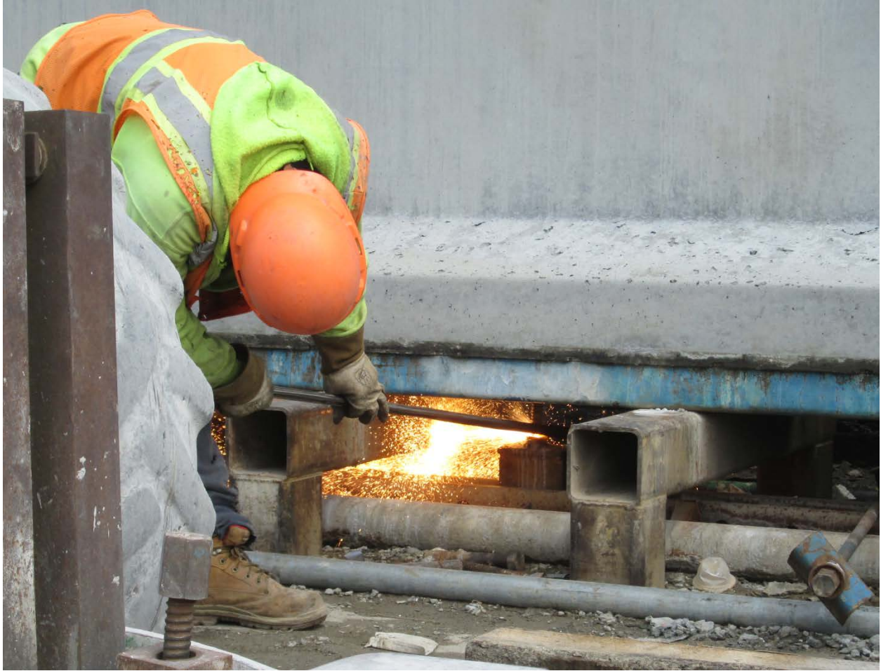
Figure 3.21: Cutting of a Tie-Down Connection
