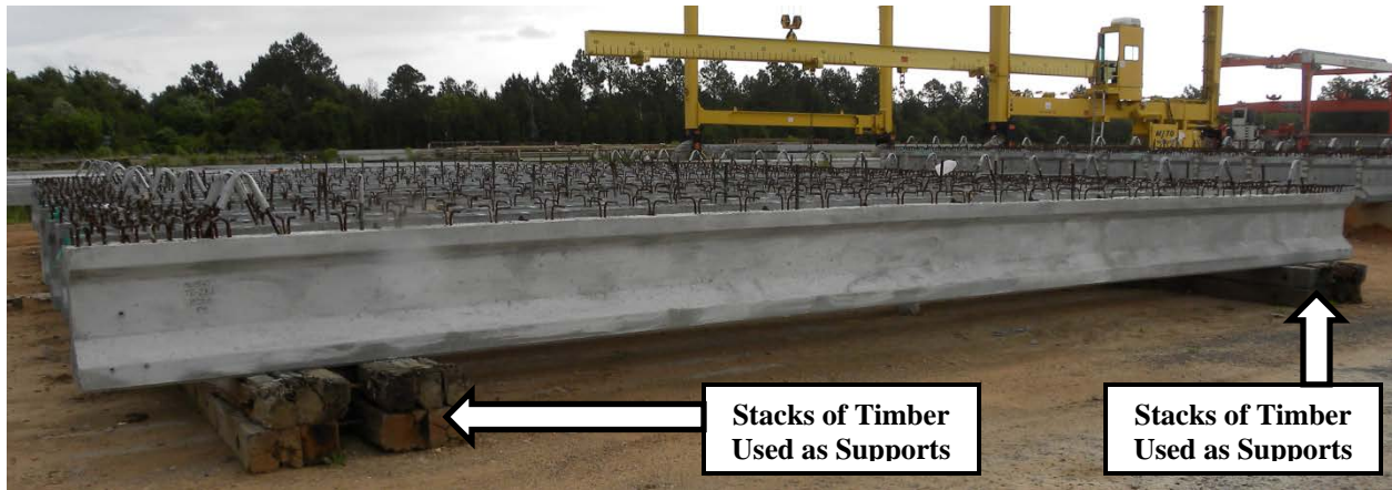
Figure 3.29: A Pile of Timber Used as Girder Supports
