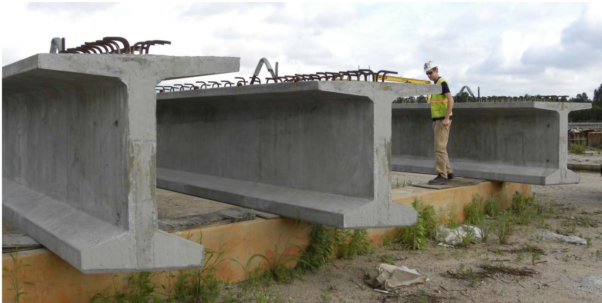
Figure 3.27: Example Girder Storage Conditions for Plant D
