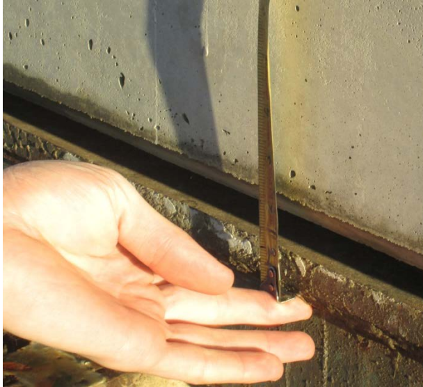
Figure 3.23: Measuring the Initial Camber of a Girder after Release
