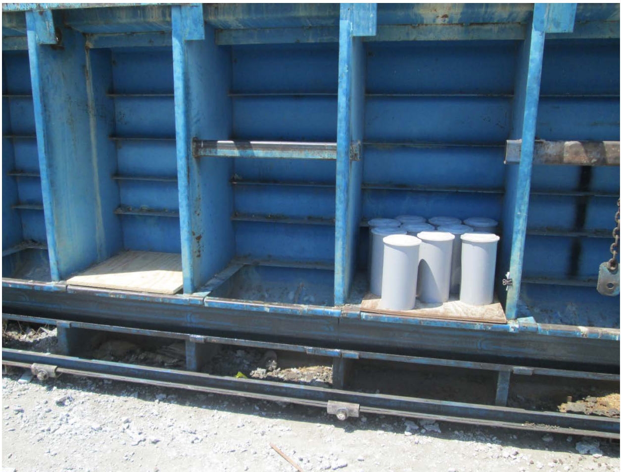
Figure 4.9: Plant Placement of Cylinders during Girder Curing
