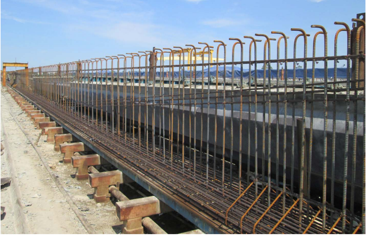
Figure 3.10: Tensioned Strands, Hung Rebar, and Diaphragm Inserts in Plant C
