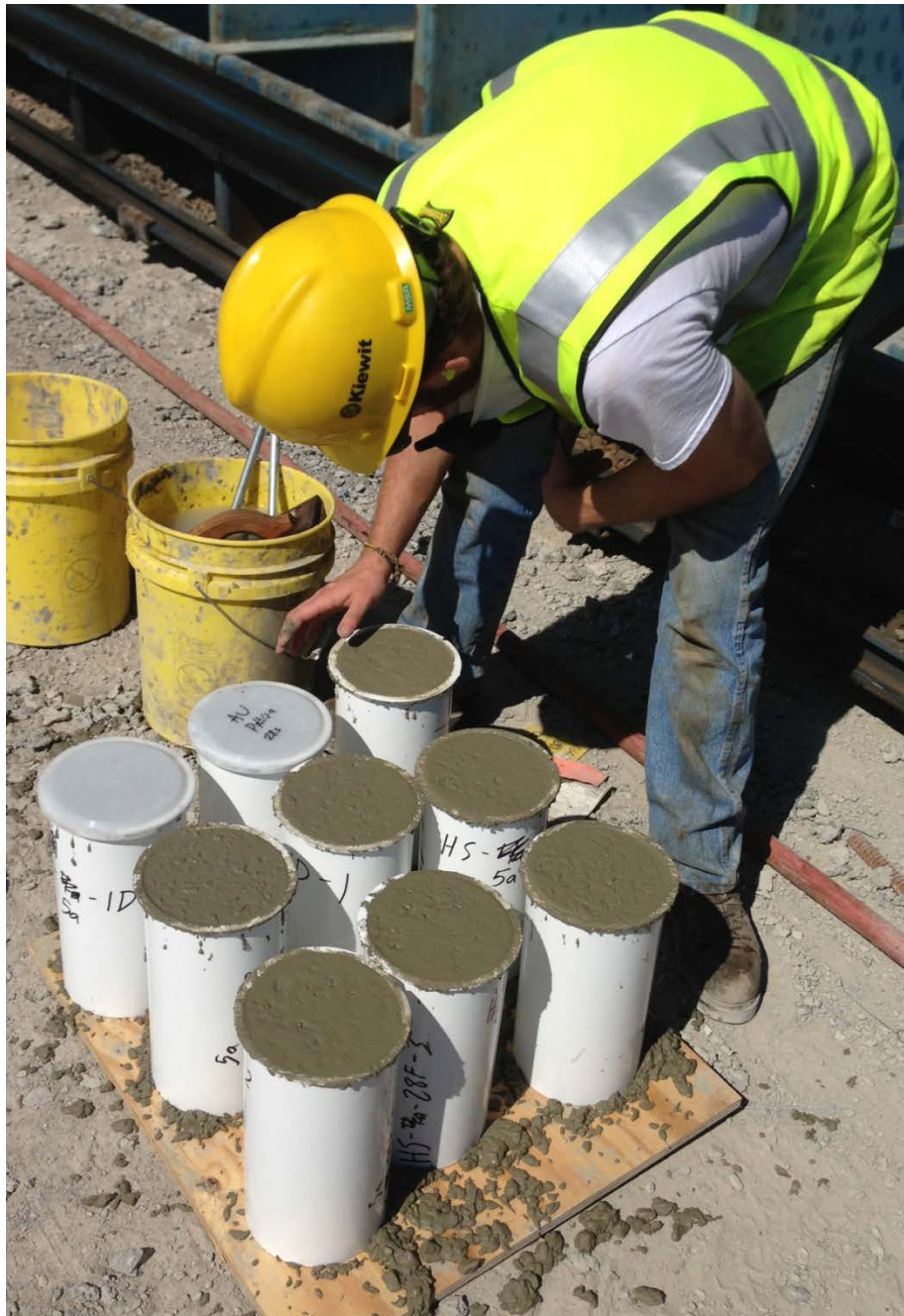
Figure 4.8: Cleaning and Capping Test Cylinder Specimens
