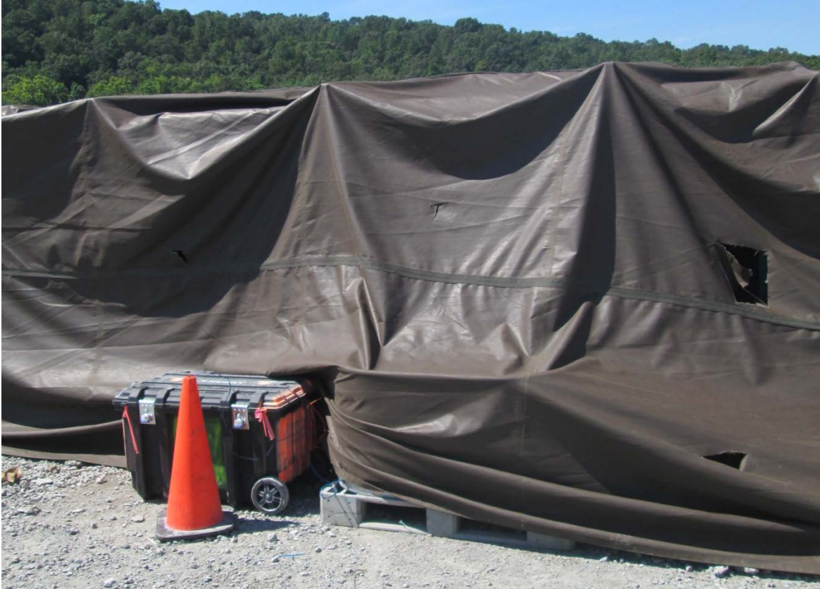
Figure 4.11: Curing Tarp Coverage Conditions
