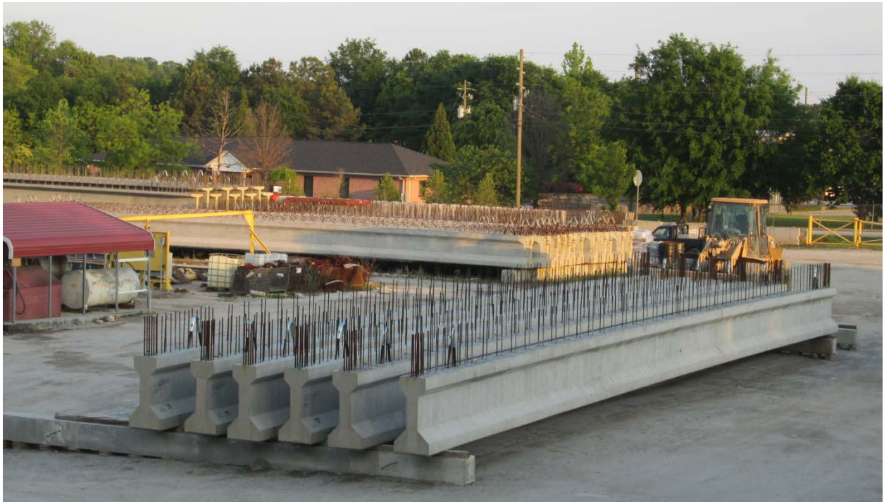
Figure 3.25: Example Girder Storage Conditions for Plant B
