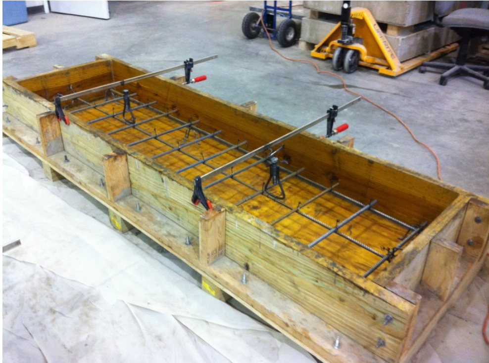
Figure 3-9: Tied reinforcing bars for a slab element
