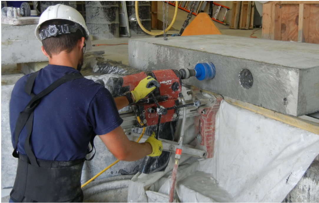
Figure 3-25: Core rig mounted to AU Structural Engineering Laboratory loading dock
