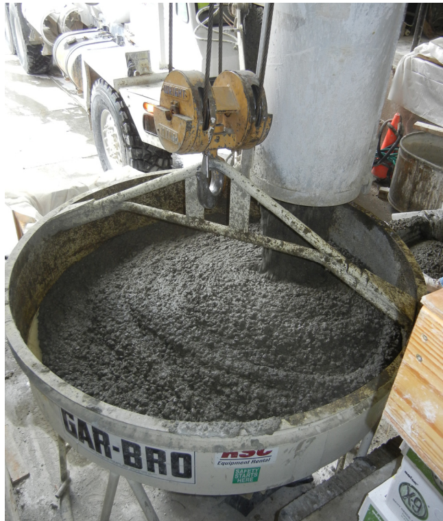
Figure 3-14: Placing concrete into placement bucket
