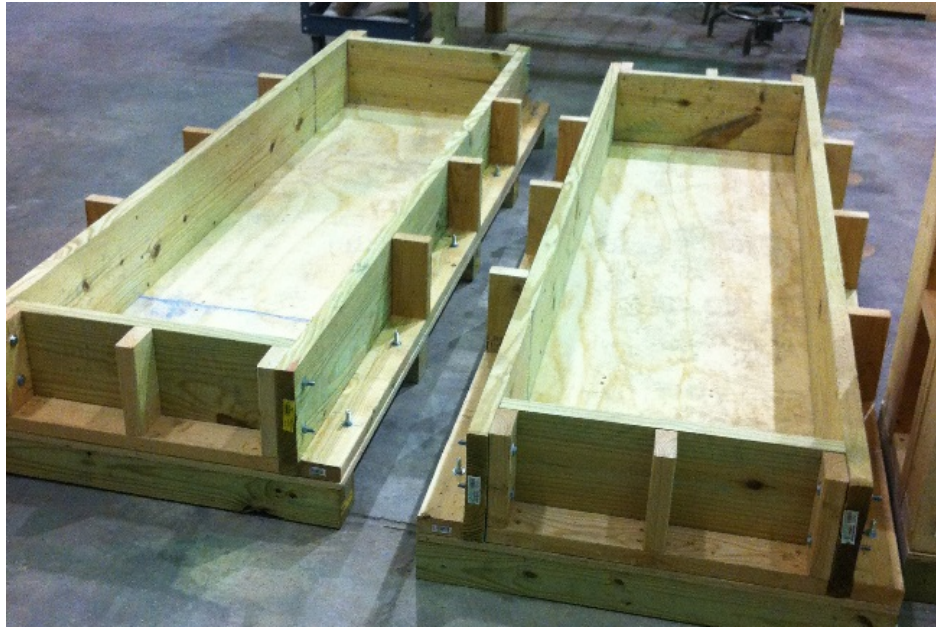
Figure 3-5: Constructed forms for two identical slab specimens
