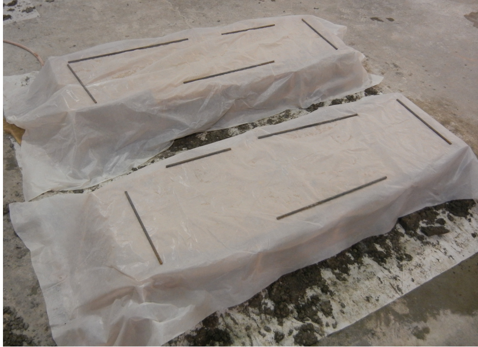
Figure 3-18: Slabs covered in burlap and wrapped in plastic
