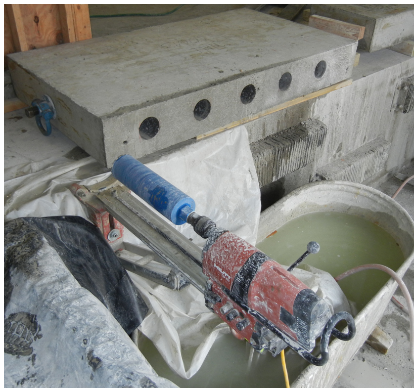
Figure 3-24: Collecting slurry when coring parallel cores from wall
