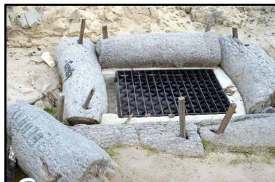
(b) In-Field Installation
