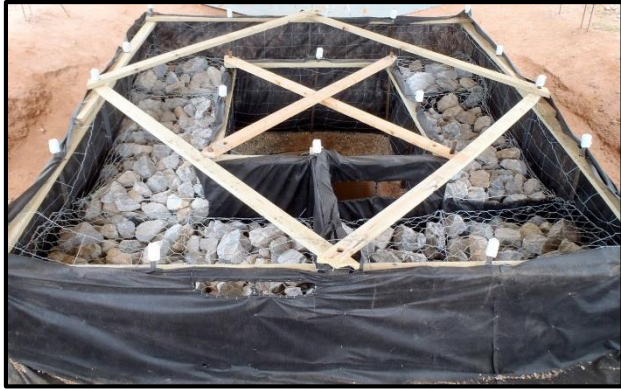
(b) Weir Placement
