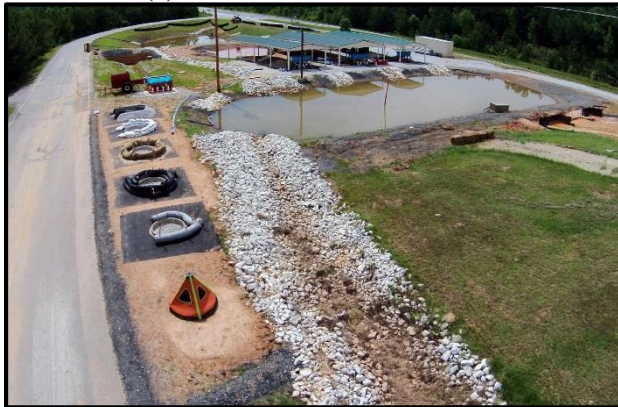
(c) Installed IPPs in Mock Inlets
