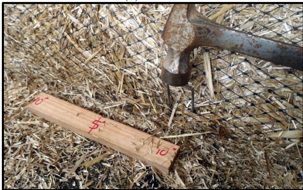
(f) MFE-I Sod Staple Installation
