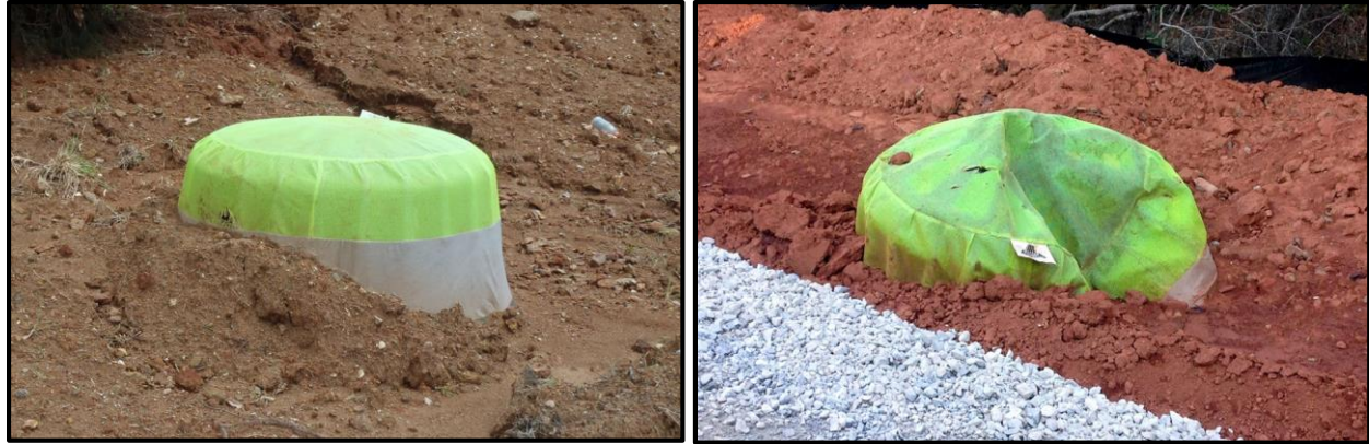
(a) Installation on Bare Soil
