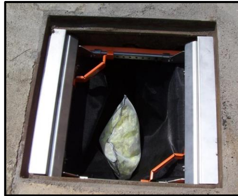
(b) Square Assembly Installed
