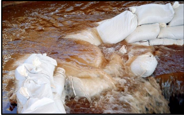
(b) ALDOT Standard Installation Failure
