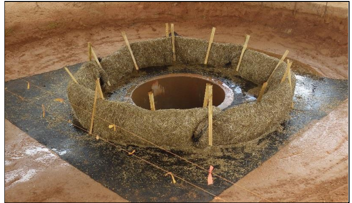
Figure 1: Wattle Barrier Installation
