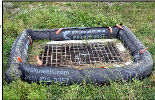
(b) Installation on Pervious Surface
