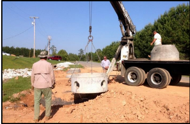
(b) Installation of Mock Inlet Structures
