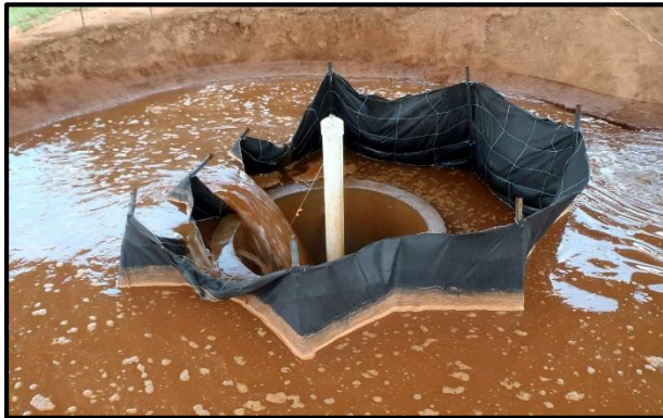
(c) Hexagonal Configuration Failure
