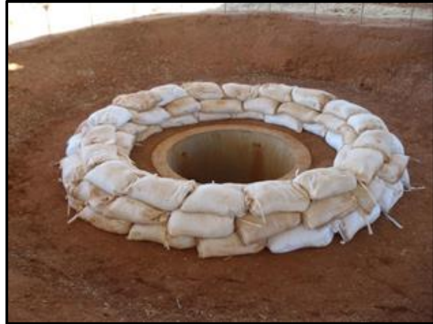
(b) sandbag inlet protection
