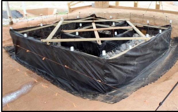
(a) Test Channel Installation
