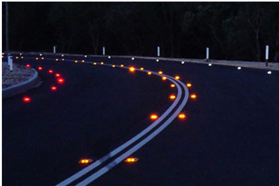
Figure 2.10: Two-Lane Road Well-Delineated by LED Road Studs
