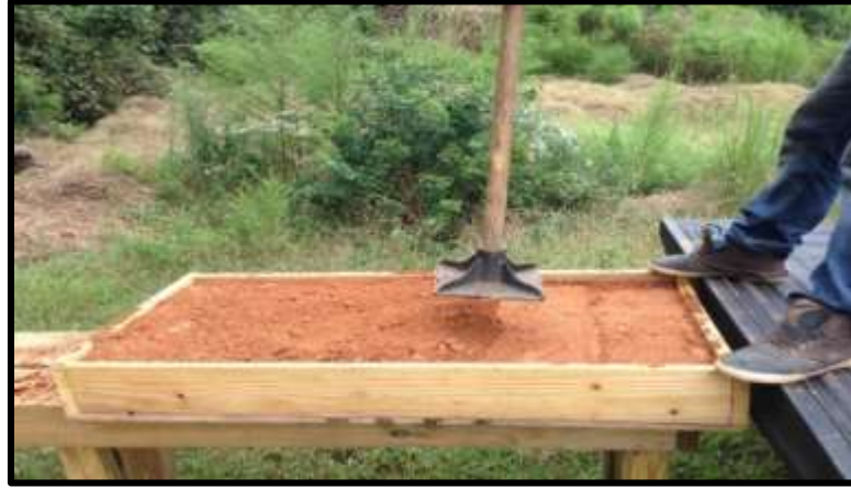
Figure 3.10: Compaction of soil boxes (119 cm x 56 cm) by hand tamping
