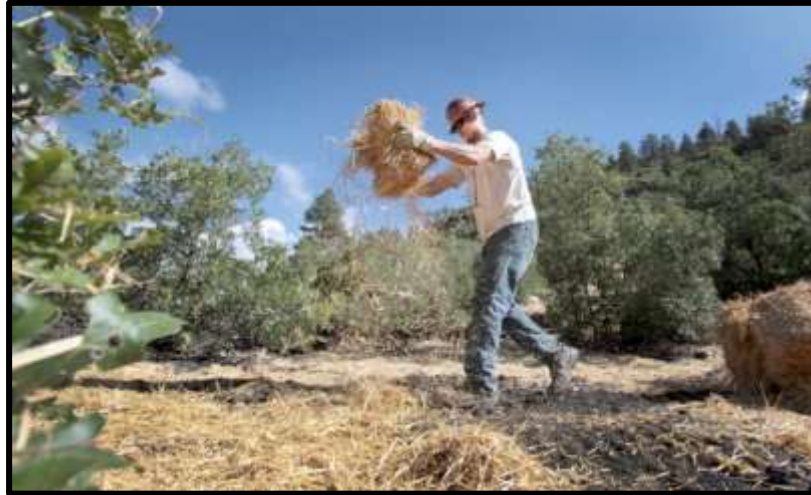
Figure 2.1: Application of wheat straw by hand over a freshly seeded area to reduce erosion in Boston, MA (Source: http://www.durangoherald.com )
