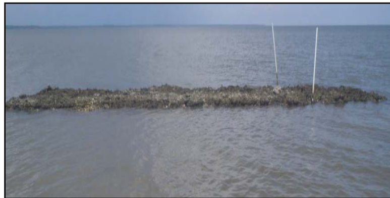
Figure 2.8 Photograph of oyster shell bags used for oyster reef restoration in Portersville Bay, Alabama.
