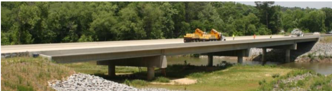
Figure 3-1: Hillabee Creek Bridge (Span 1 in Foreground)
