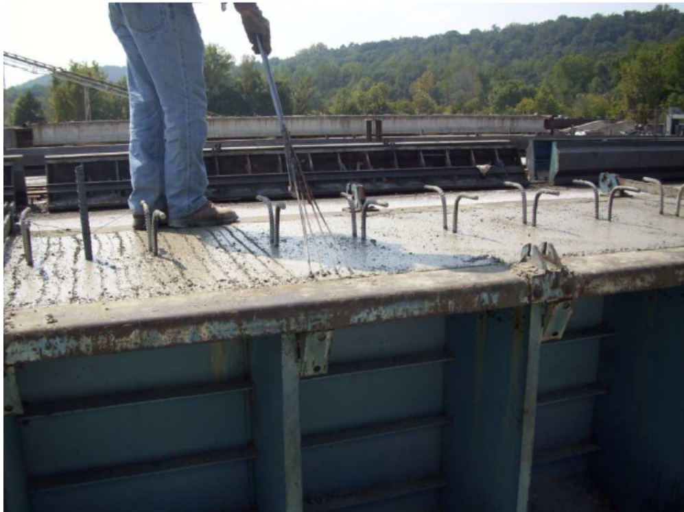
Figure 3-36: Surface Roughening of SCC Girders
