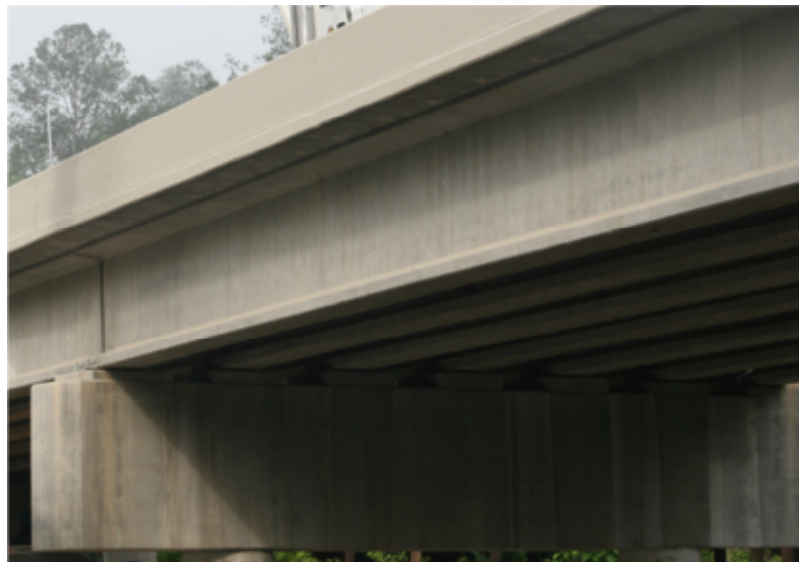
Figure 3-3: Span 2 BT-72 Girders
