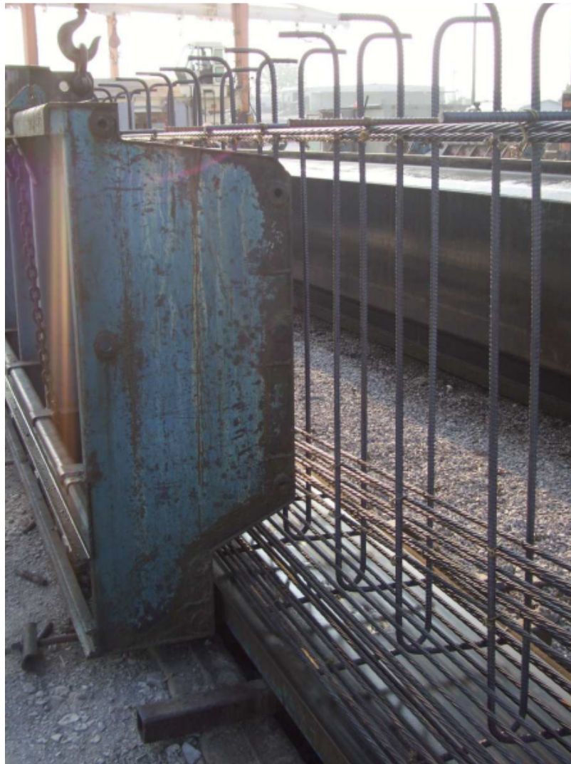
Figure 3-32: Side Form Installation
