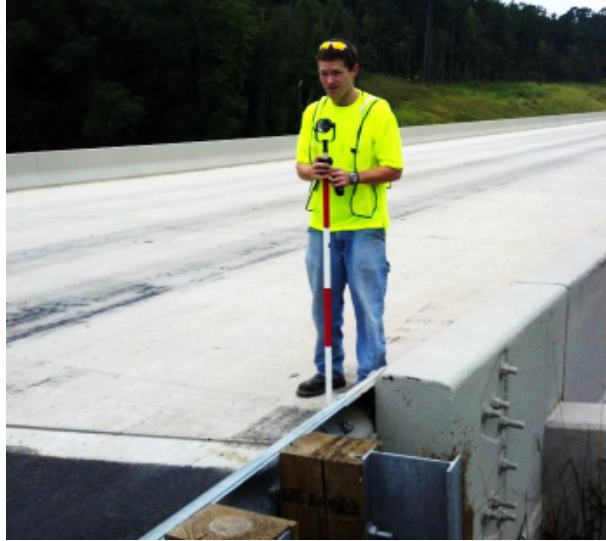
Figure 4-4: Deck Surveying Method Camber Measurements
