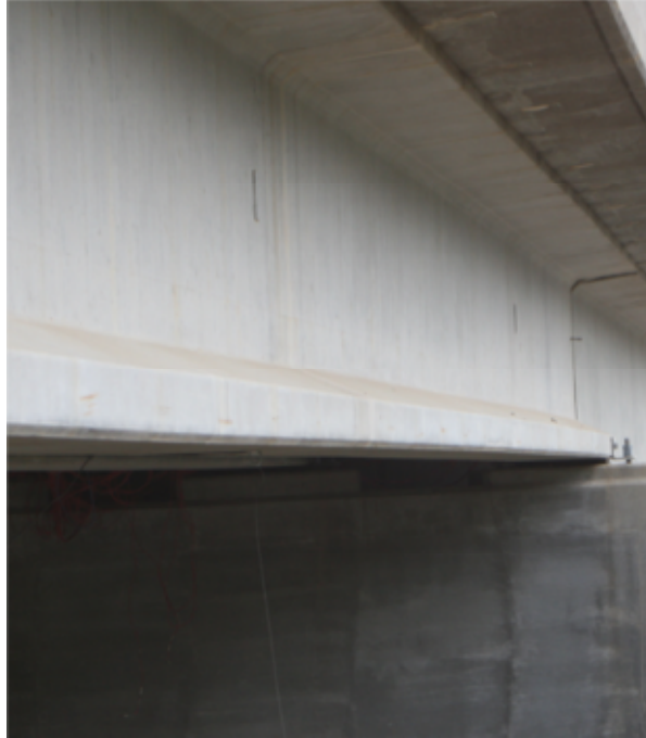
Figure 3-2: Exterior CVC BT-54 Girder in Span 4
