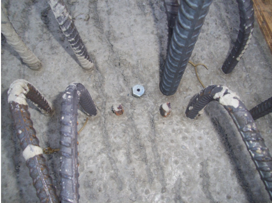
Figure 4-1: Surveying Target in Place
