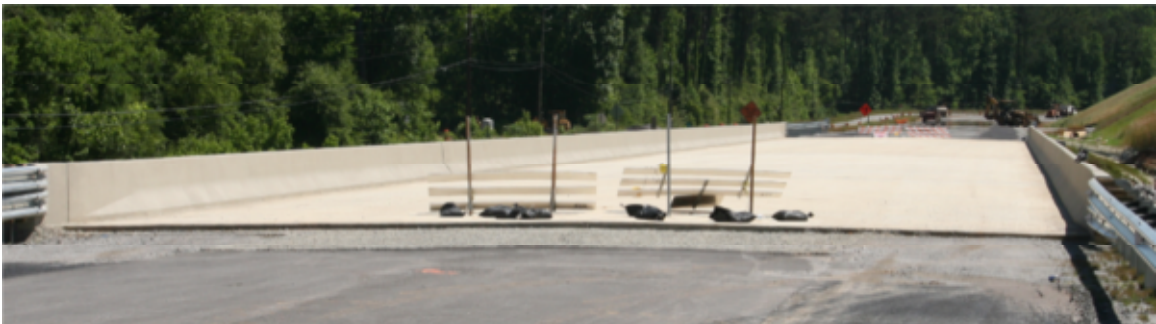
Figure 3-6: Bridge Deck and Barriers in Place
