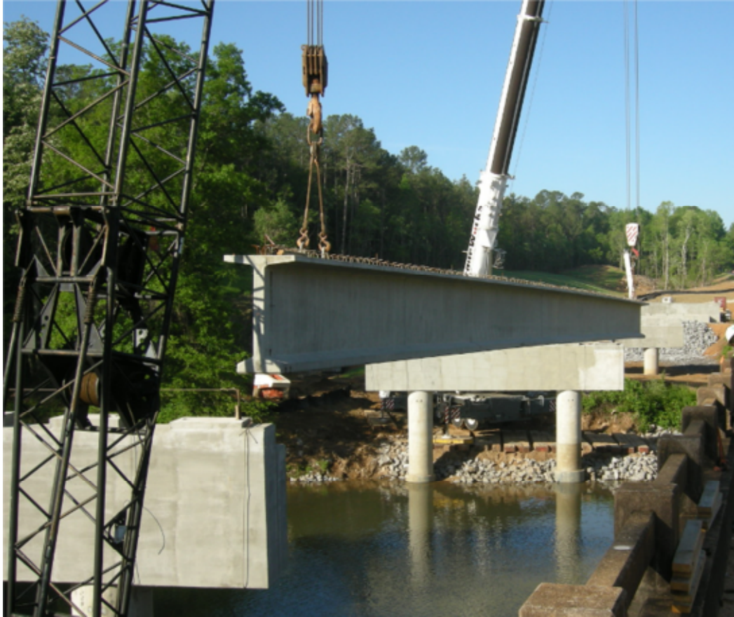
Figure 3-9: Erection of a VC Girder in Span 3
