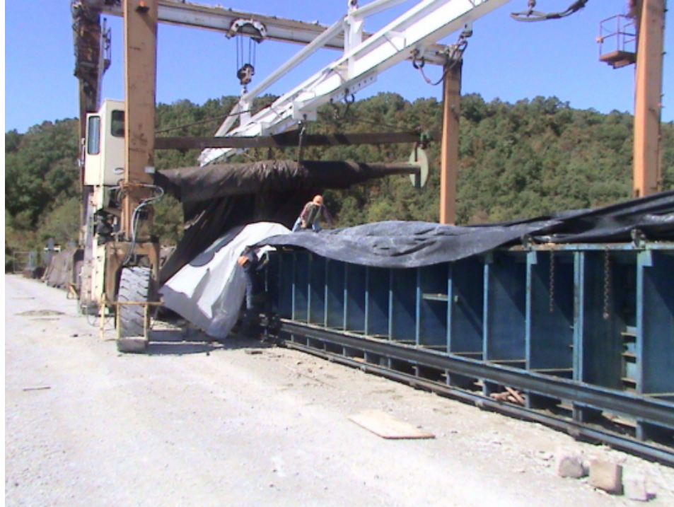
Figure 3-38: Curing Blanket and Tarp Covering
