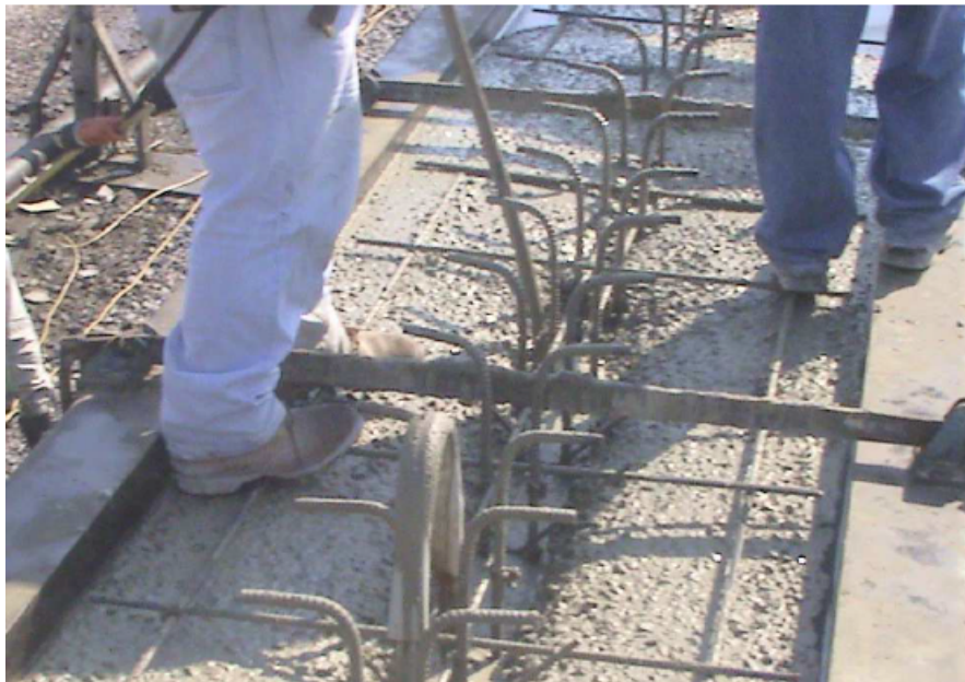
Figure 3-34: Internal Vibration Used in VC Placement
