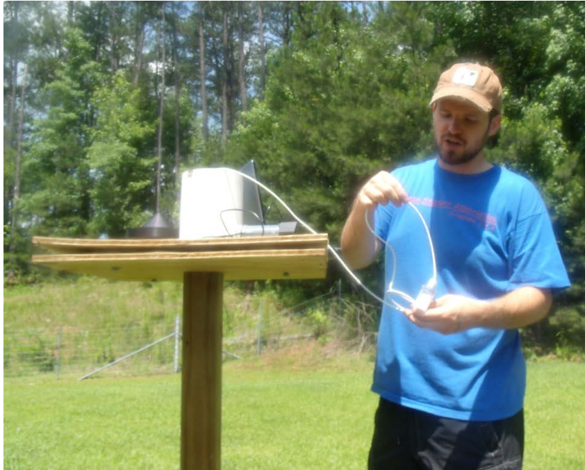
Figure 3.5: Installed Rain Gauge behind the gas station on Liles Lane off I-59. The 4x4 post holding up the platform is approximately 6ft high. A ladder is used to access the rain gauge.
