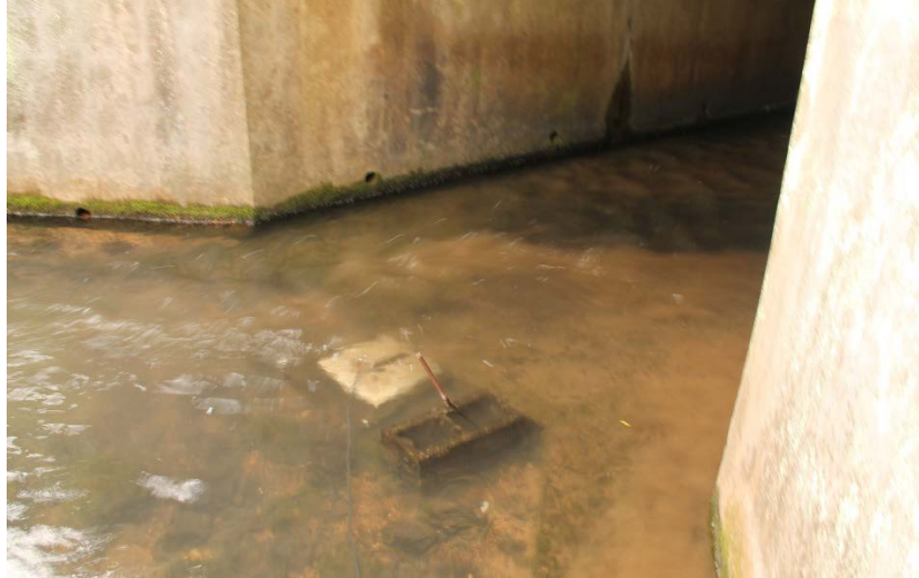
Figure 3.7: Area-Velocity Sensor attached to a thin metal sheet secured to a cinder block located upstream of interstate.
