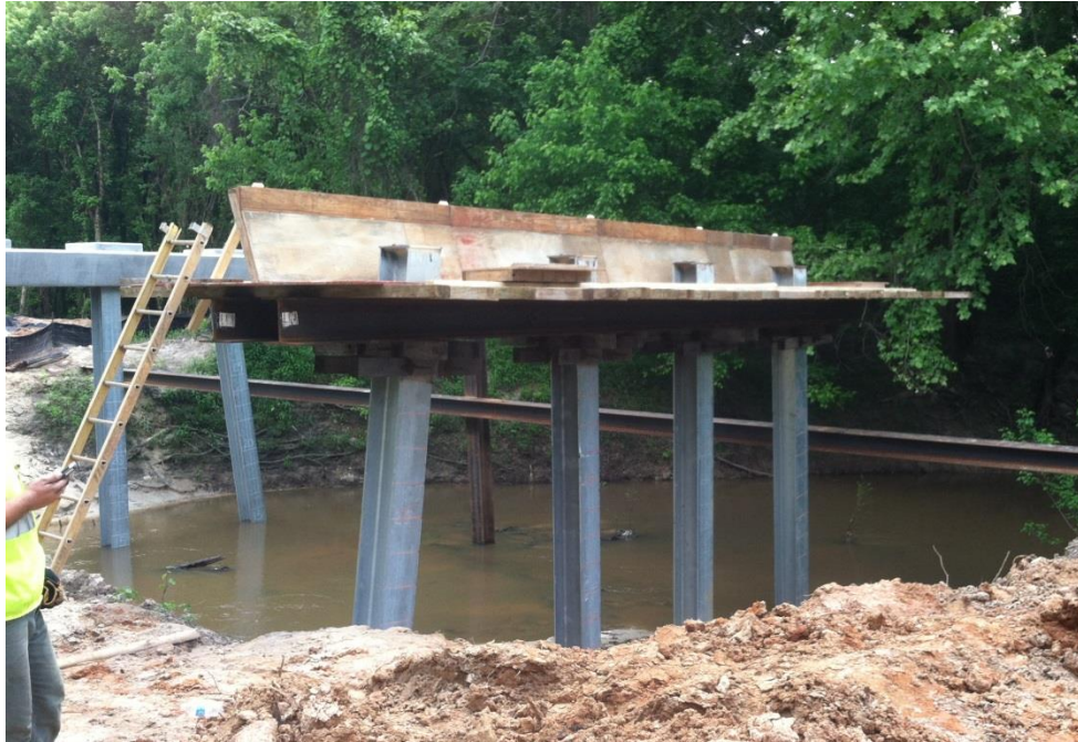
Figure 2-7 Bent Cap Formwork Being Positioned
