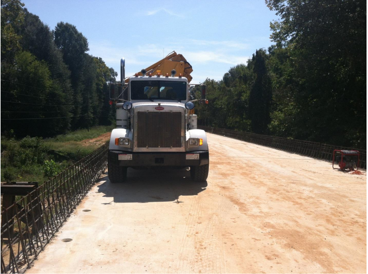
Figure 4-6 ALDOT Load Truck Positioned at Edge of Roadway
