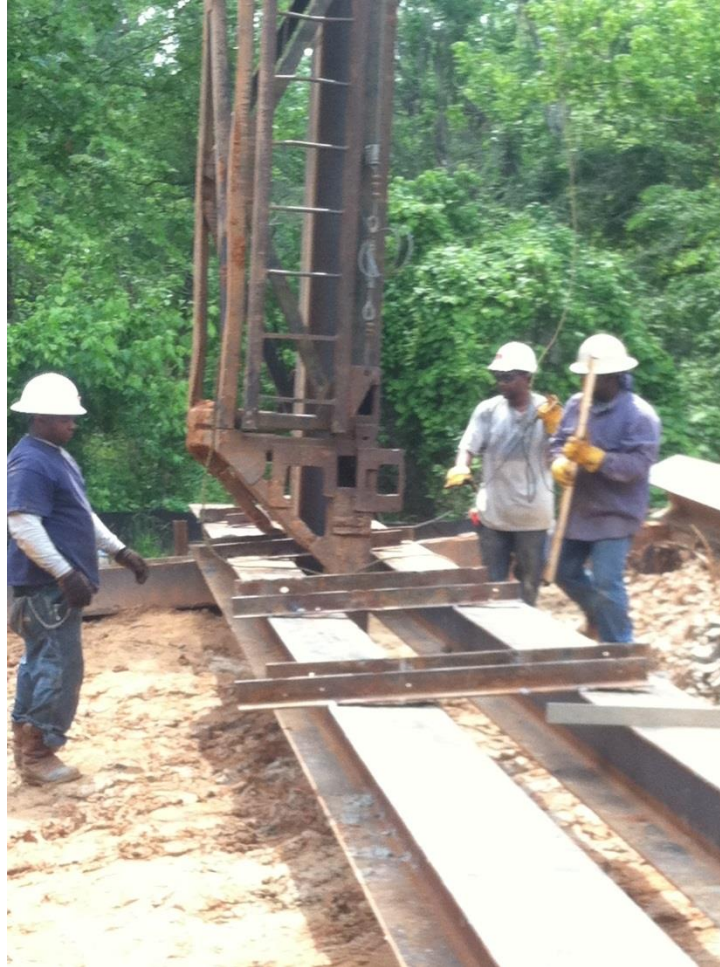
Figure 2-4 Diesel Hammer Being Lowered Into Driving Template
