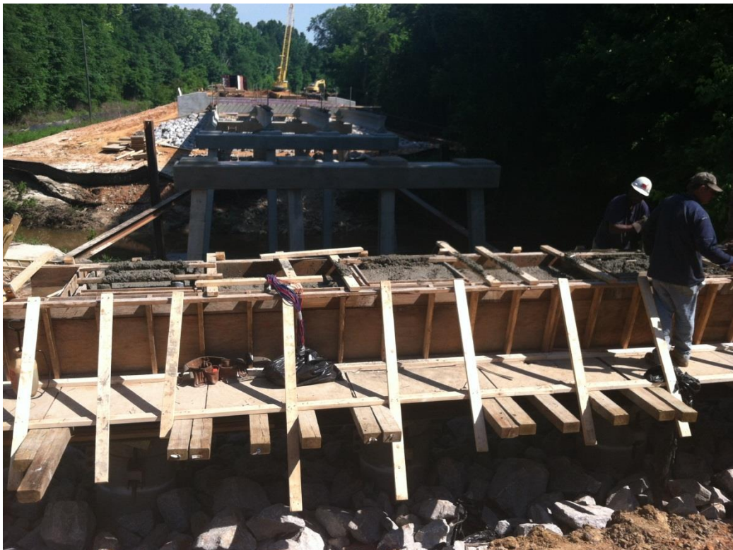
Figure 2-9 Casting of Concrete Bent Cap
