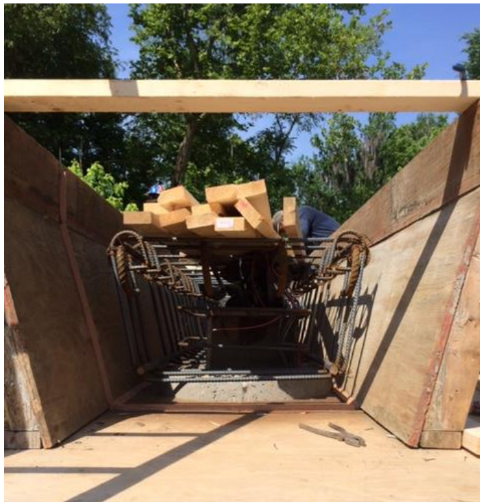
Figure 2-8 Cap Reinforcement Cage Prior to Concrete Placement
