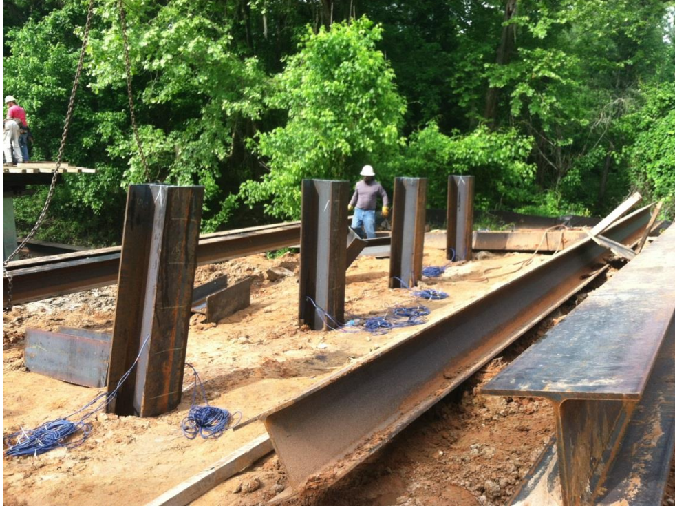
Figure 2-5 Piles Following Cut-Offs at Top of Pile Elevation
