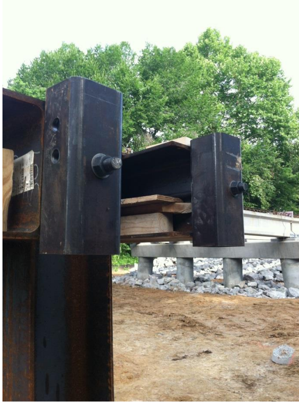
Figure 3-18 Threaded Rod End Anchorage at Reaction Frame
