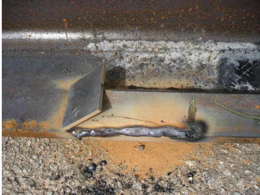
Figure 3-6 Protective Angle Welded to Pile Flange
