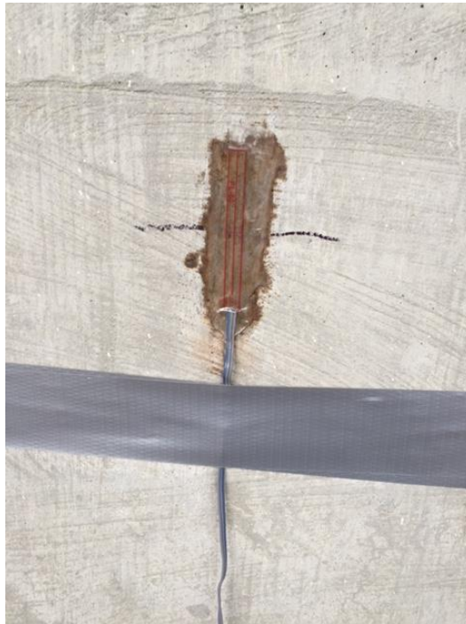
Figure 5-5 Installed Concrete Surface Strain Gage
