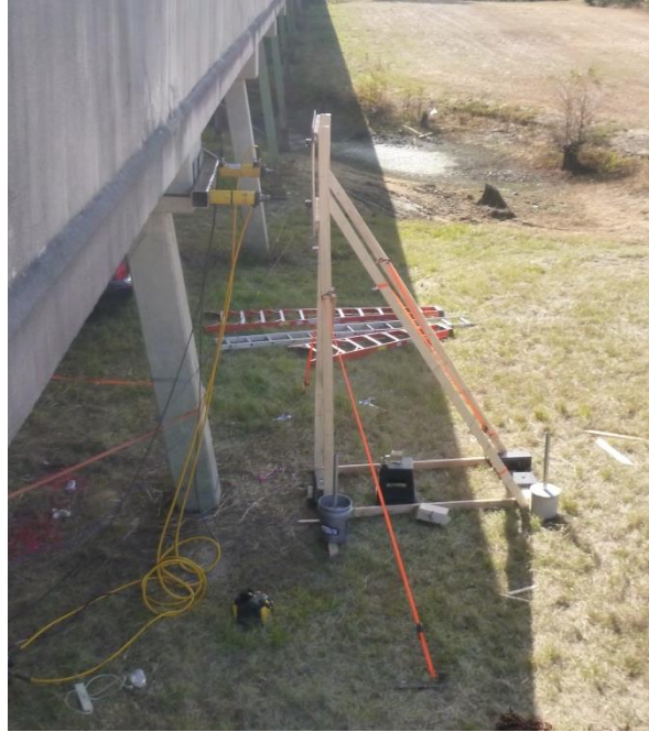
Figure 5-13 Wooden Reference Frame for Wirepots
