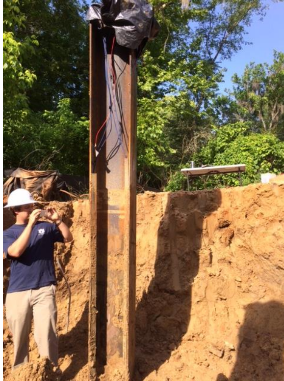
Figure 2-6 Driven HP Pile Following Excavation for Encasement Placement
