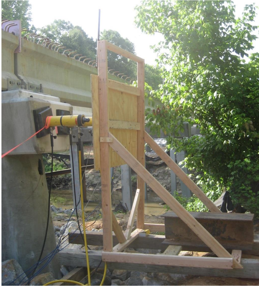
Figure 3-24 Wooden Reference Frame for Wirepot Installation
