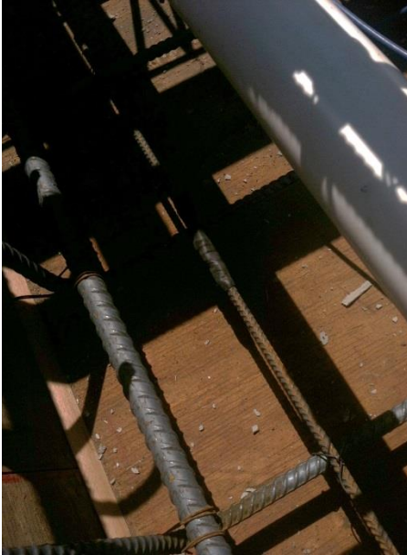
Figure 3-15 Sister Bar Tied into Bent Cap Reinforcing Cage
