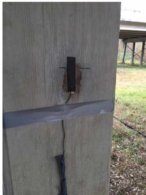
Figure 5-6 Installed Concrete Surface Gage with Strain Relief
