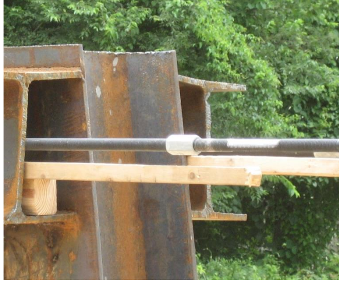
Figure 3-20 Coupled Threaded Rod Sections
