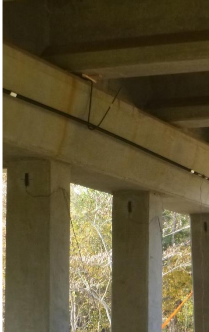
Figure 5-12 Intermediate Bracing for Threaded Rods
