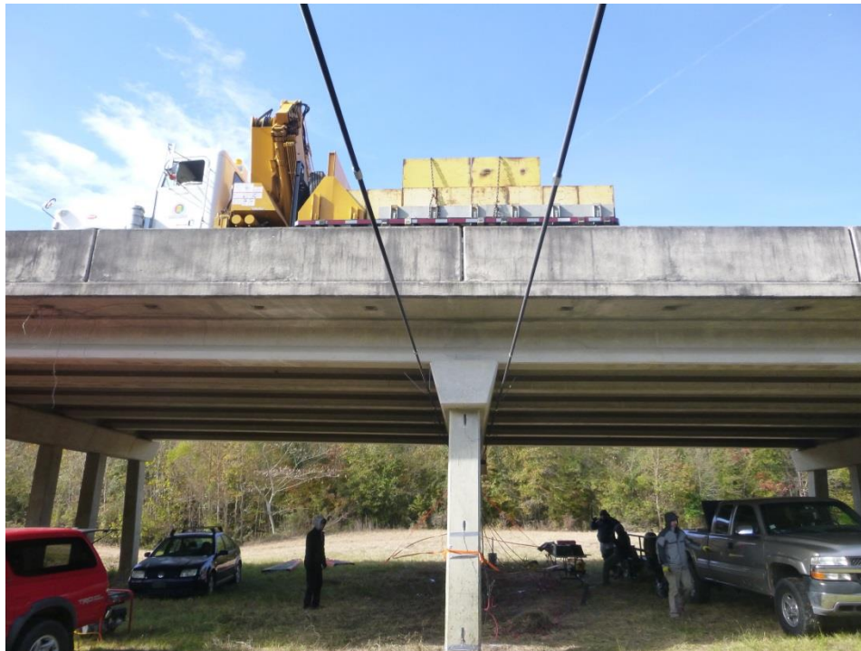
Figure 5-14 Load Truck Positioned Over Test Bent
