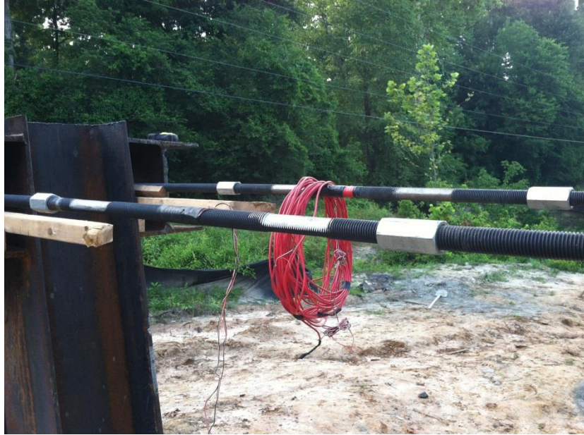
Figure 3-23 Field-Installed Threaded Rods with Instrumentation
