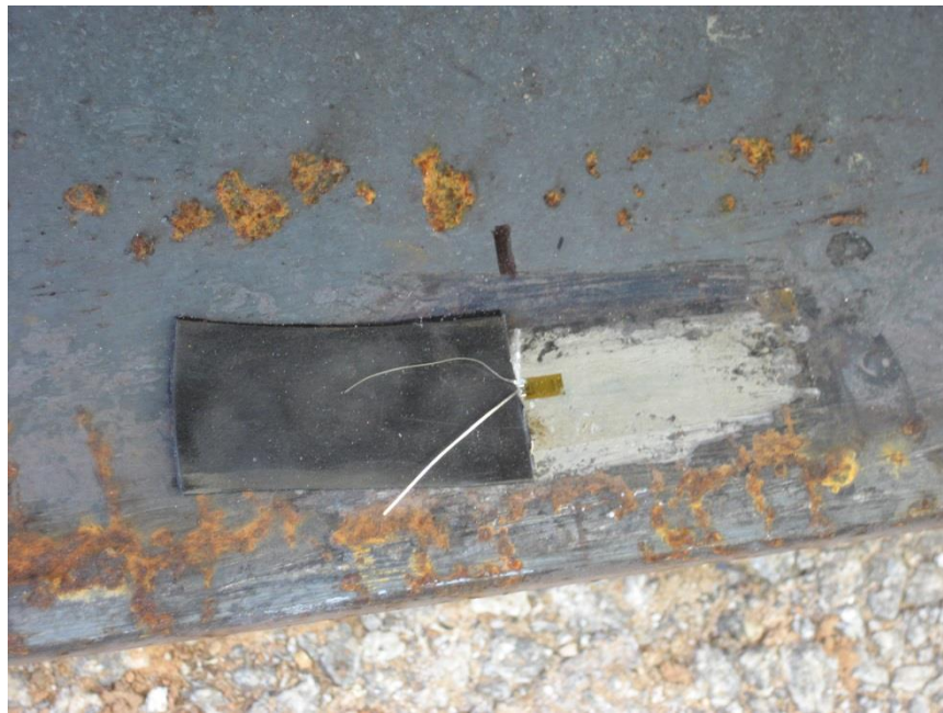
Figure 3-11 Installed Electrical Resistance Gage with Lead Wire Protection
