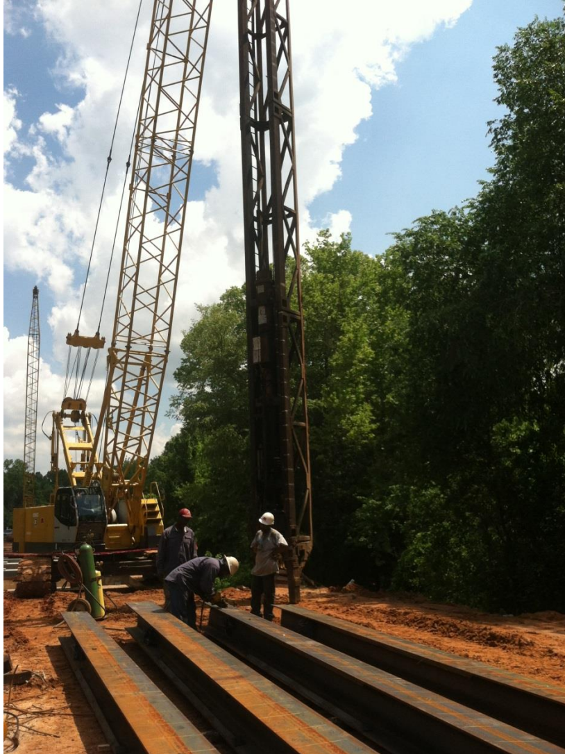
Figure 2-3 Diesel Hammer Rig Used for Driving Piles
