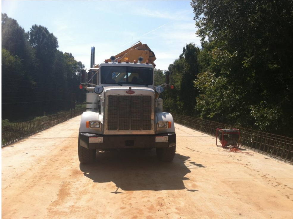
Figure 4-4 ALDOT Load Truck Centered in Roadway
