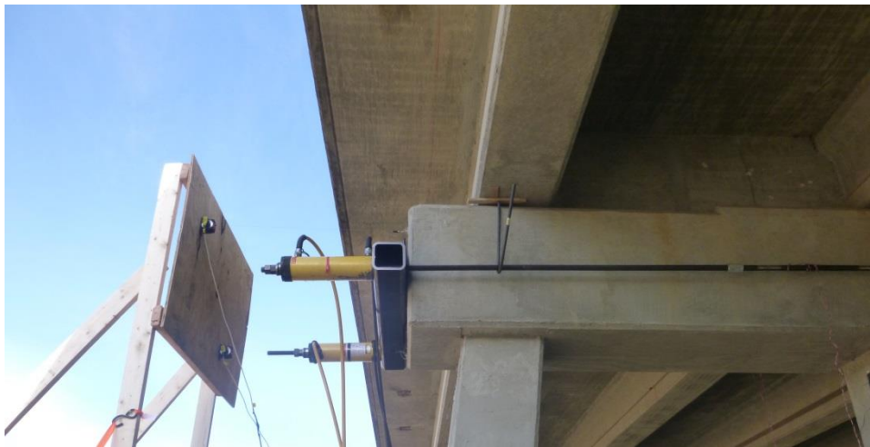
Figure 5-10 Threaded Rods Anchored on Jack End
