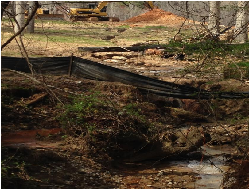
Figure 2.12: Observed silt fence (failed) and straw bale (washed out) that were installed to control sediment and runoff from the construction activities
