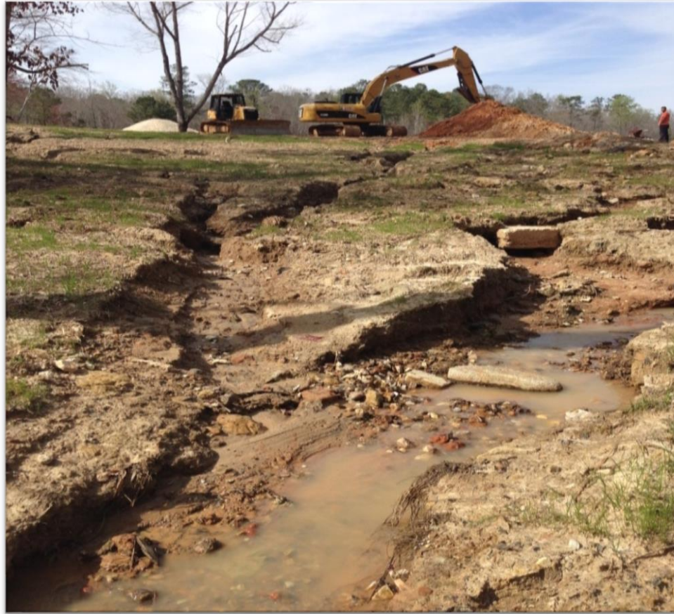
Figure 2.11: Upstream disturbances; deepening the pond with an excavator
