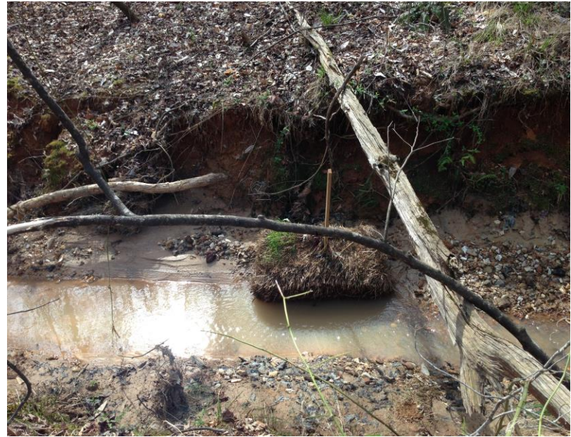
Figure 2.12: Observed silt fence (failed) and straw bale (washed out) that were installed to control sediment and runoff from the construction activities
