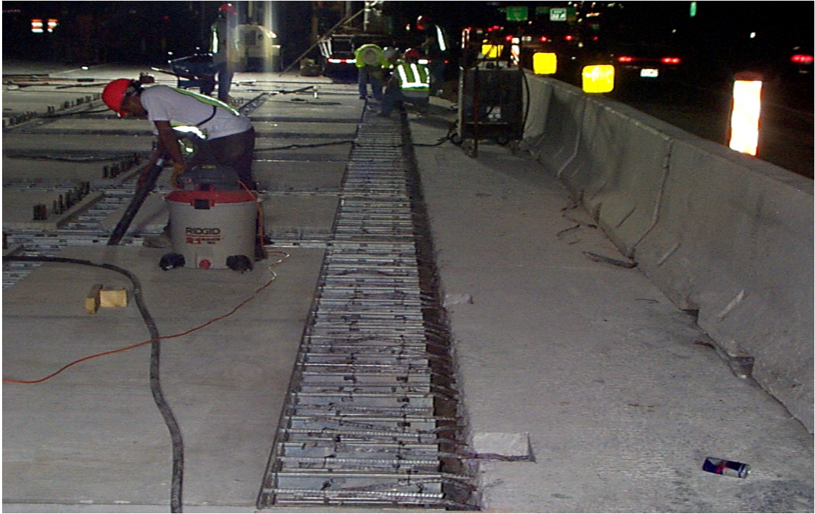
Fig. 6.26 Typical Longitudinal Joint
