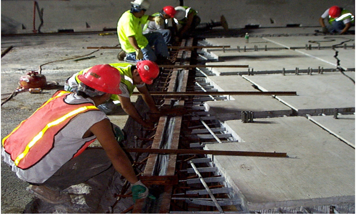
Fig. 6.24 Placement of Endwall Joint
