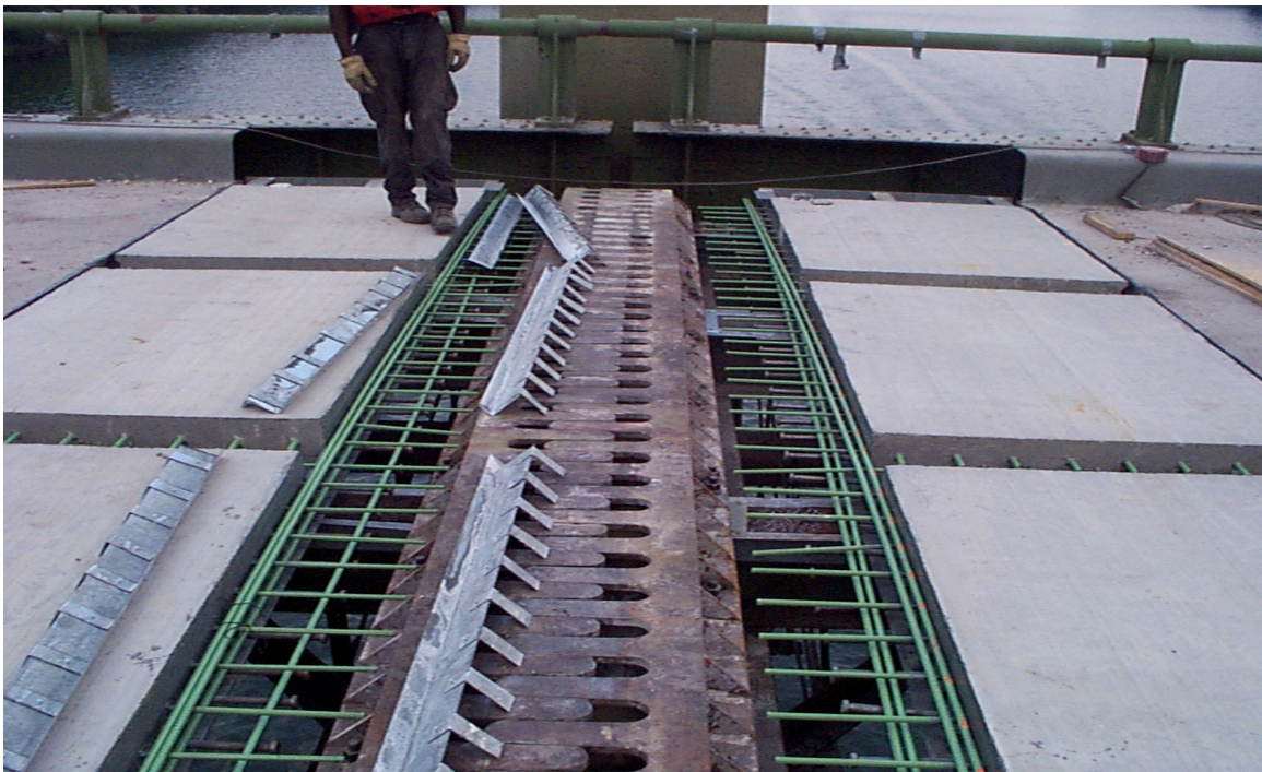
Fig. 3.42 Placement of Exodermic Deck Panels around Finger Joint
