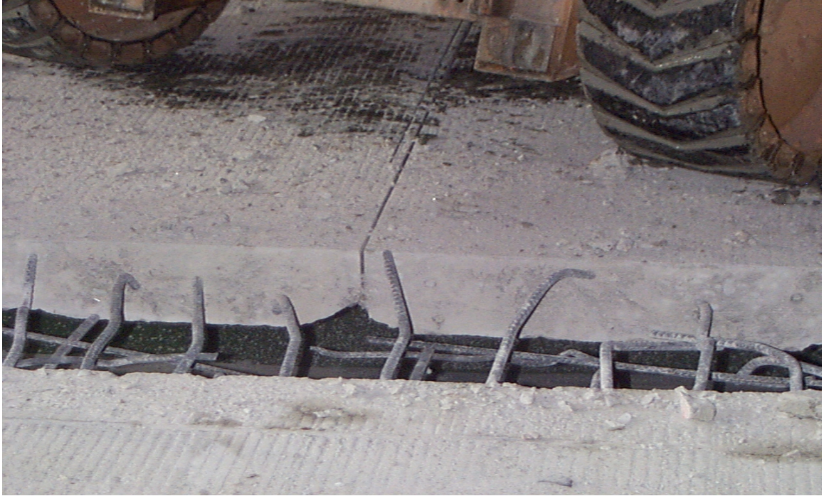
Fig. 5.8 Typical Depth of Transverse Saw Cuts
