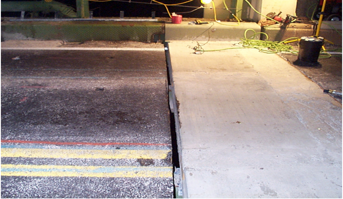
Fig. 3.33 Typical Existing Deck-New Panel Transverse Joint
