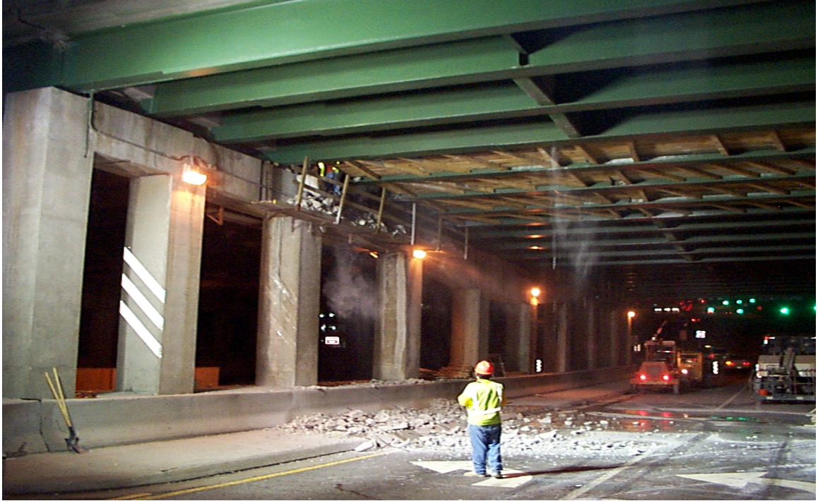
Fig. 5.12 Falling Debris from Edge Beam Removal
