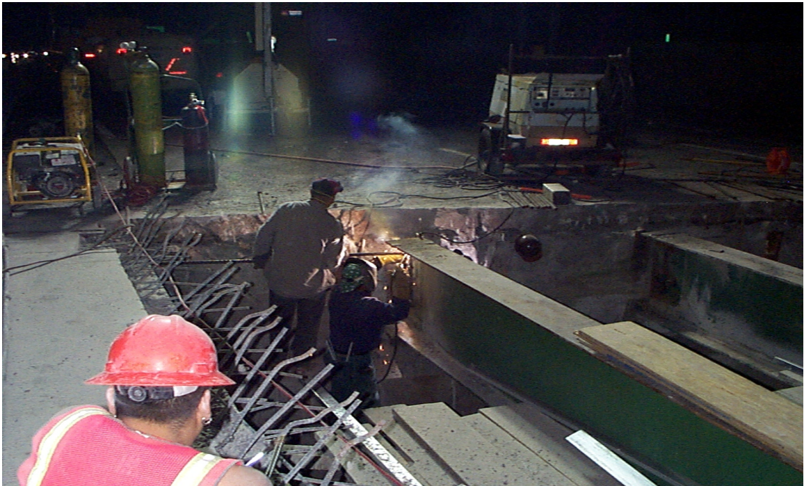
Fig. 6.11 Welding of Threaded Sleeve for Edge Beam Reinforcement
