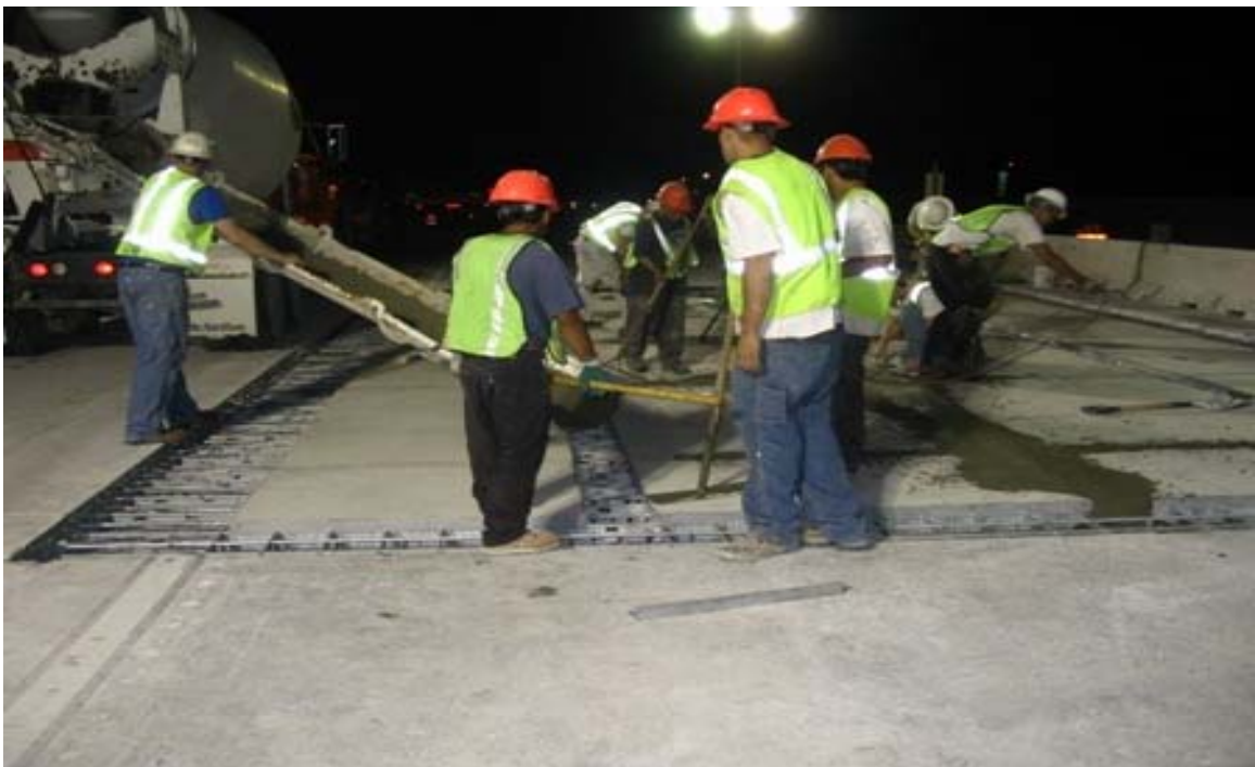
Fig. 5.39 Placement of 24 Hour Accelerated Strength Concrete
