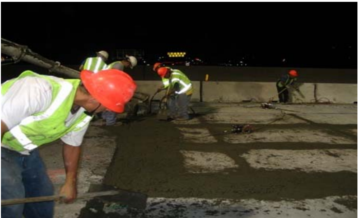
Fig. 5.41 Placement of the Accelerated Concrete
