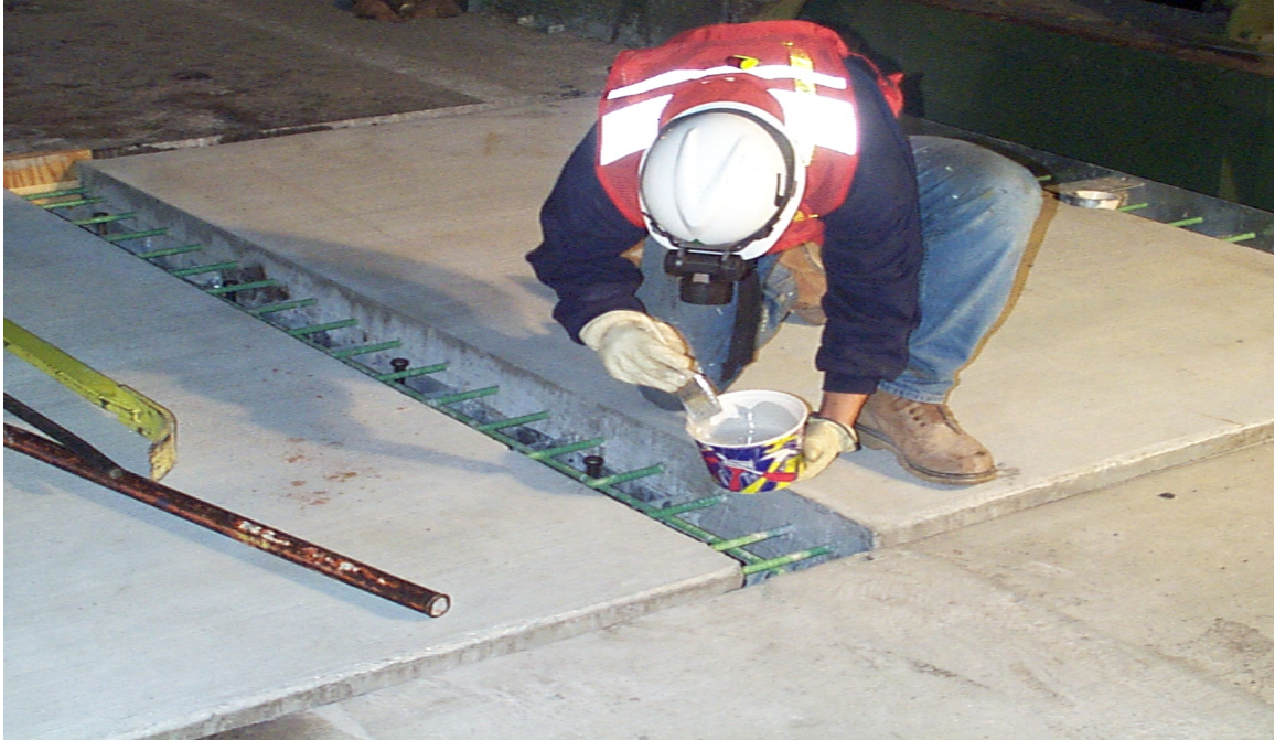
Fig. 3.27 Placing Epoxy on Sides of Closure Pours
