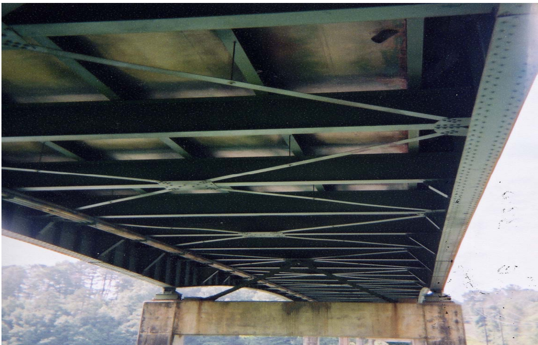
Fig. 2.5 Underneath Shot of Longstreet Bridge (2)
