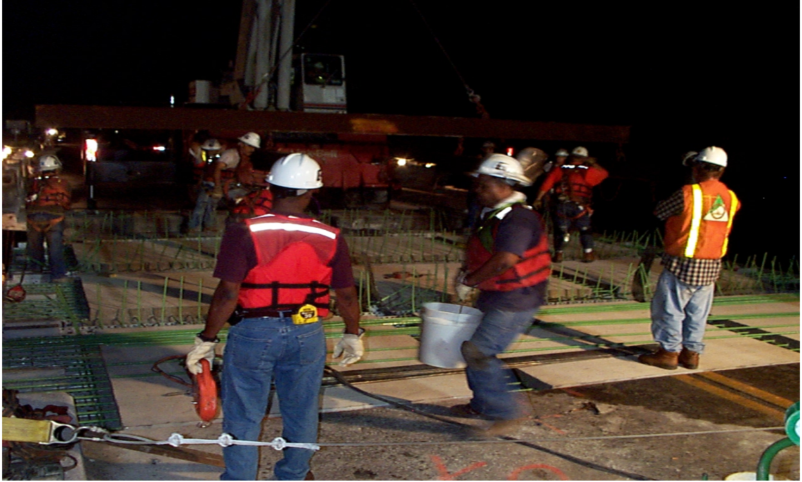
Fig. 4.12 Placement of Third Exodermic Panel
