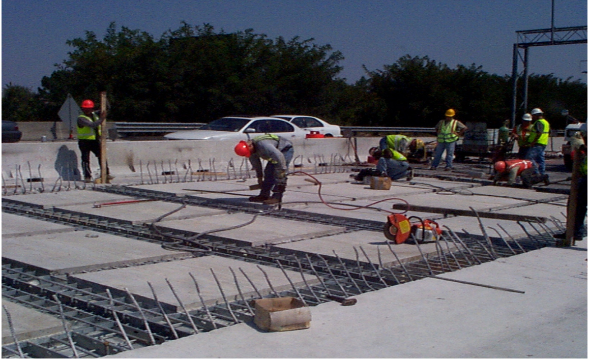
Fig. 6.20 Surface Leveling of Exodermic Panels
