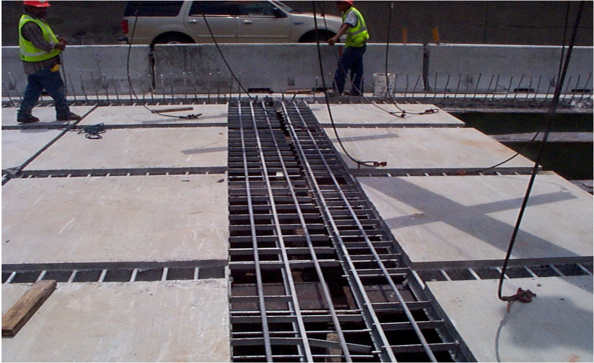
Fig. 5.36 Typical Transverse Joint Over Each Bent
