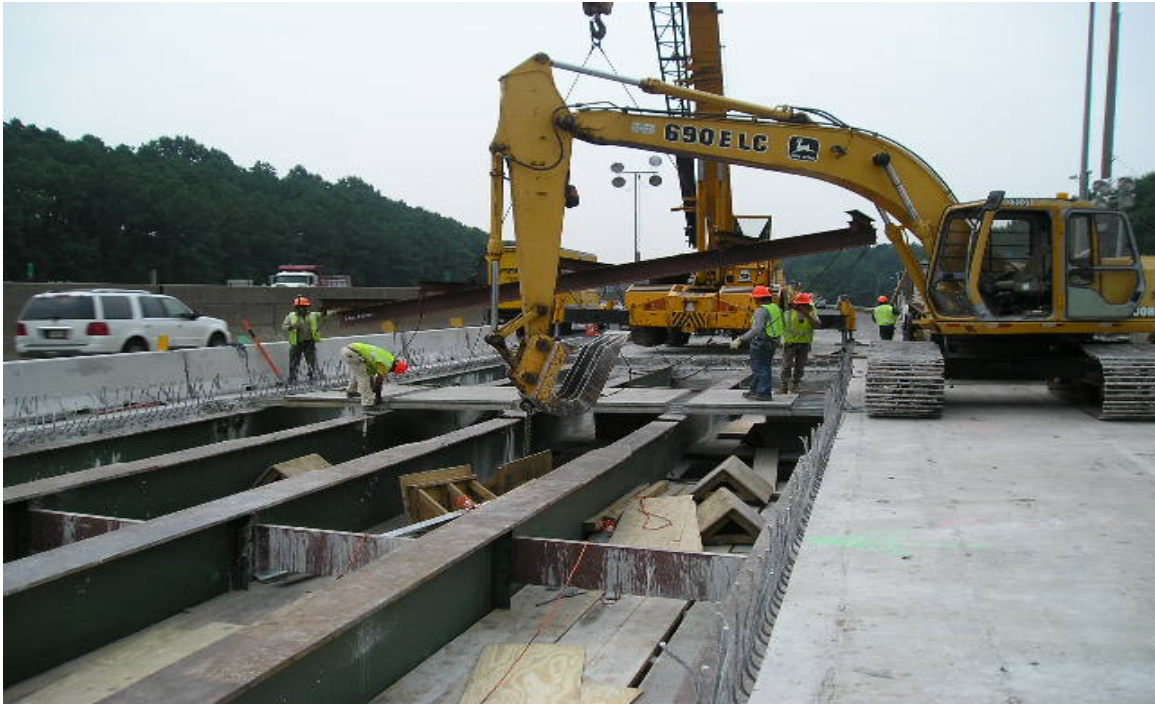
Fig. 5.34 Setting of the Exodermic Panels with Crane and Excavator
