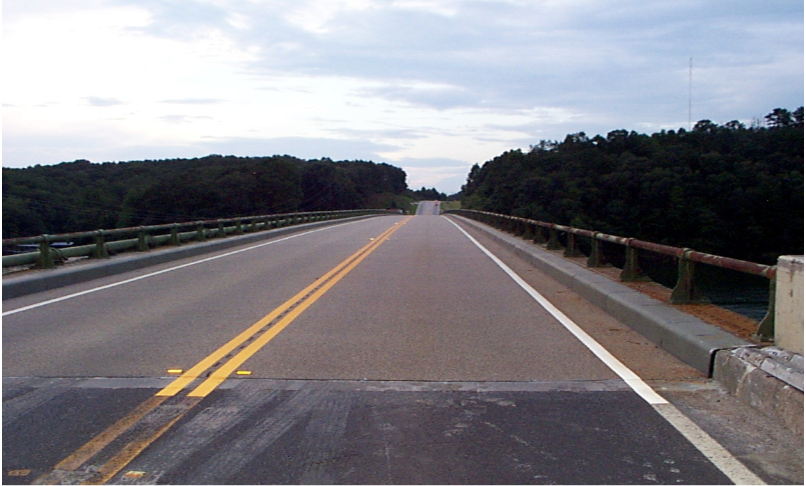
Fig. 3.53 Finished 3/8" Thick Flexogrid Overlay
