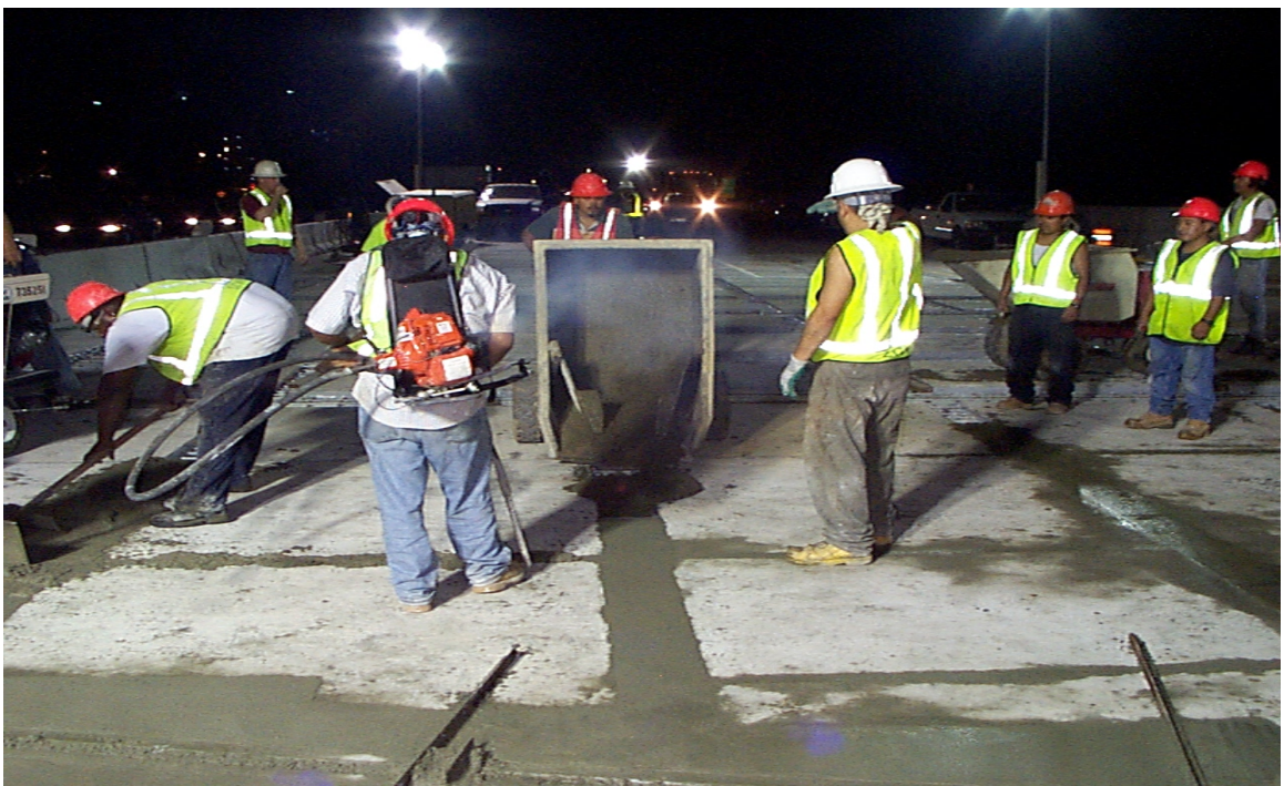
Fig. 6.37 Placement of Accelerated Concrete
