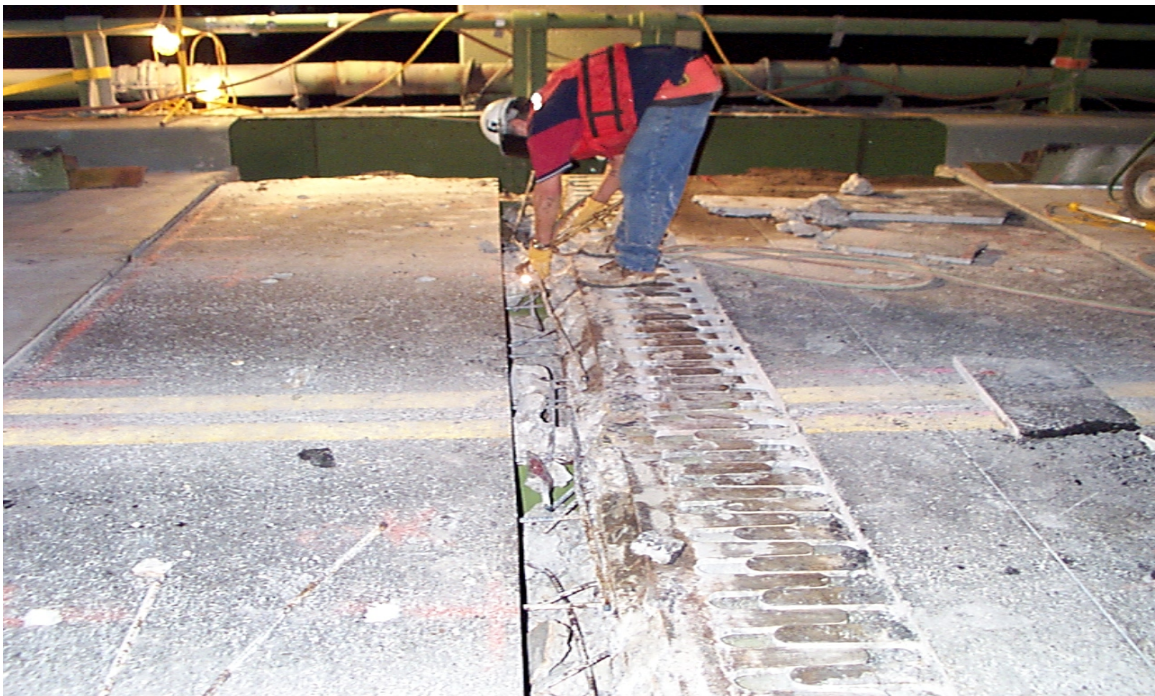
Fig. 3.38 Torch Cutting Reinforcement around Finger Joint
