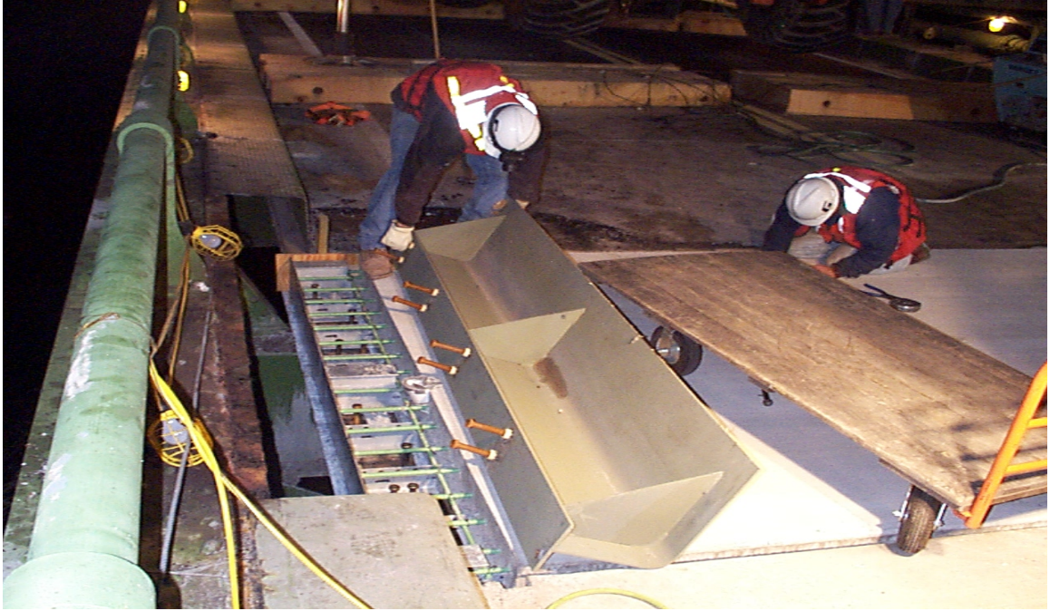
Fig. 3.25 Placing of New Curb Plate
