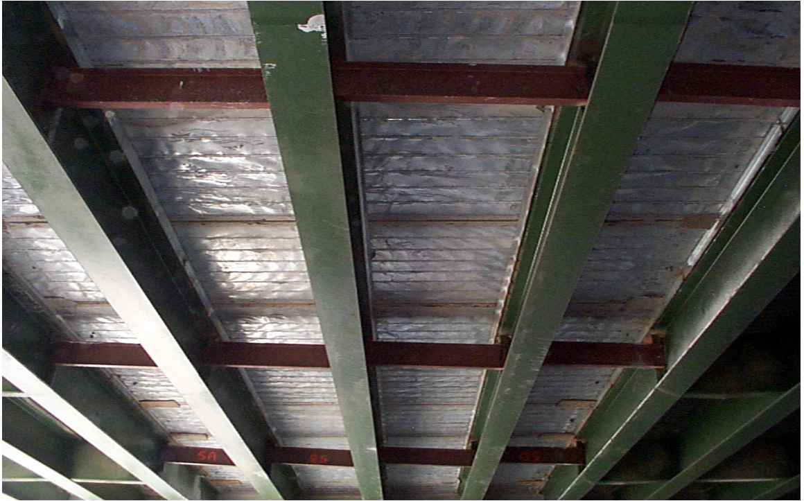
Fig. 5.52 Underneath Shot of Finished Replacement Deck
