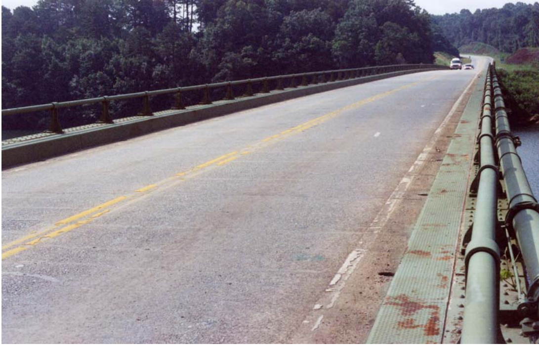
Fig. 2.6 Overview Shot of Longstreet Bridge Deck (2)
