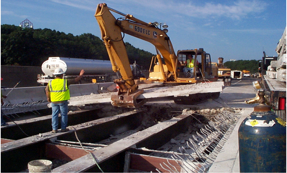
Fig. 5.18 Removal of Last Section of Existing Deck
