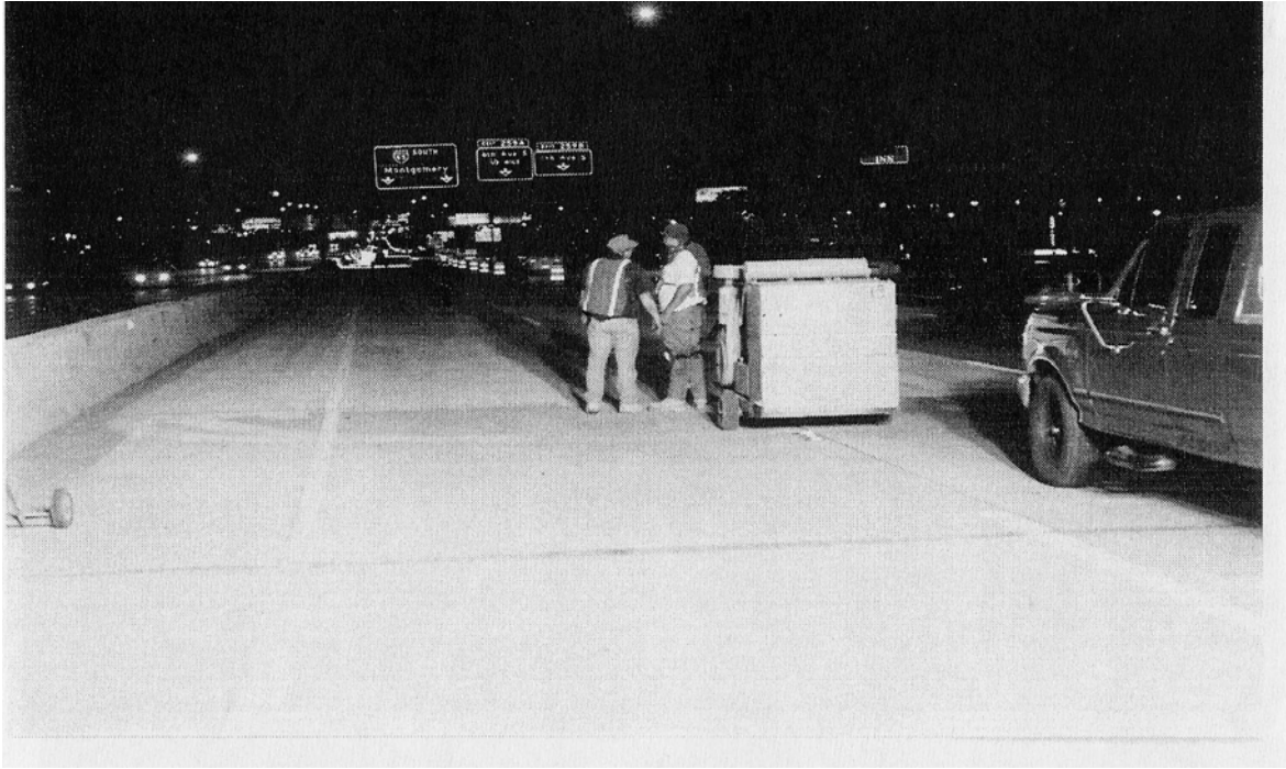
Fig. 2.24 Shot Blast Cleaning of Deck Surface (4)
