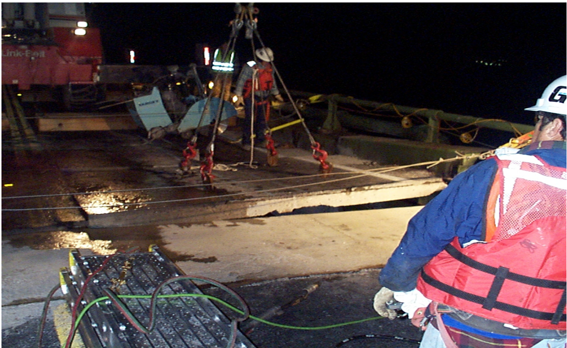
Fig. 3.10 First Section of Existing Deck Being Removed
