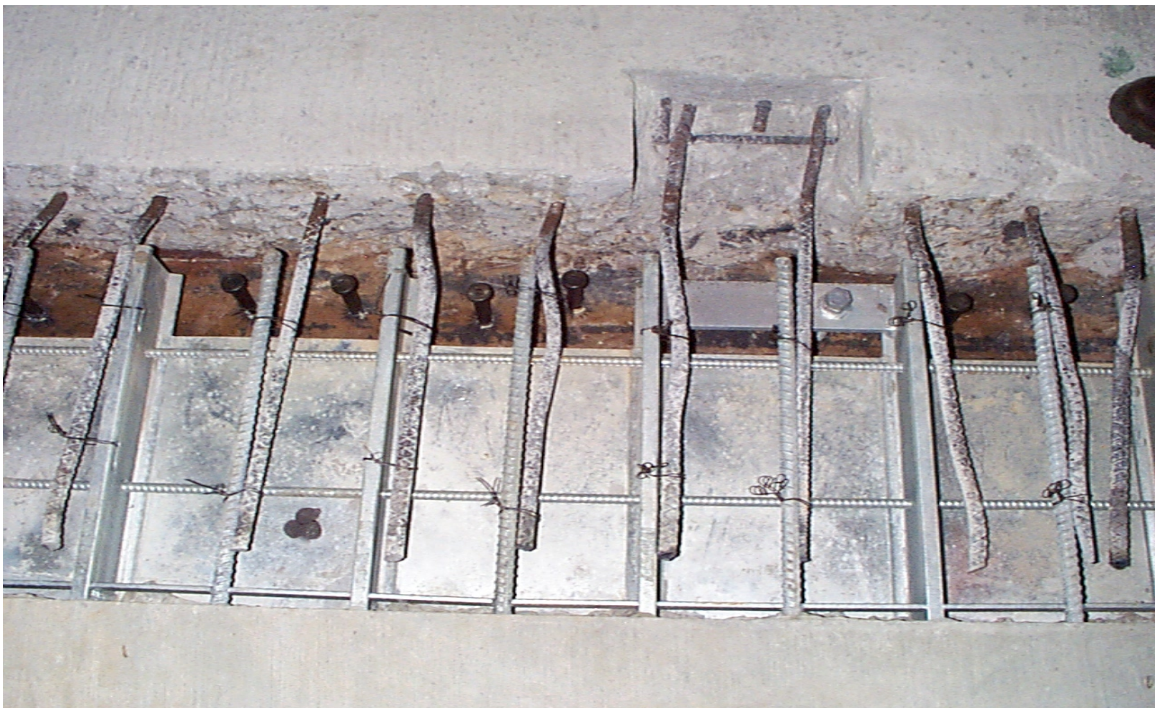
Fig. 6.31 Shear Studs Along Exterior Steel Girders
