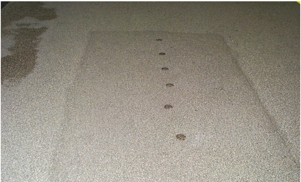
Fig. 3.46 Test Section Used to Perform Overlay Pull-Off Test
