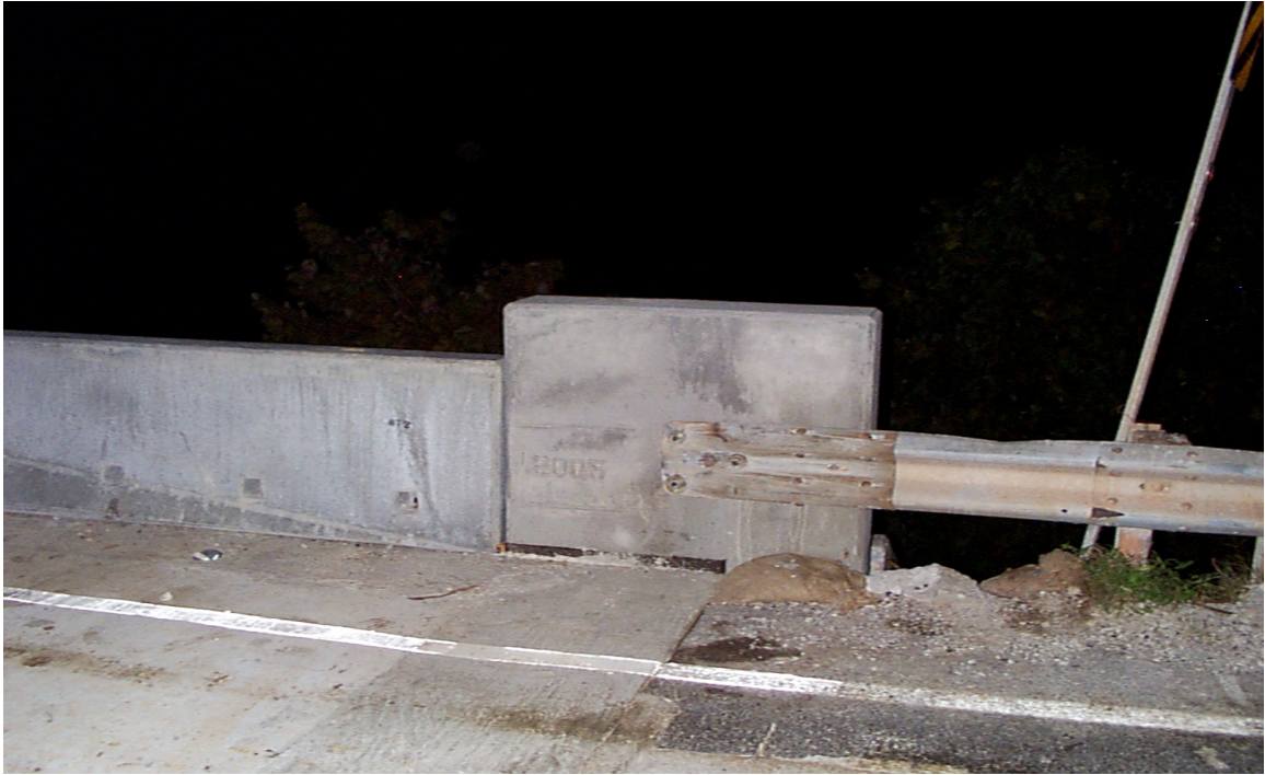
Fig. 4.26 Typical Bridge Endpost – Endpost CIP Before Deck Replacement (see Fig. 4.1)
