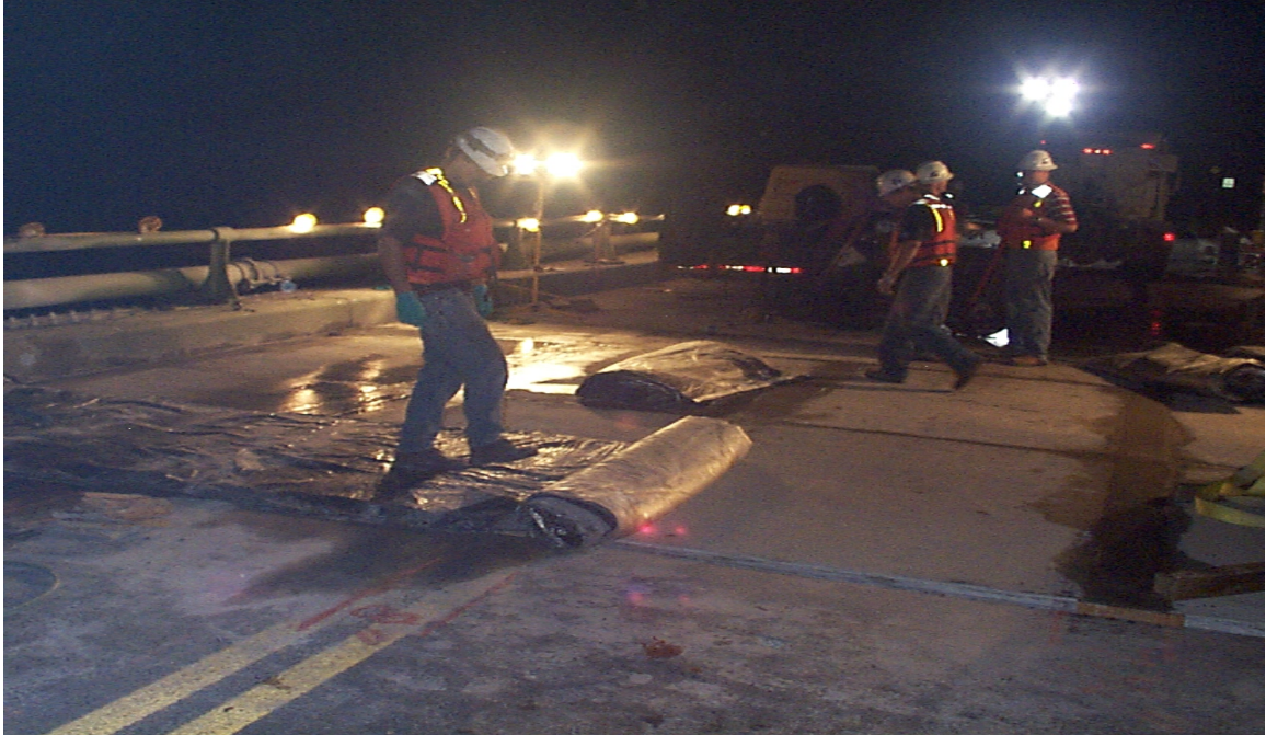
Fig. 3.31 Placement of Curing Blankets over Exodermic Panel Closure Pours
