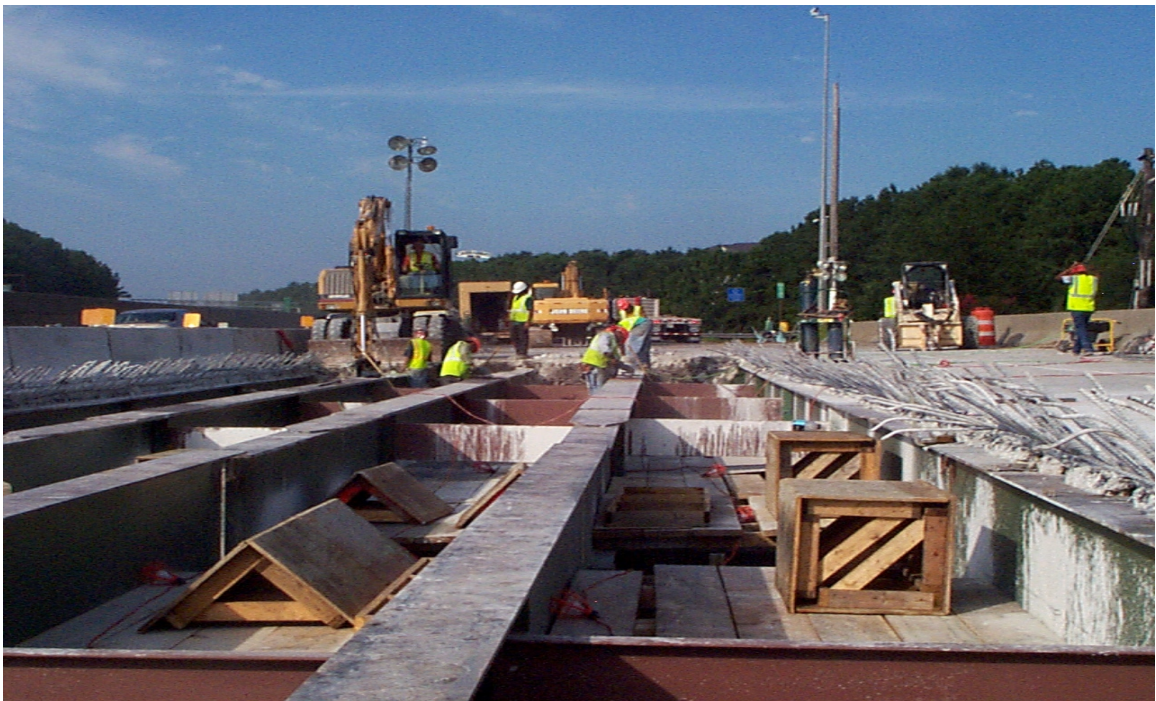
Fig. 5.21 Deck Opening for 17 Panels of Installment
