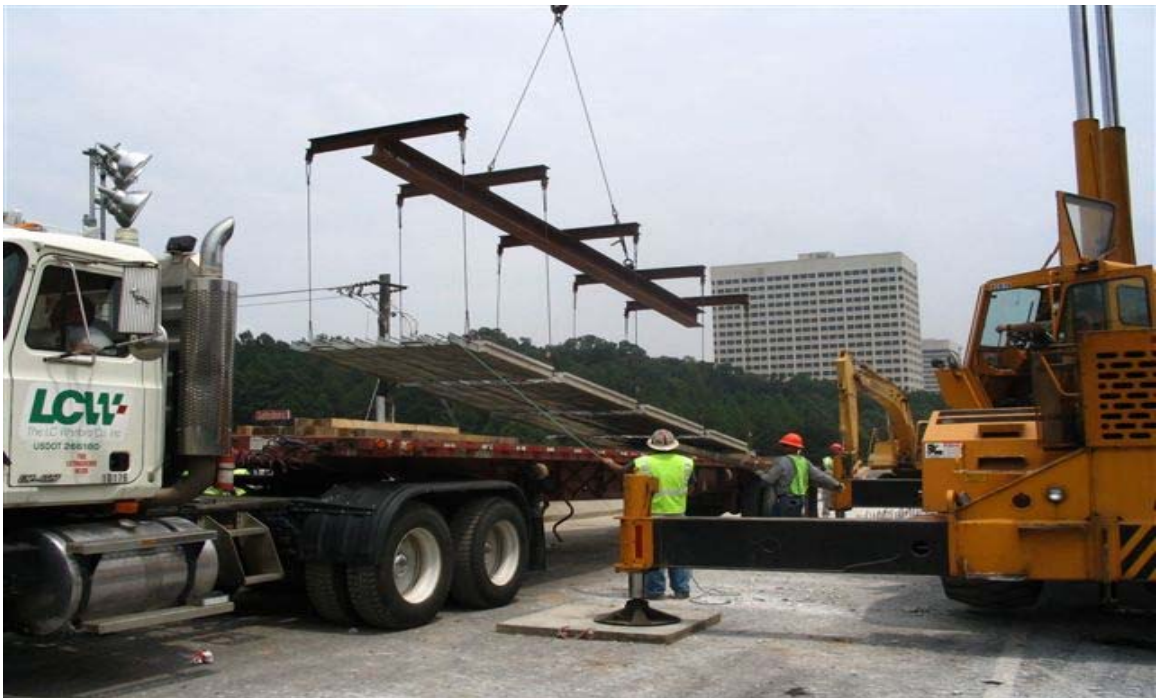
Fig. 5.25 Lift Spreader/Picking Beam Used During Deck Replacement Work
