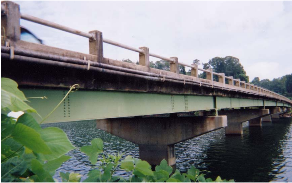
Fig. 2.9 Angled Side Elevation View of Bells Mill Bridge (2)
