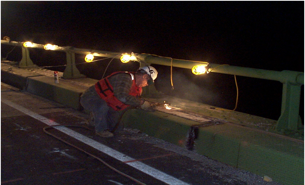
Fig. 3.6 Cutting Curb Plate from Haunch Girder with Cutting Torch
