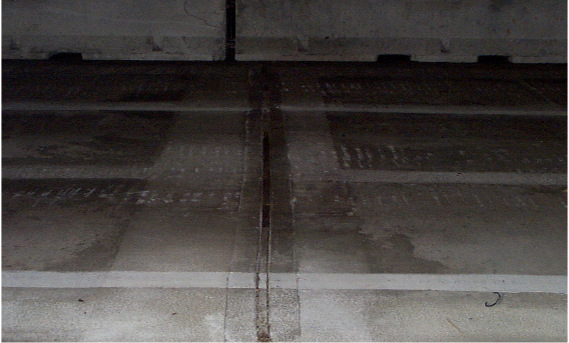
Fig. 5.48 Typical Expansion Joint Located above Each Bent after Deck Replacement
