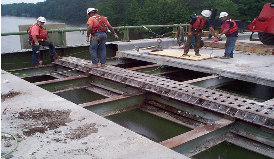
Fig. 3.41 Existing Deck Removed and Setting of Newly Shimmed Finger Joint
