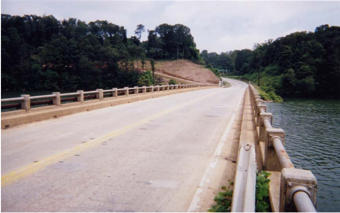
Fig. 2.11 Overview View of Bells Mill Bridge Deck (2)
