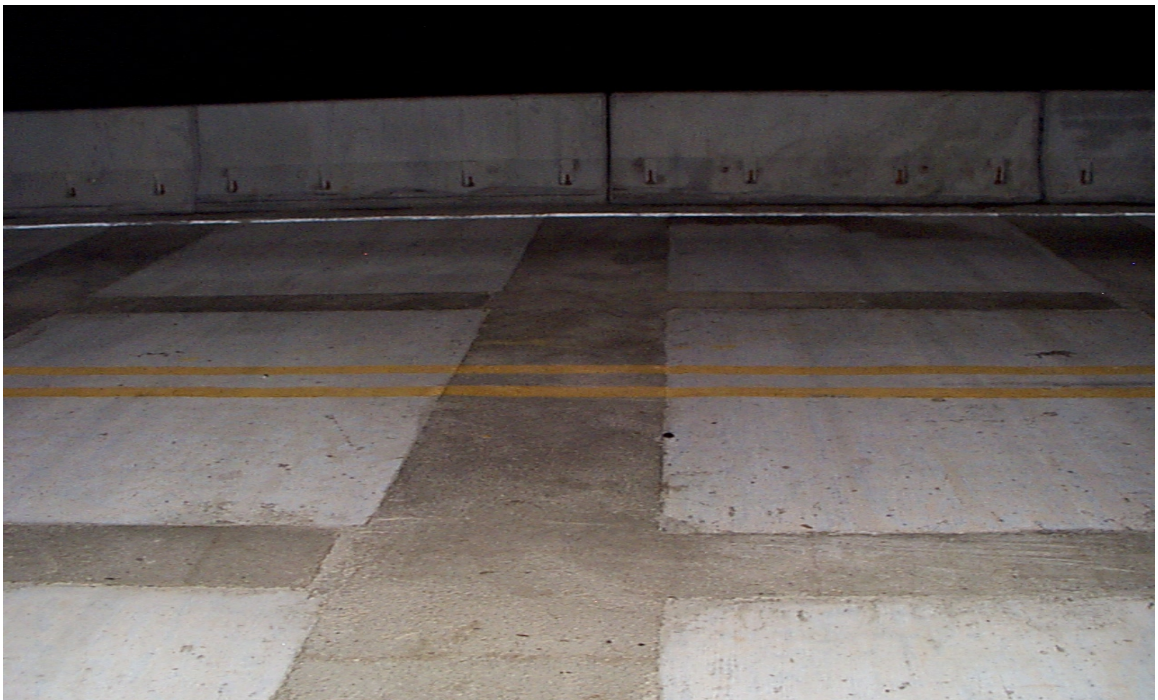
Fig. 4.23 Transverse Joint of Negative Moment Region After Concrete Hardening
