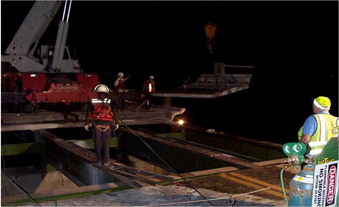
Fig. 4.6 Angled View of the Removal of Existing Deck Slab and Barrier
