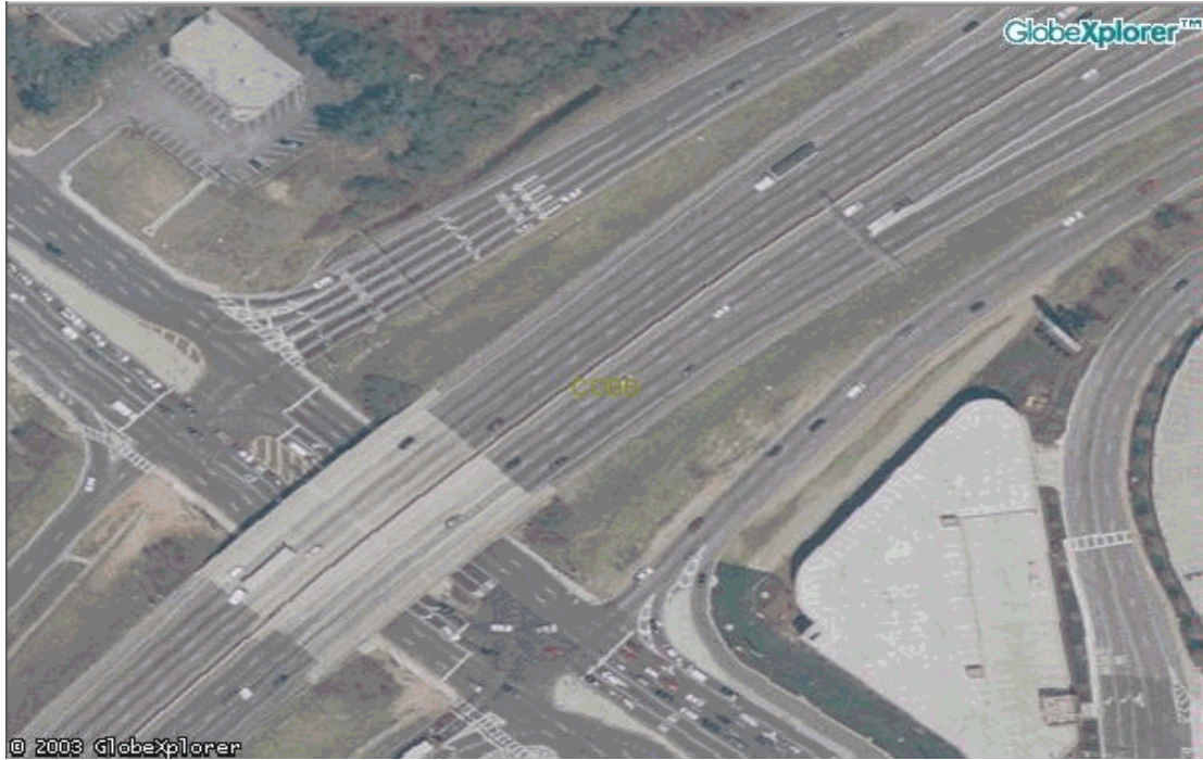
Fig. 2.19 Aerial View of I-285 over U.S. 41 (2)
