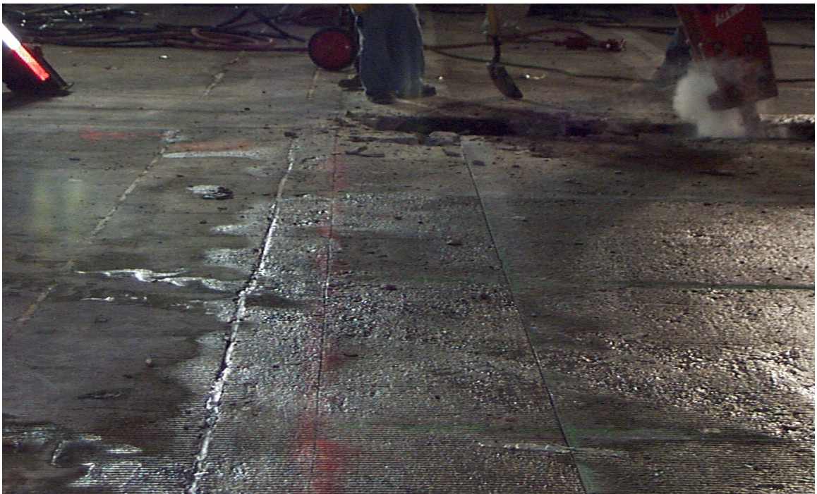
Fig. 5.9 Typical Longitudinal Saw Cuts
