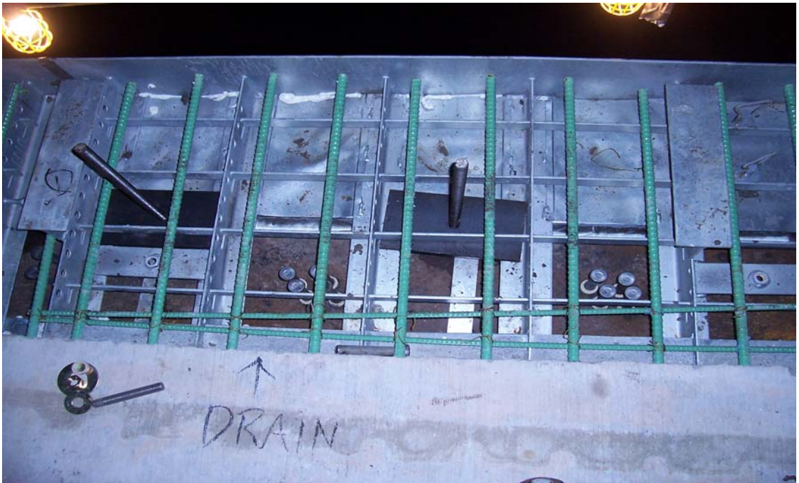
Fig. 4.17 Close-Up of the Barrier Plates and Bolts
