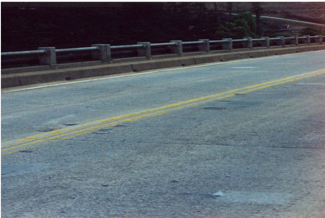
Fig. 2.12 Close-up of Bells Mill Bridge Deck (2)
