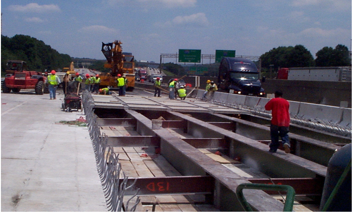
Fig. 5.32 Overview Shot of Precast Exodermic Panels Being Set
