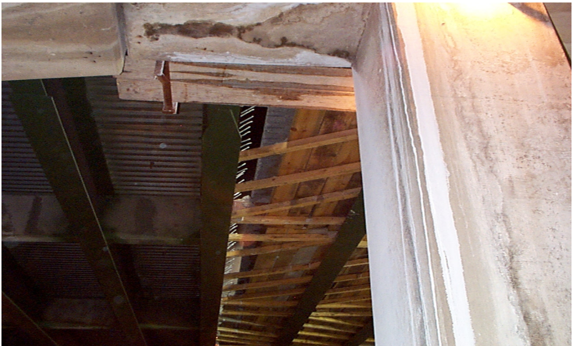
Fig. 5.15 Underneath View of Negative Moment Reinforcing Bars
