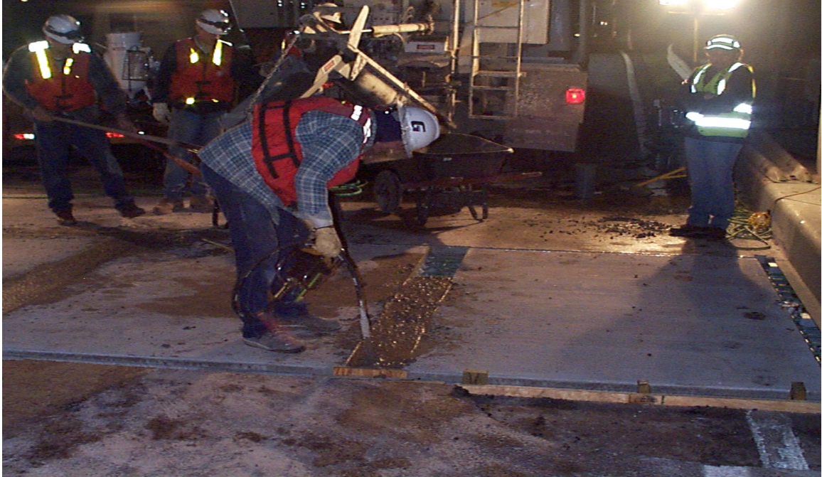
Fig. 3.29 Vibrating of Rapid-Setting Concrete at Stringers
