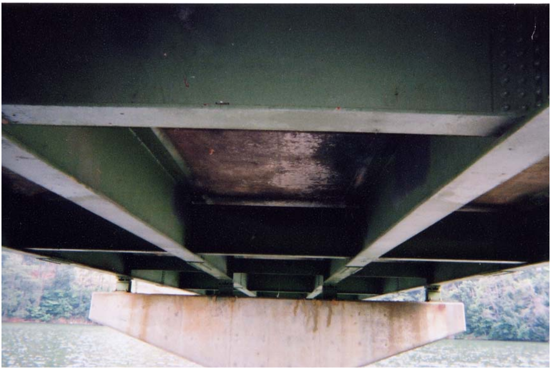
Fig. 2.10 Underneath View of Bells Mill Bridge (2)
