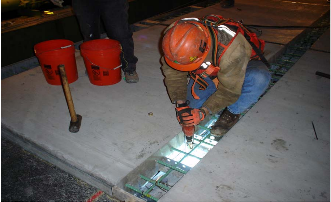
Fig. 4.18 Placing Shear Studs with Shear Gun
