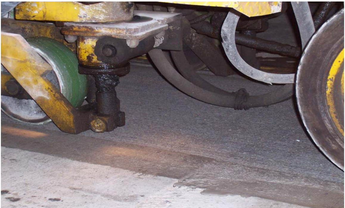
Fig. 3.44 Close-Up of Ground Bridge Deck Surface
