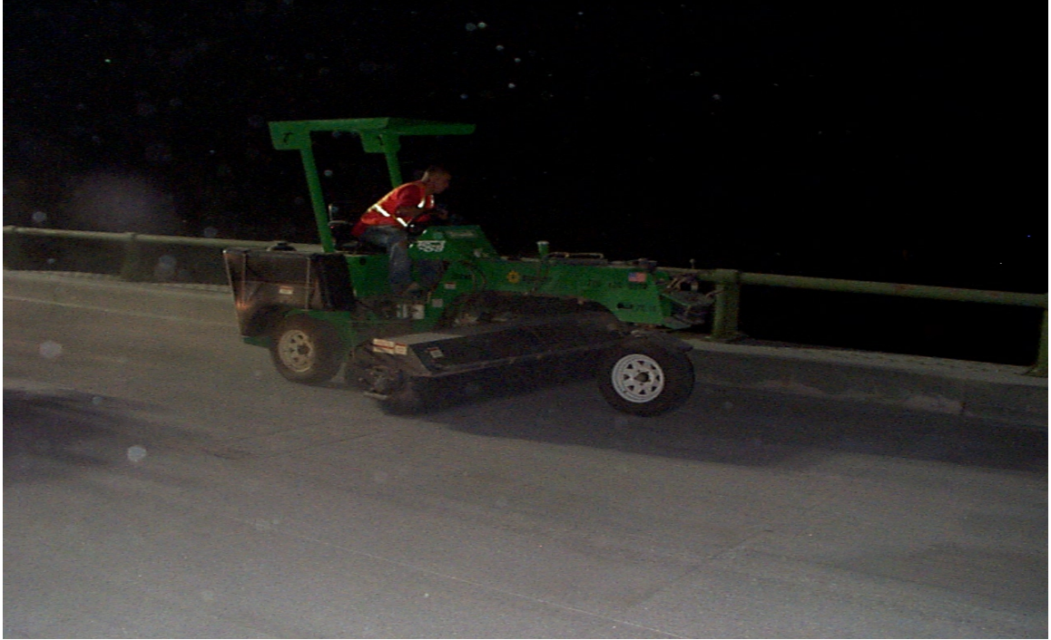
Fig. 3.47 Sweeping Deck Surface to Remove Any Loose Debris
