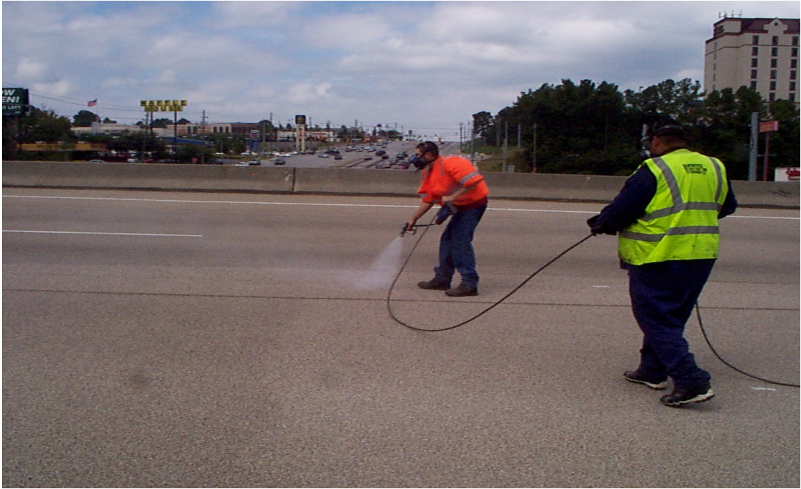
Fig. 5.60 Application of Seal Coat
