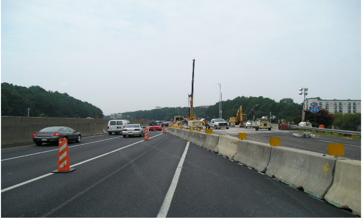
Fig. 5.4 Temporary Concrete Barrier Used During Weekend Closure
