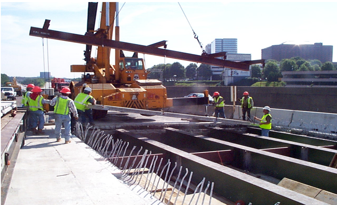
Fig. 5.29 Setting of Precast Exodermic Panel
