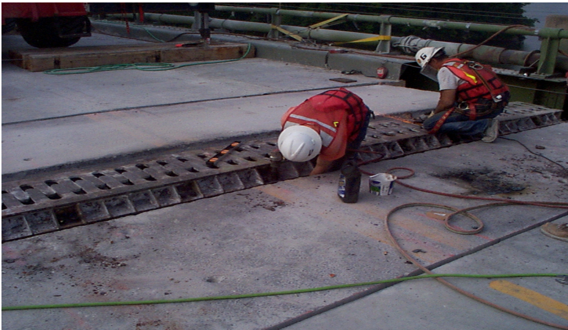
Fig. 3.40 Setting of Finger Joint and Bolt Installation
