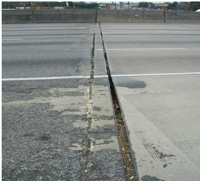
Fig. 2.17 Typical End Joint (2)
