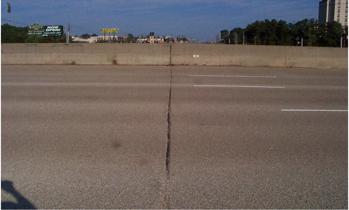
Fig. 5.62 Typical Expansion Joint on Finished Deck Surface
