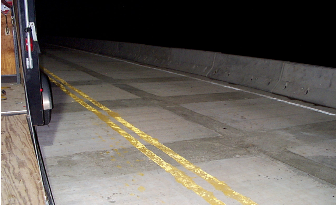
Fig. 4.24 Overview of Negative Moment Region of New Deck
