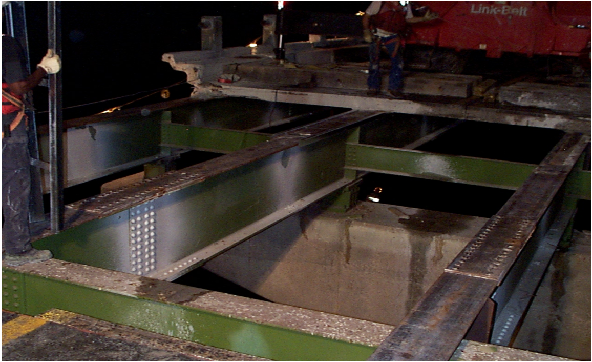
Fig. 4.8 Continuous Steel Girders
