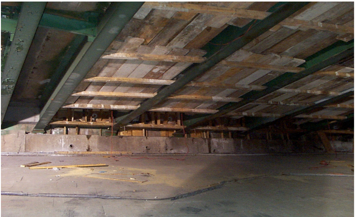
Fig. 6.23 Underneath View of Span-End Edge Beam Formwork
