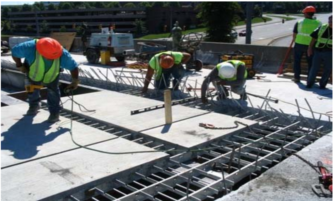
Fig. 5.31 Setting of Second Precast Exodermic Panel
