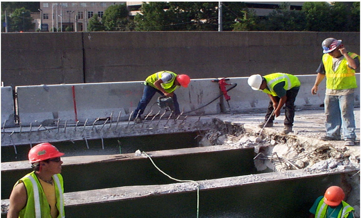
Fig. 5.23 Close-Up of Edge Beam Work
