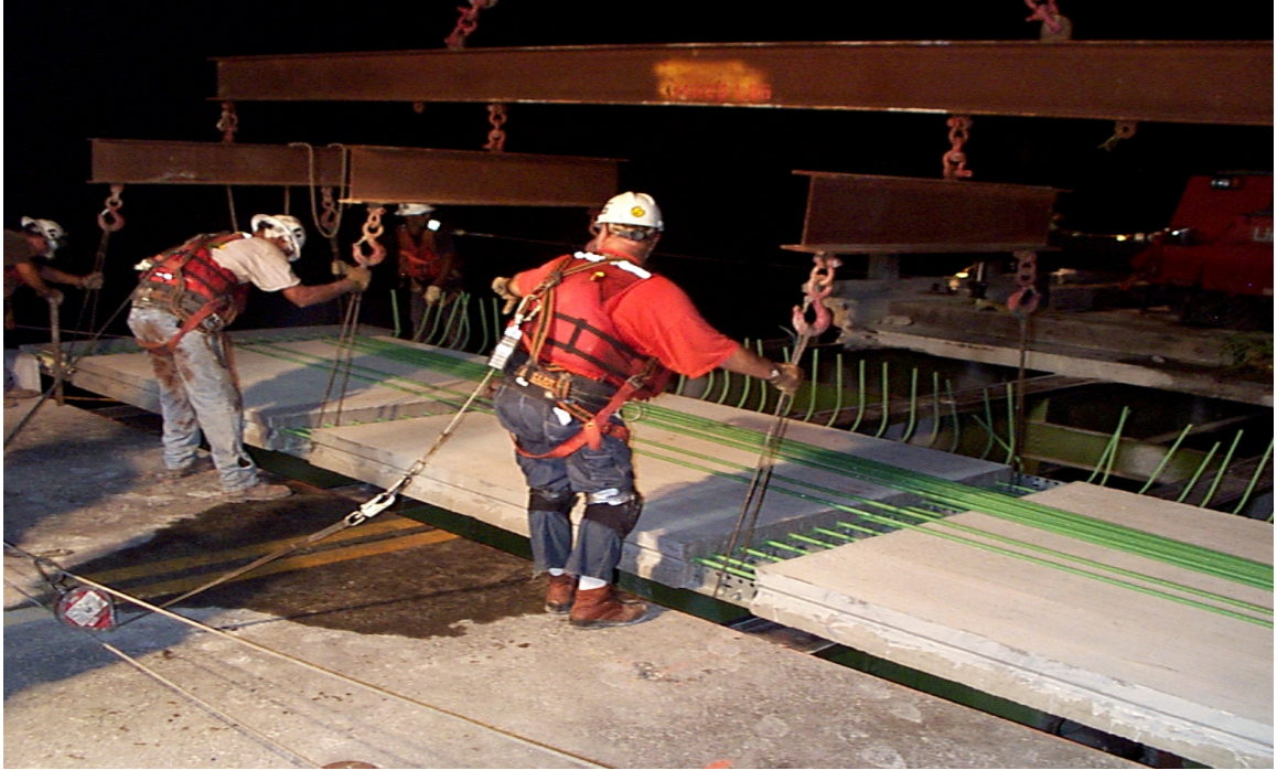
Fig. 4.10 Placement of First Exodermic Panel
