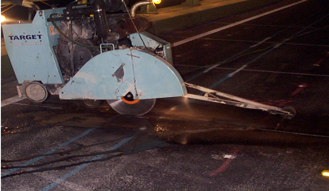
Fig. 3.3 Transverse Saw Cutting for Deck Removal
