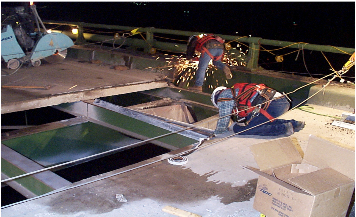
Fig. 3.18 Setting of Sheet Metal Haunch Forms
