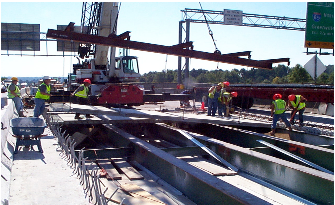
Fig. 6.15 Setting of Second Precast Exodermic Panel
