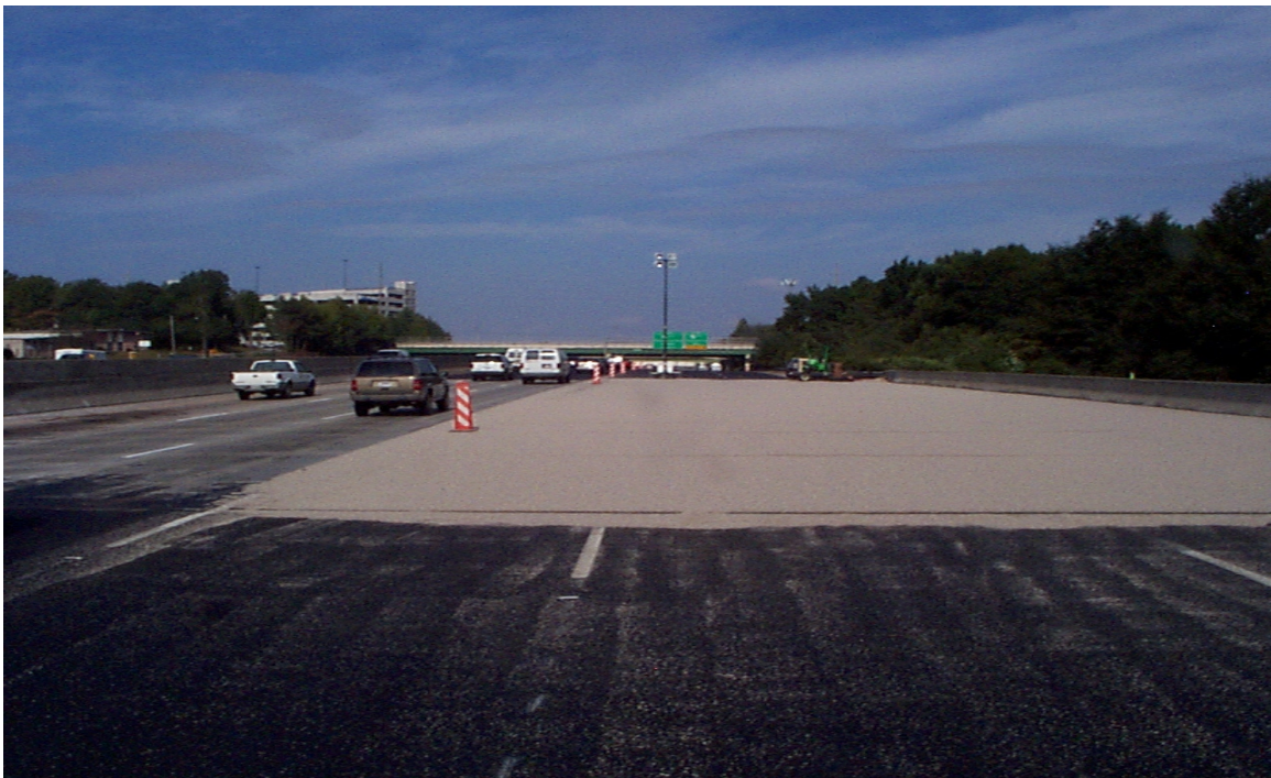
Fig. 6.43 Finished \frac{3}{8} " Thick Flexogrid Overlay on Approximately Half of I-285 Bridges over Buford Highway
