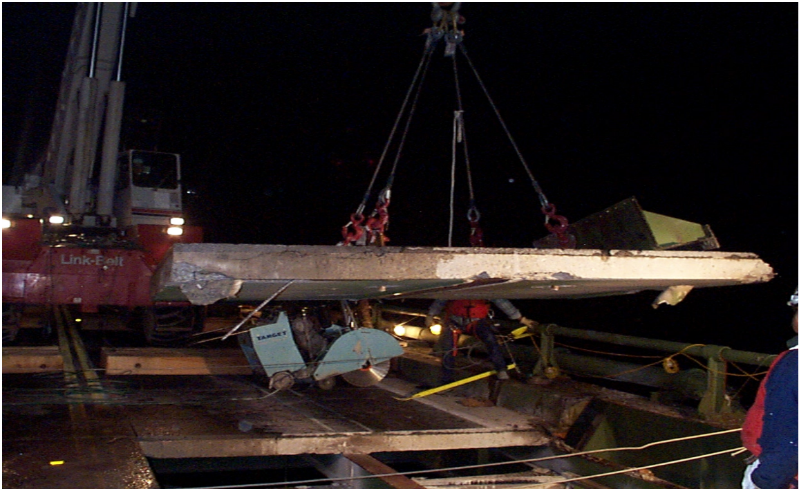
Fig 3.12 First Section of Existing Deck Removed
