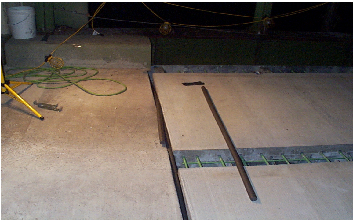
Fig. 3.22 Foam Backer Rods Placed Below Concrete Shear Keys
