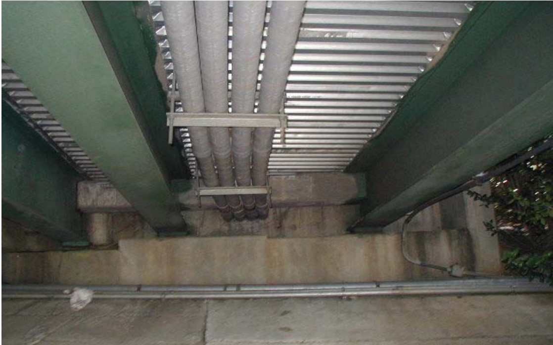
Fig. 2.16 Underside View of Widened Section of Bridge (2)
