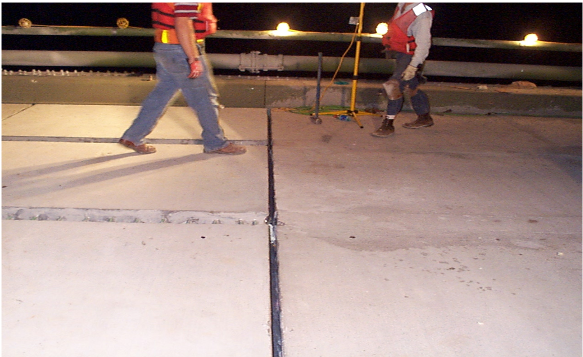
Fig. 3.32 Typical New Panel-New Panel Transverse Joint
