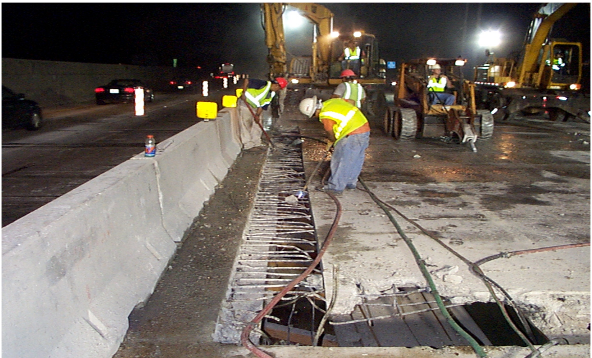
Fig. 5.13 Deck Removal around Existing Negative Moment Reinforcing Bars
