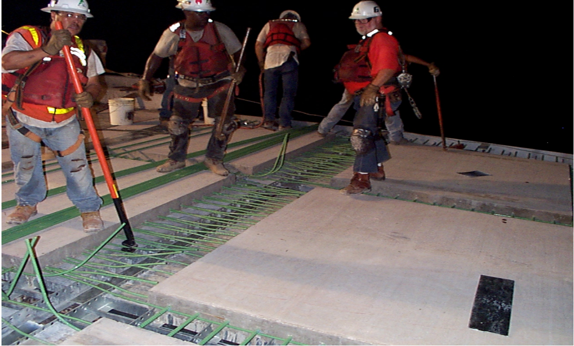
Fig. 4.14 Lapping of the Negative Moment Reinforcing Bars
