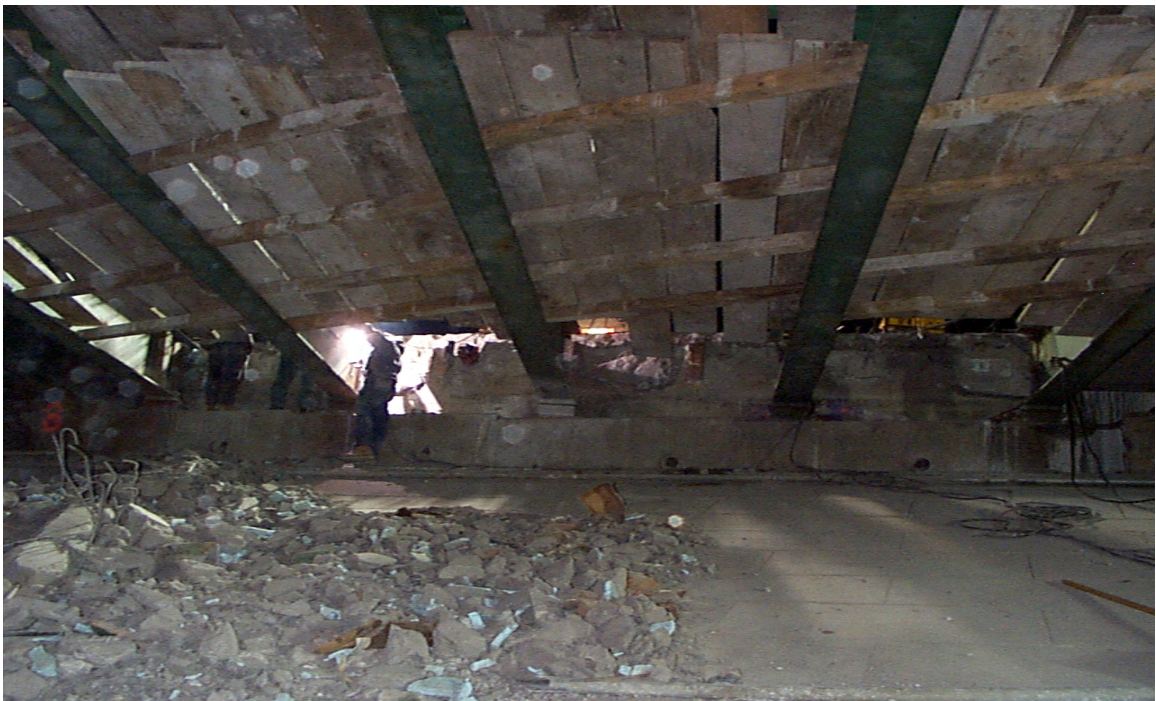
Fig. 6.9 Underneath View of the End-Span Transverse Edge Beam
