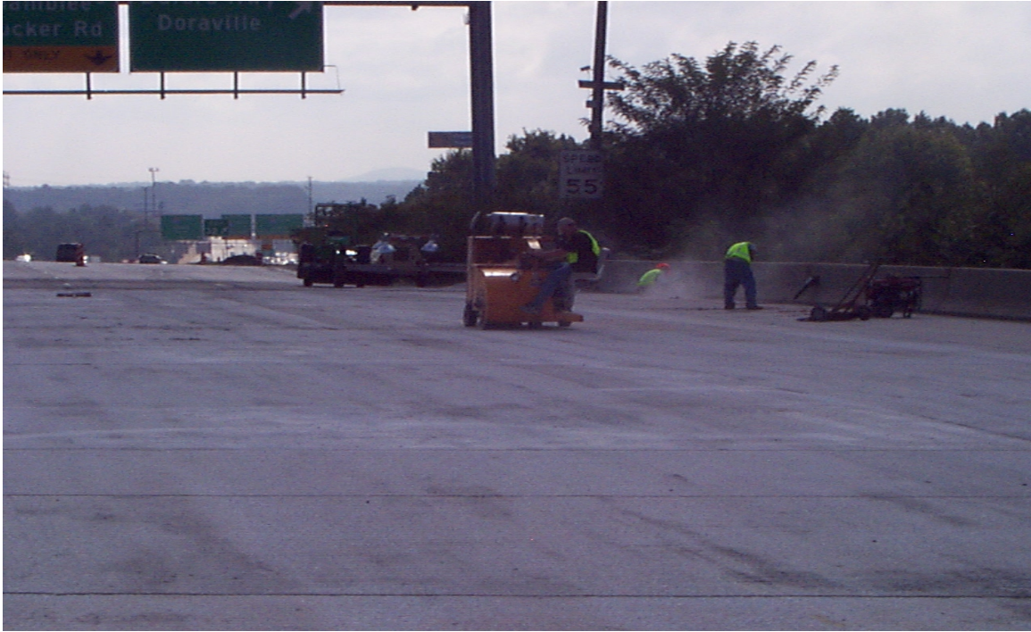
Fig. 5.54 Shot Blast Cleaning of Deck Surface
