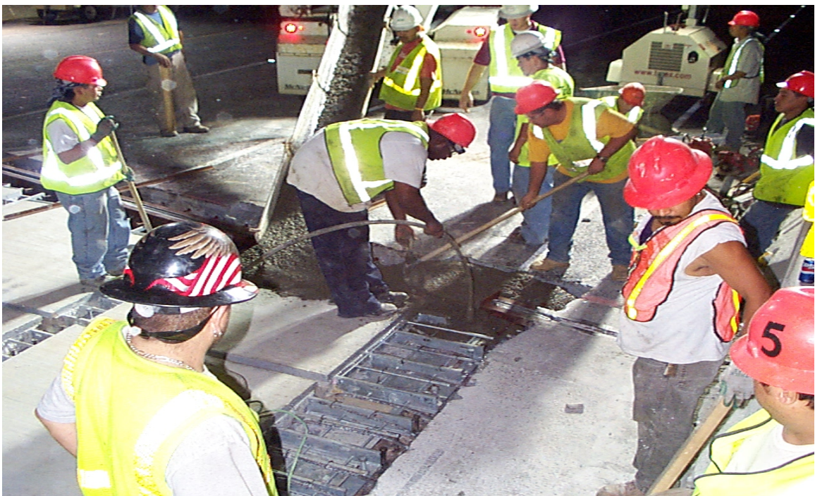
Fig. 6.35 Consolidation of Field Placed Concrete
