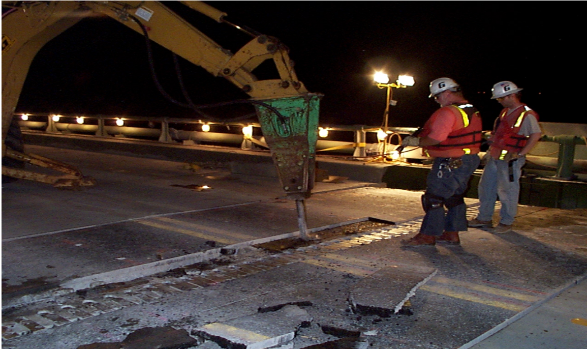
Fig. 3.37 Jack Hammering Existing Deck around Finger Joint
