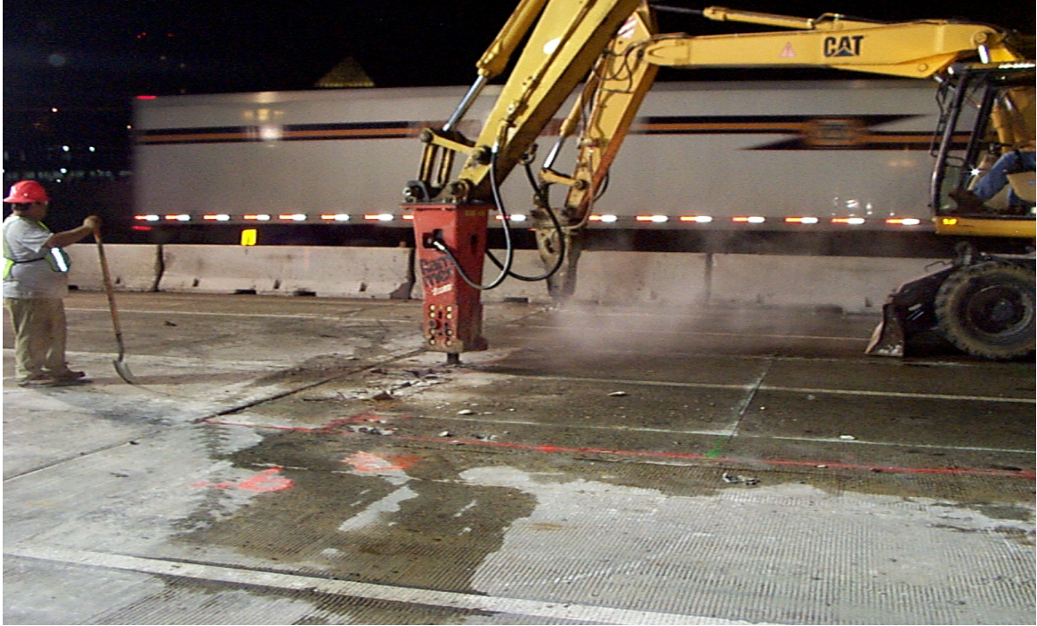
Fig. 5.10 Jack Hammering at Locations Above Edge Beams
