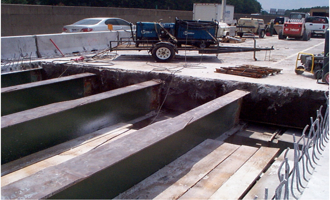
Fig. 5.24 Close-Up of Edge Beam After the Removal of the Existing Concrete
