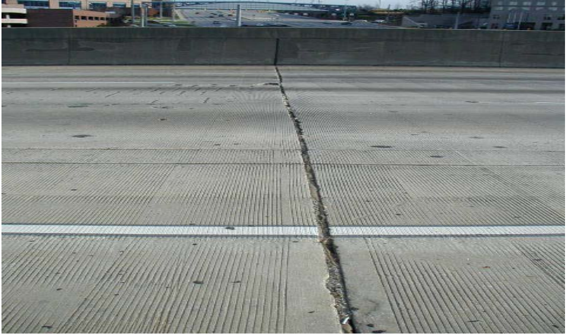
Fig. 2.23 Typical Transverse Joint on Northbound Bridge (2)
