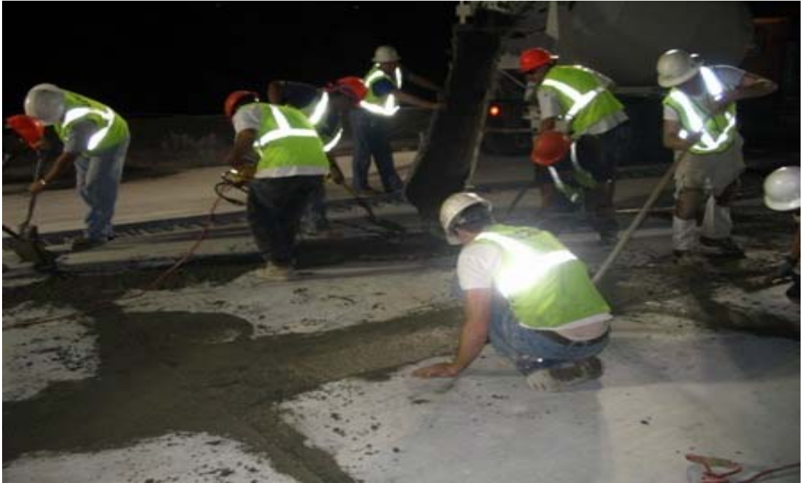
Fig. 5.40 Smoothing and Consolidating of the 24 Hour Accelerated Concrete
