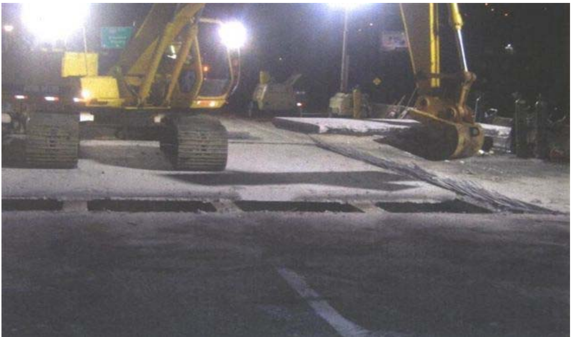
Fig. 5.17 Removal of First Section of Existing Deck
