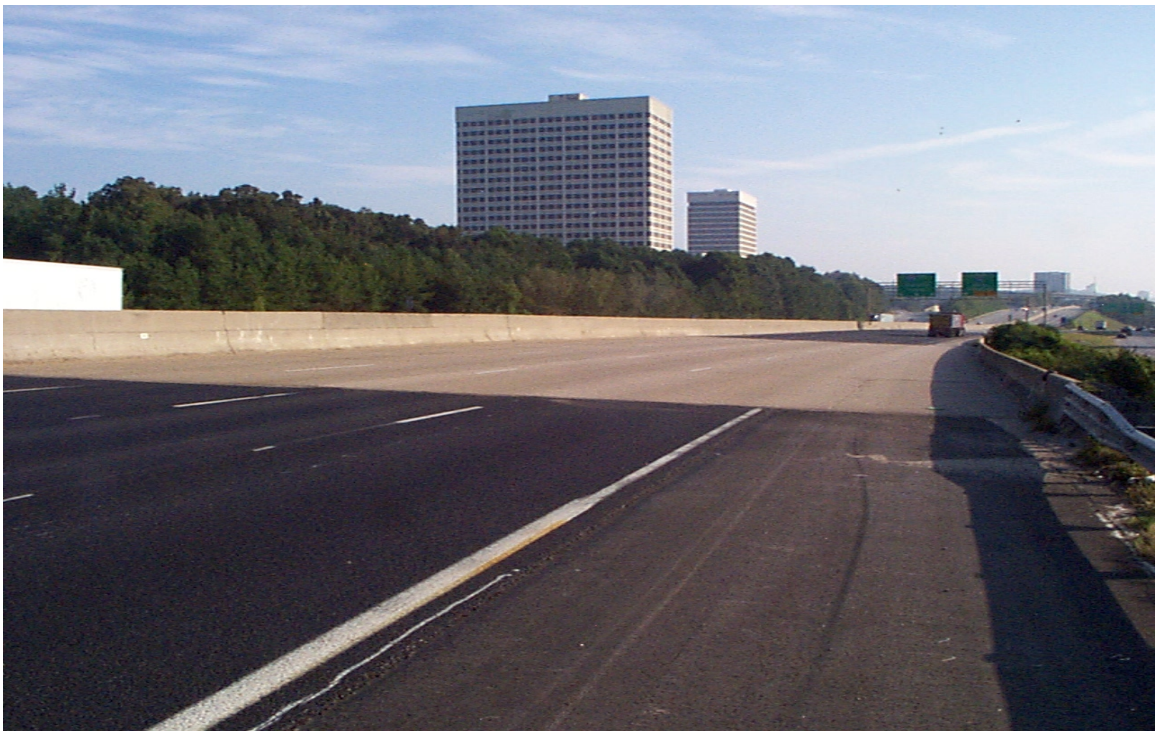
Fig. 5.63 Finished \frac{3}{8} " Thick Flexogrid Overlay on Westbound Bridge
