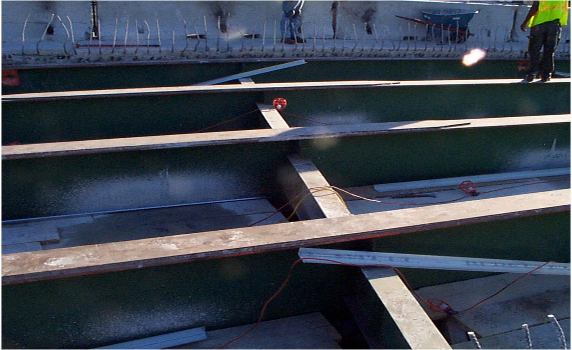
Fig. 6.12 Surface View of Continuous Steel Girders
