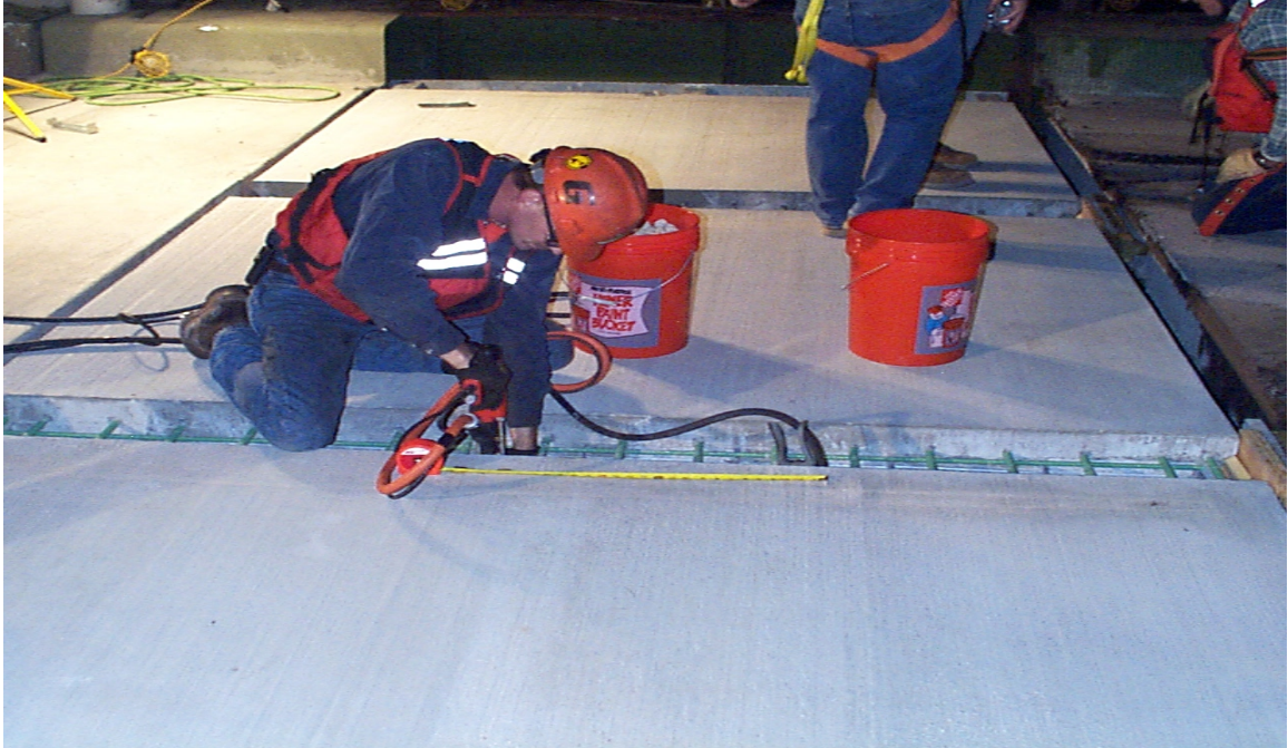
Fig. 3.23 Placing Shear Studs with Stud Gun
