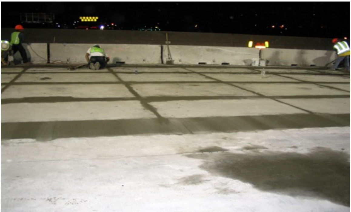
Fig. 5.43 Overview Shot of Longitudinal and Transverse Closure Pours
