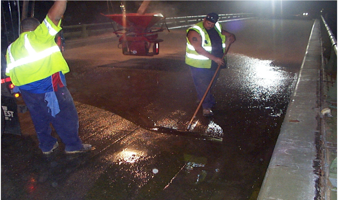
Fig. 3.49 Squeegeeing-on of Epoxy Based Copolymer Binder
