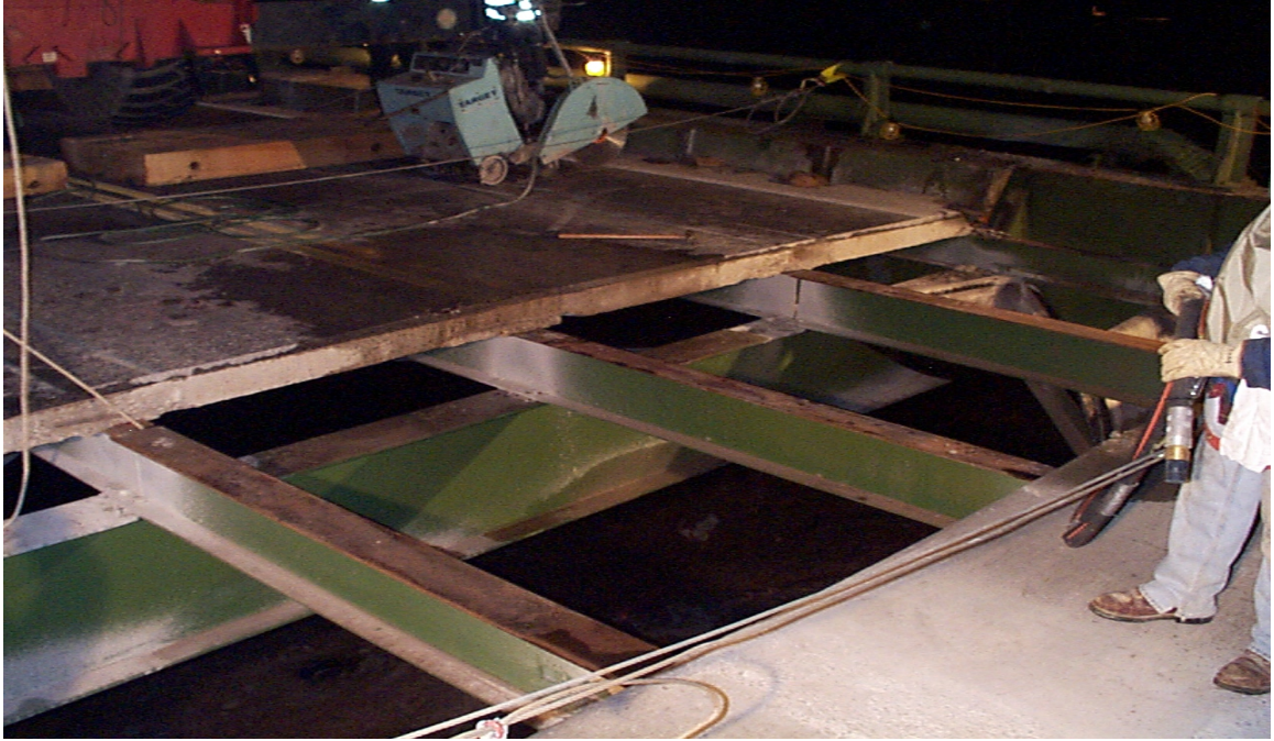
Fig. 3.15 Existing Deck Removed and Preparation for Top Flange Cleaning
