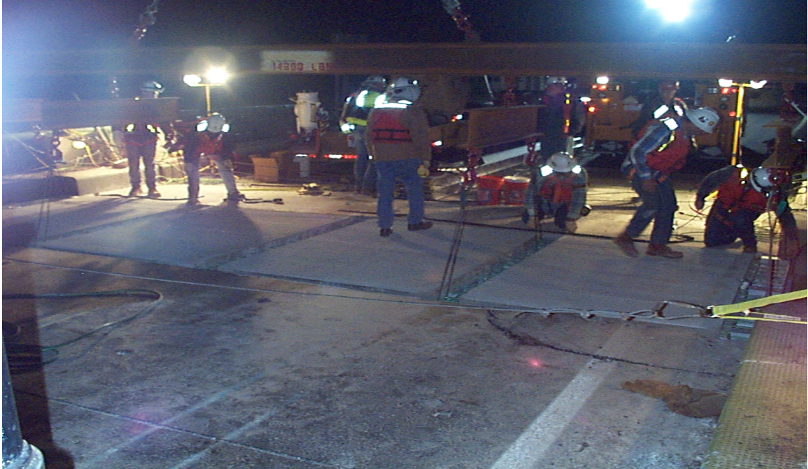
Fig. 3.21 First Exodermic Panel In-Place
