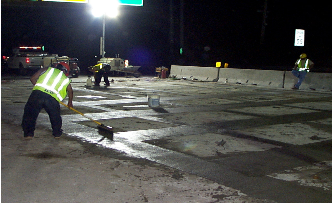
Fig. 6.40 Overview Shot of Longitudinal and Transverse Closure Pours
