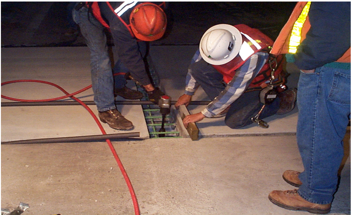
Fig. 3.24 Adjustment of Leveling Bolts on Exodermic Panel
