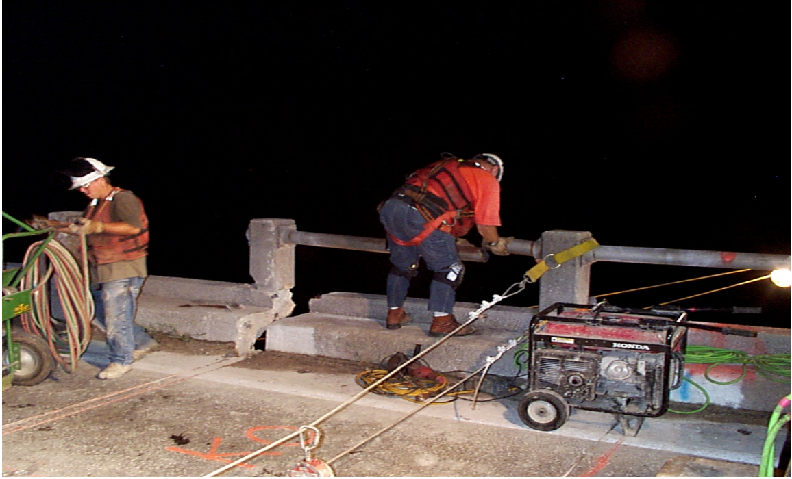
Fig. 4.4 Removal of the Barrier Rails
