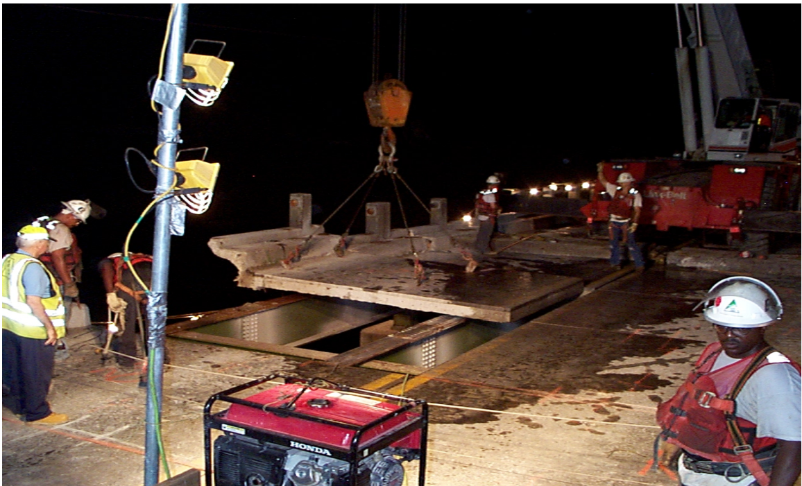
Fig. 4.5 Removal of Existing Deck Slab and Barrier
