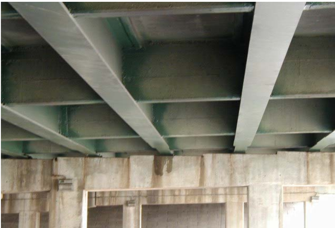
Fig. 2.20 Underneath View of Original Bridge Superstructure and Bents (2)
