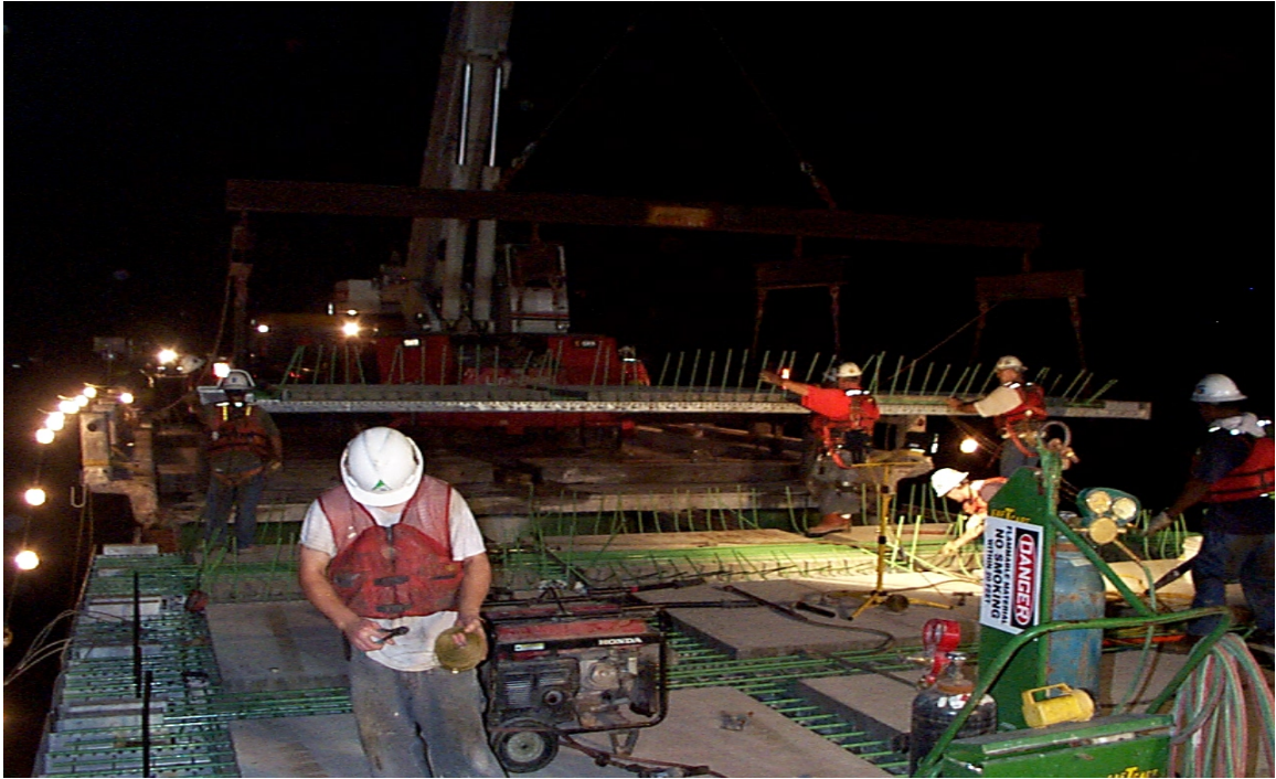
Fig 4.20 Placement of Final Two Exodermic Panels
