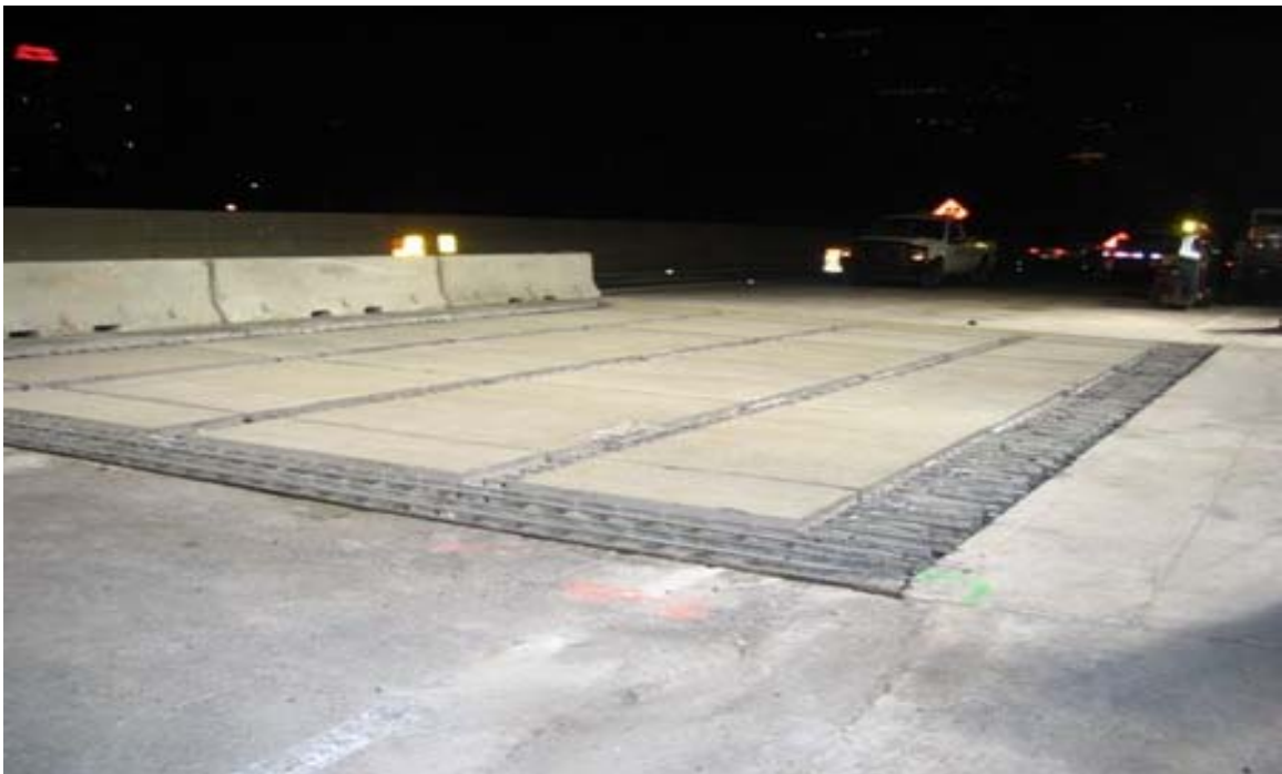
Fig. 5.37 Overview Shot of Precast Exodermic Panels In-Place
