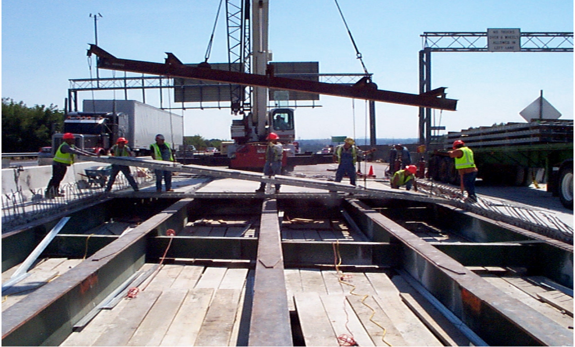
Fig. 6.16 Setting of Third Precast Exodermic Panel
