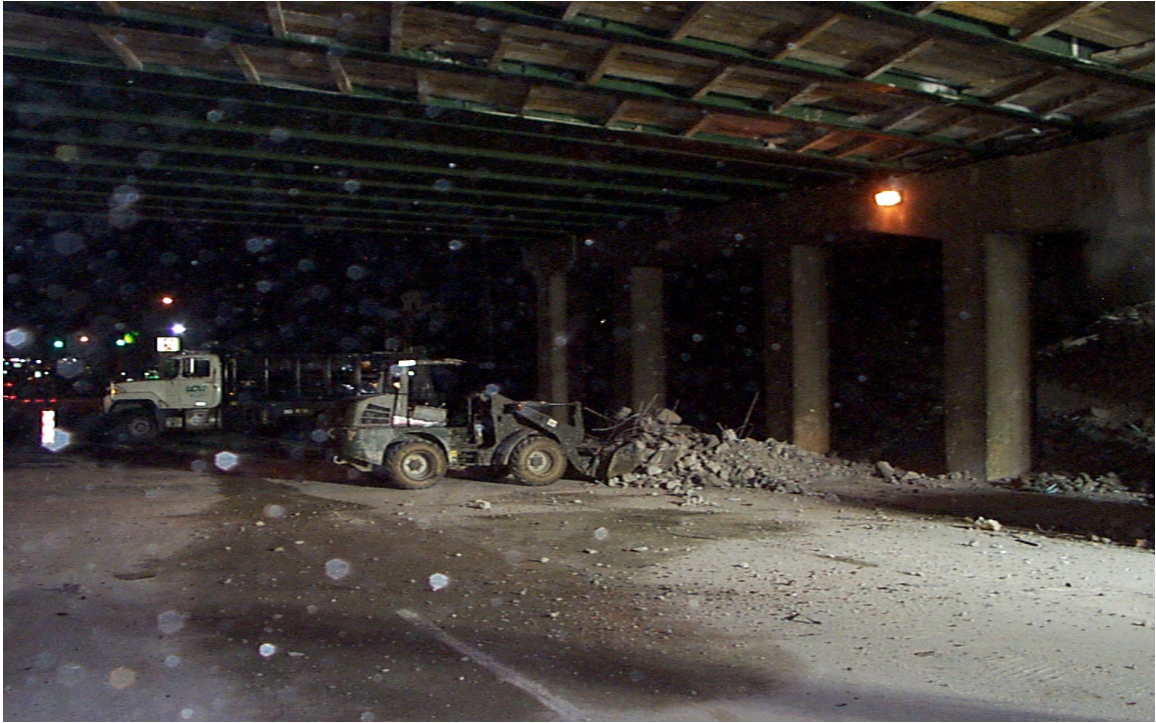
Fig. 6.10 Loading of Reinforced Concrete Debris from End-Span Edge Beam
