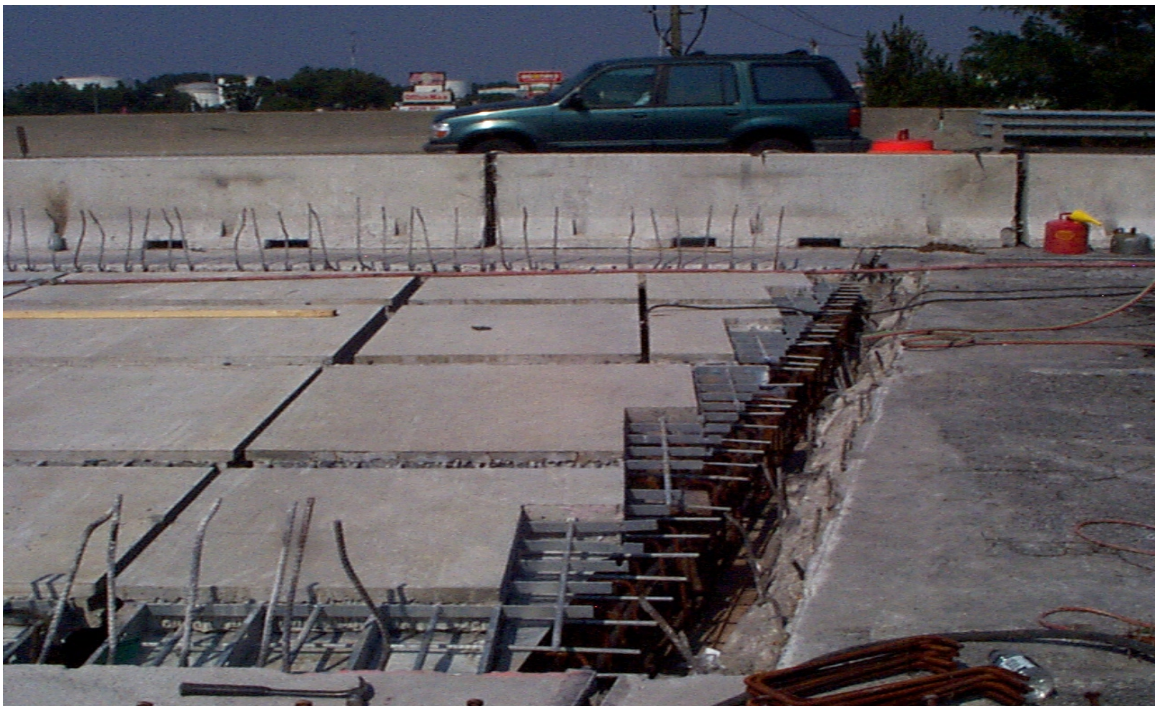
Fig. 6.21 Typical Transverse Joint at the Endwall
