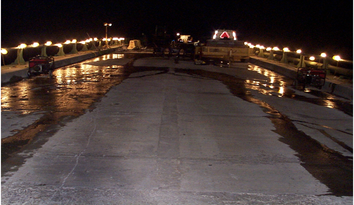
Fig. 3.35 Overview Look of Exodermic Panels before Overlay
