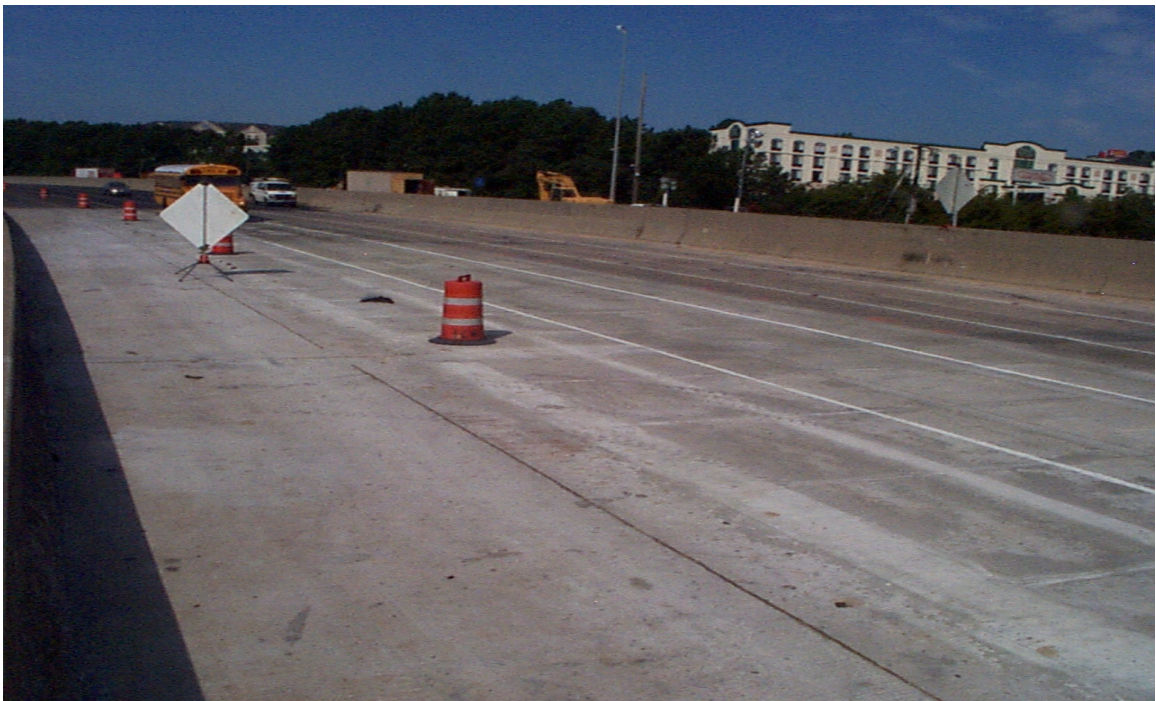
Fig. 5.47 Finished Deck Surface after Deck Replacement Work
