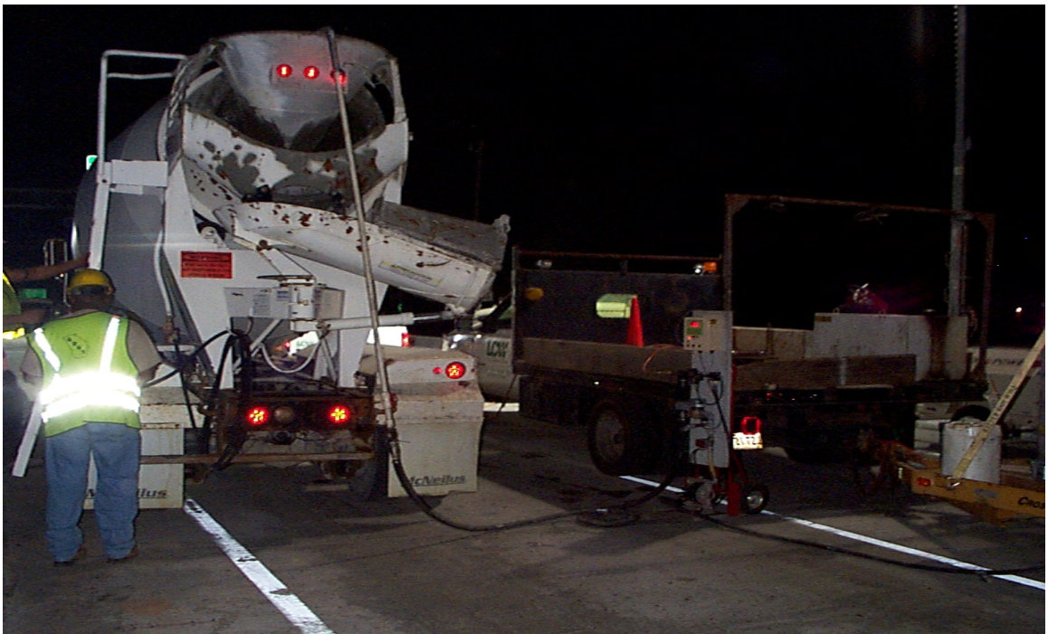
Fig. 6.33 Placement of the DCI Corrosion Inhibitor and Accelerator Admixture
