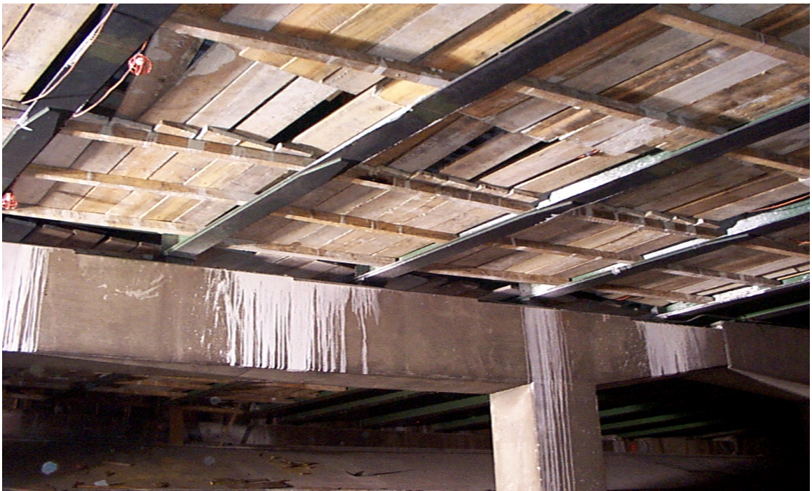
Fig. 6.13 Underneath View of Continuous Steel Girders
