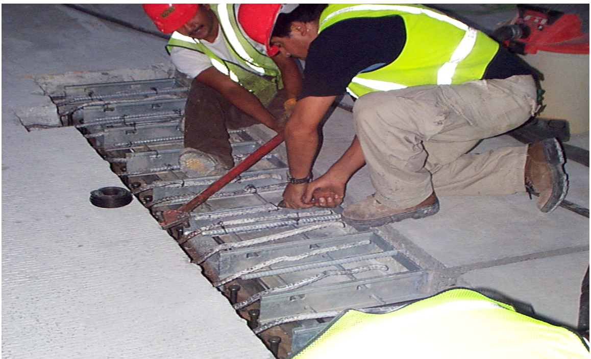
Fig. 6.25 Tying of Longitudinal Joint Negative Moment Reinforcing Bars
