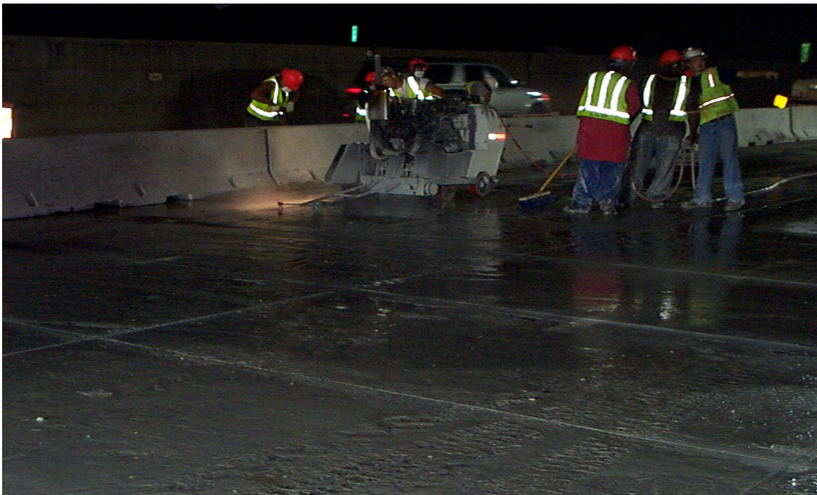
Fig. 6.3 Saw Cutting for Deck Removal
