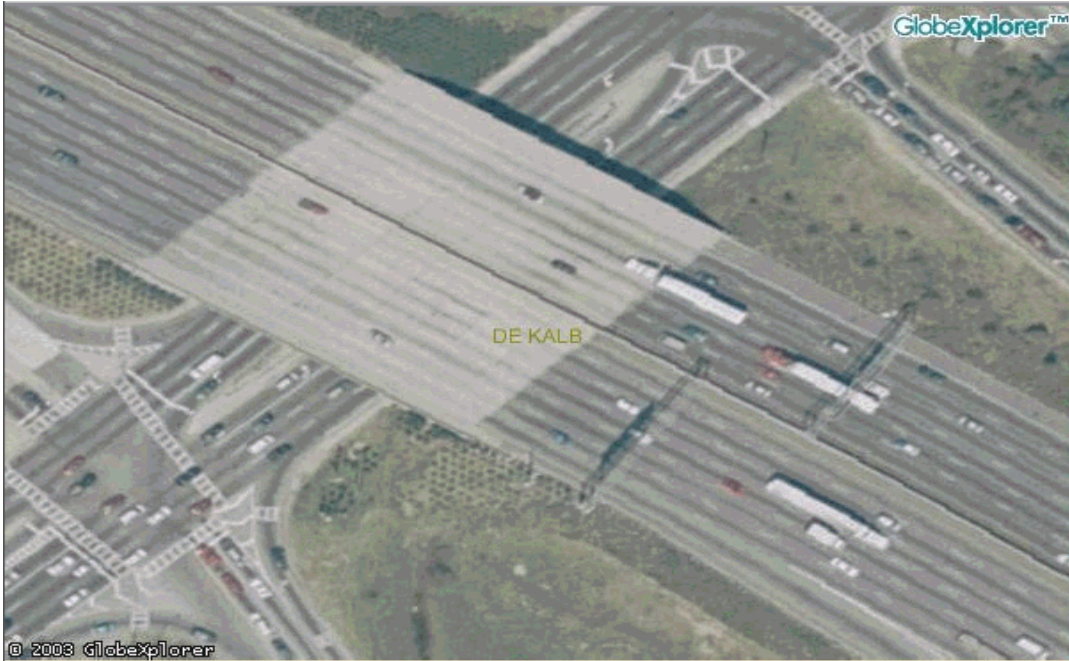
Fig. 2.14 Aerial View of I-285 over Buford Highway (2)
