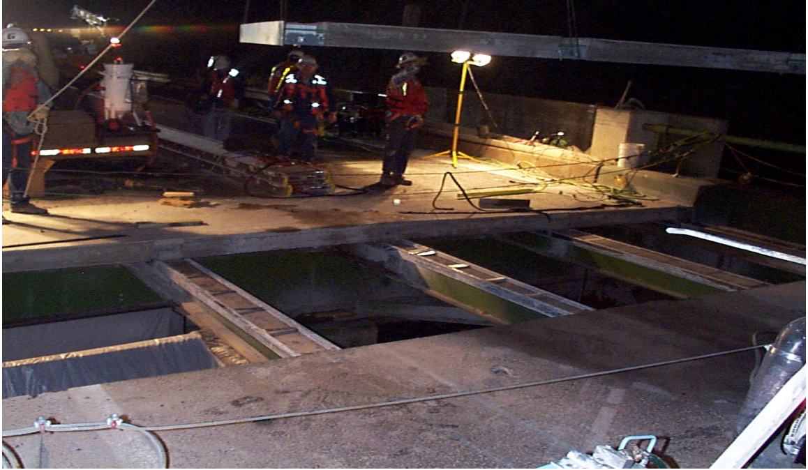
Fig. 3.19 Setting of First Exodermic Panel
