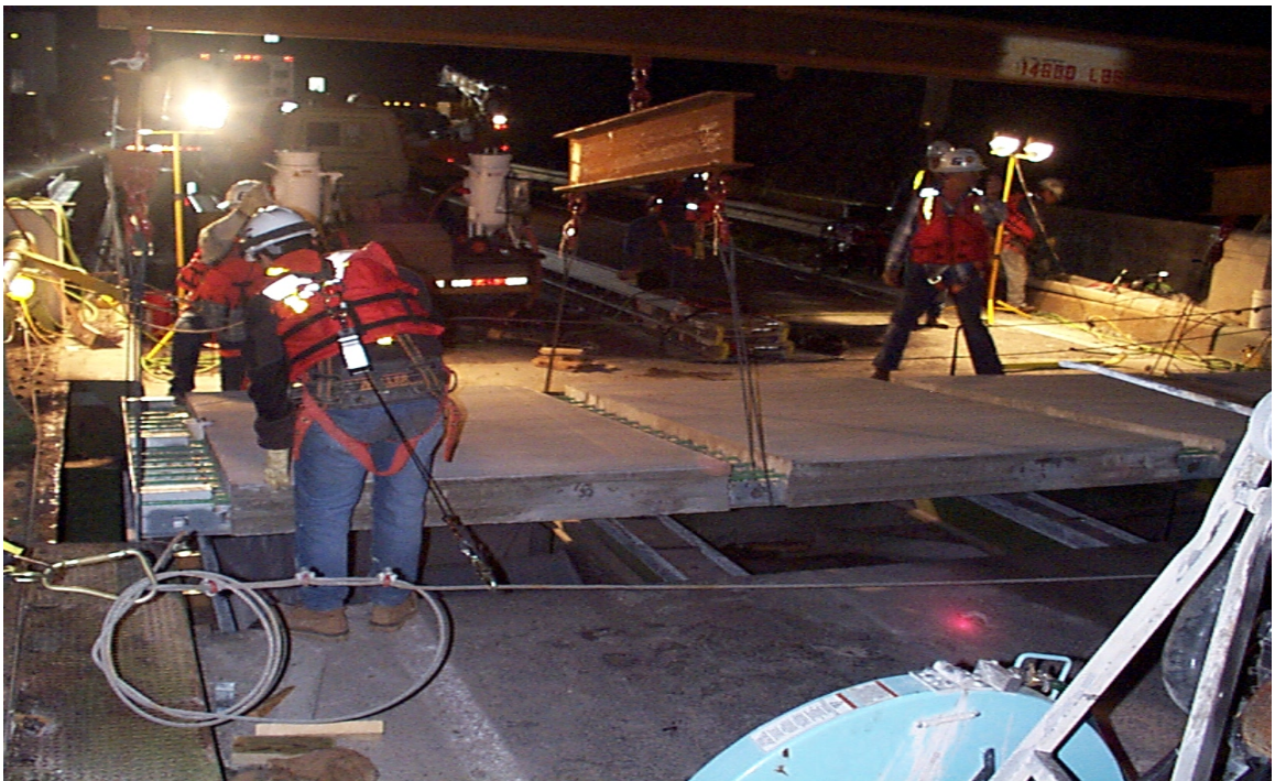
Fig. 3.20 Setting of Second Exodermic Panel
