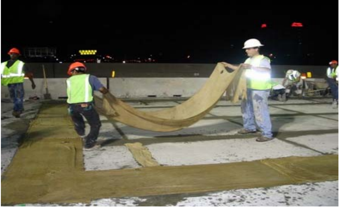
Fig. 5.44 Placement of Burlap on the Field Placed Concrete
