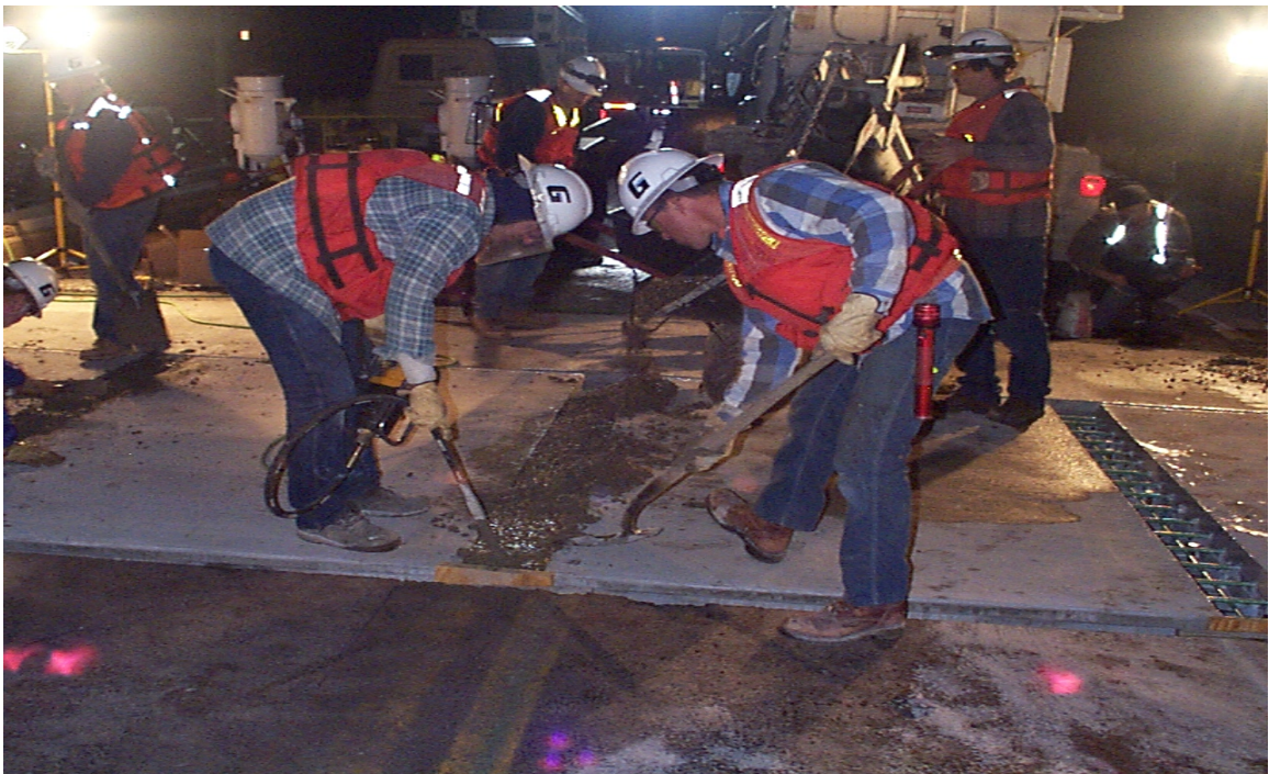
Fig. 3.28 Placement of Rapid-Setting Concrete at Stringers
