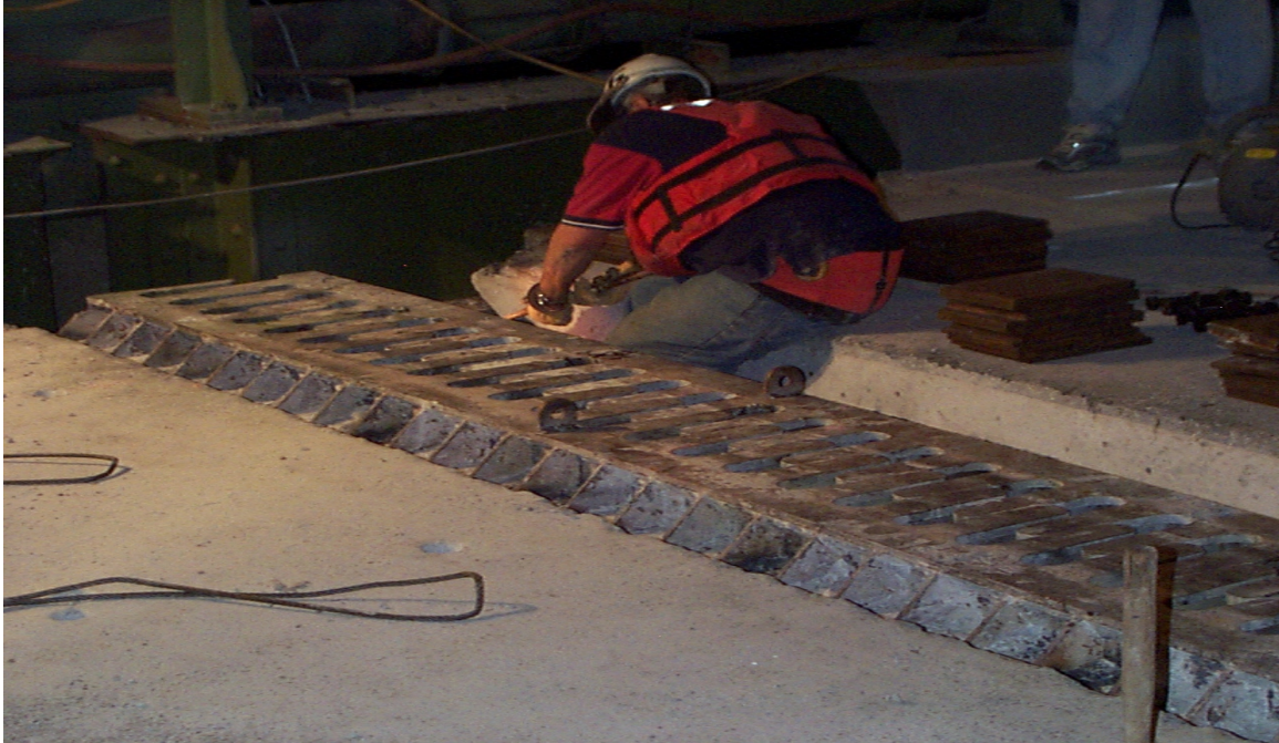
Fig. 3.39 Cutting of the Existing Bolts of Finger Joint
