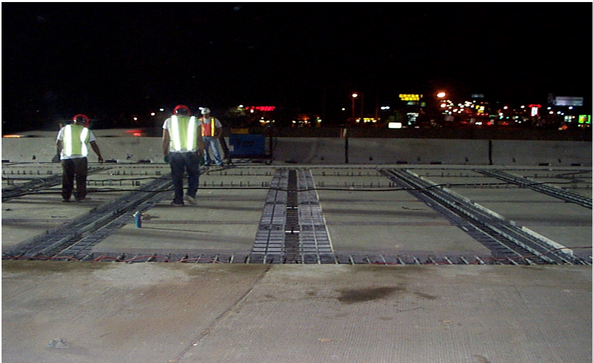
Fig. 6.27 Placement of Panels in Negative Moment Region
