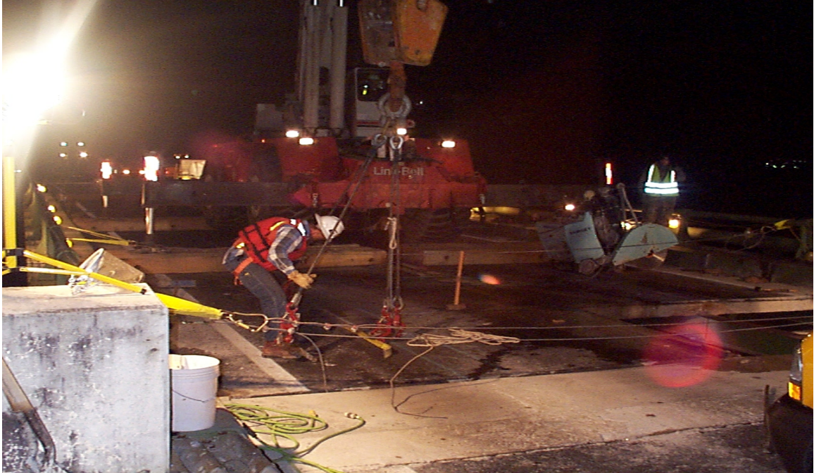
Fig 3.13 Preparing to Lift Second Section of Existing Deck
