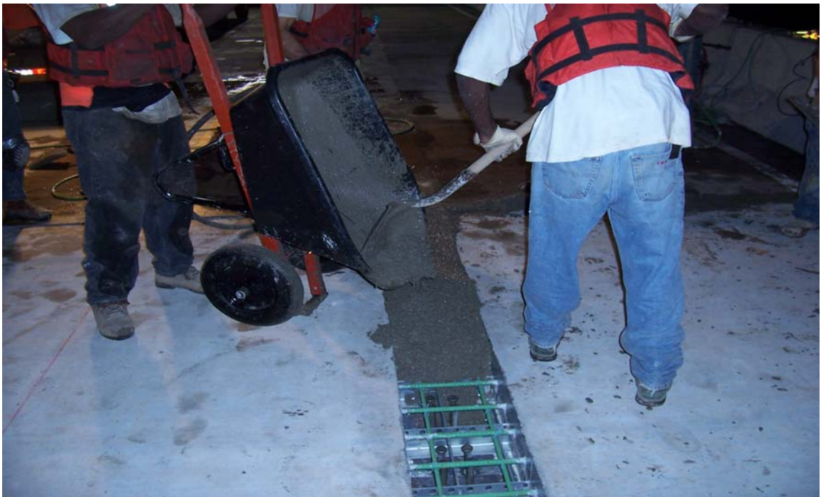
Fig. 4.21 Placement of Rapid Setting Concrete Above Stringers
