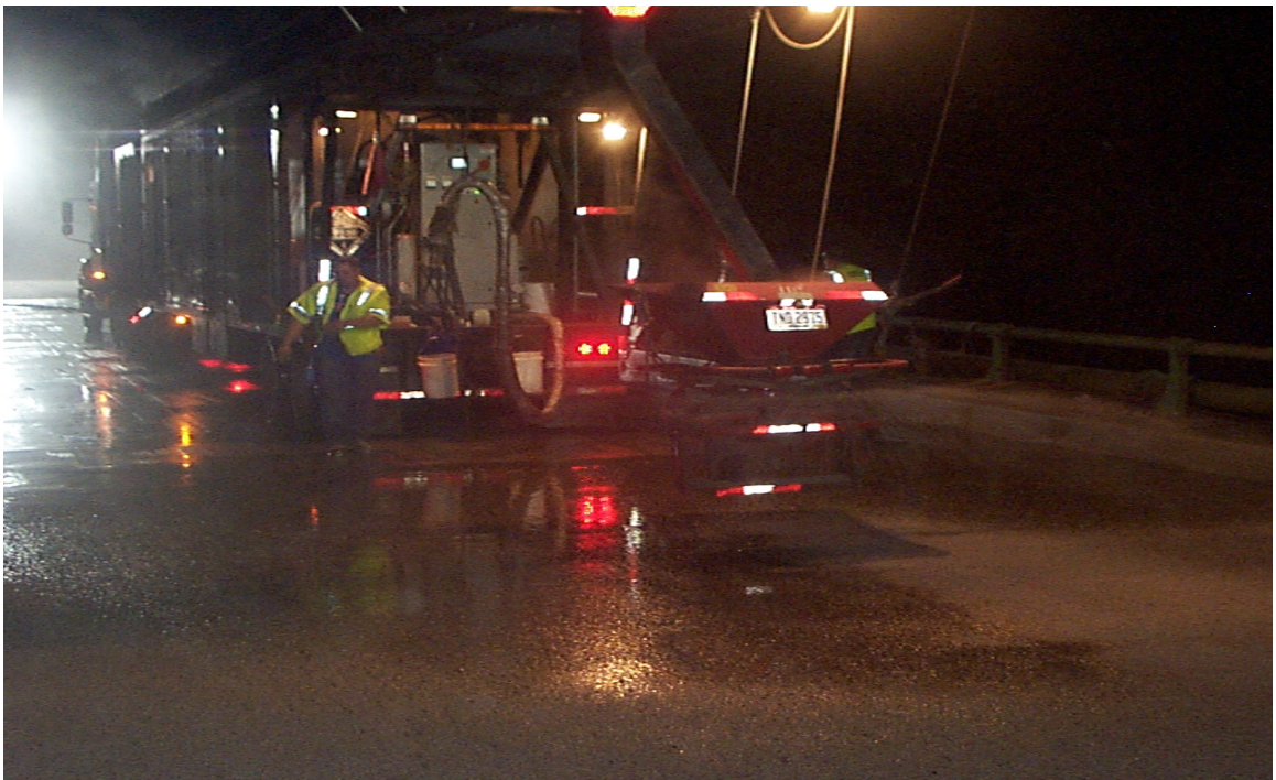
Fig. 3.50 Broadcasting of First Layer of Aggregate on Polymer Binder
