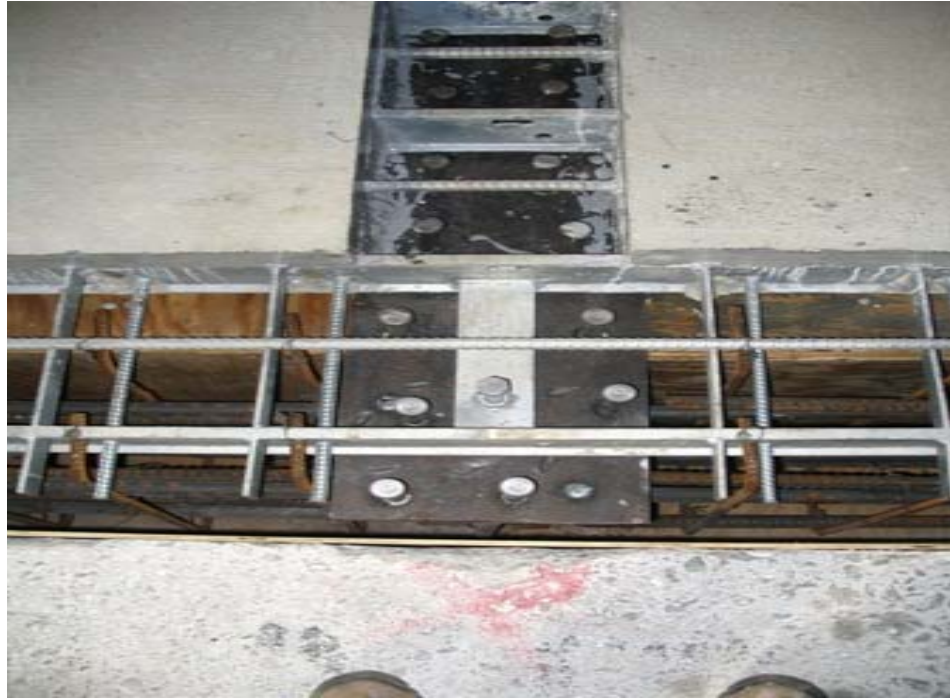
Fig. 5.38 Placement of Shear Studs
