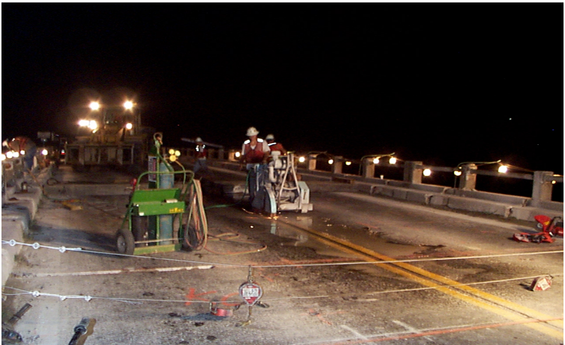
Fig. 4.3 Longitudinal Saw Cutting for Deck Removal
