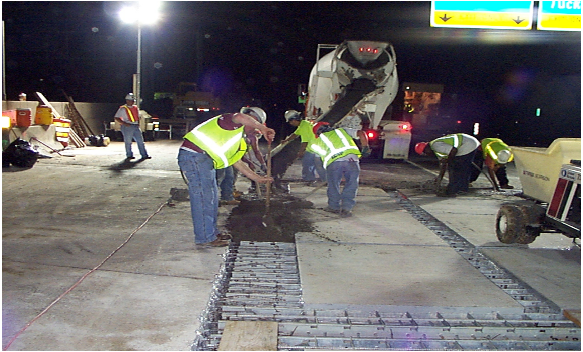
Fig. 6.36 Placement of 24 Hour Accelerated Strength Concrete
