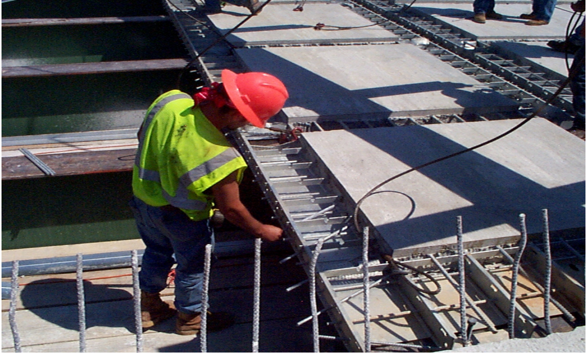
Fig. 6.18 Installation of Transverse Joint Negative Moment Reinforcing Bars
