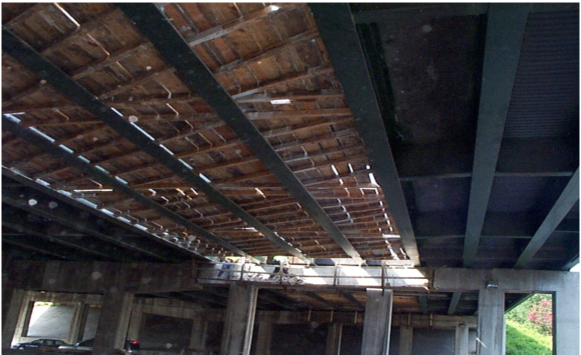
Fig. 5.51 Protective Platform Used During Deck Replacement Work
