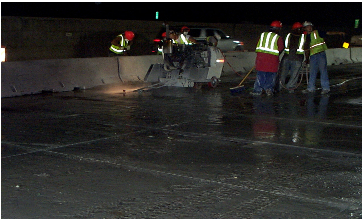
Fig. 5.7 Saw Cutting Grid Used for Deck Replacement
