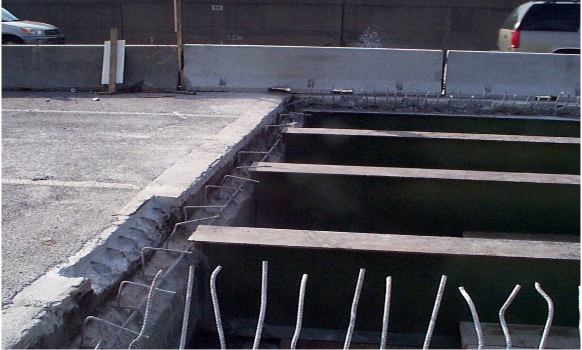
Fig. 5.42 Typical Endwall After Deck Removal
