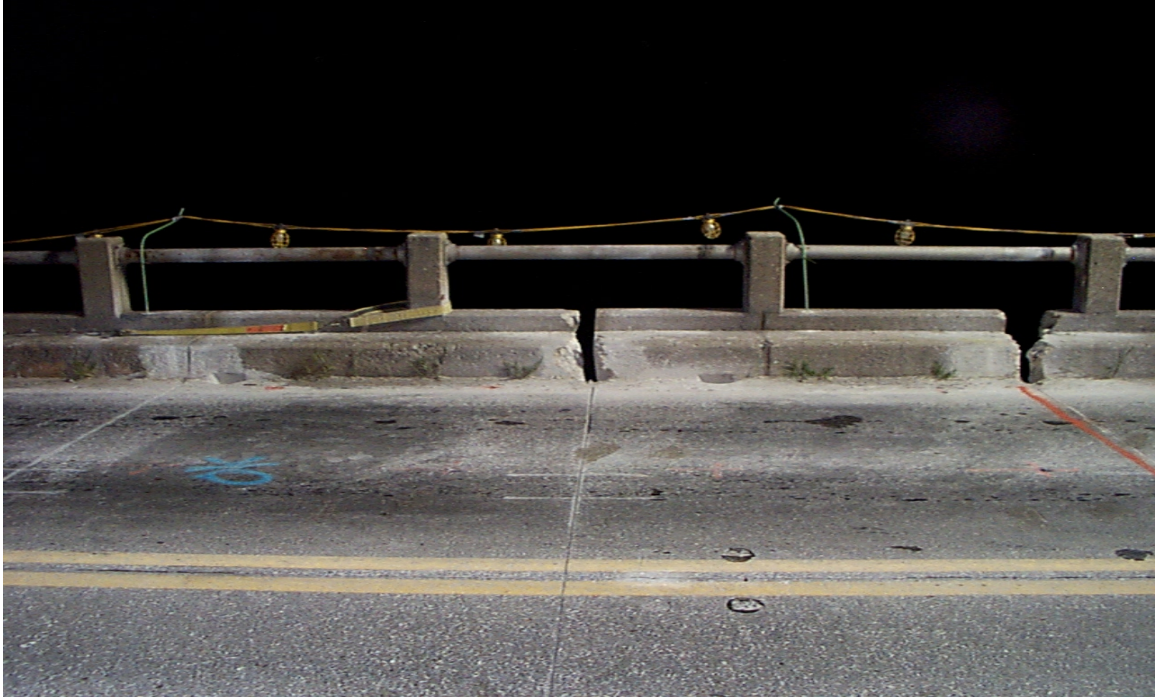
Fig. 4.2 Typical Transverse Saw Cuts for Deck Removal
