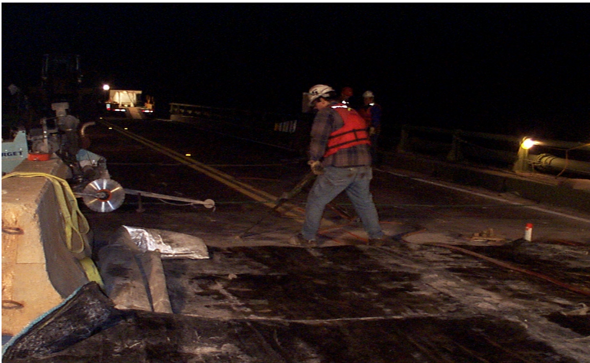
Fig. 3.4 Core Drilling of Pick-Up Points for Deck Removal Next Night
