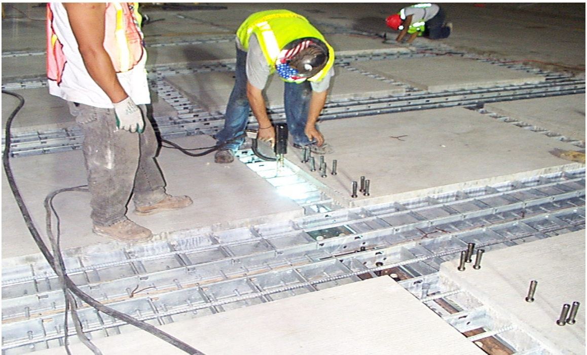
Fig. 6.29 Placement of Shear Studs
