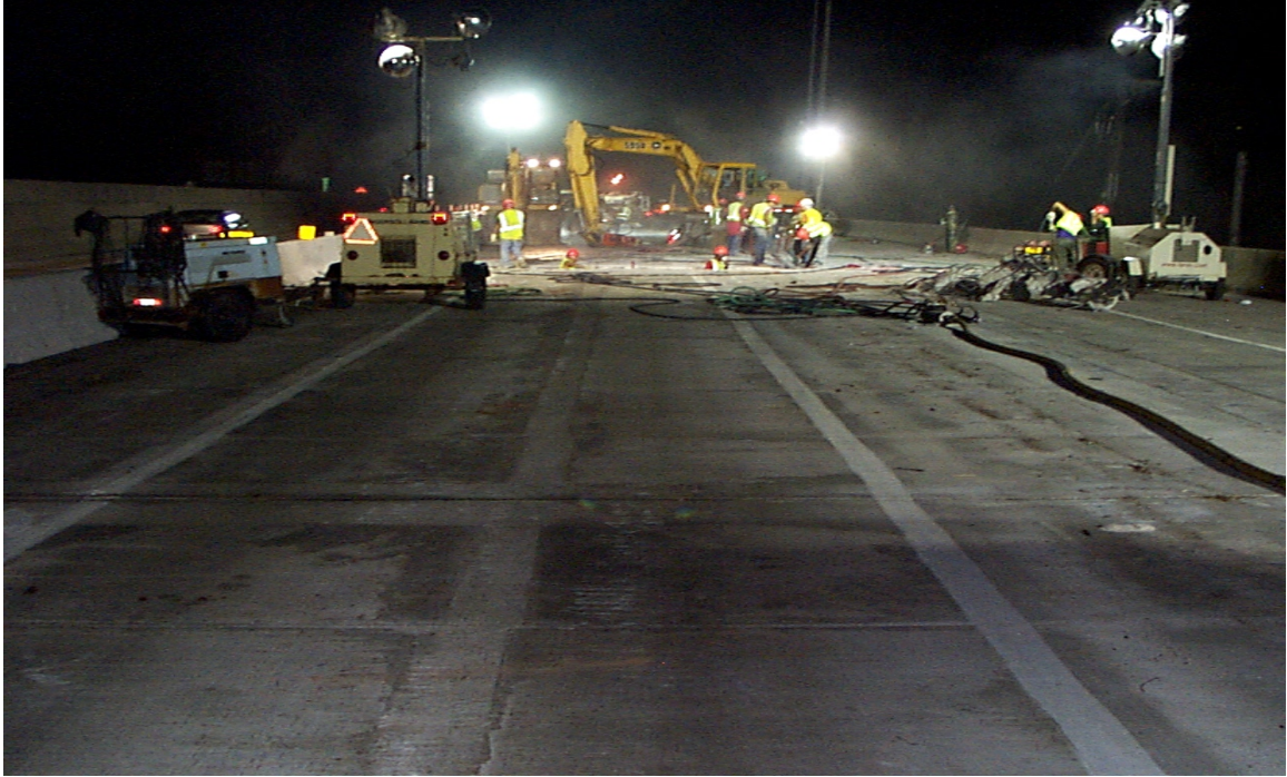
Fig. 5.46 Overview Shot of Approximately 120' of Deck Replacement
