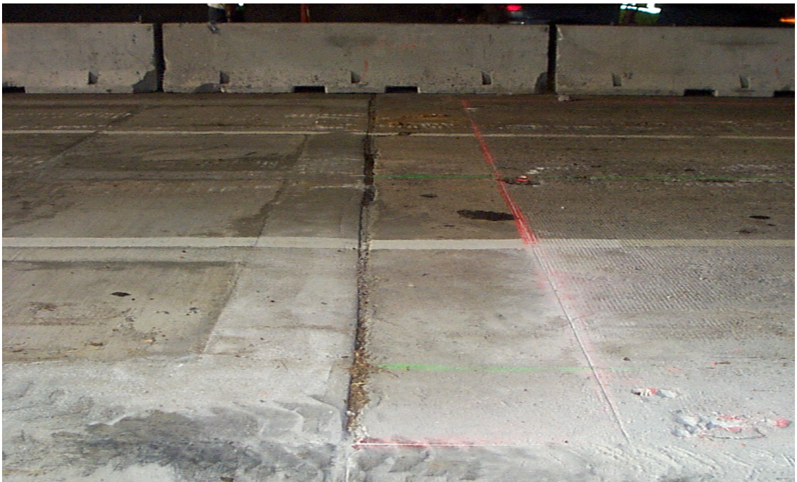
Fig. 5.49 Typical Existing Expansion Joint during Deck Replacement
