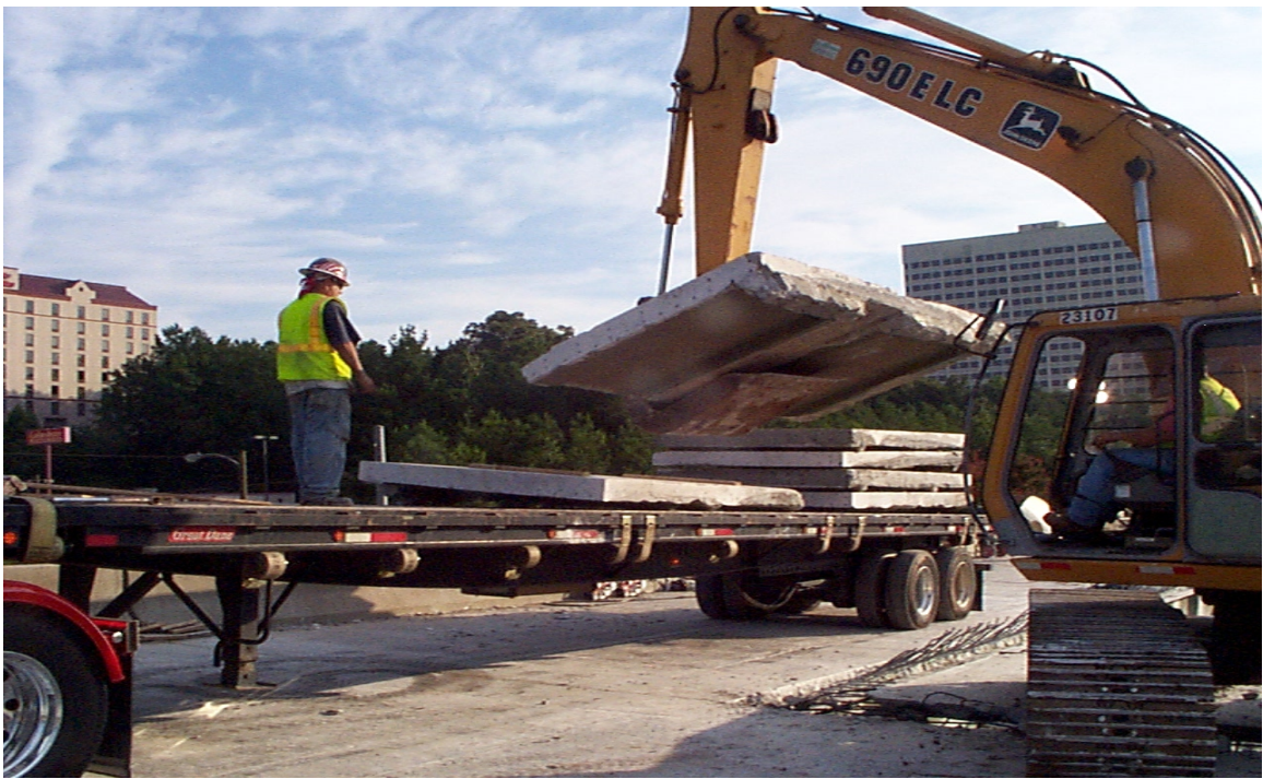
Fig. 7.11 Loading the Existing Deck with Excavator
