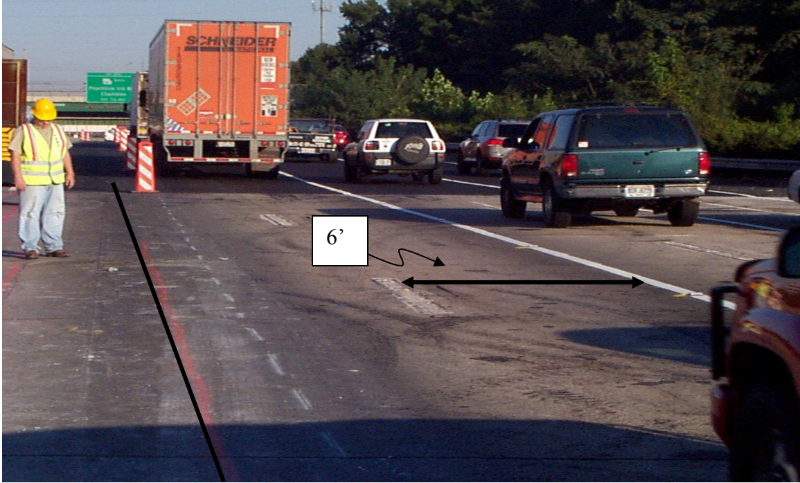
Fig. 6.2 Installation of Lane Shift
