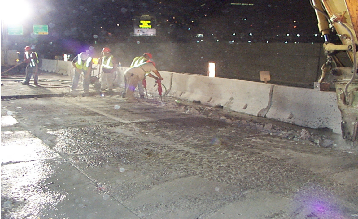
Fig. 6.6 Chipping around Negative Moment Reinforcing Bars
