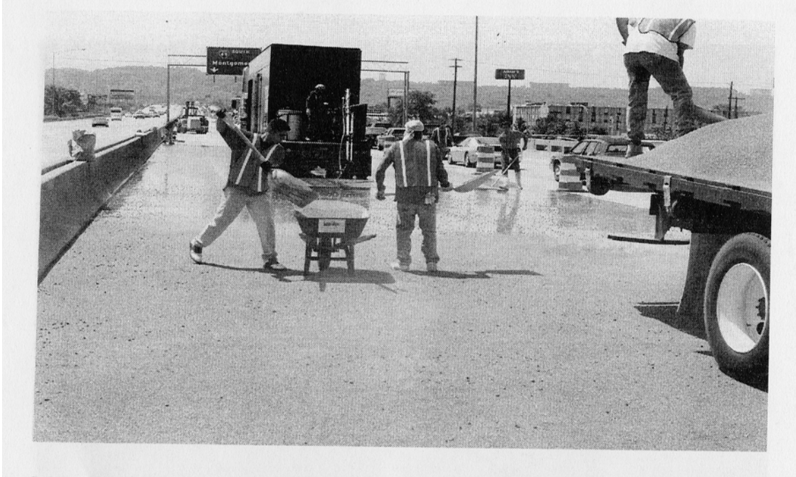
Fig. 2.26 Broadcasting Fine Aggregate from Truck as it Moves Along Bridge Deck (4)
