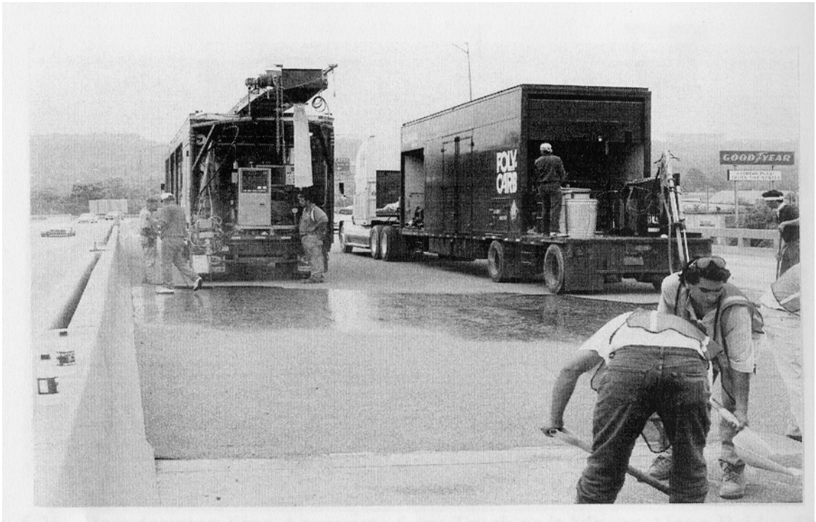
Fig. 2.27 Application of Second Polymer Concrete Layer (4)
