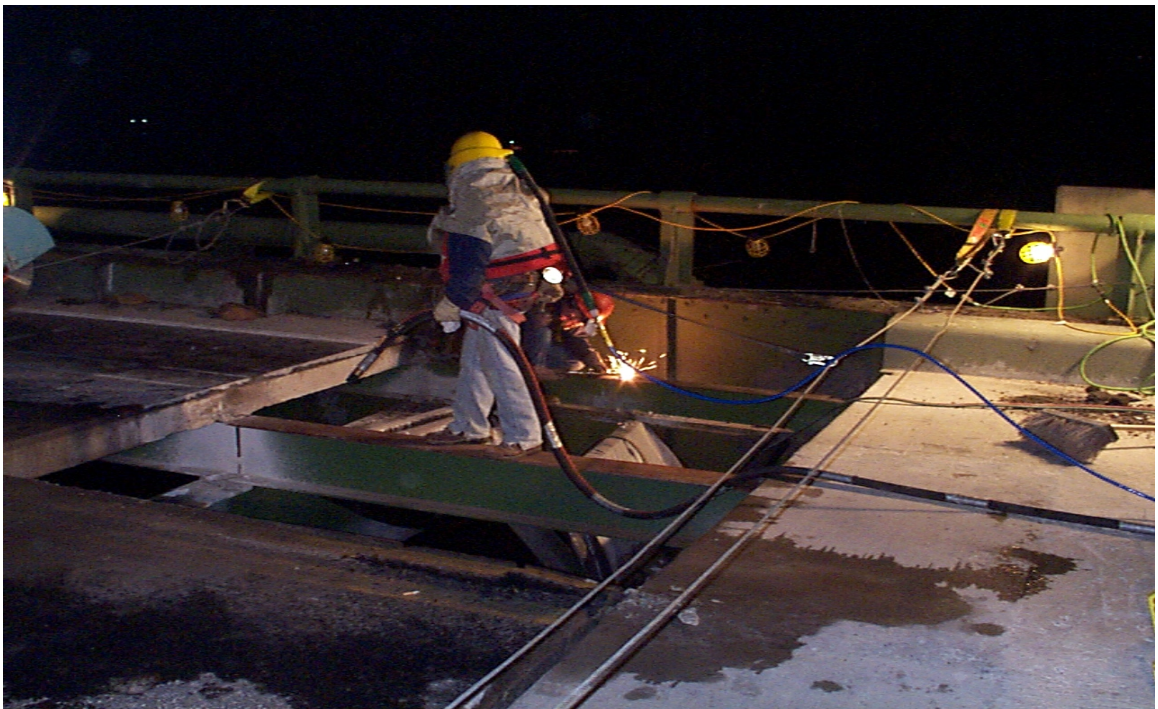
Fig. 3.16 Sand Blasting and Torching of Stringer's Top Flange
