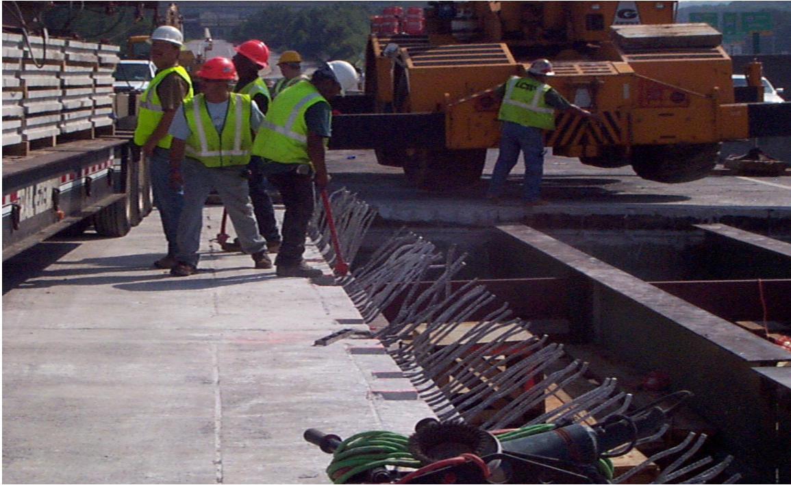
Fig. 5.28 Additional Bending of Rebar for Placement of Exodermic Panels
