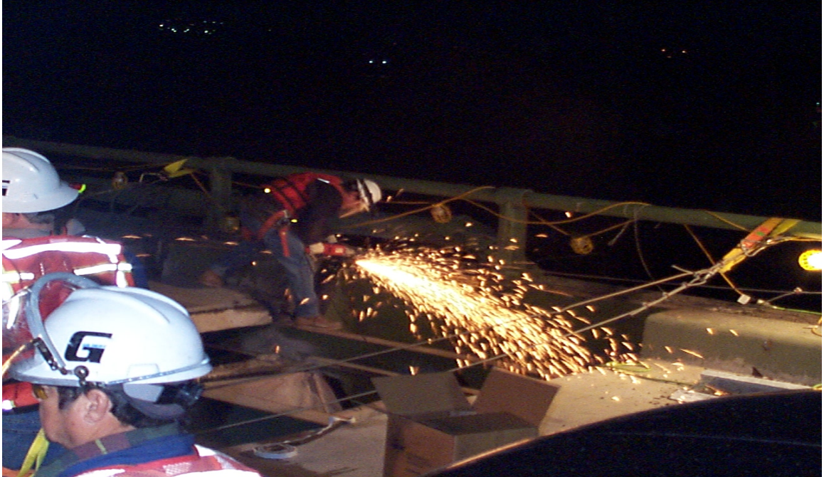
Fig. 3.17 Grinding of Weld Plugs
