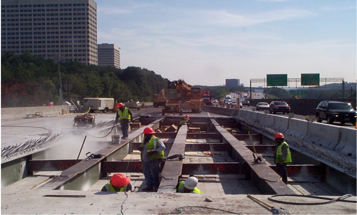
Fig. 5.20 View of Steel Girders After the Removal of the Existing Deck
