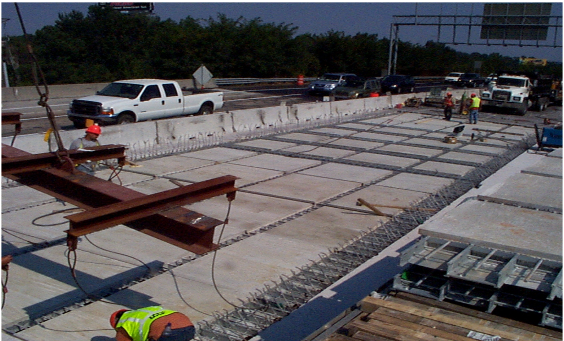
Fig. 6.19 Overview Shot of Precast Exodermic Panels In-Place
