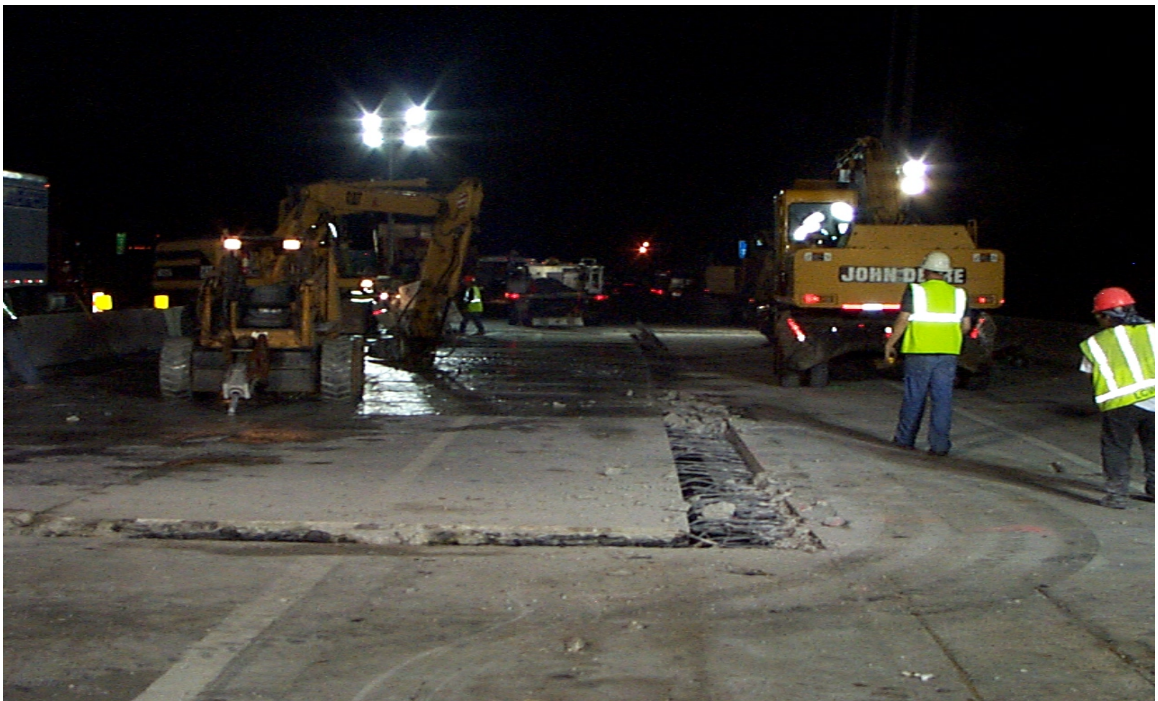
Fig. 6.5 Deck Removal around Existing Negative Moment Reinforcing Bars
