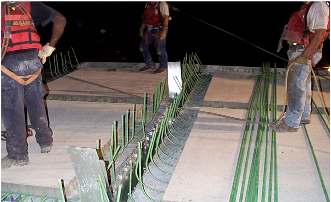
Fig. 4.13 Typical Transverse Joint in Negative Moment Region
