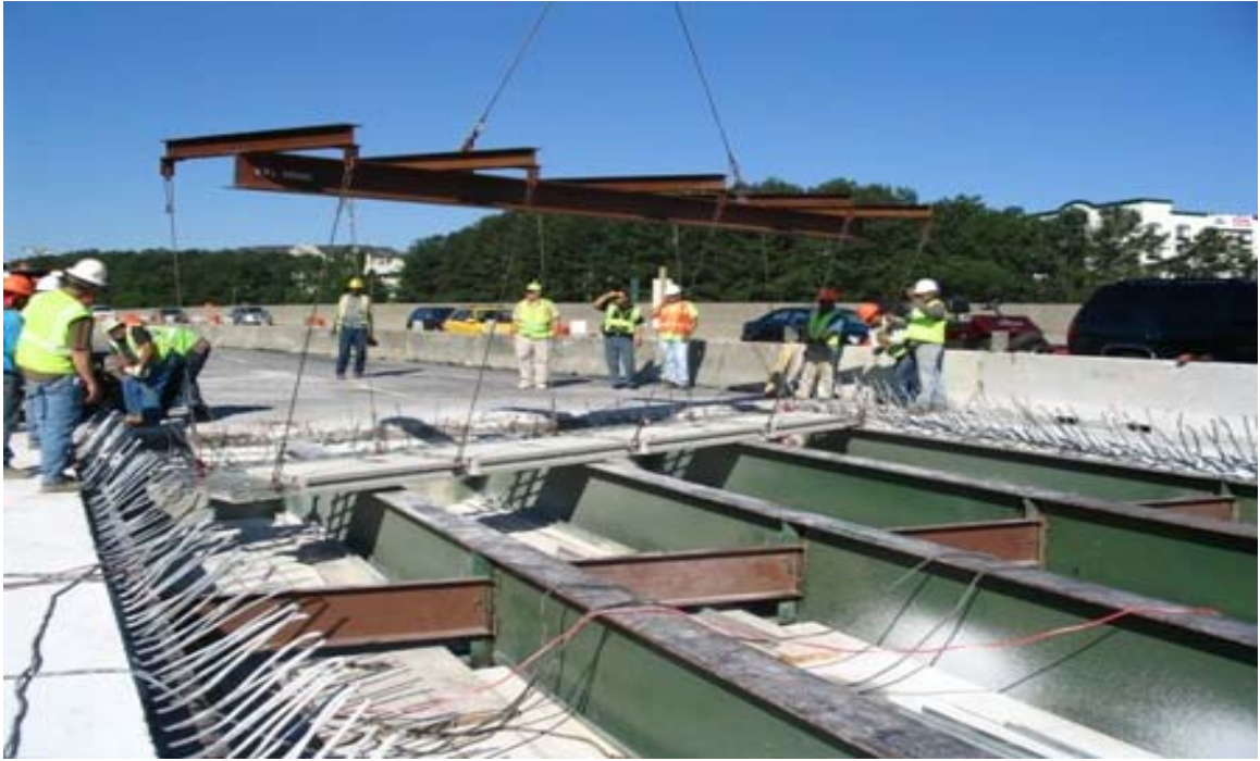
Fig. 5.26 Setting of First Exodermic Panel
