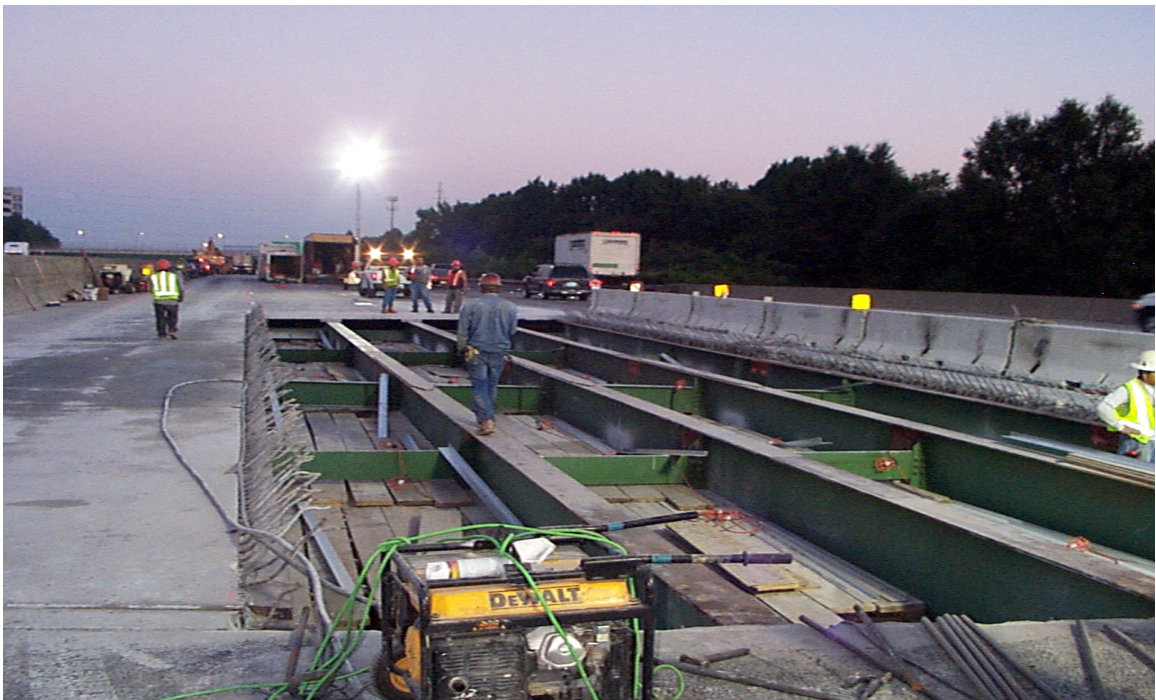
Fig. 6.7 View of Steel Girders after the Removal of the Existing Deck
