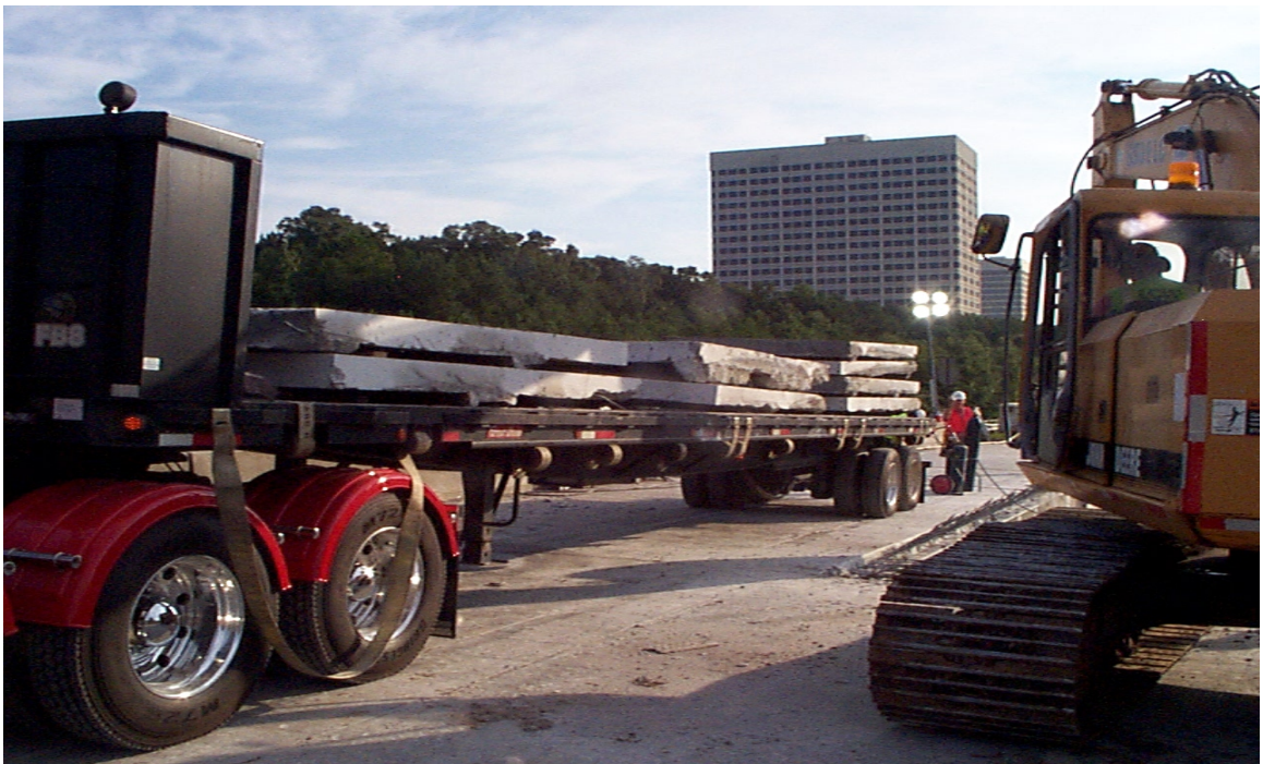
Fig. 5.19 Loading of Deck Panels onto Low-Boy Trailer
