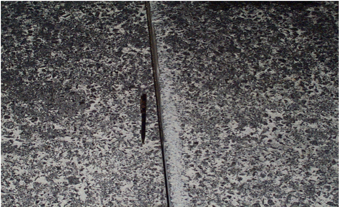
Fig. 3.8 Close-Up of Typical Saw Cut
