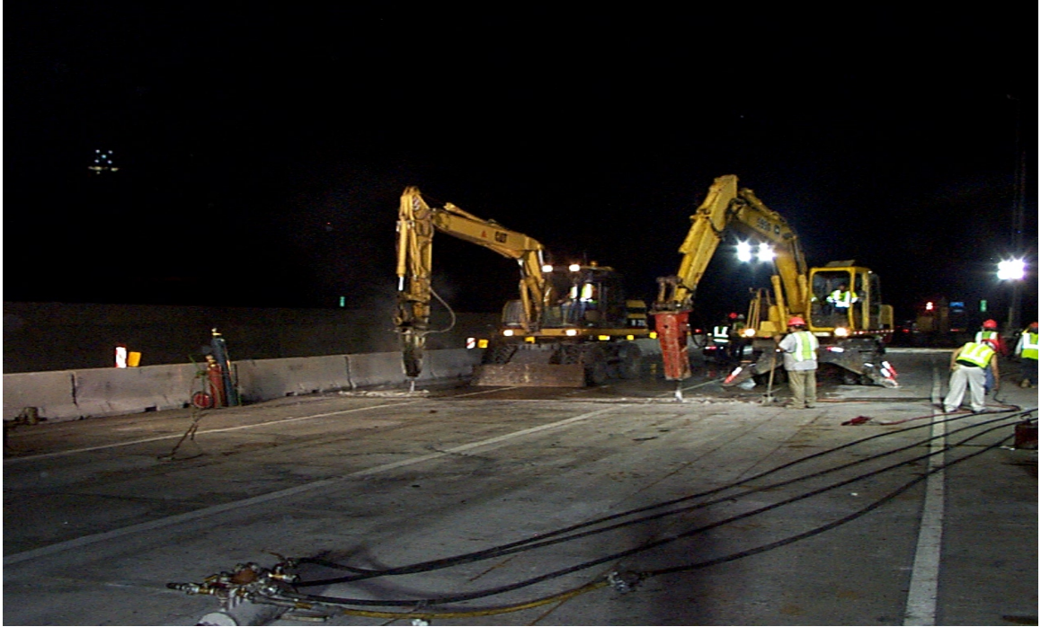
Fig. 6.4 Removal of Existing Deck
