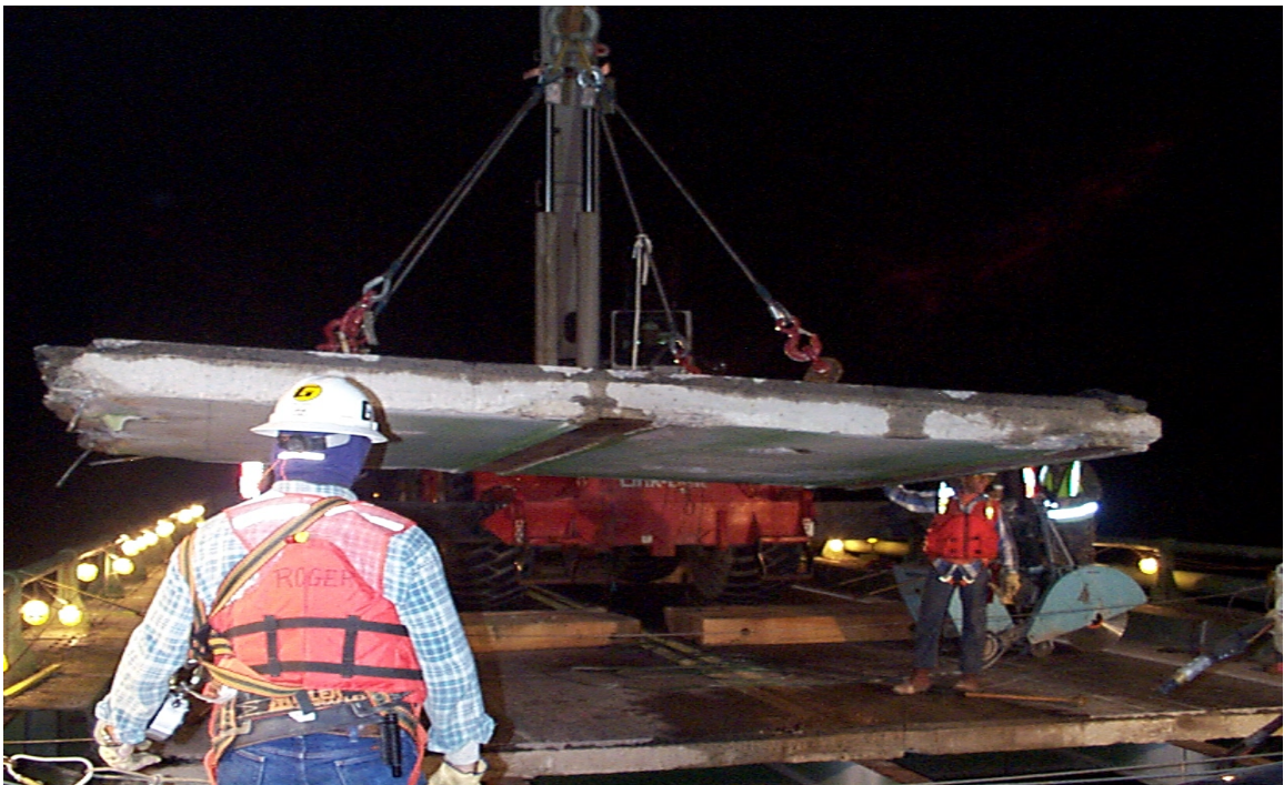
Fig 3.14 Second Section of Existing Deck Removed
