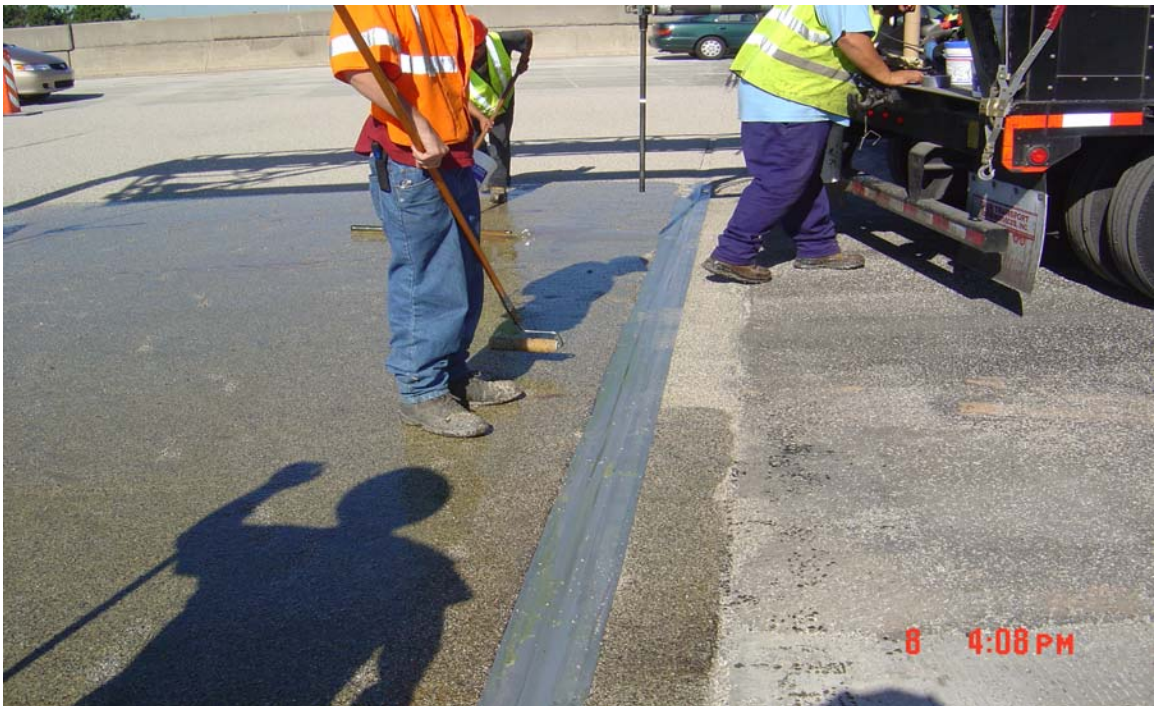
Fig. 5.61 Typical Endwall Joint During Second Application of Co-Polymer Overlay
