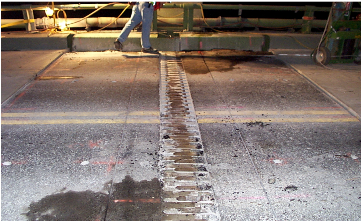
Fig. 3.36 Finger Joint View before the Replacement Process
