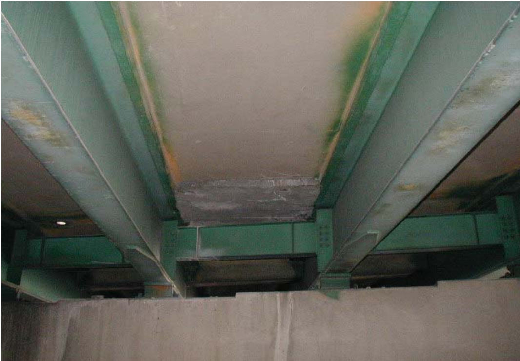
Fig. 2.15 Underside View of Original Section of Bridge (2)
