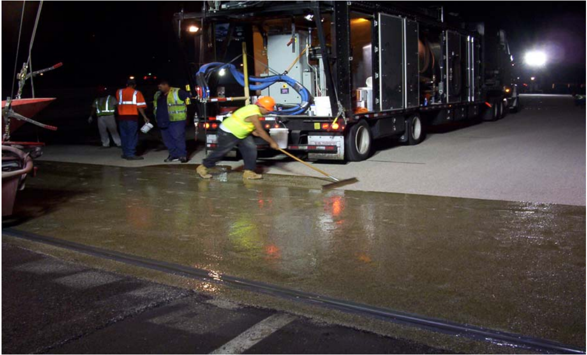
Fig. 5.58 Squeegeeing-on of the Epoxy Based Co-Polymer Binder
