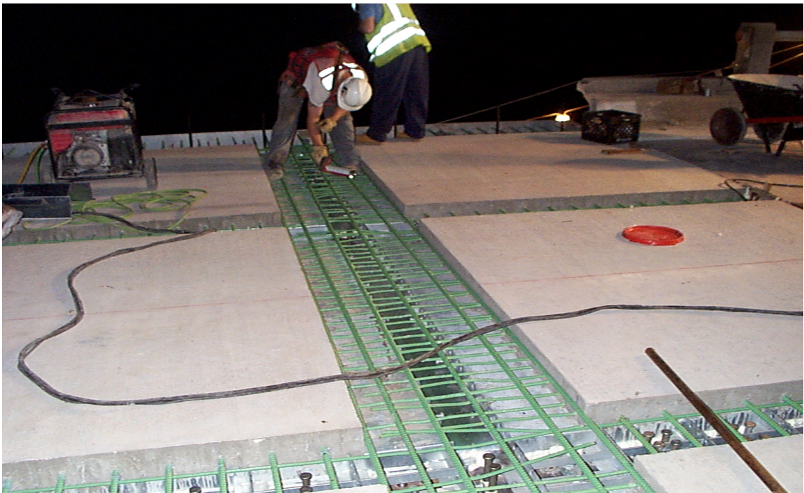
Fig. 4.15 Steel Reinforcement in the Negative Moment Regions
