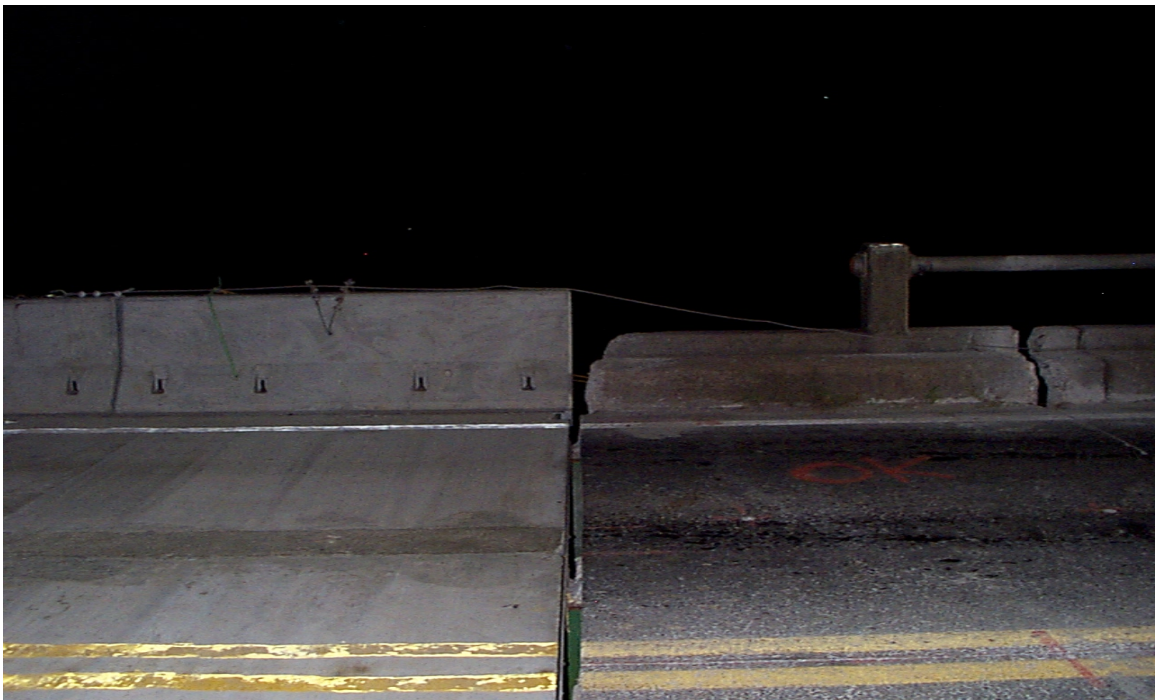
Fig. 4.25 Typical New Deck-Existing Deck Transverse Joint
