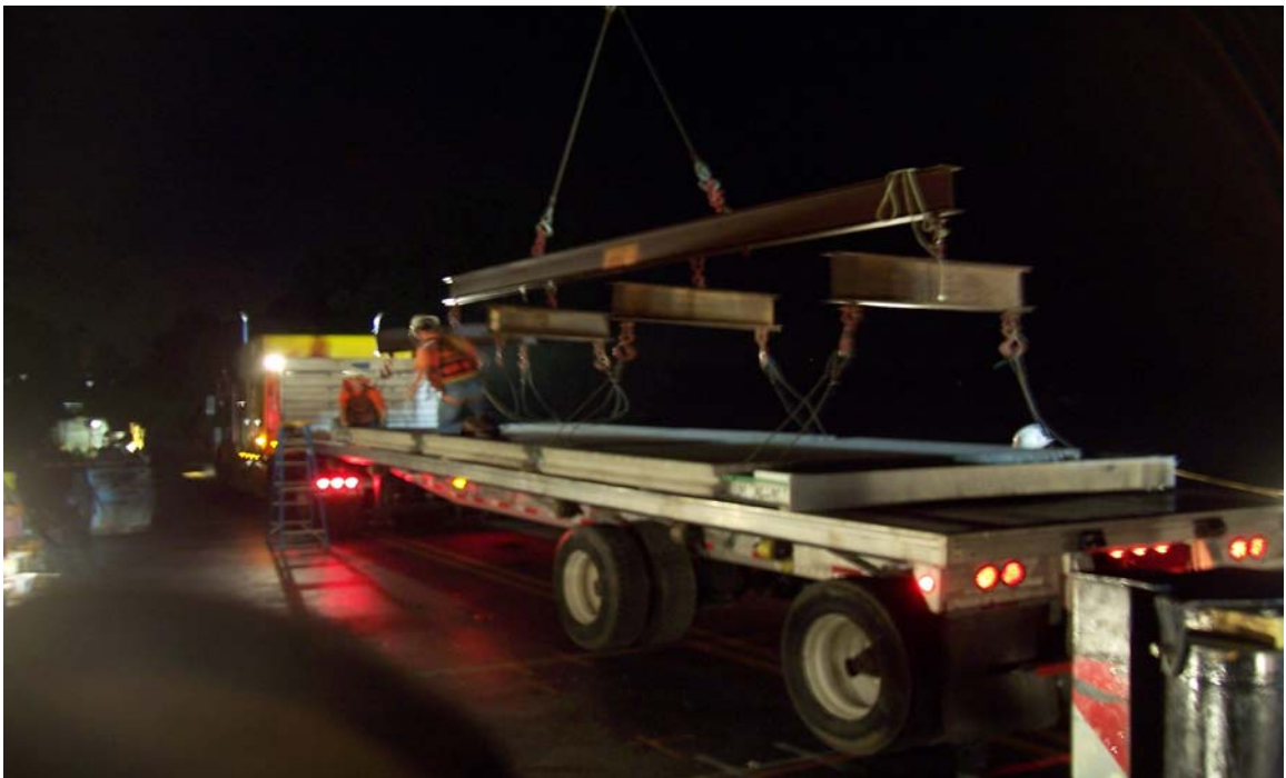
Fig. 4.9 Delivery of Precast Exodermic Panels on Low-Boy Truck
