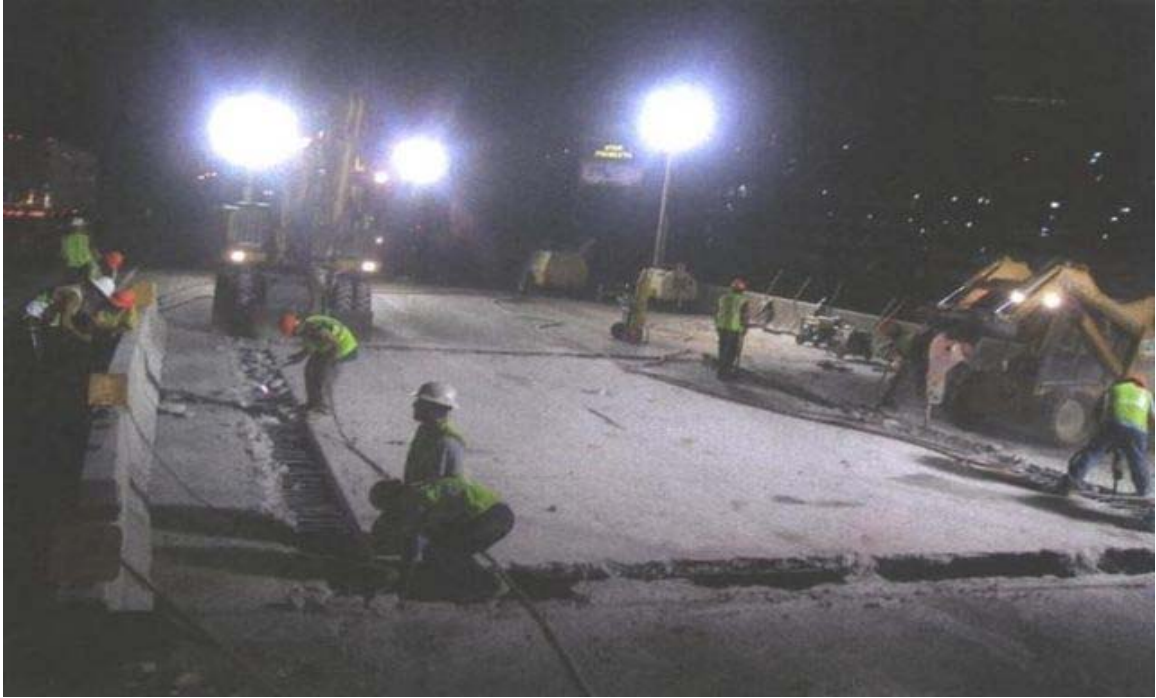
Fig. 5.16 Approximately 2' Width of Deck Removal Around Perimeter
