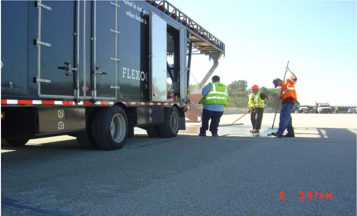
Fig. 5.56 Application of Second Co-Polymer Overlay Layer
