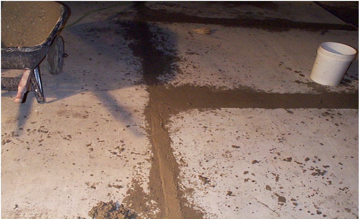
Fig. 3.30 Concrete Shear Key Just after Closure Pour
