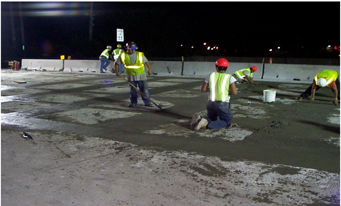
Fig. 6.39 Finishing of the Accelerated Concrete
