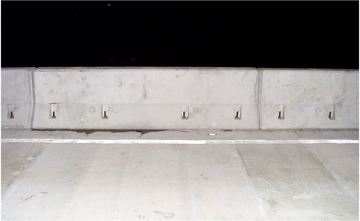
Fig. 4.22 Precast Jersey Barrier In-Place
