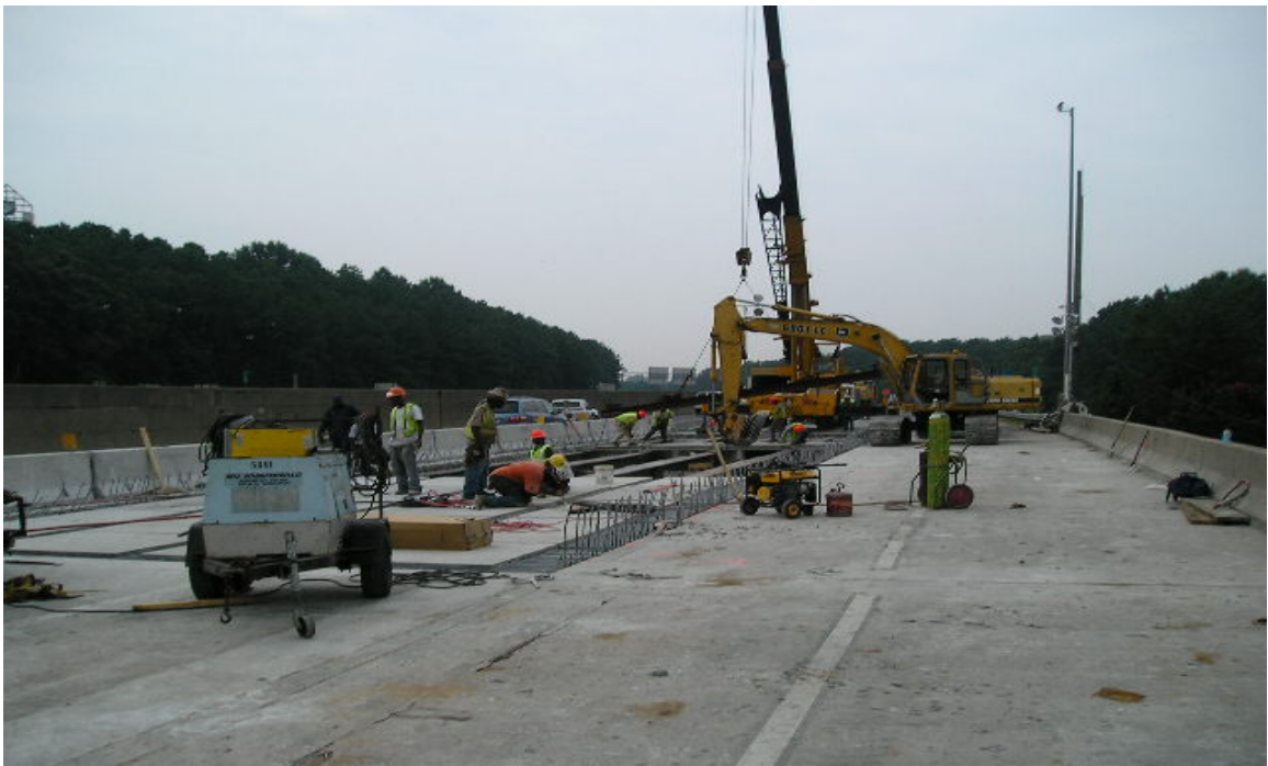
Fig. 5.33 Continuous Setting of the Exodermic Panels
