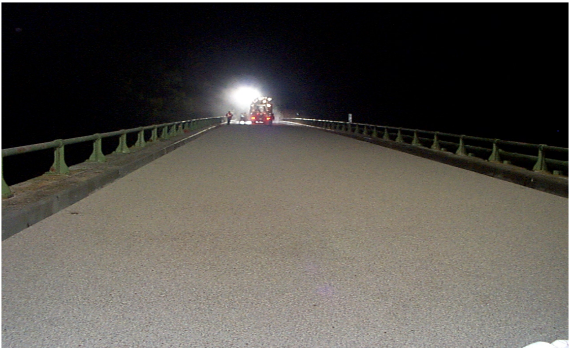
Fig. 3.52 View of First Layer of Overlay on Spans 1 through 3
