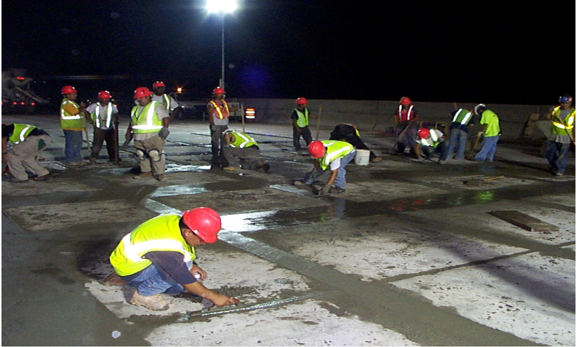
Fig. 6.38 Smoothing of the 24 Hour Accelerated Concrete
