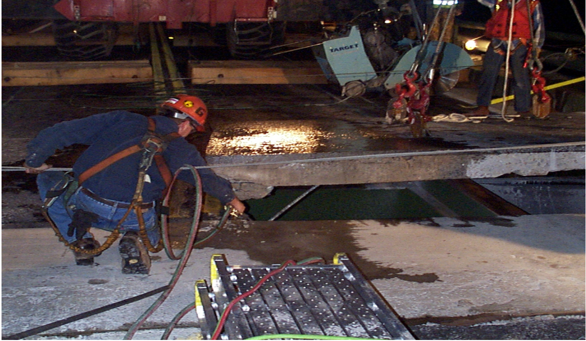
Fig. 3.11 Cutting of Reinforcement Bars Next to Stringers
