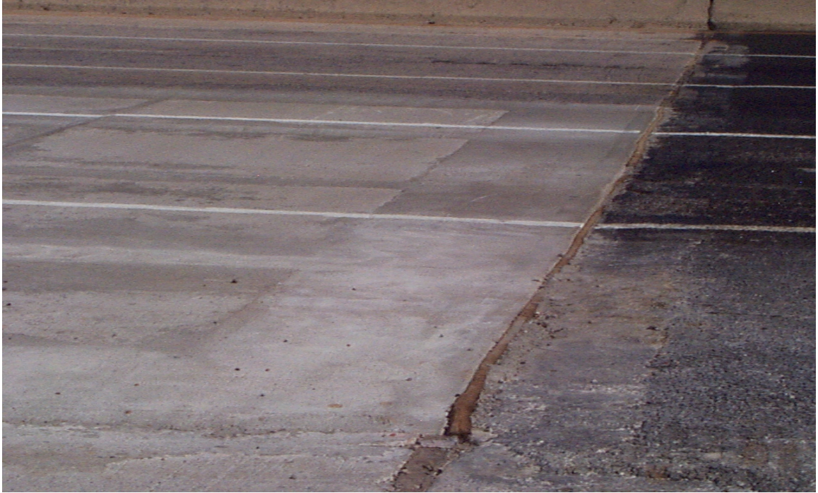
Fig. 5.50 Typical Expansion Joint Located at Endwall
