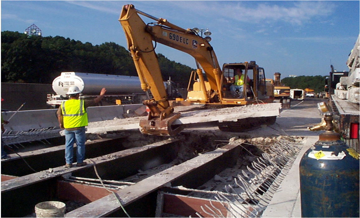
Fig. 7.10 Excavator with Grapple Attachment
