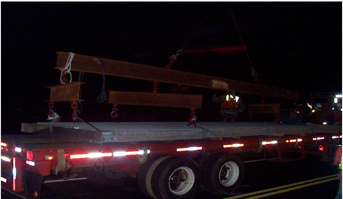
Fig. 3.2 Lift Spreader Being Assembled to Exodermic Panel
