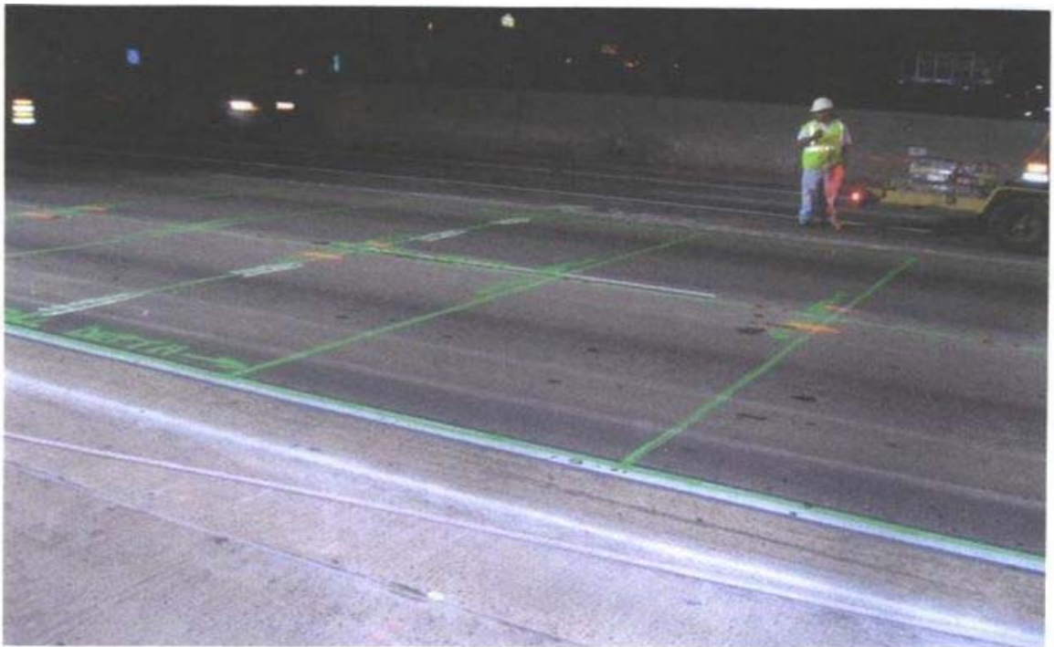
Fig. 5.5 Layout of Saw Cutting
