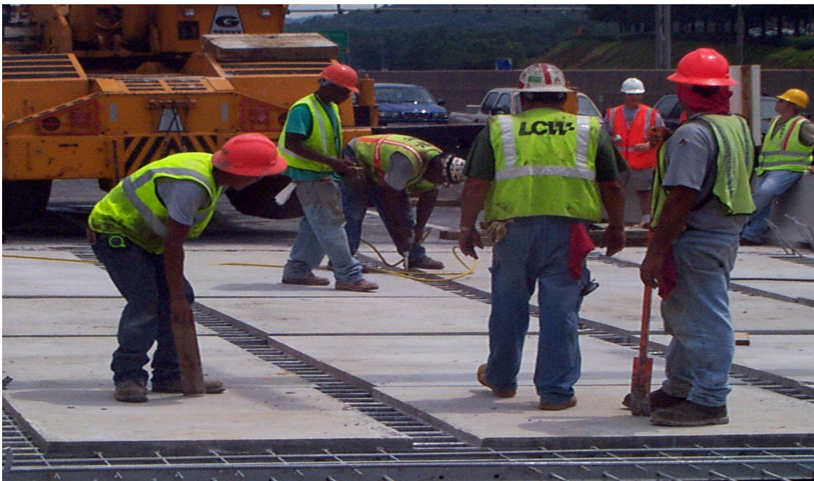
Fig. 5.35 Adjustment of the Leveling Bolts
