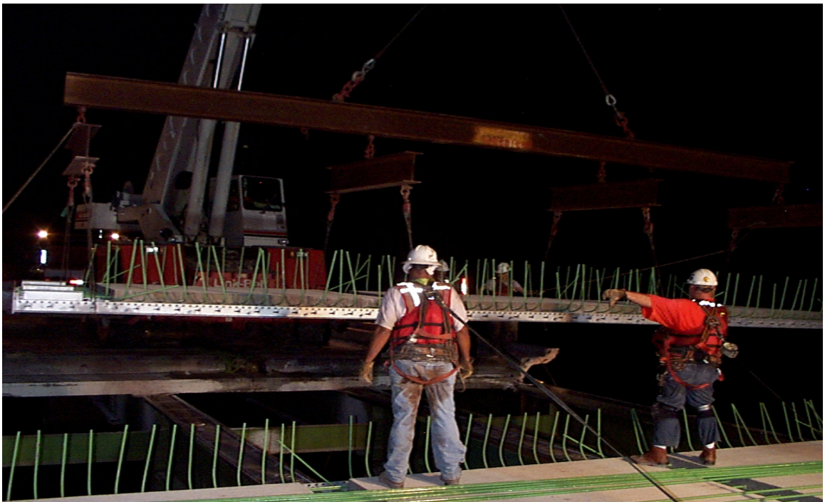
Fig. 4.11 Placement of Second Exodermic Panel
