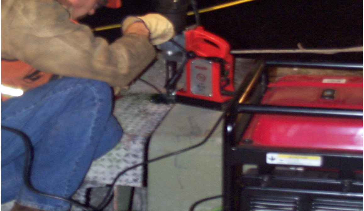
Fig 3.5 Drilling of Weld Plugs for Curb Plate Removal
