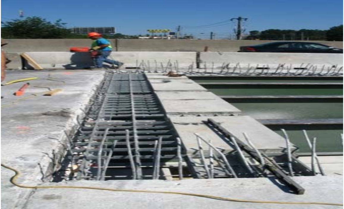
Fig. 5.30 First Exodermic Panel In-Place
