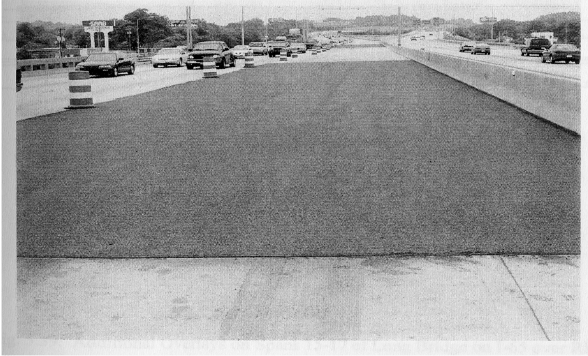
Fig. 2.28 Finished 3/8" Thick Polymer Concrete Overlay (4)
