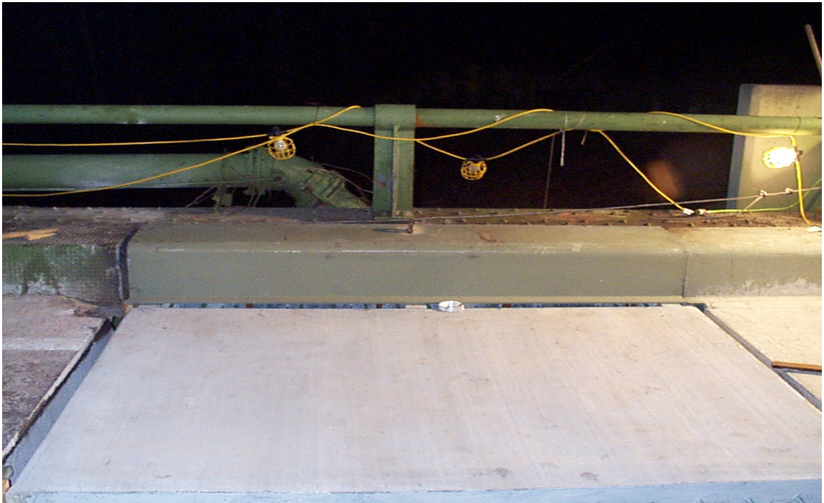
Fig. 3.26 New Curb Plate Set In-Place
