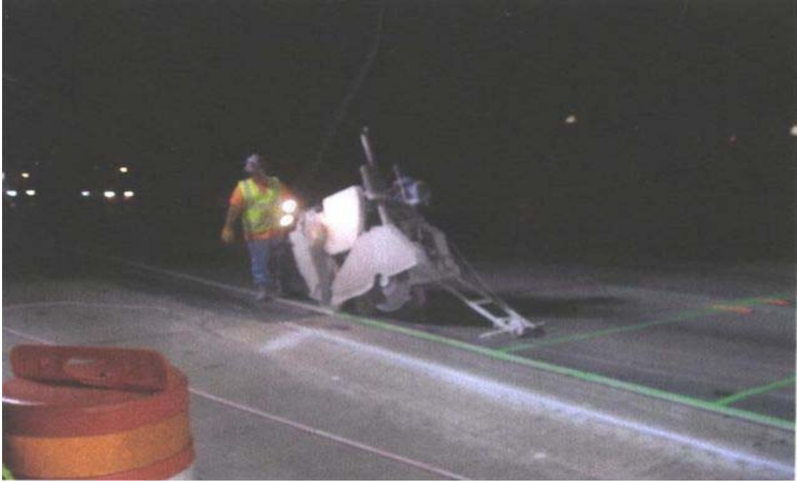
Fig. 5.6 Saw Cutting for Deck Removal
