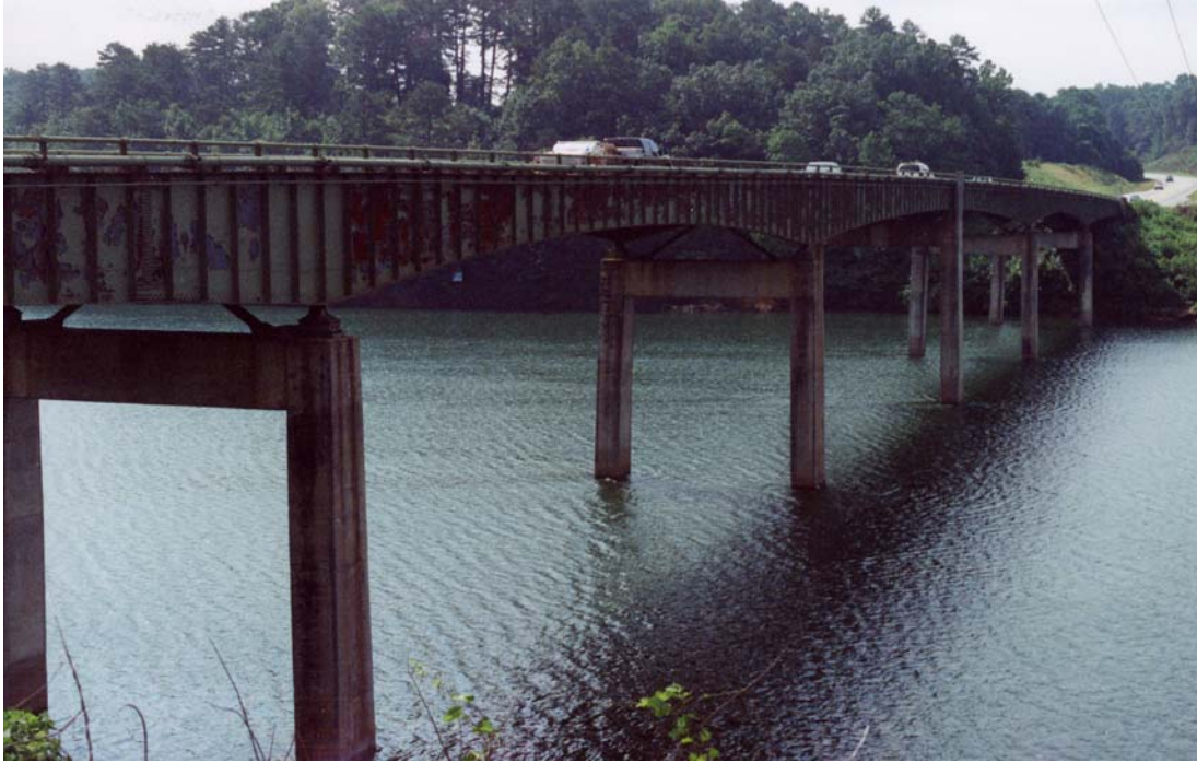
Fig. 2.4 Angled Side Elevation View of Longstreet Bridge (2)
