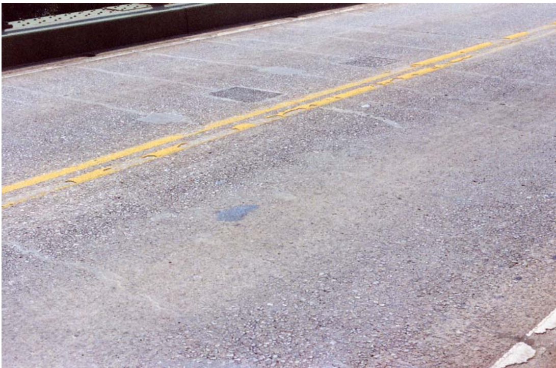
Fig. 2.7 Longstreet Bridge Deck (2)
