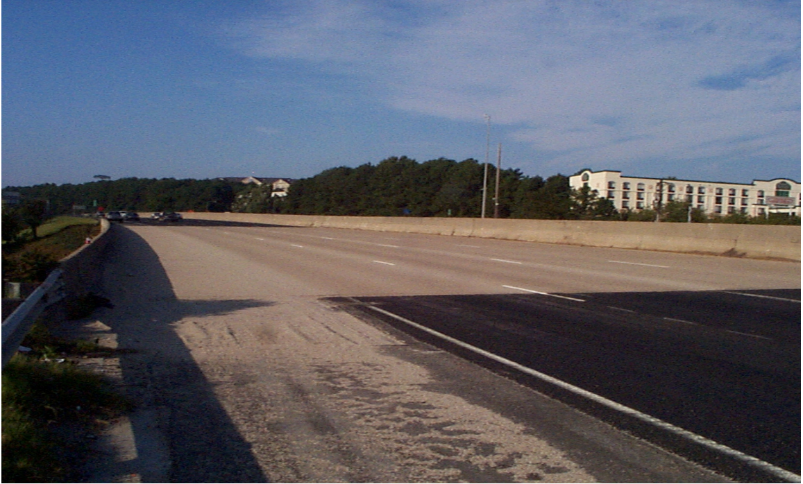
Fig. 5.64 Finished \frac{3}{8} " Thick Flexogrid Overlay
