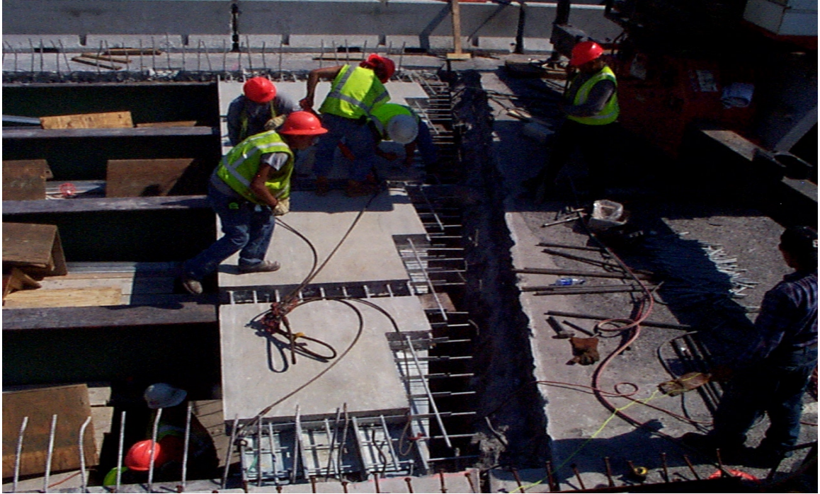
Fig. 6.14 Setting of First Precast Exodermic Panel
