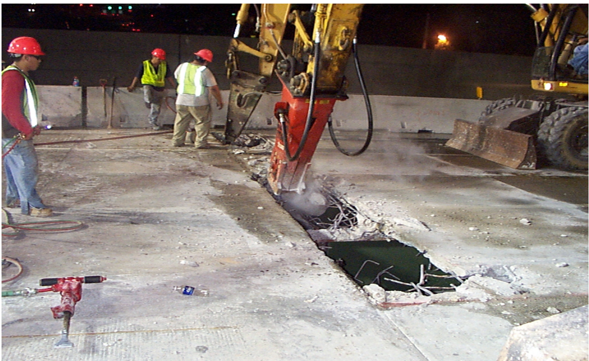
Fig. 5.11 Removal of Edge Beam
