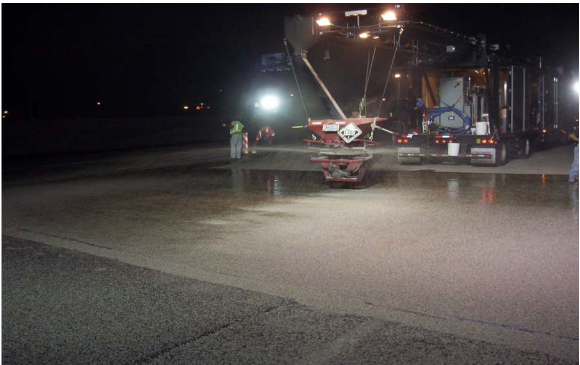
Fig. 5.59 Broadcasting of Second Layer of Aggregate on Polymer Binder
