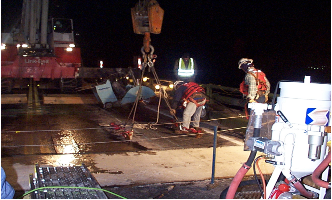
Fig. 7.12 Crane with Lifting Apparatus
