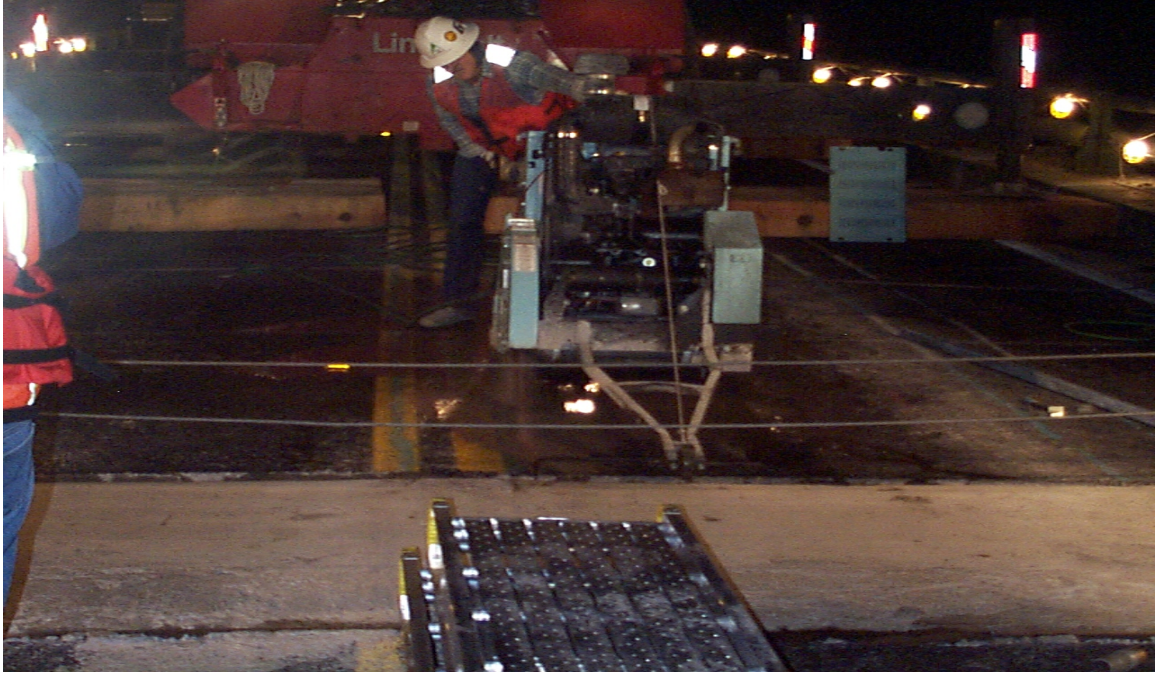
Fig. 3.7 Longitudinal Saw Cutting for Deck Removal
