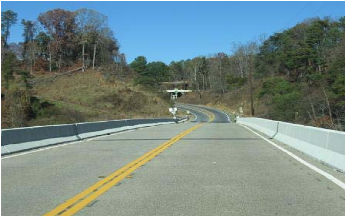
Fig. 4.27 Finished 3/8" Thick Flexgrid Overlay With Precast Jersey Barriers
