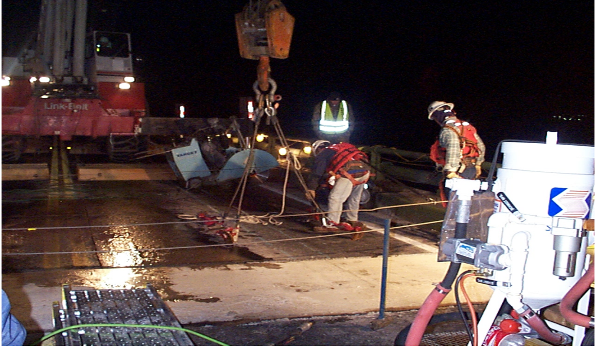
Fig 3.9 Preparing to Lift Out First Section of Existing Deck
