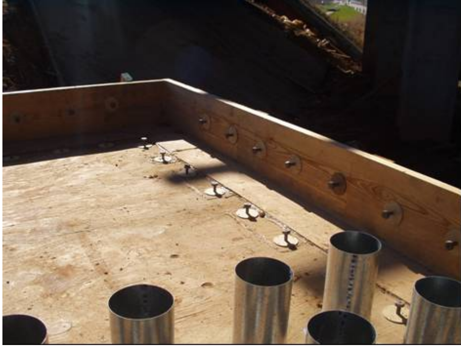
Figure C-100: Side and bottom pullout inserts
