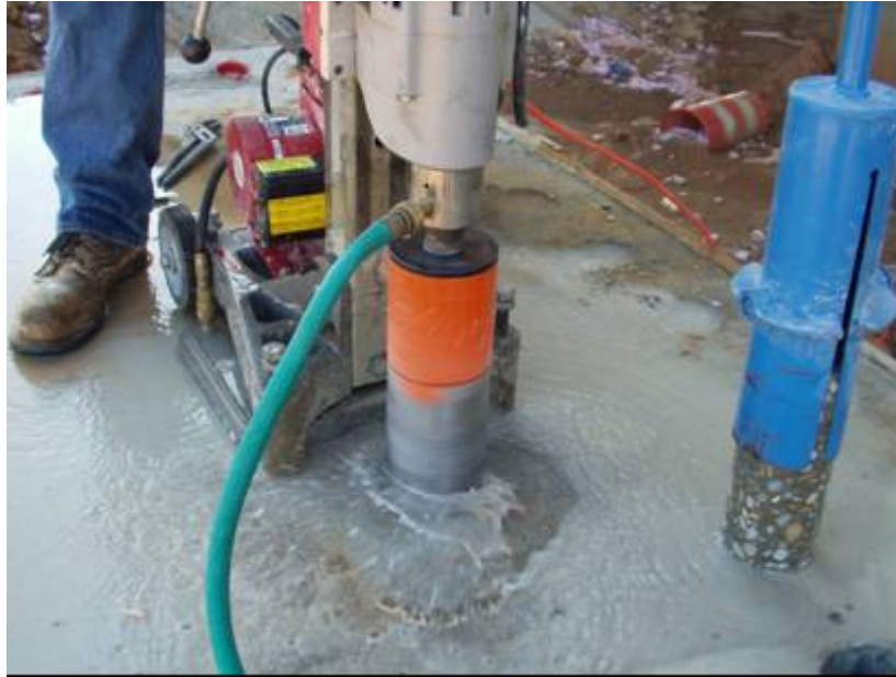
Figure C-110: Coring mock bridge deck
