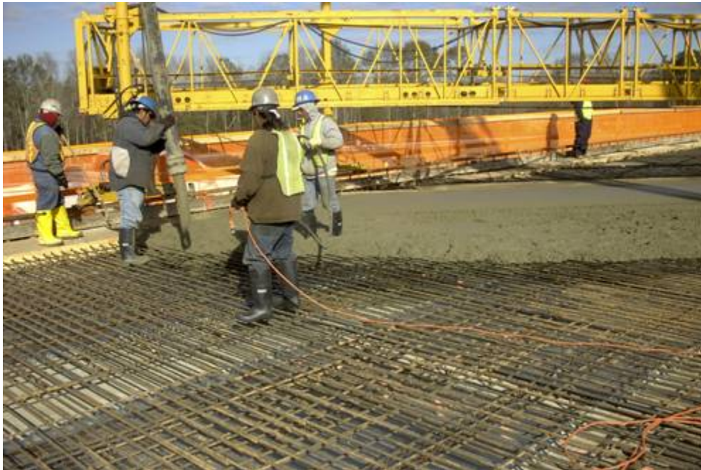
Figure C-126: Placing concrete in Pour 1 of I-85 Bridge deck
