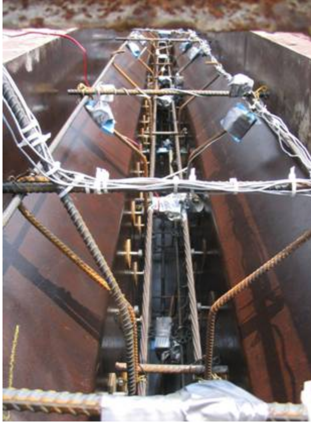
Figure B-72: Inside of flange of girder form before concrete cast
