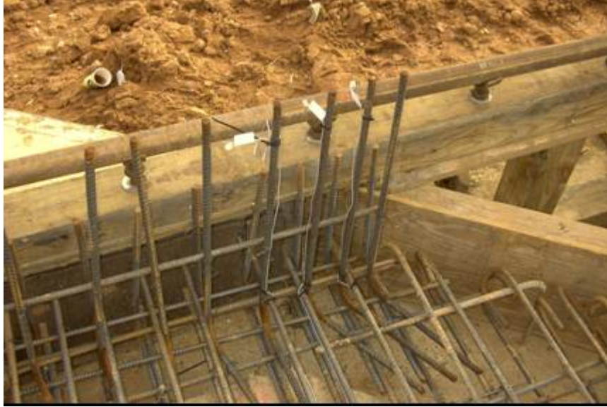
Figure C-123: iButton wire with phone jack secured to the barrier wall reinforcement
