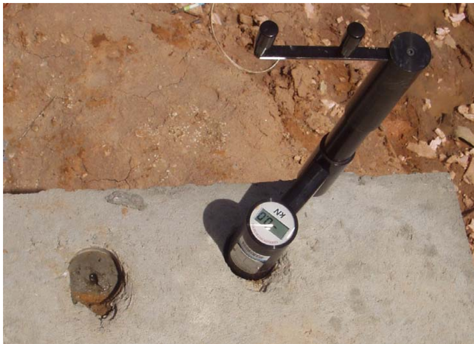
Figure 2-22: Pullout test equipment
