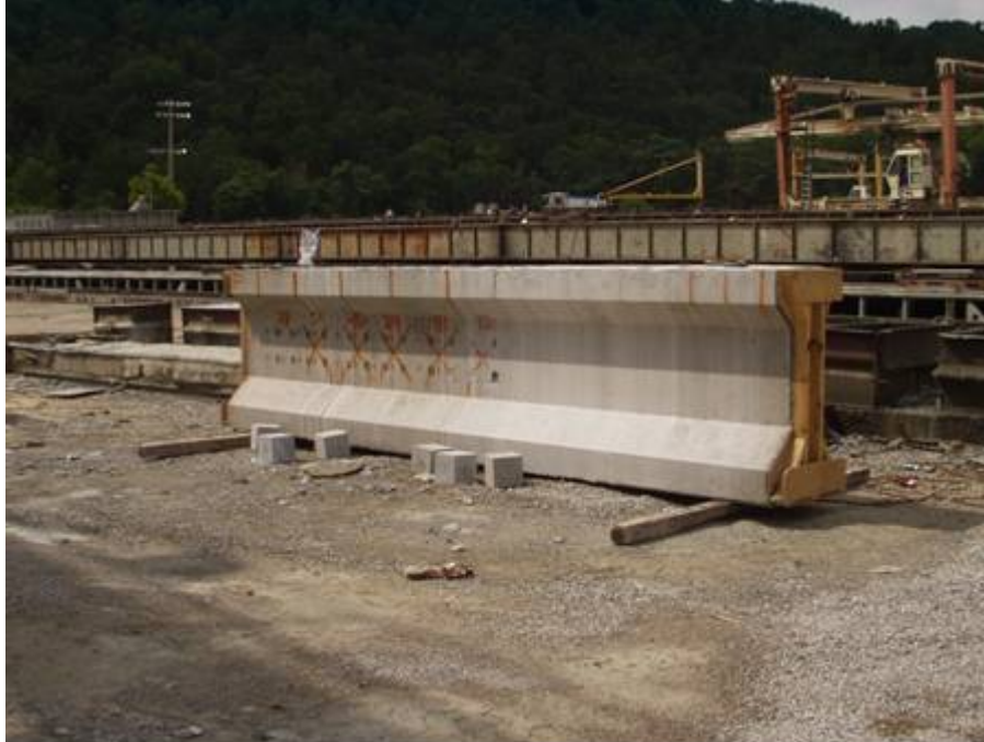
Figure B-92: Girder final storage area in stock yard
