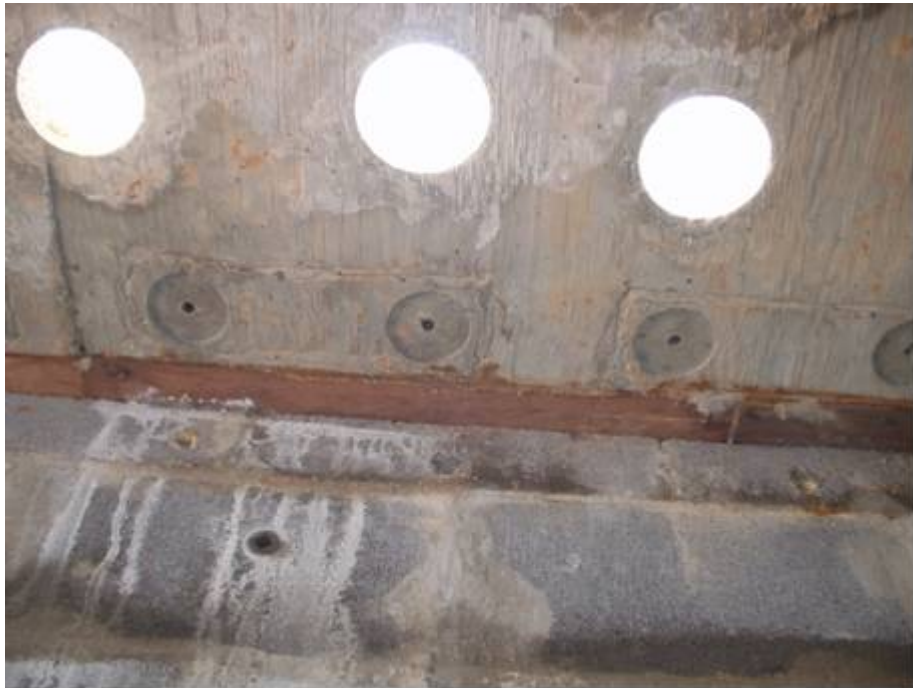
Figure C-115: Bottom pullout inserts for mock bridge deck (2)
