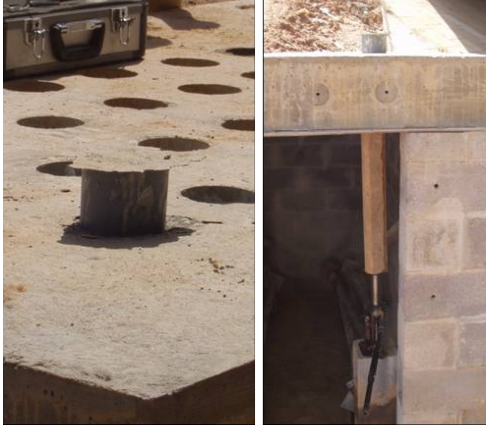
Figure 5-18: Removal of the cast-in-place cylinders
