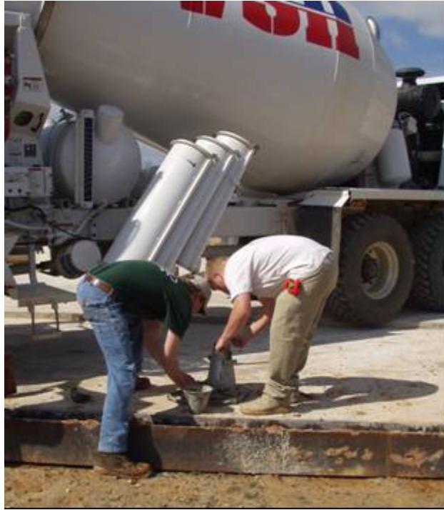
Figure C-104: Sam Wade conducting slump test
