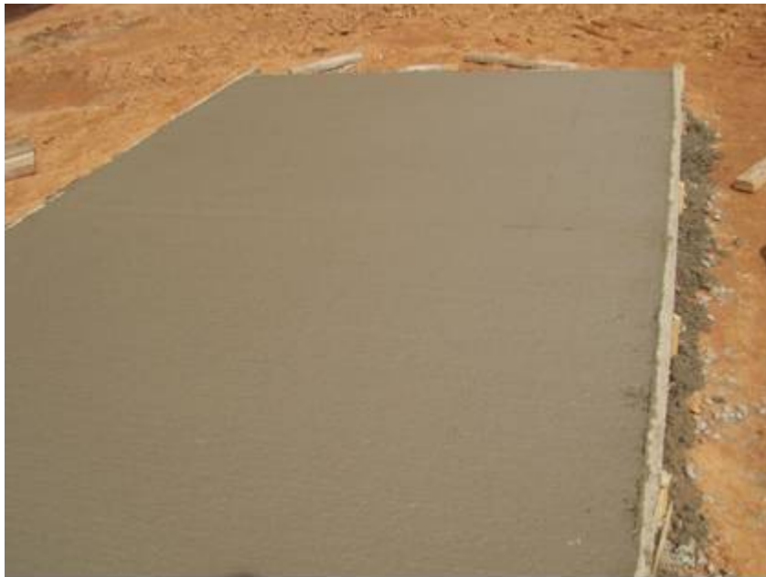
Figure C-95: Mock bridge deck base slab
