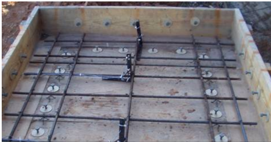
Figure 5-14: Reinforcement and pullout inserts
