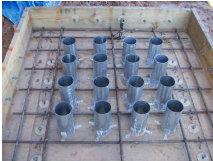
Figure 5-16: Cast-in-place cylinders installed in the mock bridge deck
