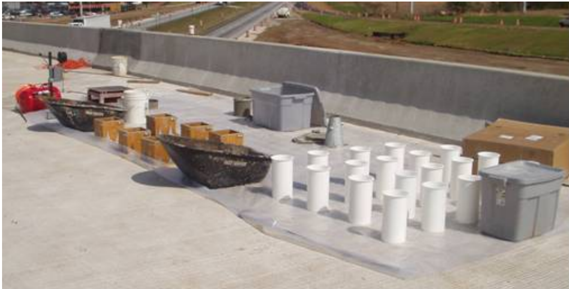
Figure 5-9: Casting of concrete specimens
