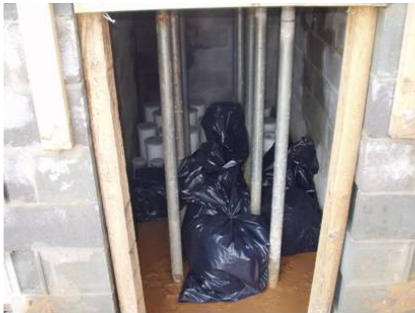
Figure C-109: Field-cured specimens storage area for the first 24 hours
