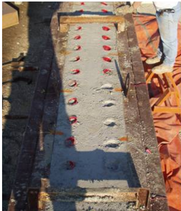
Figure B-81: Top of girder with floating inserts
