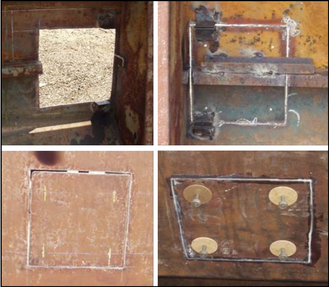
Figure 4-22: Access panels in mock girder forms
