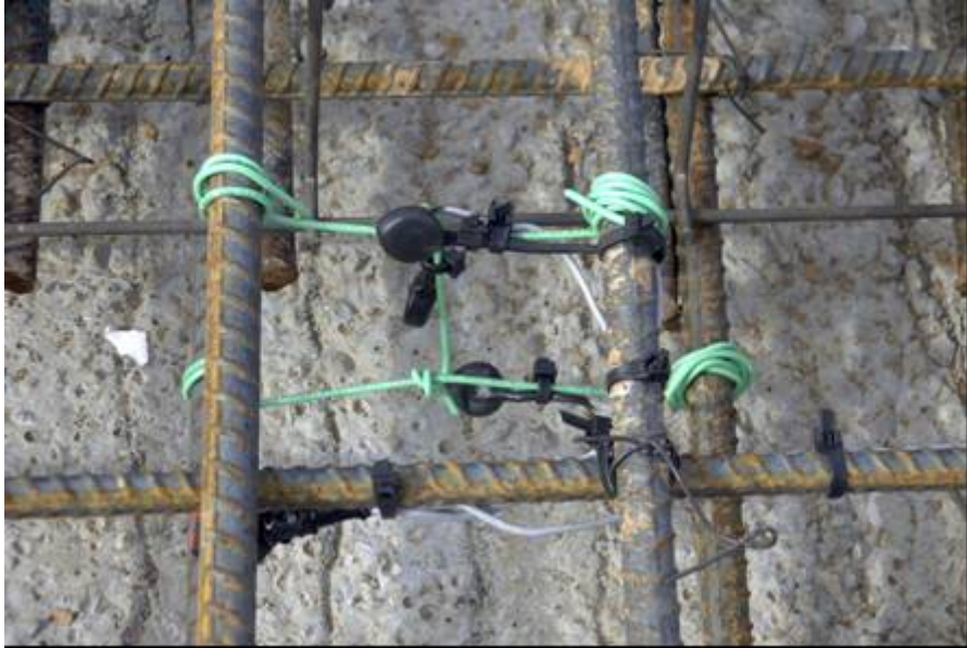
Figure C-117: iButtons suspended between reinforcement
