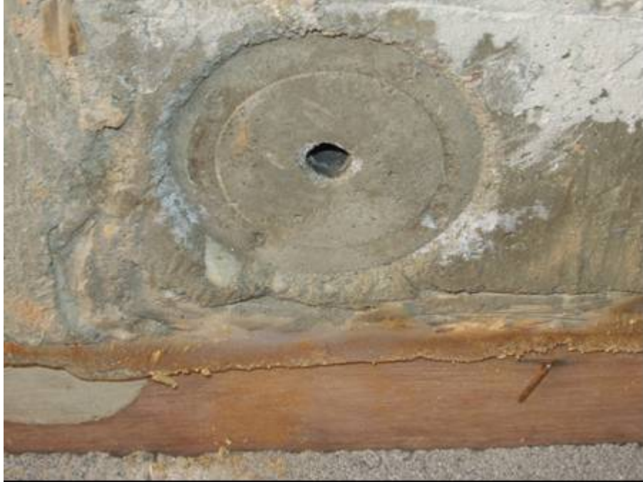
Figure C-114: Bottom pullout inserts for mock bridge deck
