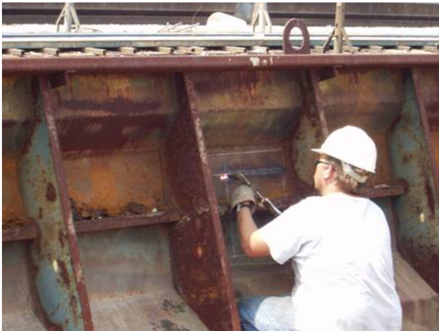
Figure B-65: Sherman prestress medal worker cutting access panel
