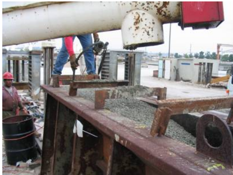
Figure B-77: Fresh concrete placement
