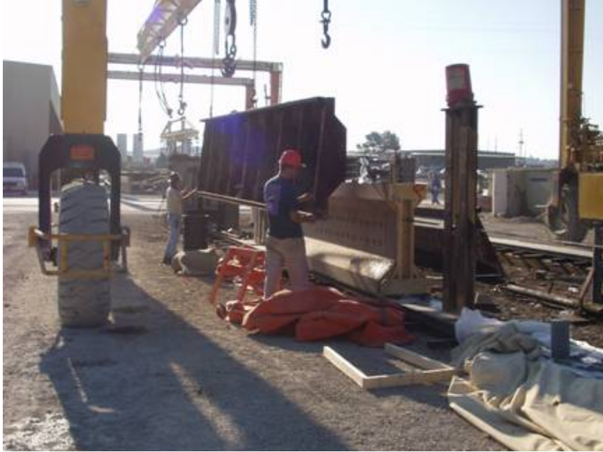
Figure B-82: Removal of girder forms
