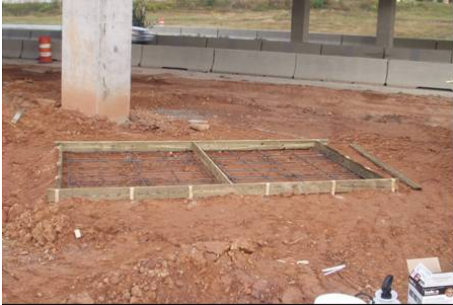
Figure C-94: Mock bridge deck base slab reinforcement
