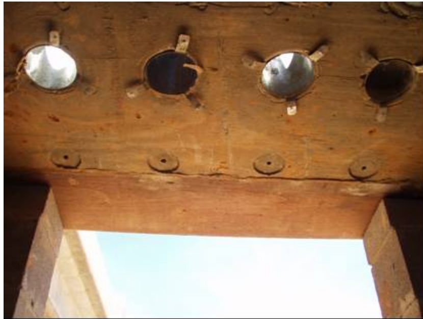
Figure C-113: Bottom pullout inserts and cast-in-place cylinder for mock bridge deck
