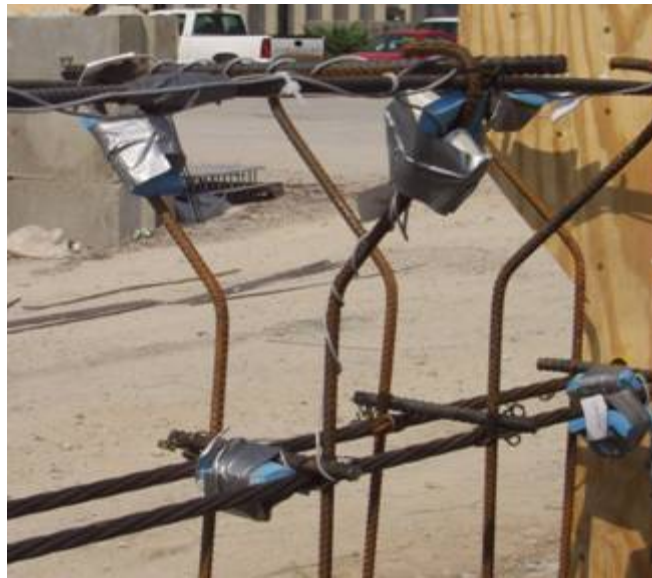
Figure B-63: iButton installation (2)
