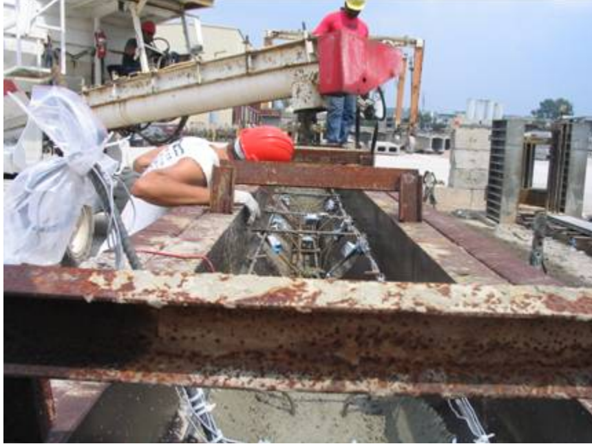
Figure B-76: Concrete transport placing concrete
