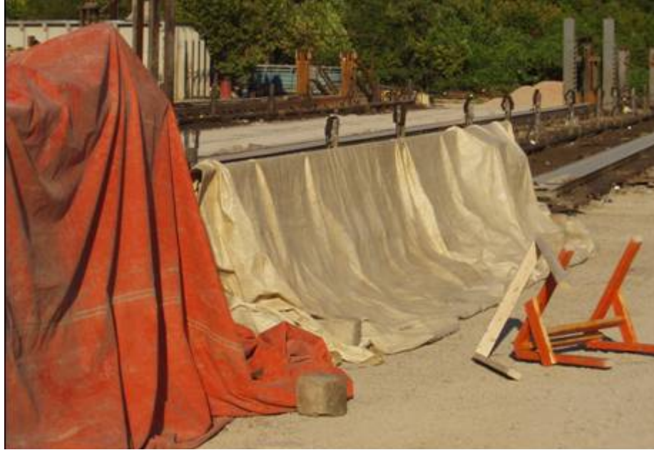
Figure B-80: Curing blanket covering the concrete specimens
