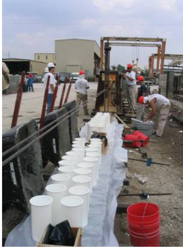
Figure B-74: Fresh concrete work area
