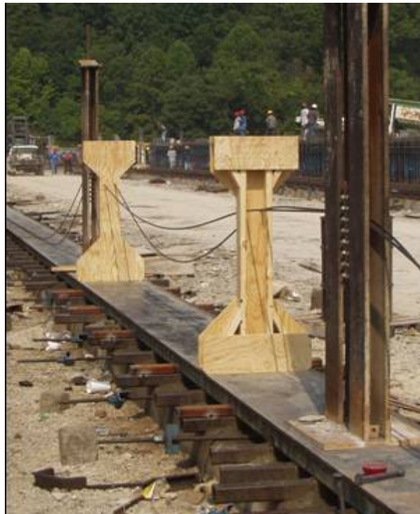
Figure B-59: Prestressed strand being installed
