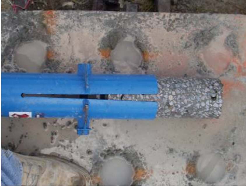
Figure B-88: Core removal process
