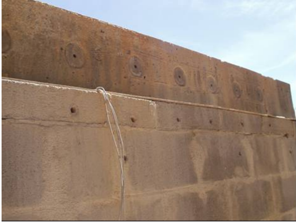
Figure C-116: Side pullout test for mock bridge deck
