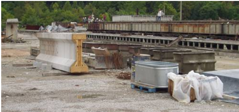
Figure B-93: Girder and field curing tank in stock yard
