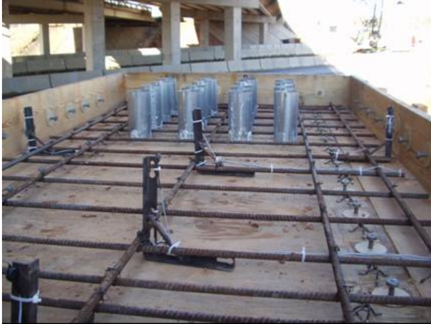
Figure C-102: Mock bridge deck in-place testing and iButtons
