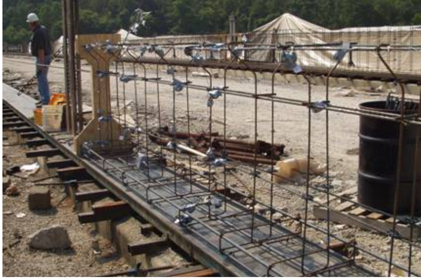
Figure B-64: iButton installation (3)
