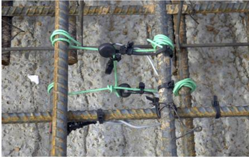
Figure 5-19: iButtons installed in the bridge decks
