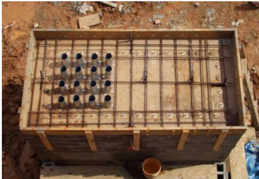
Figure C-97: Mock bridge deck in-place testing and reinforcement
