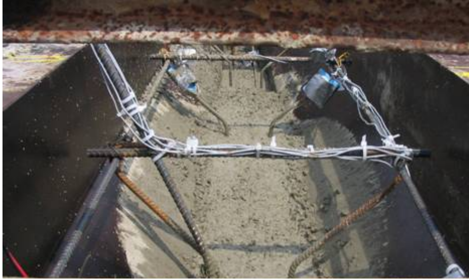
Figure B-78: Fresh concrete being placed in flange
