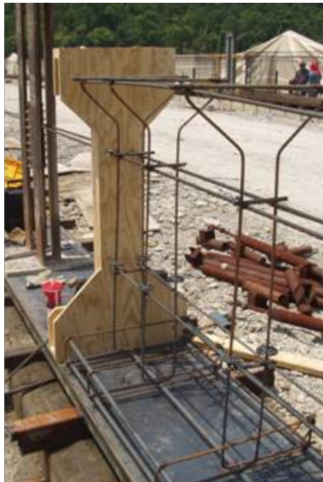
Figure B-61: Steel reinforcement cage (2)
