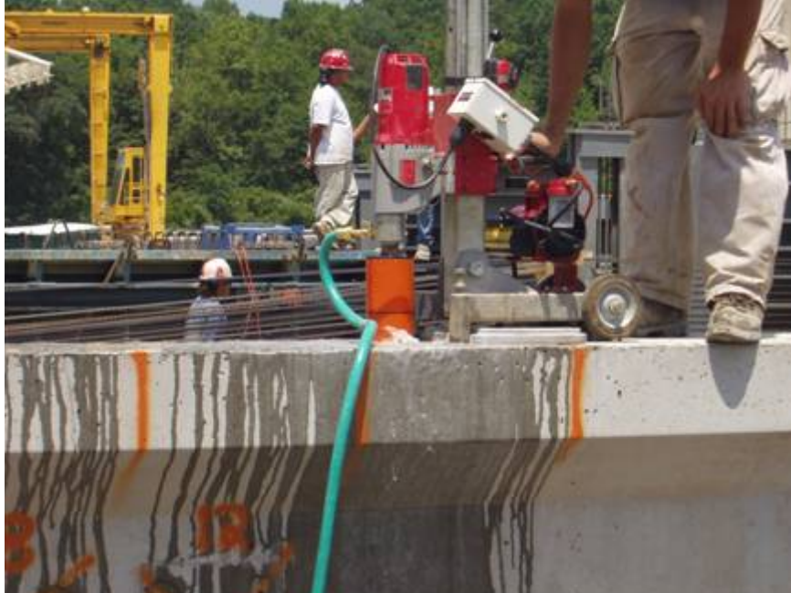
Figure B-86: Coring process (1)
