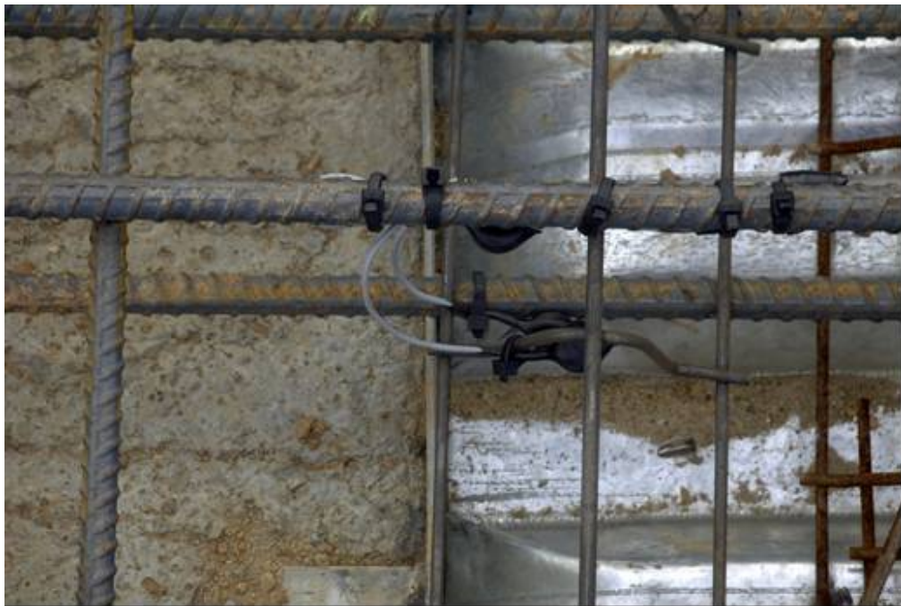
Figure C-120: iButtons attached to reinforcement
