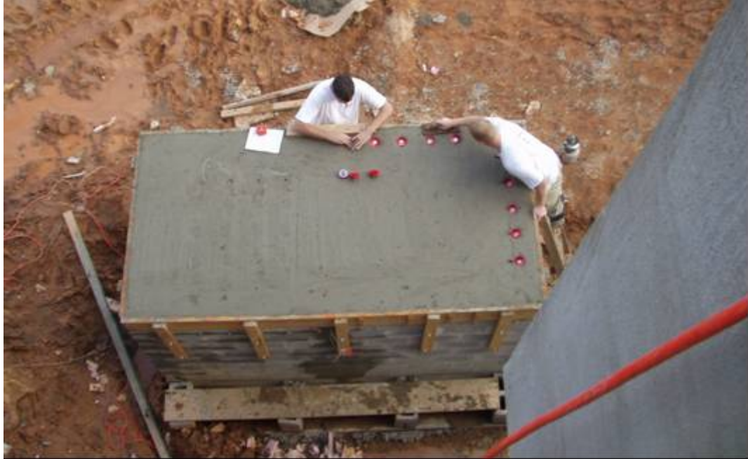
Figure C-106: Installing top pullout inserts
