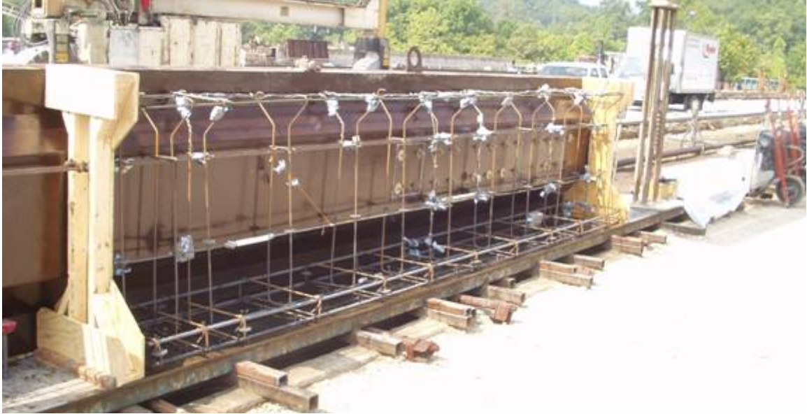
Figure B-70: Girder forms and steel cage
