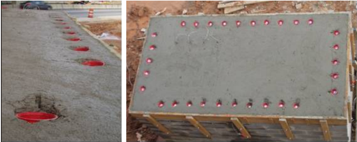
Figure 5-12: Top pullout inserts for the mock bridge deck
