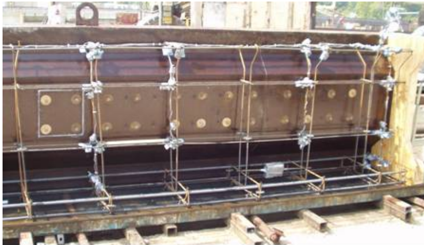
Figure 4-21: Mock girder form with pullout inserts and stirrups
