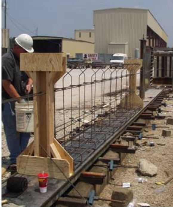
Figure B-60: Steel reinforcement cage (1)
