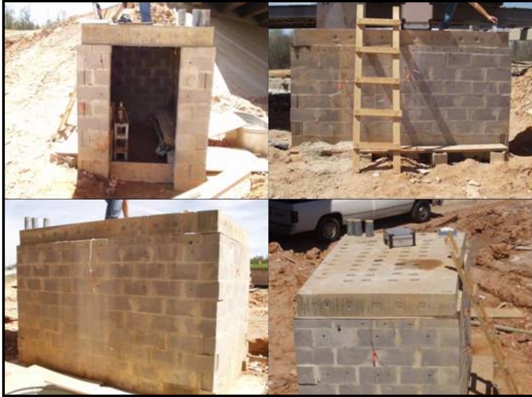
Figure 5-5: Mock bridge deck structure
