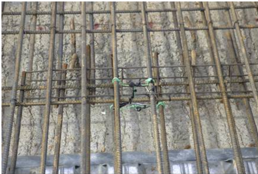
Figure C-118: iButtons suspended between reinforcement (2)
