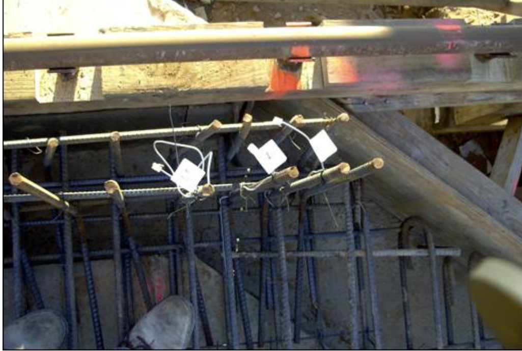
Figure C-125: iButton wire with phone jack secured to the barrier wall reinforcement (3)
