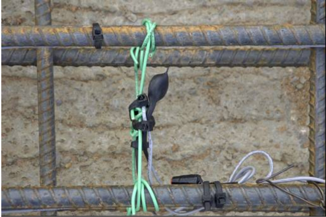
Figure C-119: iButtons suspended between reinforcement (3)
