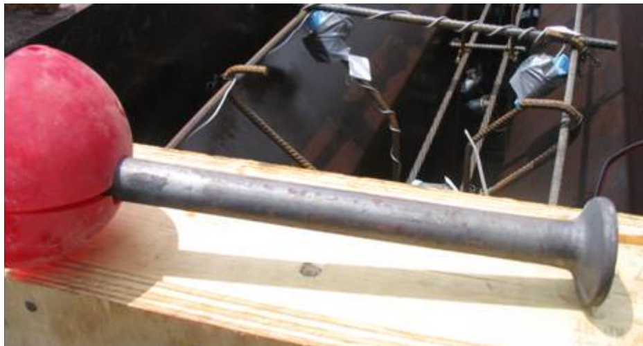
Figure B-73: Lifting anchor installed in mock girder
