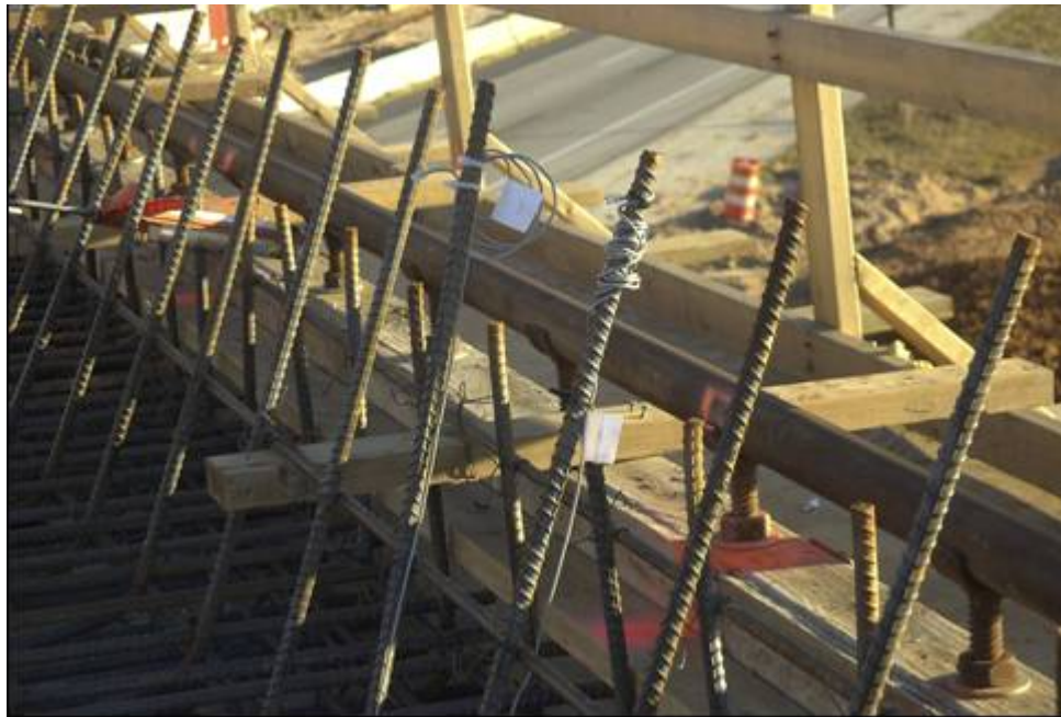
Figure C-124: iButton wire with phone jack secured to the barrier wall reinforcement (2)
