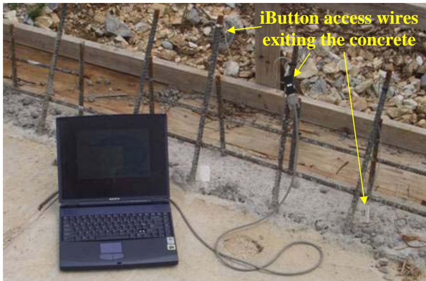
Figure 5-20: iButton wires exiting the concrete
