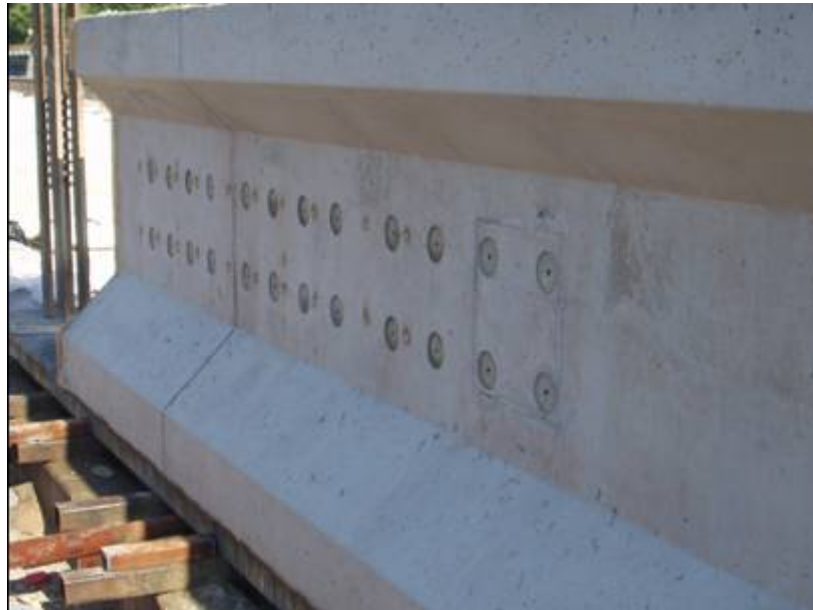
Figure B-83: Side insert after girder forms removed
