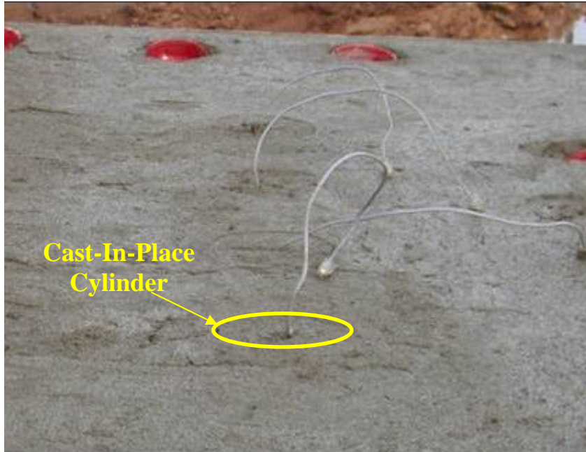
Figure 5-11: iButtons embedded in the cast-in-place cylinders
