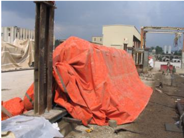
Figure B-79: Curing tarp over mock girder
