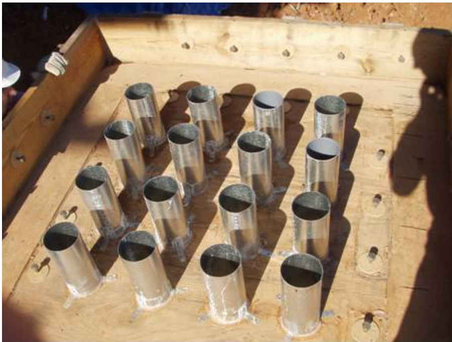
Figure C-99: Cast-in-place cylinders and pullout inserts (2)
