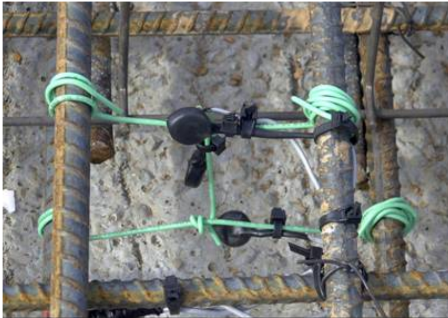
Figure 6-4: Suspending the maturity recording device between reinforcement bars
