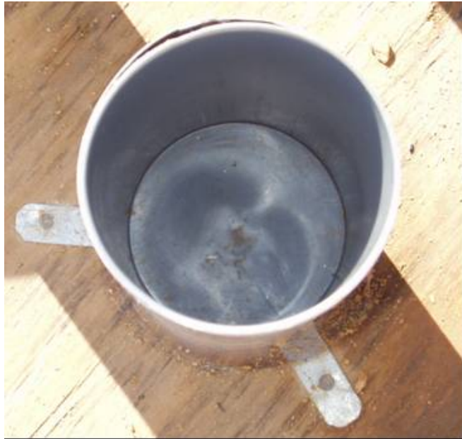
Figure C-101: Cast-in-place cylinder with 4 x 8 plastic mold
