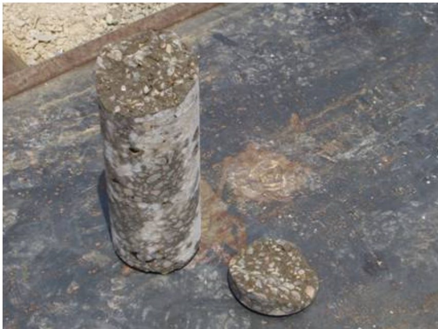
Figure B-89: Core right after removal from girder
