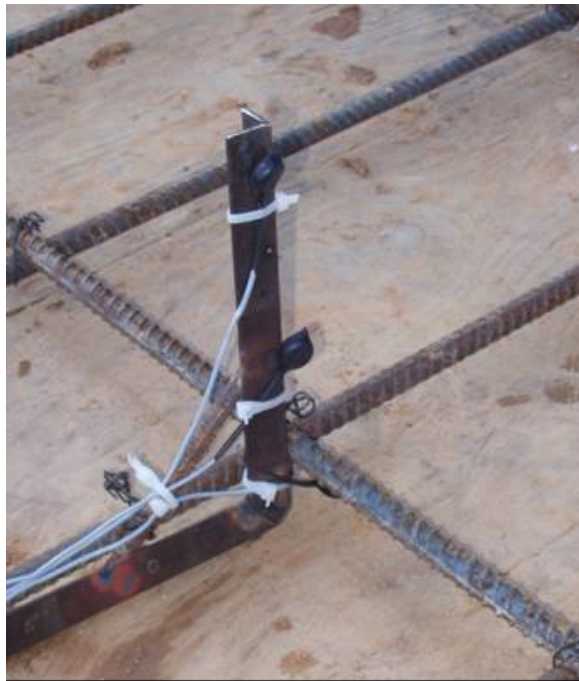
Figure C-103: iButton stands to measure concrete temperatures
