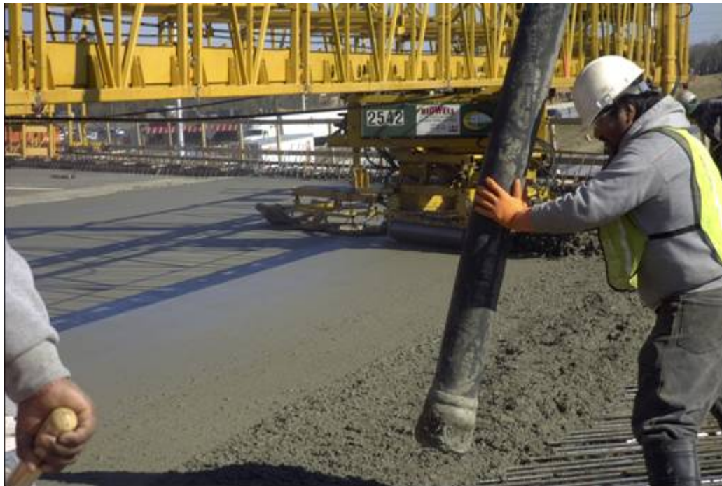
Figure C-128: Placing concrete in Pour 1 of I-85 Bridge deck (3)
