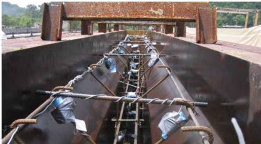
Figure B-71: Stirrups, iButtons and girder forms before concrete cast
