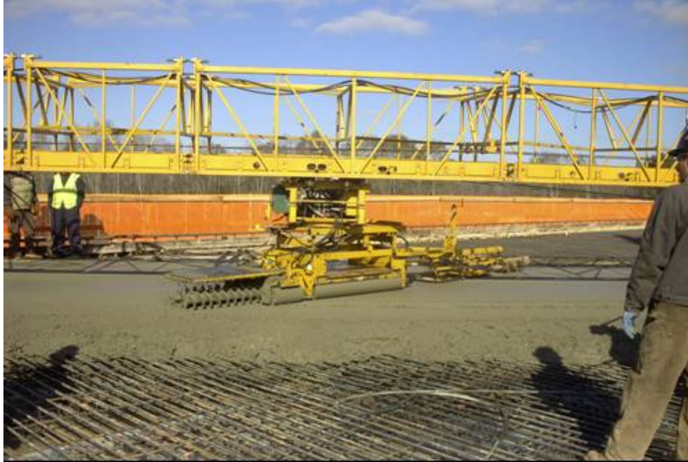
Figure C-127: Placing concrete in Pour 1 of I-85 Bridge deck (2)
