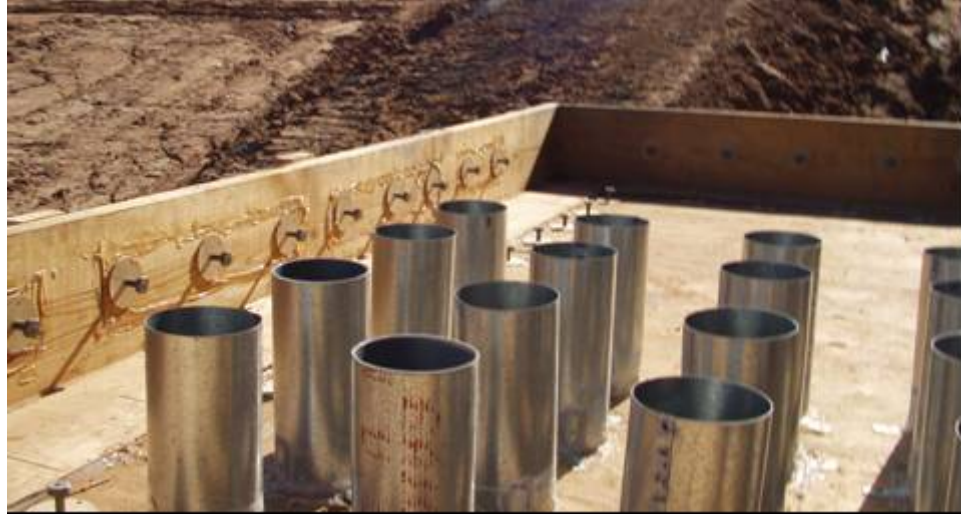
Figure C-98: Cast-in-place cylinders and pullout inserts
