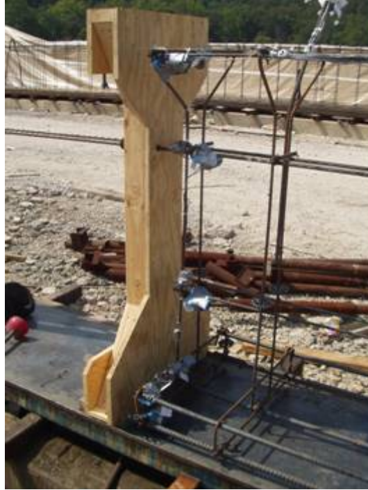
Figure B-62: iButton installation (1)
