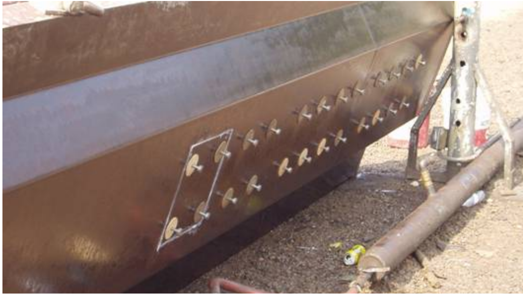
Figure B-69: Side mounted inserts
