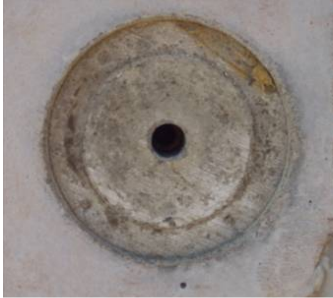
Figure B-84: Side pullout inserts
