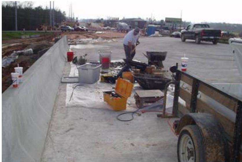
Figure C-105: Fresh concrete testing area
