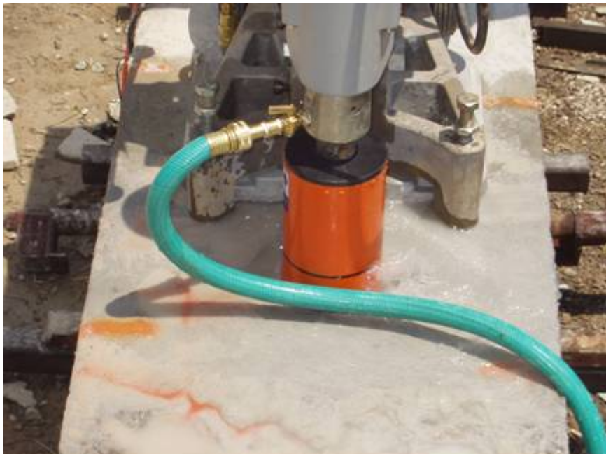
Figure B-87: Coring process (2)
