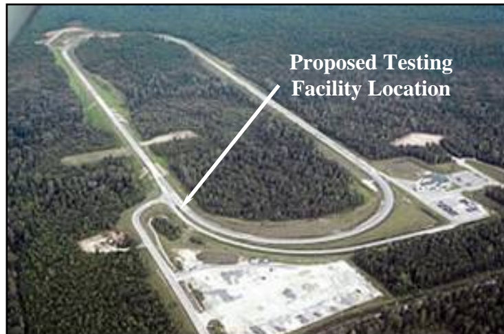
Figure 7.1 NCAT Test Facility.
