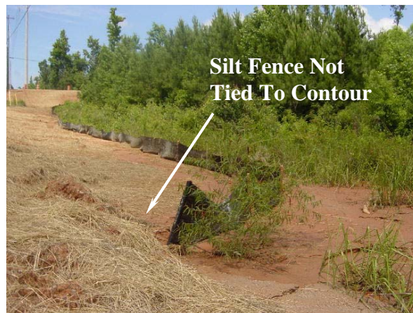
Figure 3.3 Failure Mode: Tie to the Contour.
