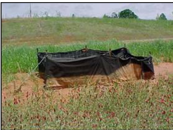
c. Inlet Protection
