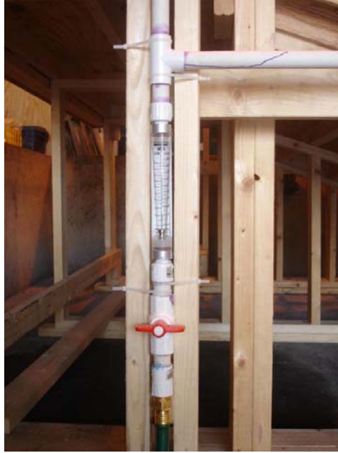
Figure 4.14 Rainfall Simulator Connection, Gate Valve, and Flowmeter.
