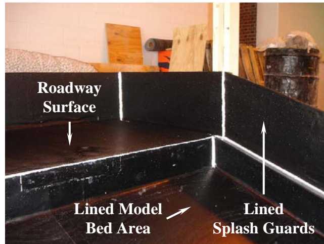
Figure 4.10 Roadway Surface, Waterproofing, and Sealing.
