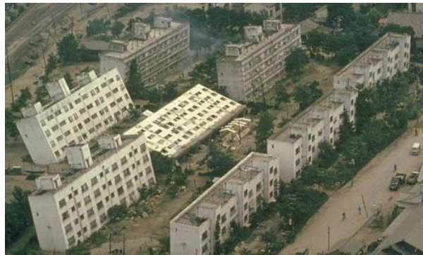
Figure 1.2: Effects of earthquake liquefaction in Niigata, Japan, 1964
