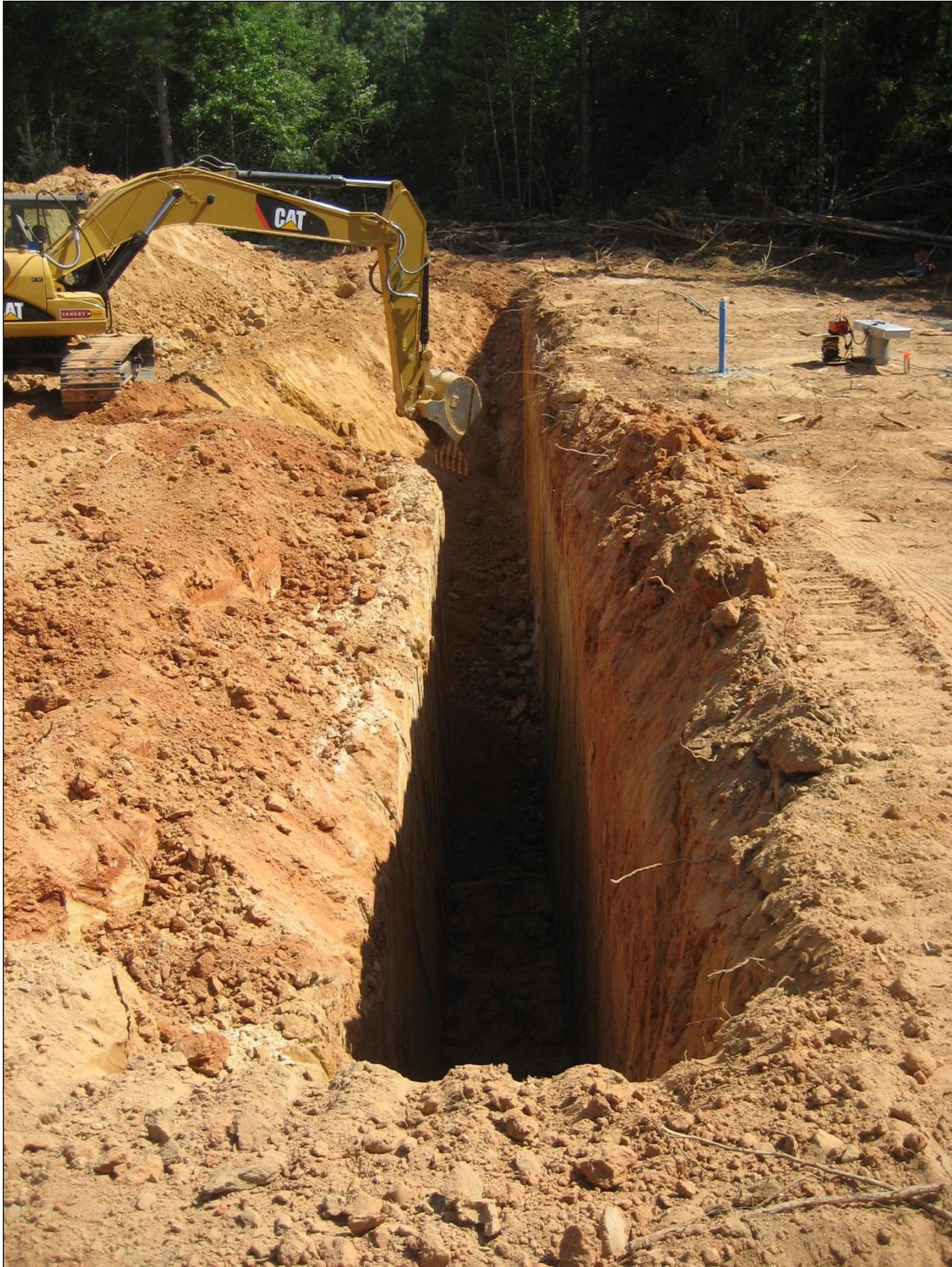
Figure 57 – Material being removed from non-instrumented side of Excavation #2.
