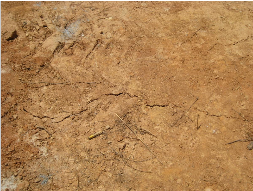
Figure 61 – Tension cracks developed during Excavation #2.
