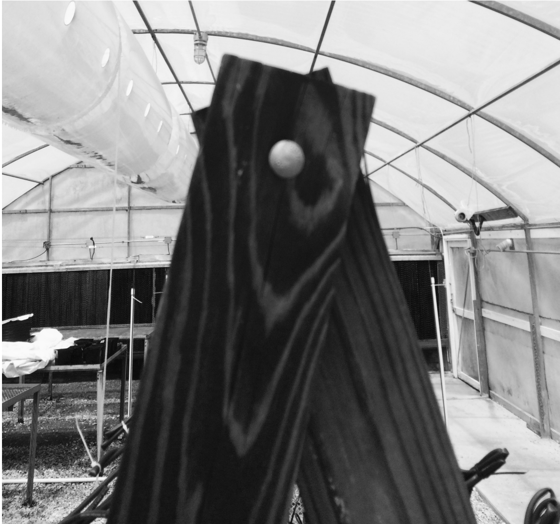
Figure 4.3. Two treated wood boards measuring 2" x 4" x 7' are connected with two, 3/8 inch x 3 inch galvanized steel carriage bolts, 5/16 inch galvanized steel hex nuts, and 5/16 inch galvanized steel washers. This image shows the top of one leg of the A-frame vertical structure connected with one bolt, nut, and washer. Each leg of the structure requires two bolts, nuts, and washers.
