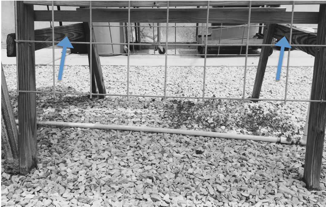
Figure 4.4. The 3-foot board is connected to the two legs, or 2" x 4" boards. The smaller board was connected to the legs of the structure with a total of four 3/8 inch x 3 inch galvanized steel carriage bolts, 5/16 inch galvanized steel hex nuts, and 5/16 inch galvanized steel washers. Once the 3' boards are attached to both legs, the structure occupies 16 ft 2 of production space.
