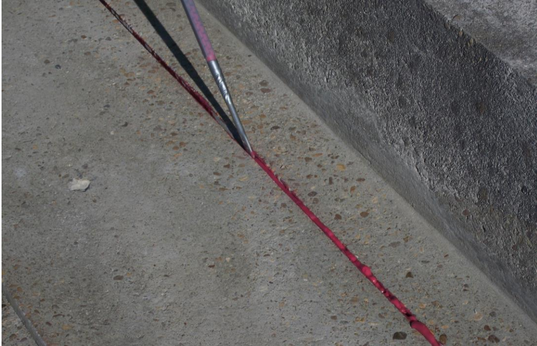
Figure 4.31 Epoxy Injection after Properly Seating FRP Strip
