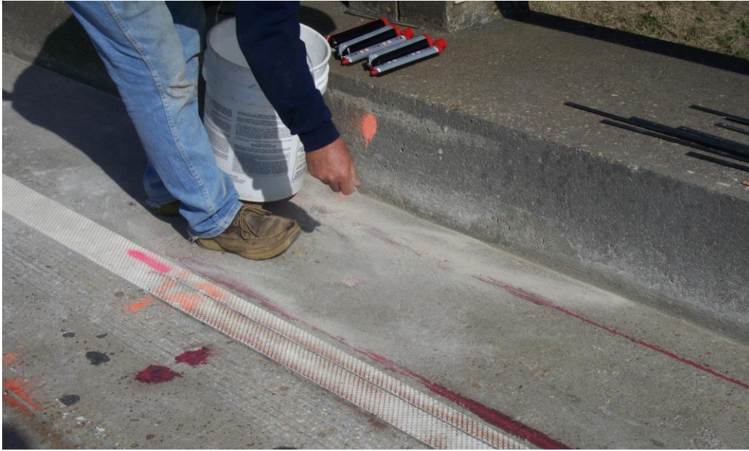
Figure 4.33 Sand Spread on Finished Epoxy to Provide Traction
