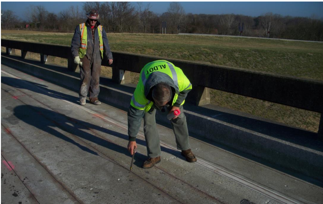
Figure 4.24 ALDOT Inspector Checking Groove Depth
