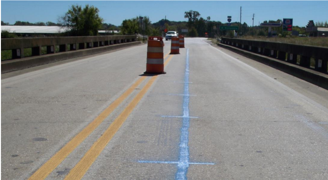
Figure 5.16 Load Truck Guideline Striping on Bridge Deck
