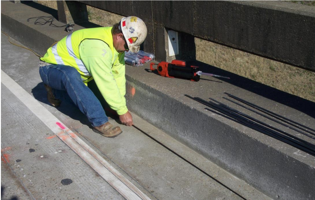
Figure 4.29 FRP Strip Placement within Epoxy Injected Groove
