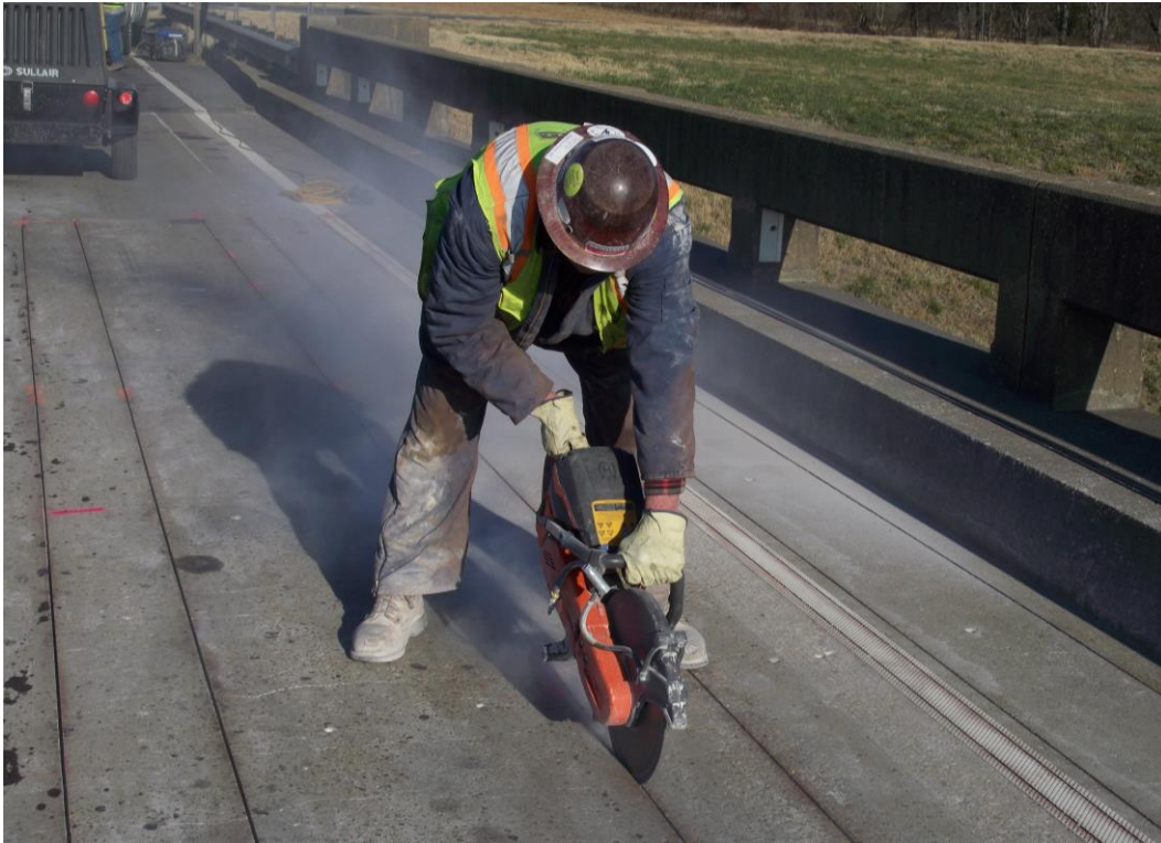
Figure 4.25 Shallow Locations Fixed by Handheld Concrete Saw
