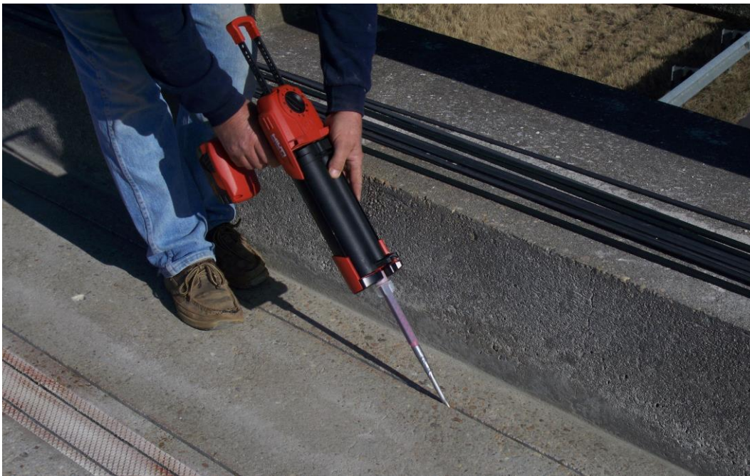
Figure 4.28 Epoxy Injected into Bottom of Prepared Groove
