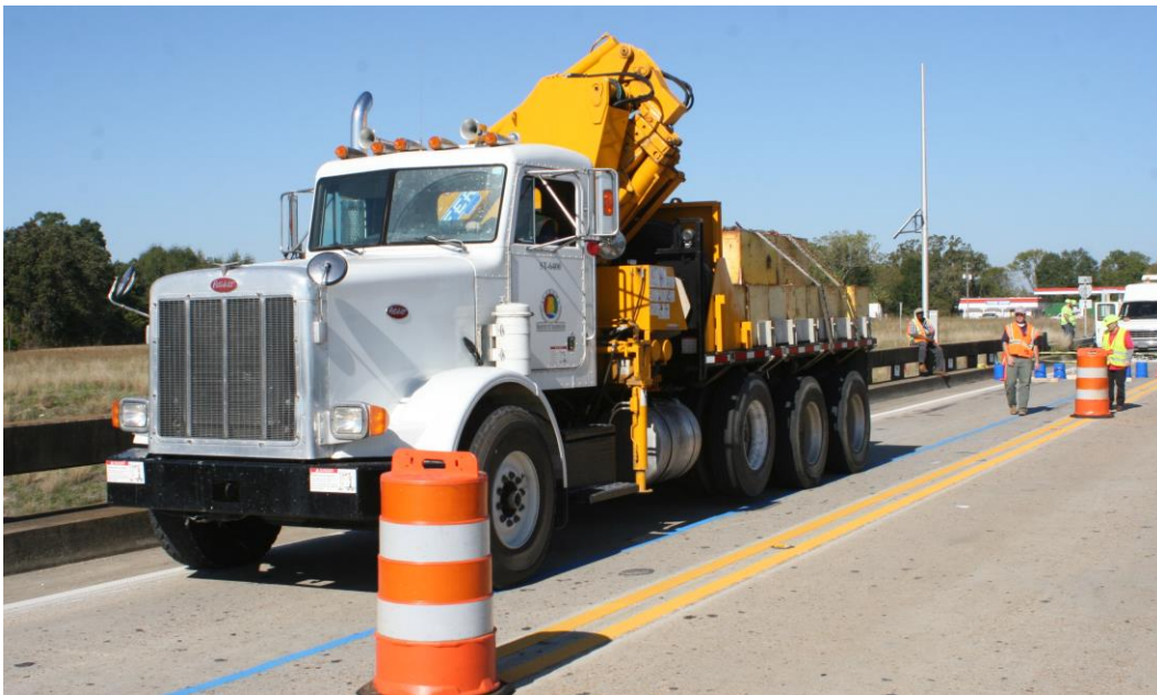
Figure 5.27 LC-4 Load Truck Backed into Position during Testing
