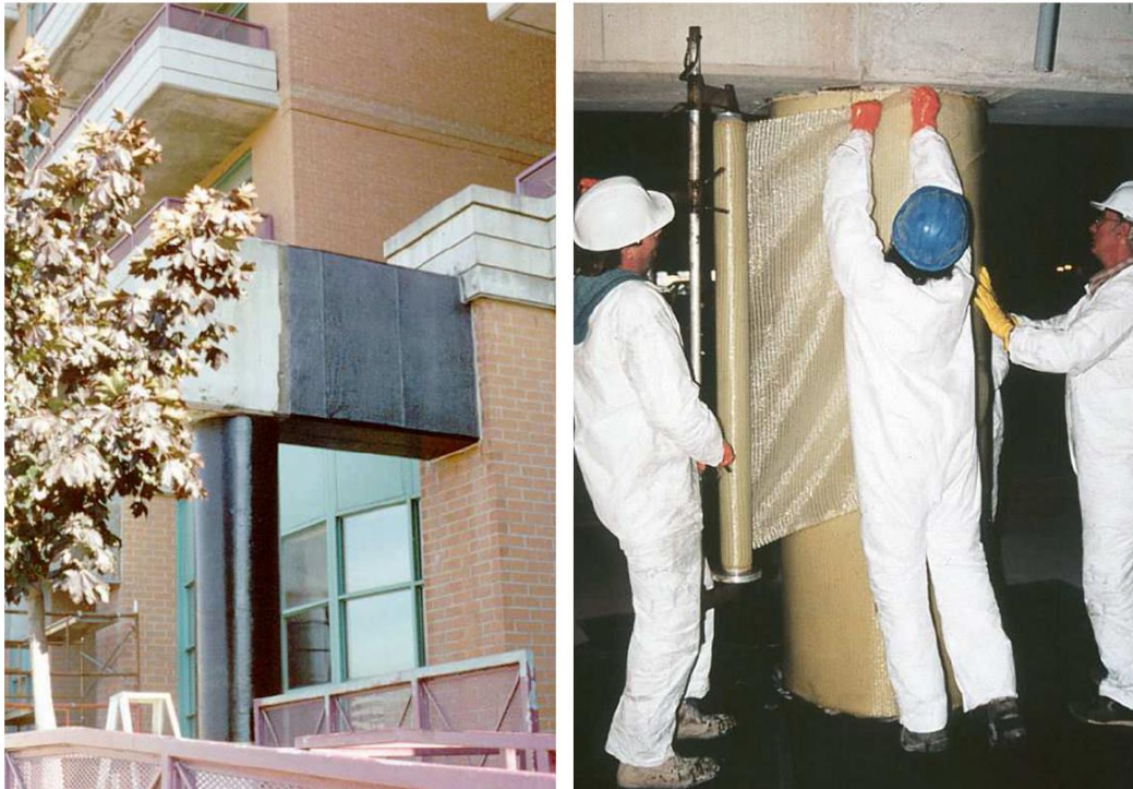
Figure 2.3 FRP Fabric Wraps of Beam (Left) and Column (Right) (Sheikh and Homam 2004)
