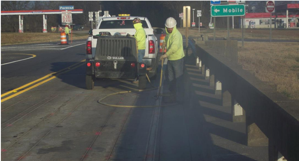
Figure 4.23 Cleaning Dry Grooves with Compressed Air
