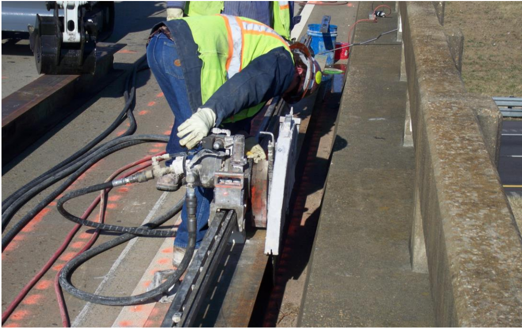
Figure 4.34 Attempted H-Pile Mounted Track Saw Setup
