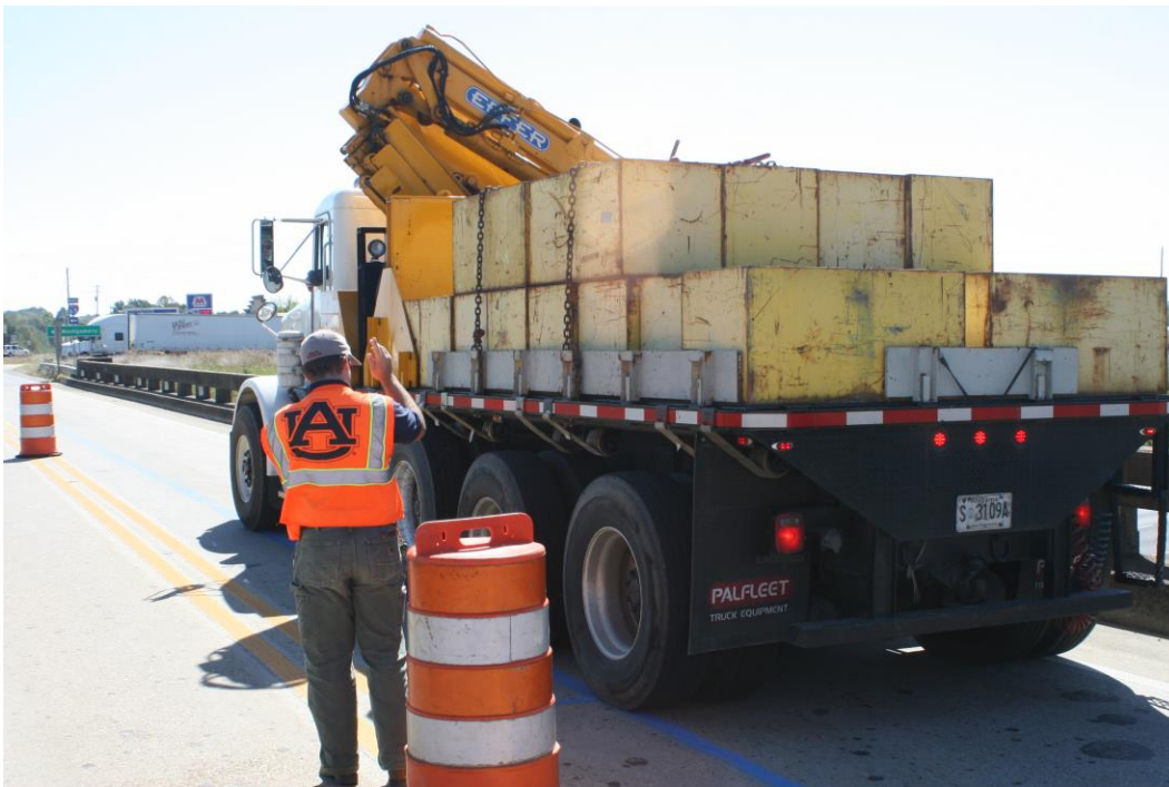
Figure 5.28 LC-5 Load Truck during Pre-Retrofit Load Test
