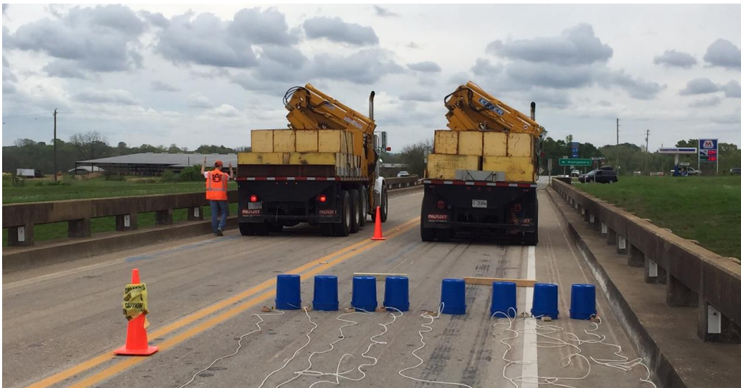
Figure 5.31 Load Test with Two Load Trucks
