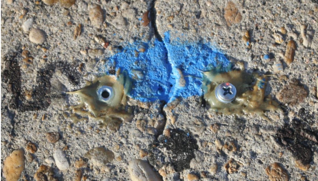
Figure 5.12 One Hex Nut Mount After Installation Bracket Removal (Left) and One Completed Mount Installation Capped with Washer and Screw (Right)
