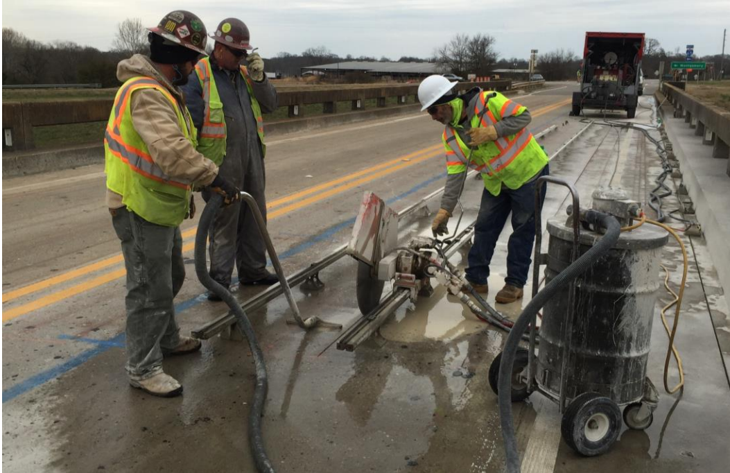
Figure 4.21 Vacuuming Slurry behind Saw Cutting
