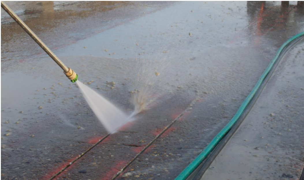
Figure 4.22 Groove Cleaning with Pressurized Water
