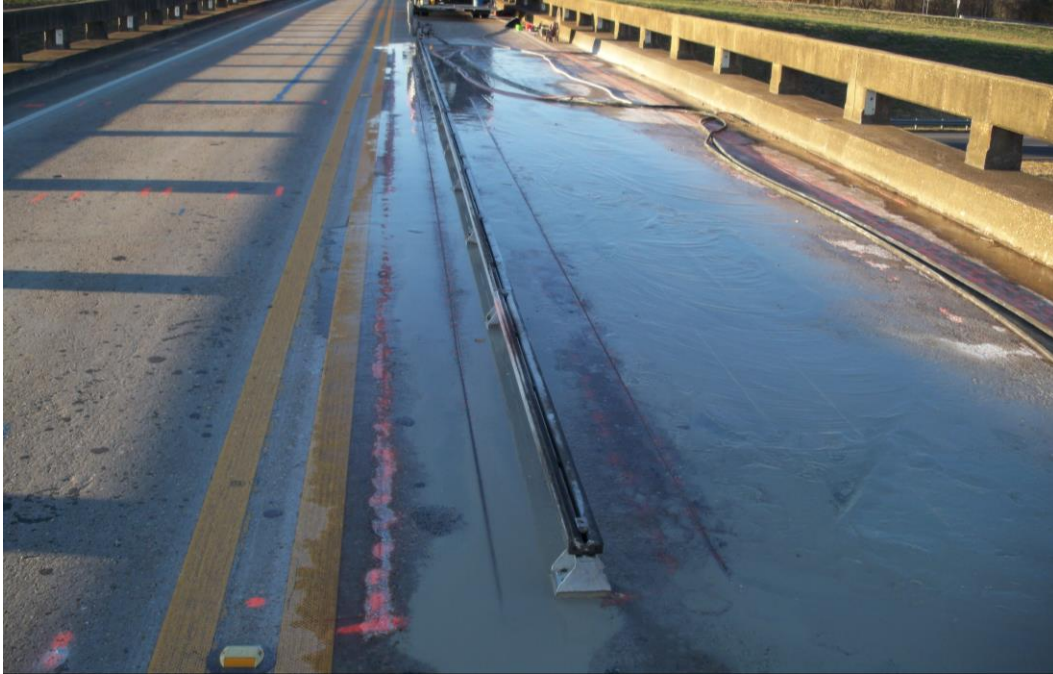
Figure 4.35 Slurry on Deck after One Day of Cutting
