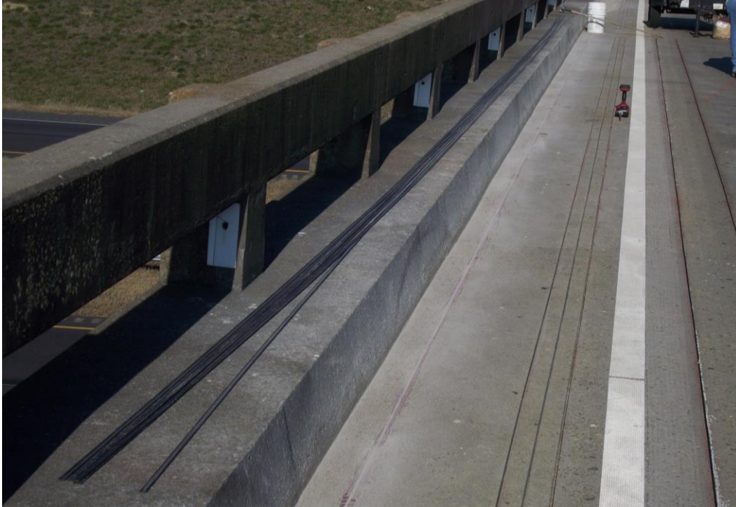
Figure 4.27 FRP Strips Cut and Ready for Placement
