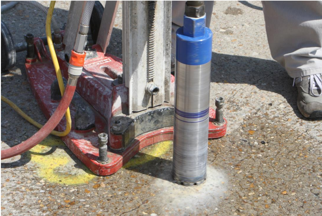
Figure 4.9 Coring of the Letohatchee Bridge
