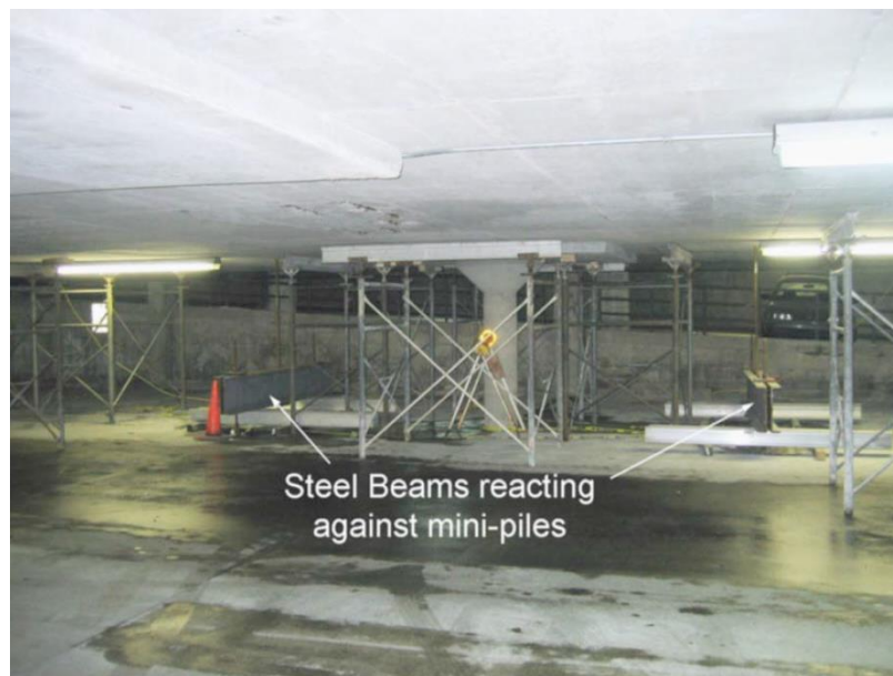
Figure 2.13 Reaction Beams on Mini-Piles to Load Decks Above (Tumialan, Vatovec, and Kelley 2007).
