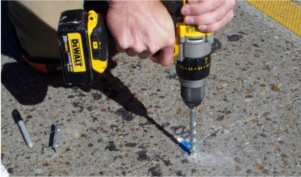
Figure 5.8 Drilled Holes for Transducer Mount Installation
