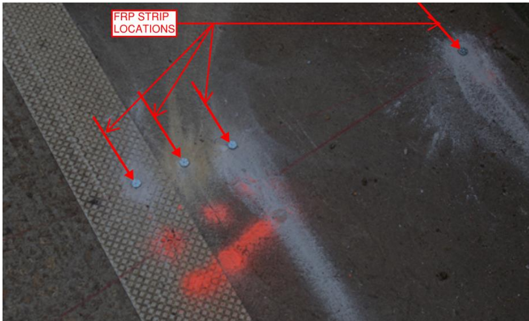
Figure 4.8 Mag Nails Marking FRP Strip Locations
