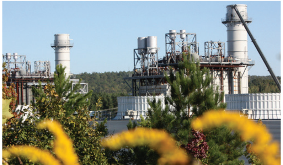
Figure 16. Hilabee Power Plant view. Alex city.
