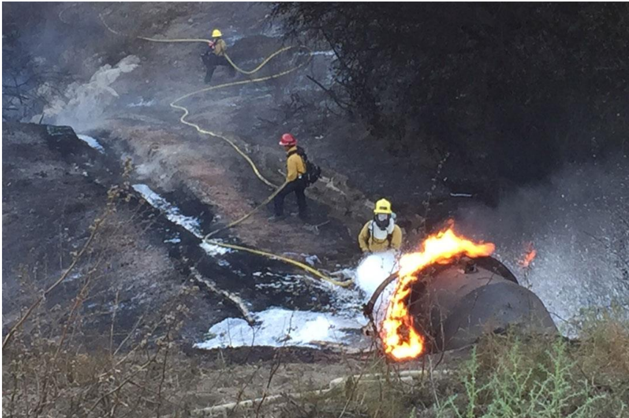
Figure 2-33: Plastic Culvert on Fire in Santa Barbara, California (Scully 2015)
