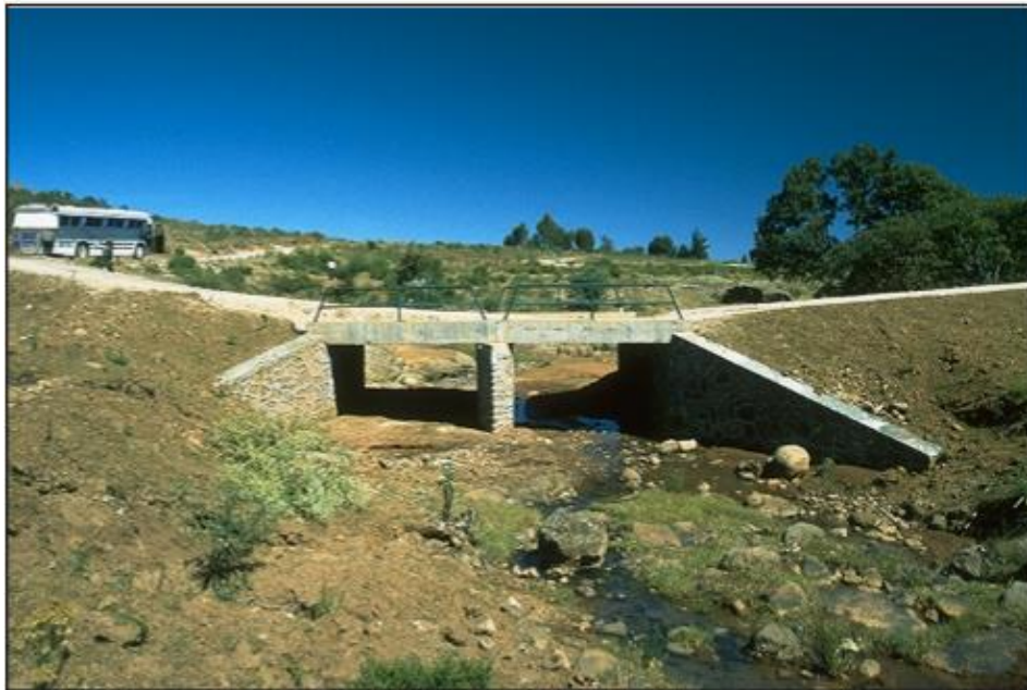
Figure 2-43: Reinforced Concrete Box Culvert (Keller 2003)
