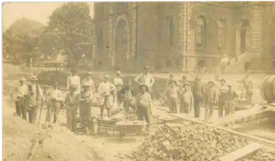
Figure 2-5: Installation of Corrugated Metal Culvert (Baldwin 2014)
