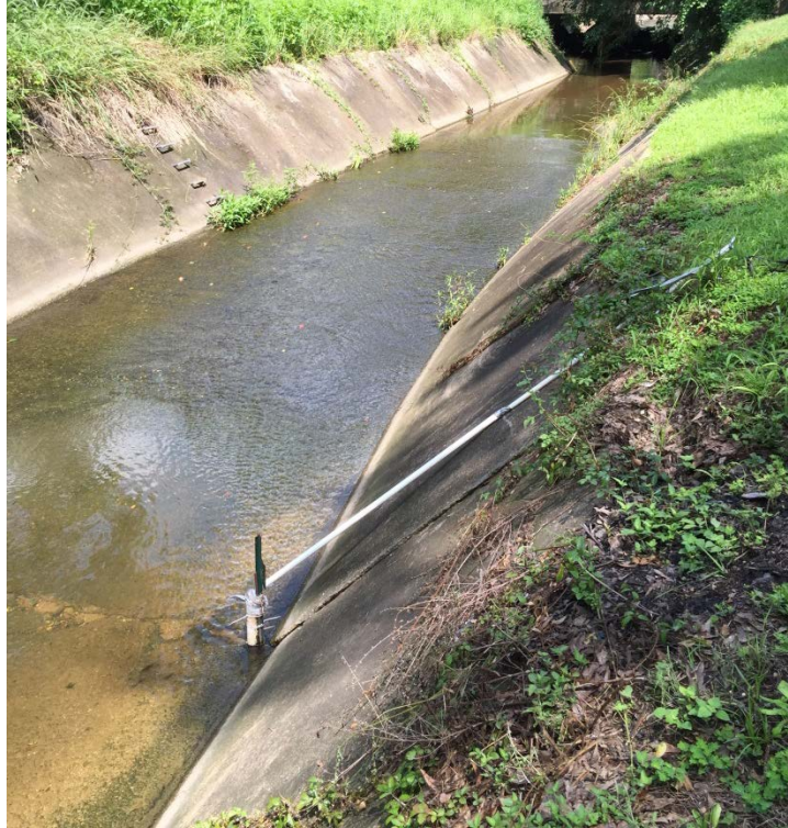
Figure 2.9: Installed pressure transducer using two-inch PVC pipes secured with the T-posts at site 5
