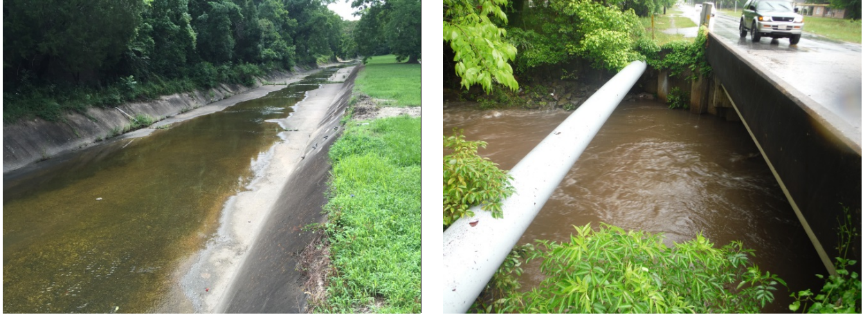
Figure 2.11: Left picture is shown in concrete channel and right picture is shown in natural stream in TSB Watershed
