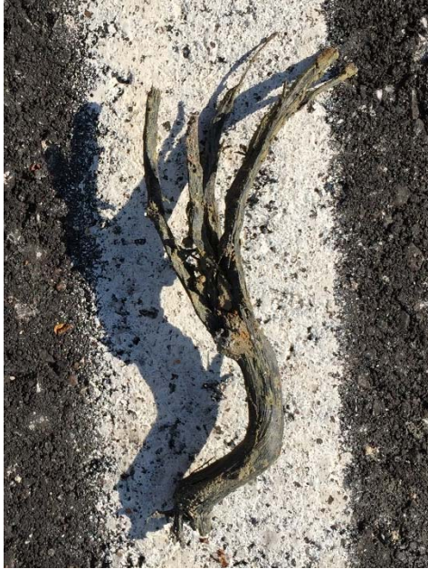
Figure 112: Tree Root Extracted from Boring Hole 4.5 (Photo Taken 5/23/16)
