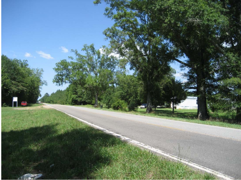
Figure 105: AL5 Facing North MP 54.22 (Photo Taken 06/16/15)
