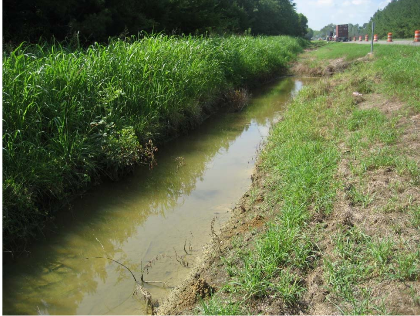
Figure 83: Standing Water Observed between Borings 1.0 and 1.5 (Photo Taken 7/10/15)
