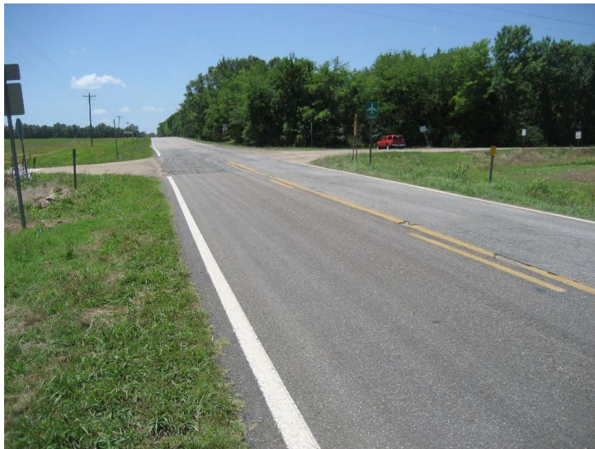
Figure 76: AL5 Facing South of Boring B3.0 MP 51.85 (Photo Taken 06/15/15)
