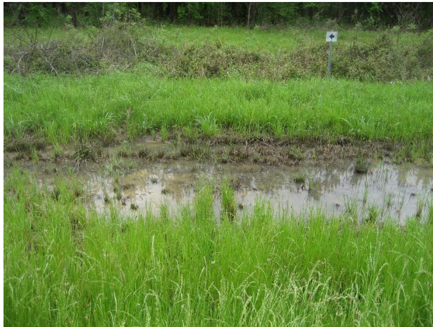
Figure 82: Standing Water Observed in Ditch (Photo Taken 4/14/2015)
