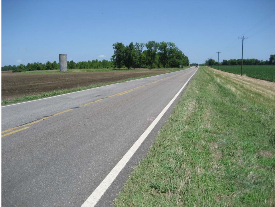
Figure 90: AL5 Facing North of Boring B3.0 MP 51.85 (Photo Taken 06/16/15)
