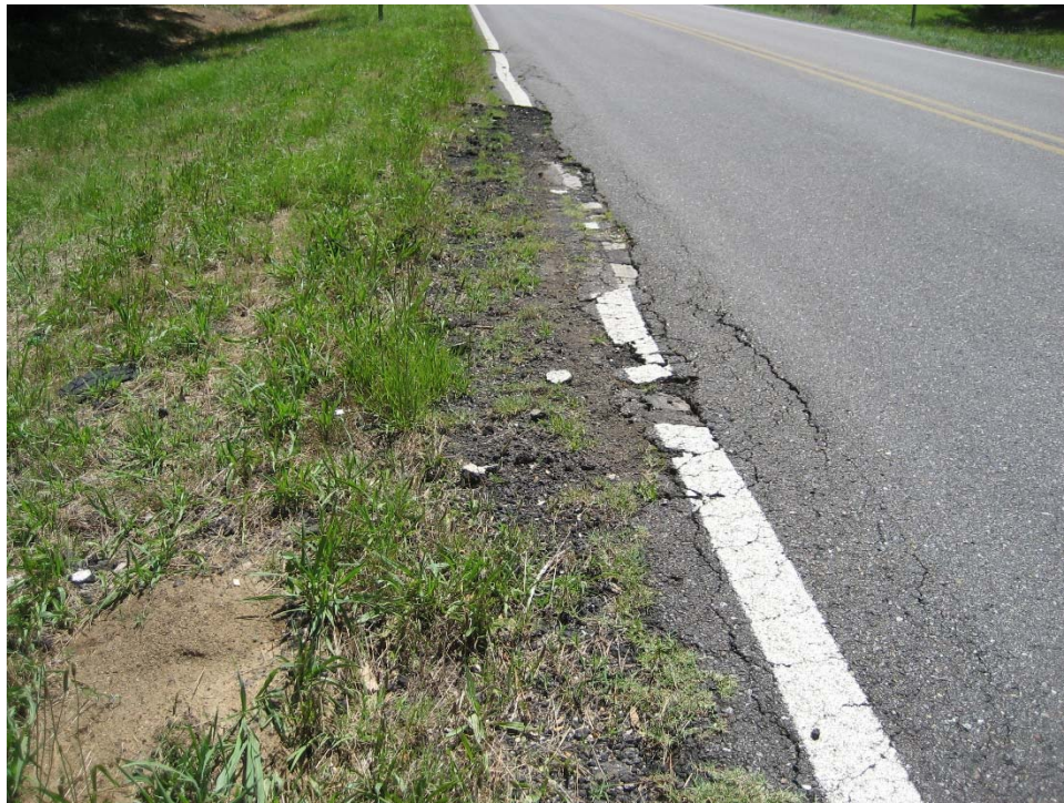
Figure 102: AL5 Facing South MP 53.52 (Photo Taken 06/16/15)
