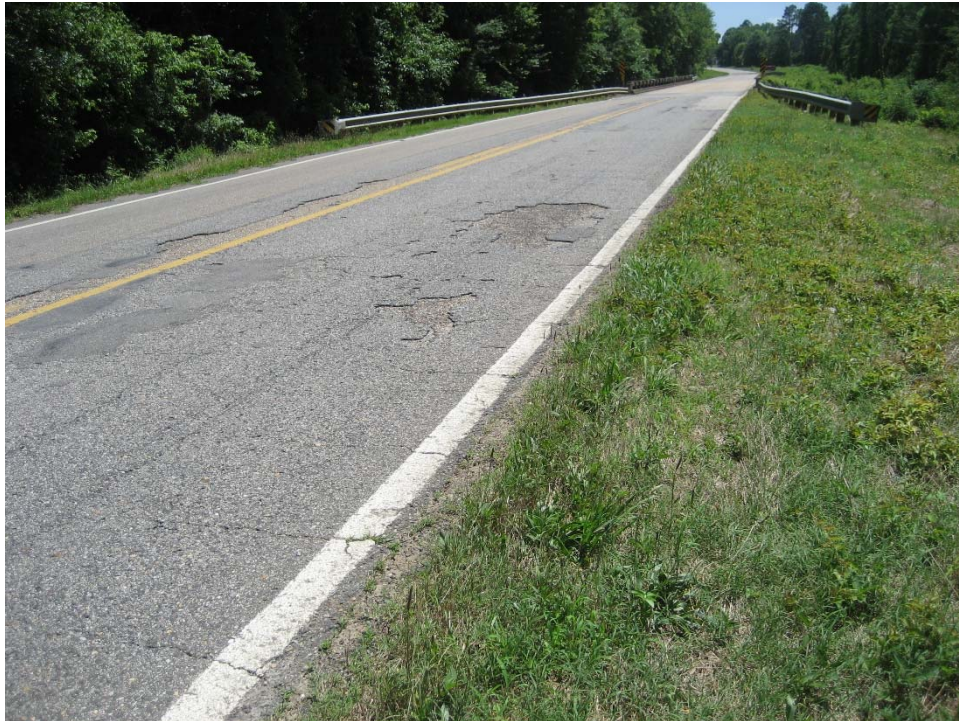
Figure 103: AL5 Southbound Approach to Bridge Facing South (Photo Taken 06/16/15)
