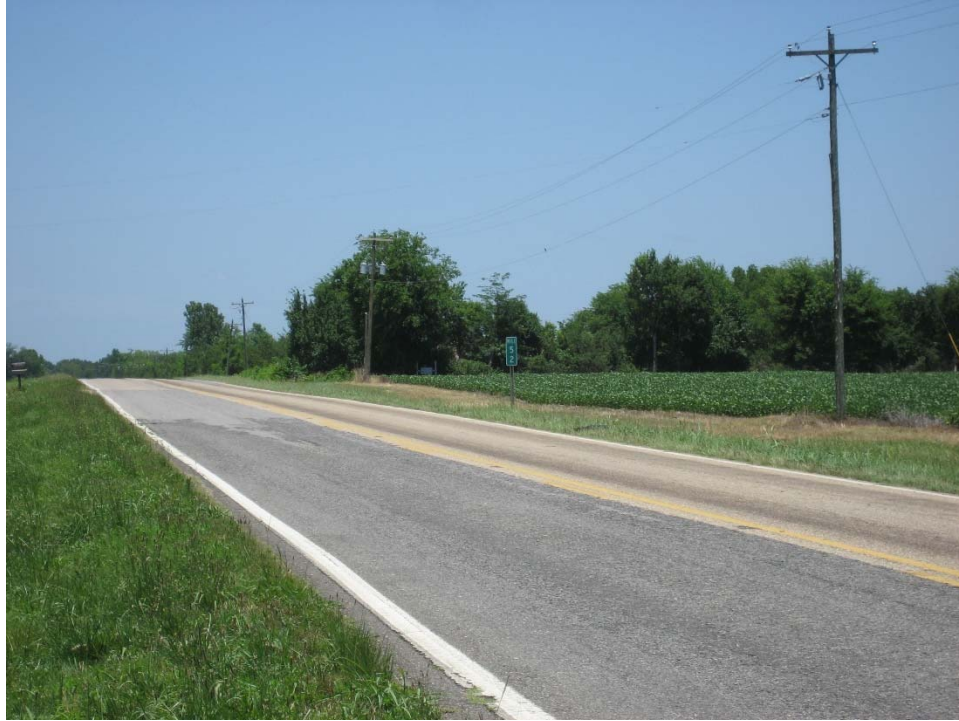
Figure 95: AL5 Facing North MP 52 (Photo Taken 06/16/15)
