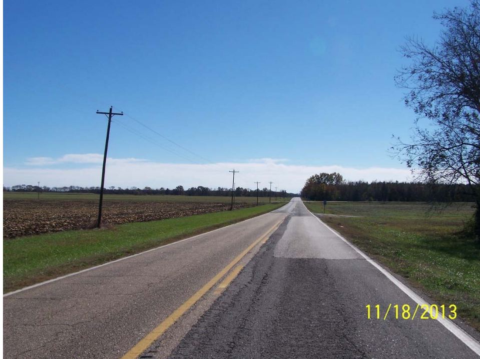
Figure 92: AL5 Facing South of MP51.915 (Photo Taken 11/18/2013)
