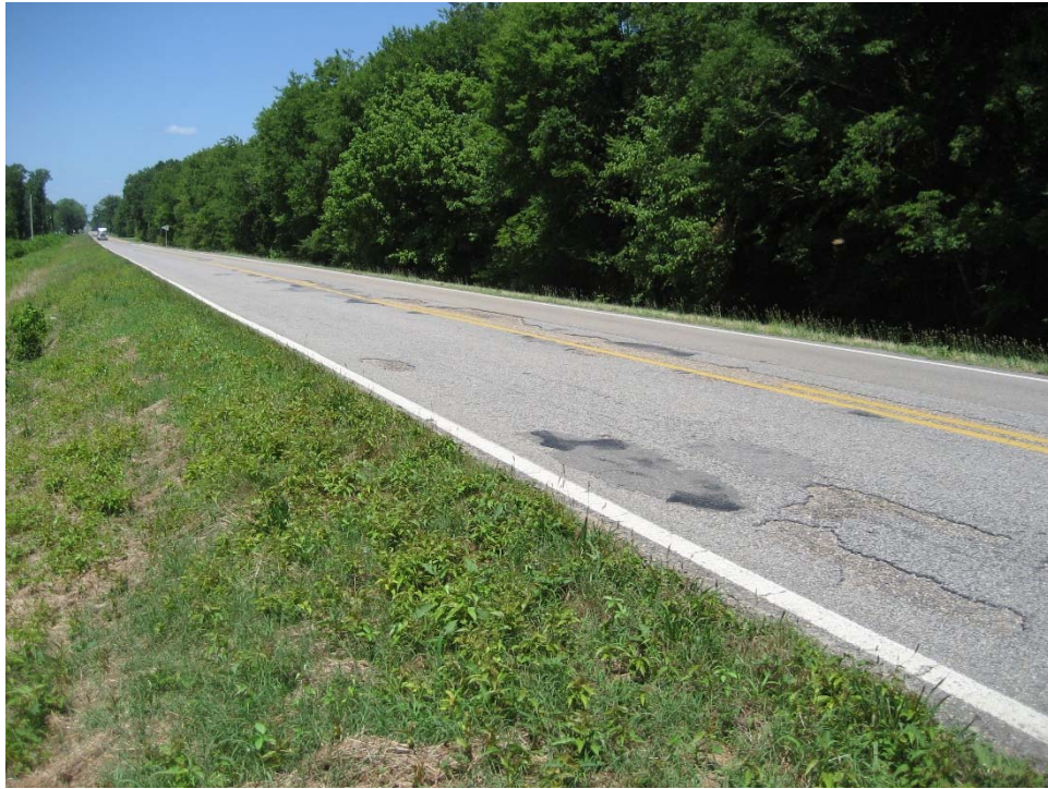
Figure 104: AL5 Southbound Approach to Bridge Facing North (Photo Taken 06/16/15)
