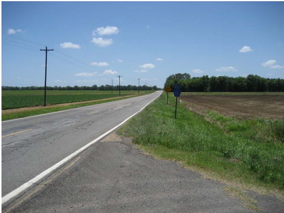
Figure 91: AL5 Facing South of MP 51.915 (Photo Taken 06/16/15)
