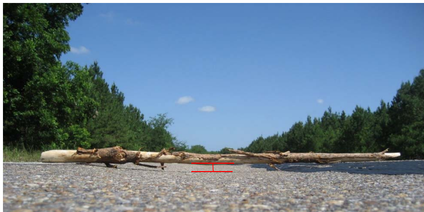
Figure 86: Observed Rutting
