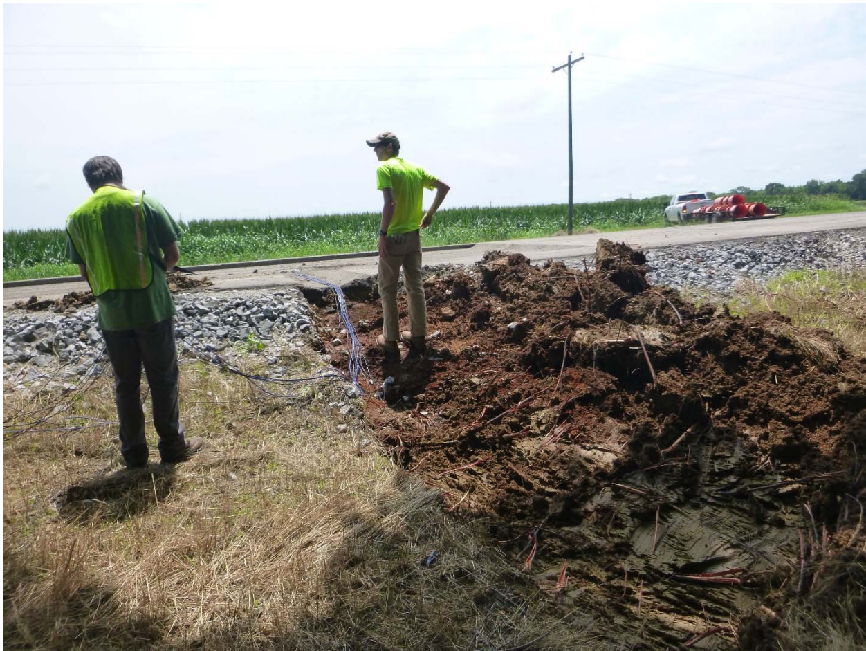
Figure 110: Tree Roots Observed During Installation of Sensors (Photo Taken 06/28/16)
