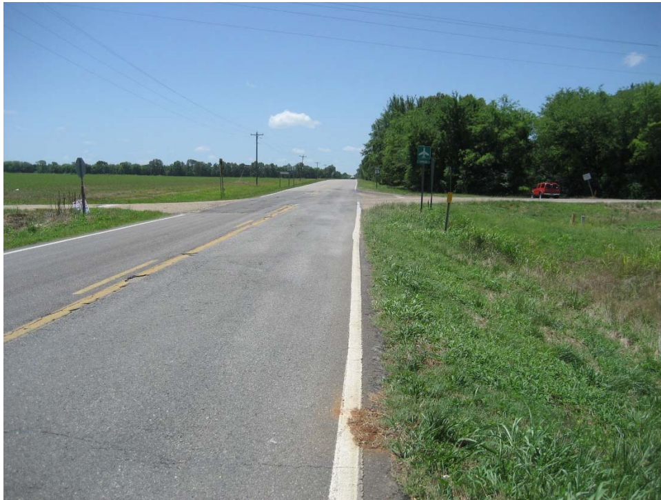
Figure 89: AL5 Facing South of Boring B3.0 MP 51.85 (Photo Taken 06/16/15)
