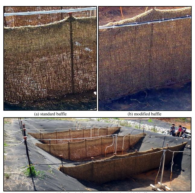
(c) modified first baffle vs. standard second and third baffles
