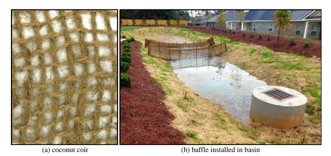
Figure 2.1 Sediment Basin Baffles.
