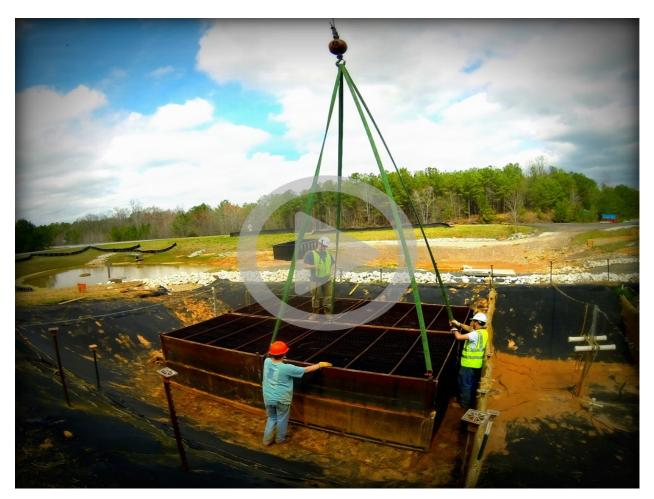
Video 4.5 Removal and Re-Installation of Lamella Plates in Parallel Flow Configuration.
