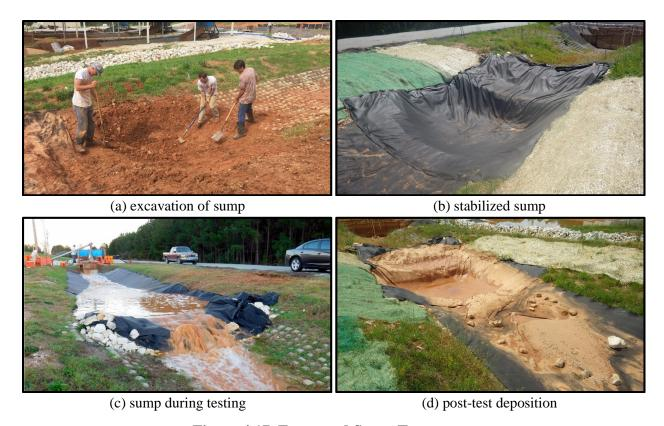
Figure 4.17 Excavated Sump Treatment.
