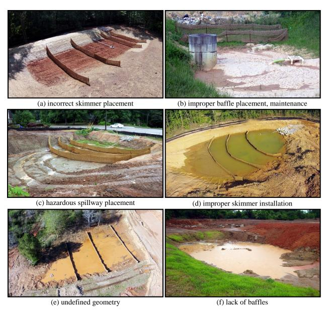
Figure 2.7 Poorly Designed and Constructed Sediment Basins.
