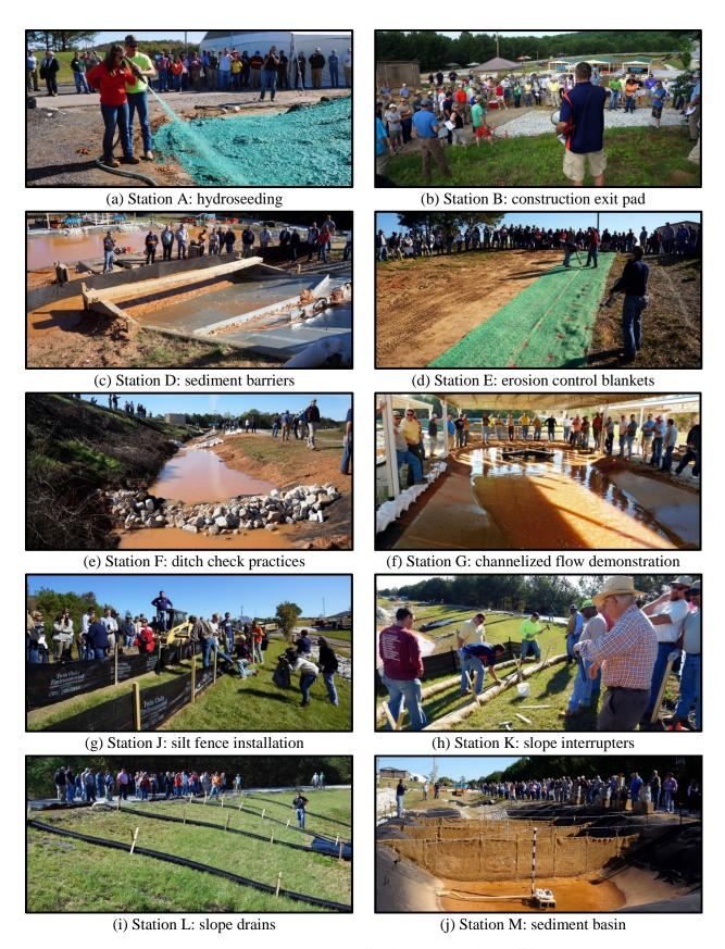
Figure 6.2 Demonstration Stations at the AU-ESCTF.
