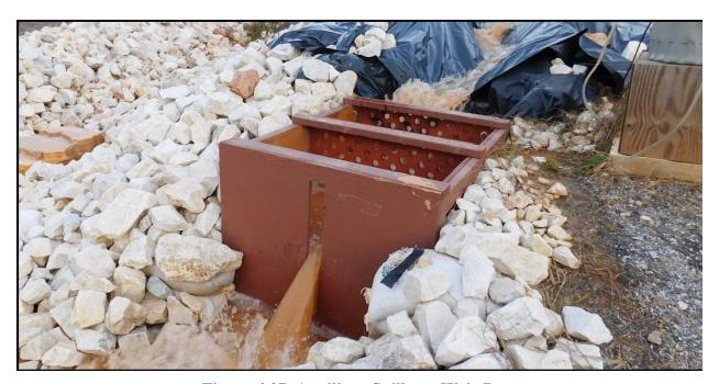
Figure 4.27 Auxiliary Spillway Weir Box.
