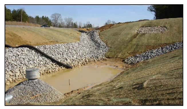
Figure 2.4 Perforated Riser Structure in ALDOT Sediment Basin.
