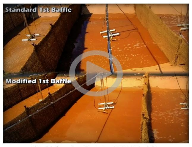
Video 4.7 Comparison of Standard and Modified First Baffle.
