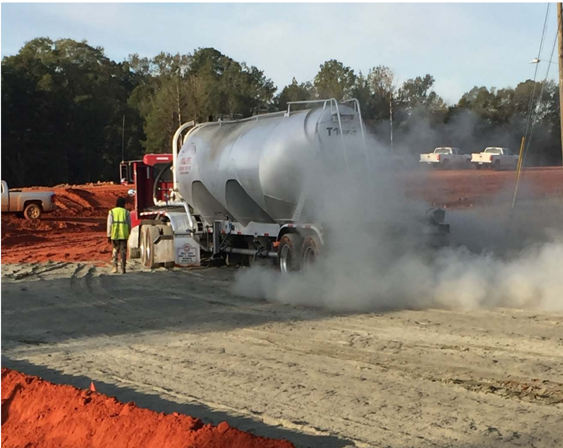
Figure 2.1: Cement truck with mechanical spreader used to place cement
