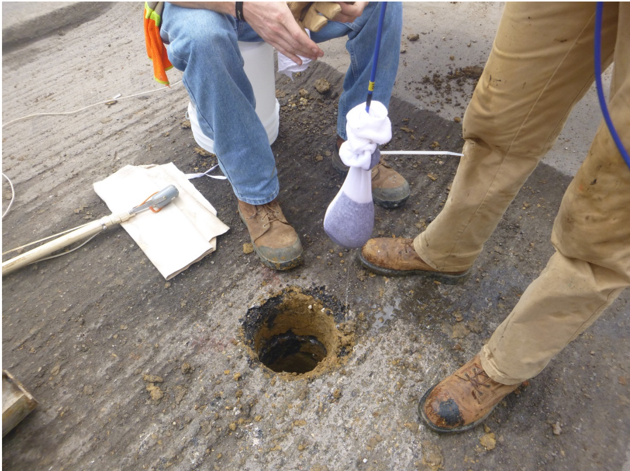
Figure 68: Piezometer in Sand-Filled Bag being Lowered Down the Borehole
