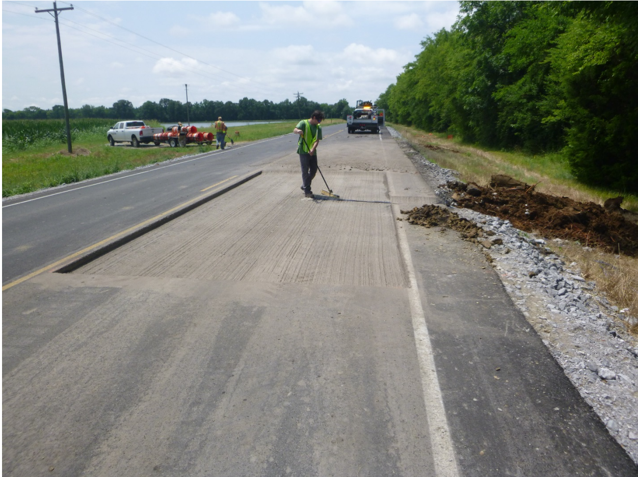
Figure 73: Section Milled and Cleaned for placement of ASG Array
