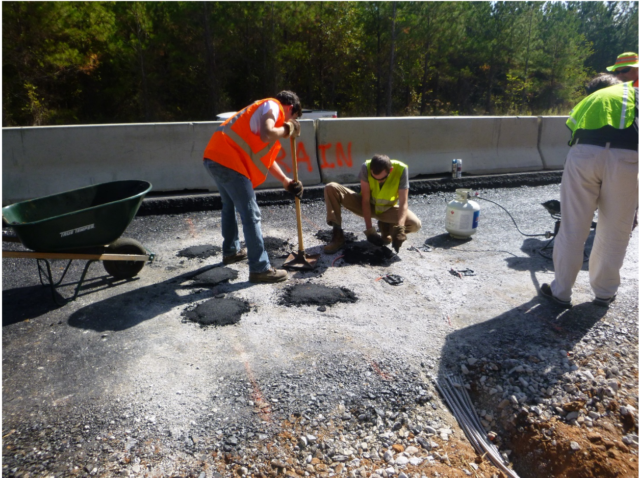
Figure 72: Screened Asphalt being Placed and Compacted over Gages
