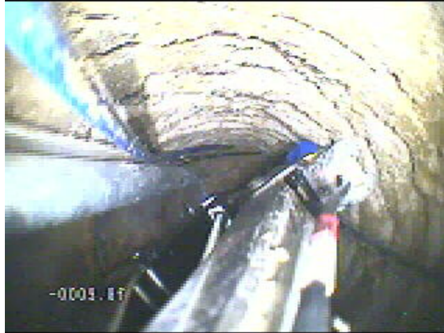
Figure 65: Fully Installed Moisture Sensor
