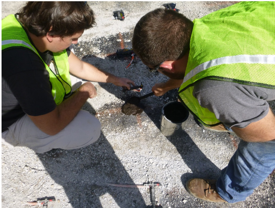
Figure 71: ASGs being Tacked with Tack-Sand Mixture
