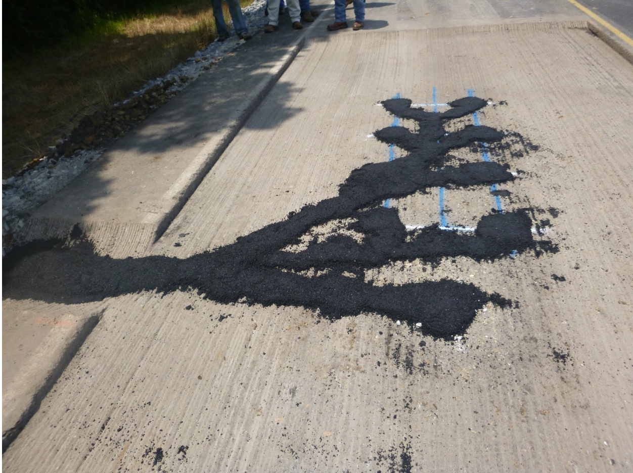
Figure 74: Gage Array on Milled Surface Covered with Screened Asphalt
