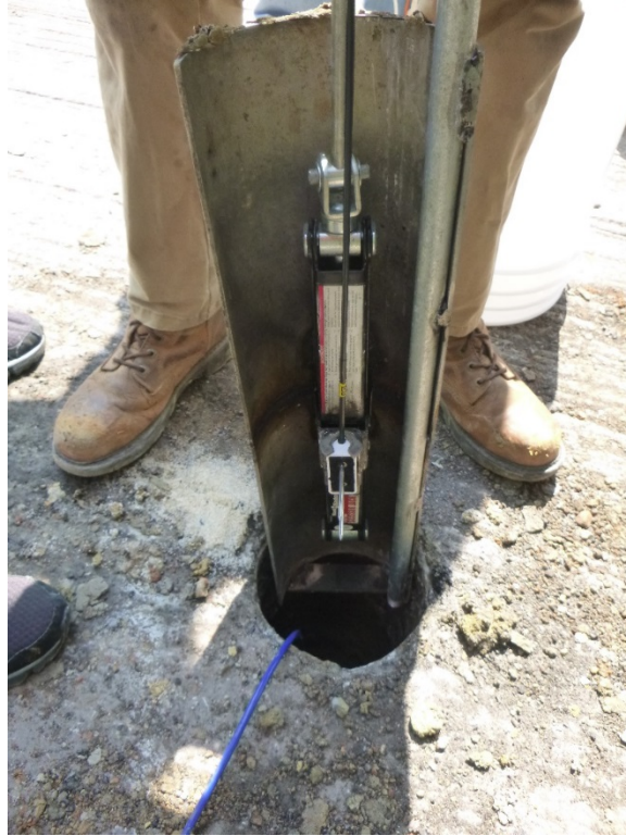
Figure 63: Moisture Sensor and Installation Tool being Lowered down Borehole
