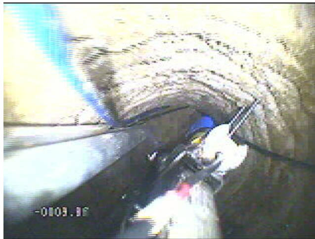
Figure 64: Moisture Sensor Installation
